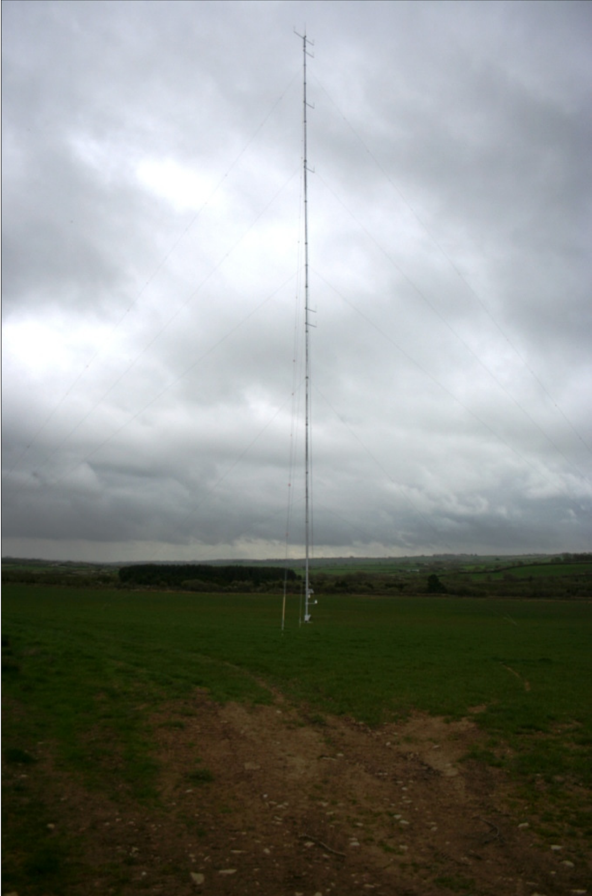
Fig 3 Anemometer mast with stays down to anchor points (looking SE)
