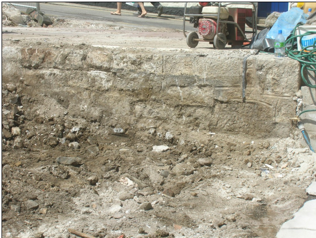
Figure 6. Granite faced wall and quoin stones. Possible part of 19 th century cottages on this site prior to building of the Day Care Centre.
