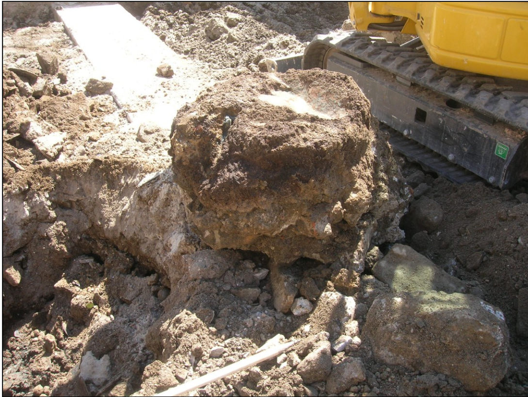
Figure 5. Stone and concrete capping of shaft, here inverted after removal
