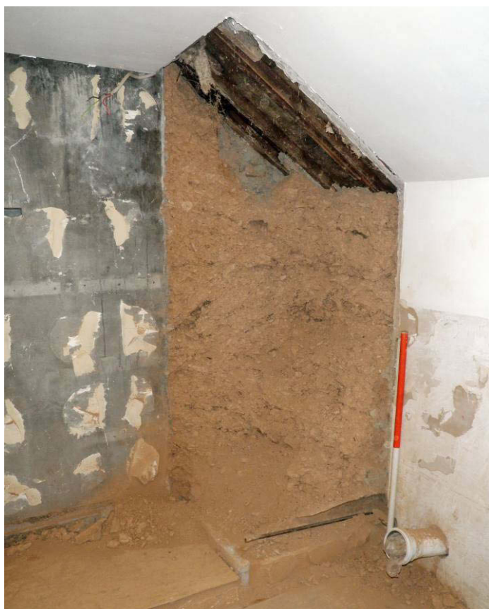
Fig 8 Corner of bathroom during removal of cob wall
