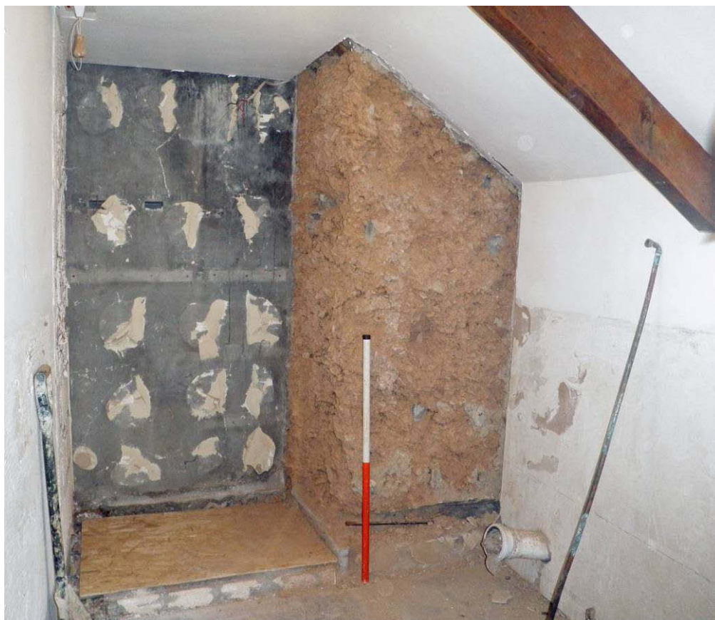
Fig 7 Remaining section of cob wall in bathroom before removal
