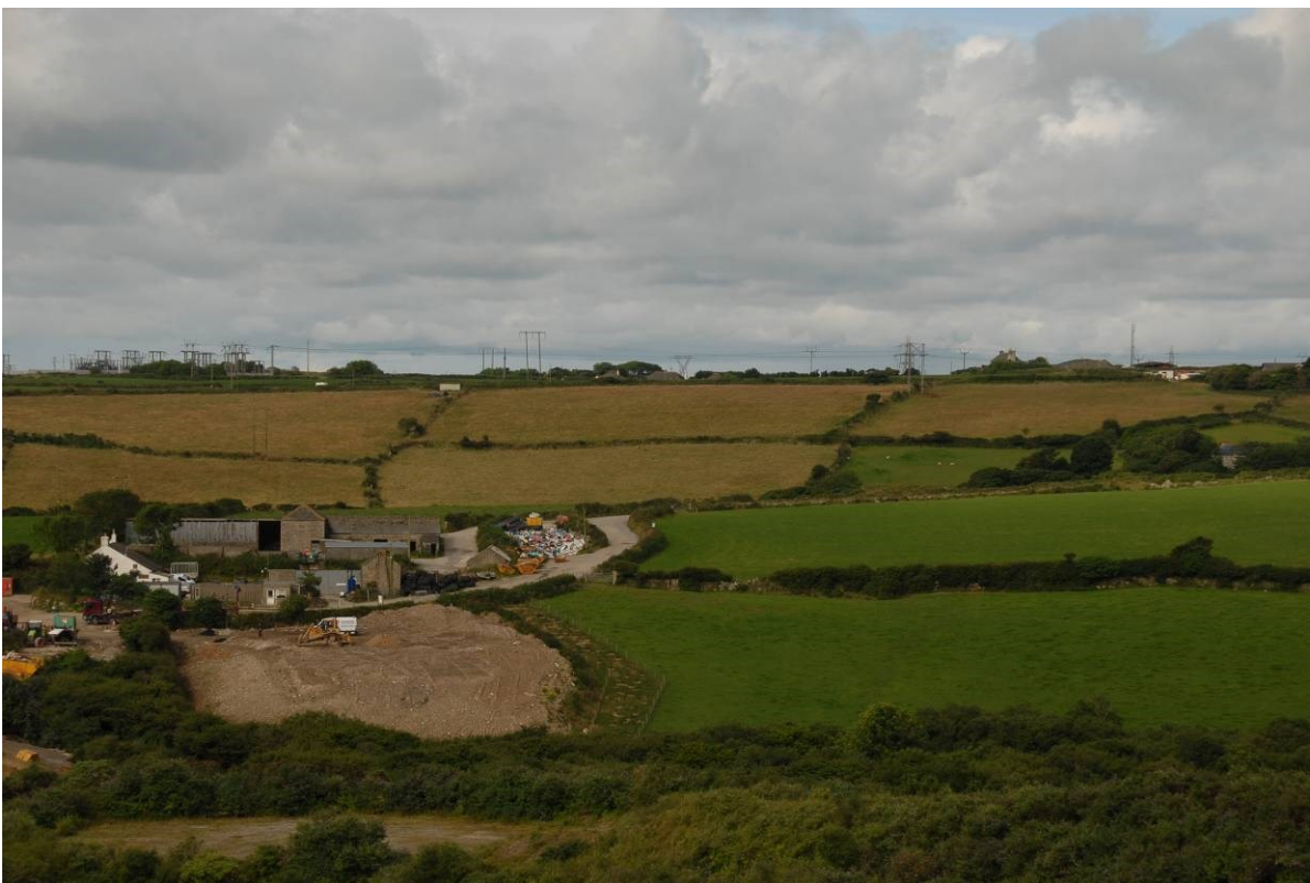
Fig 26. Looking east south east from Kessel Downs quarry towards Herniss Farm with the Rame transformer station on the skyline.
