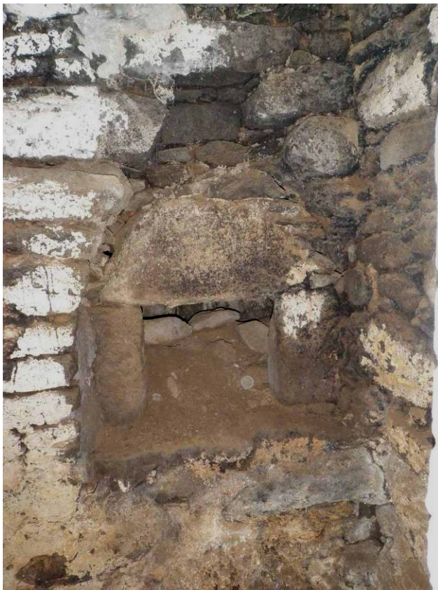
Fig 24 Stone-lined oven in the cottage fireplace
