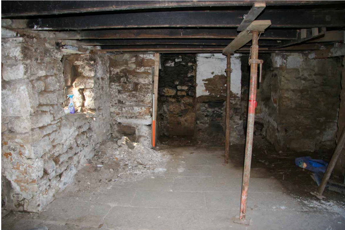
Fig 19 Ground floor interior of the cottage
