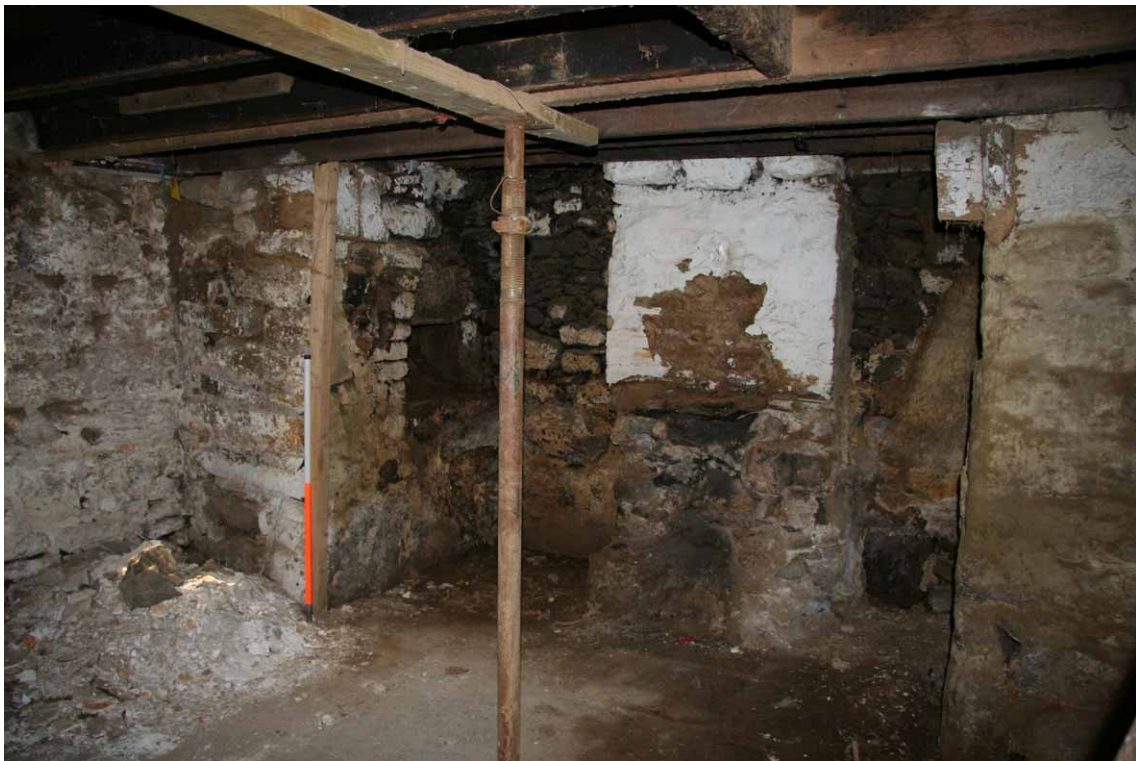
Fig 20 Cottage fireplace (with inserted central flue for washhouse)
