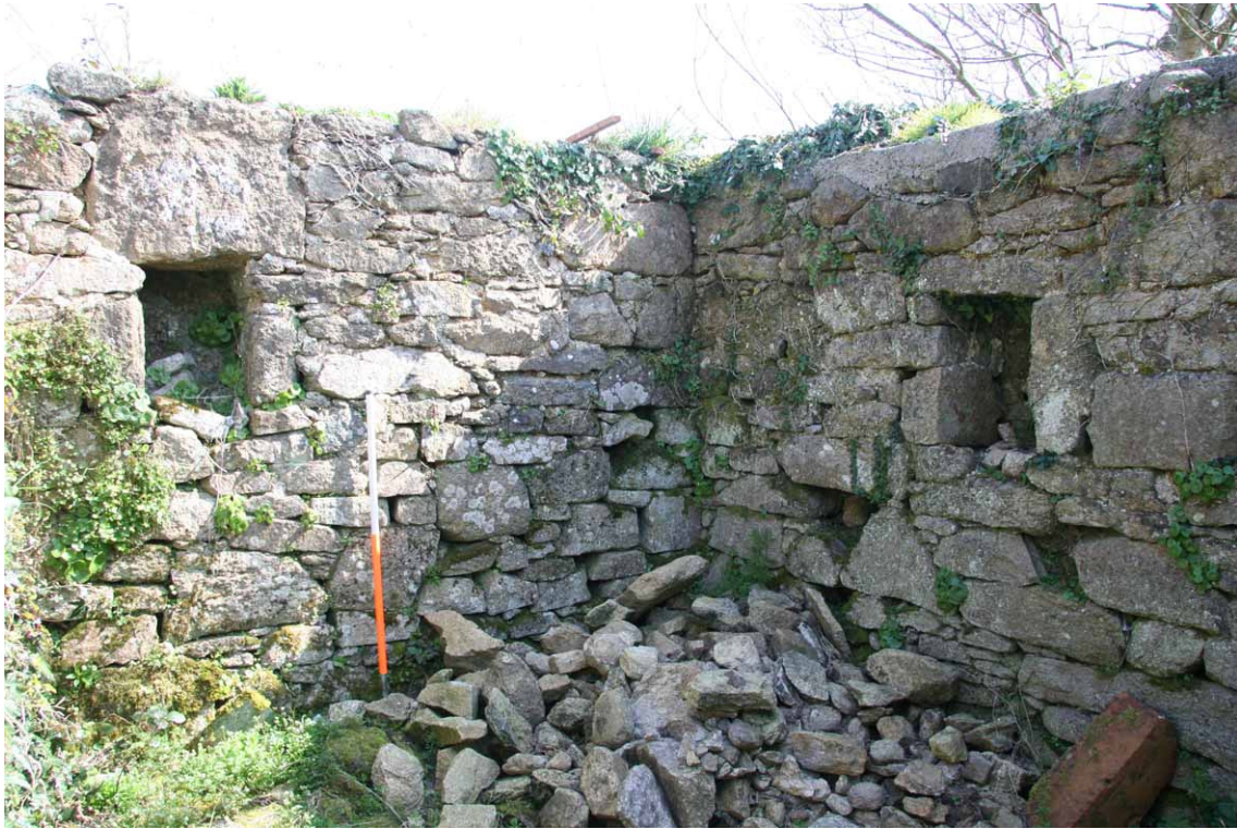
Fig 31 Bee hole recesses in earlier farmyard wall, later incorporated within Piggery 2
