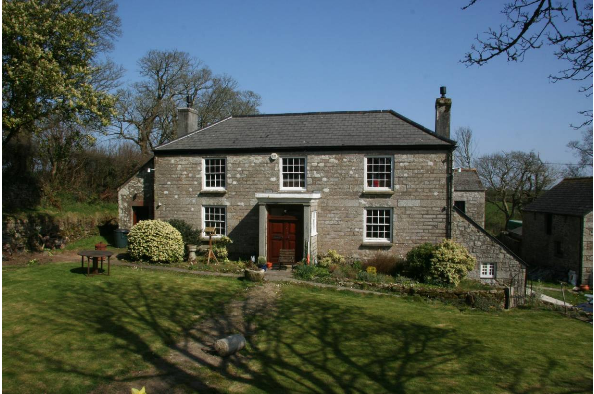
Fig 7 The gardens and front of Helland House, viewed from the west.
