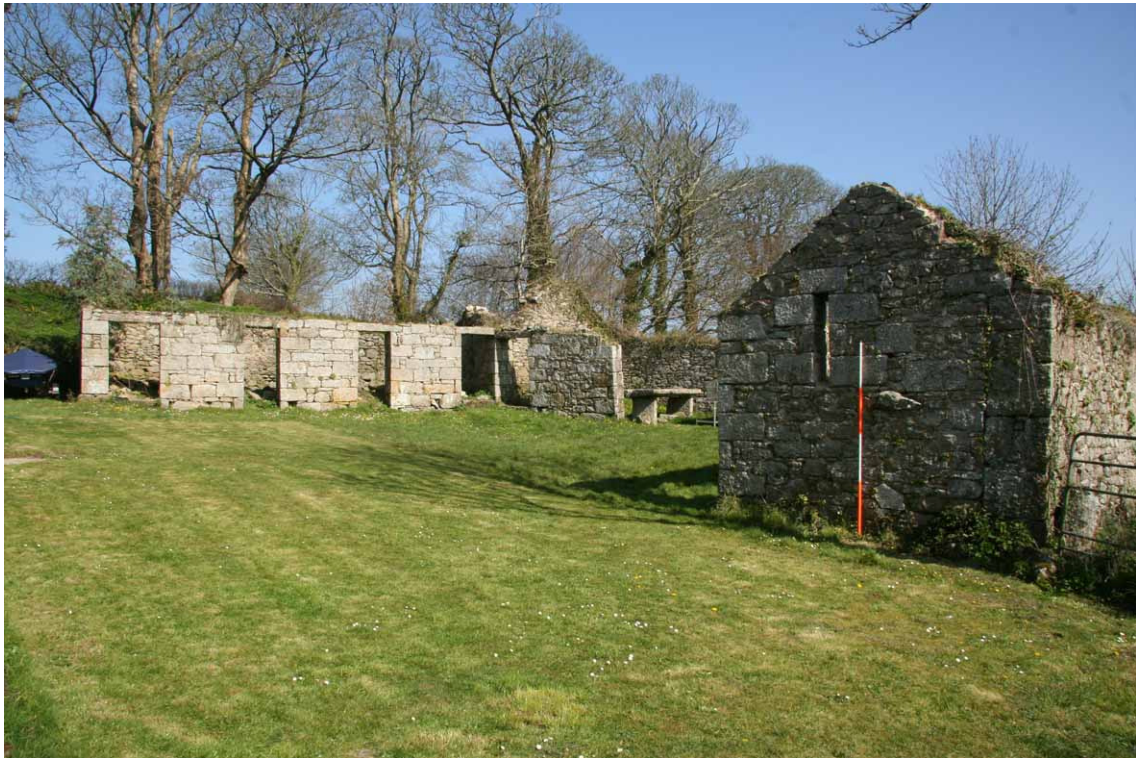
Fig 27 SW view of the former farmyard and piggeries
