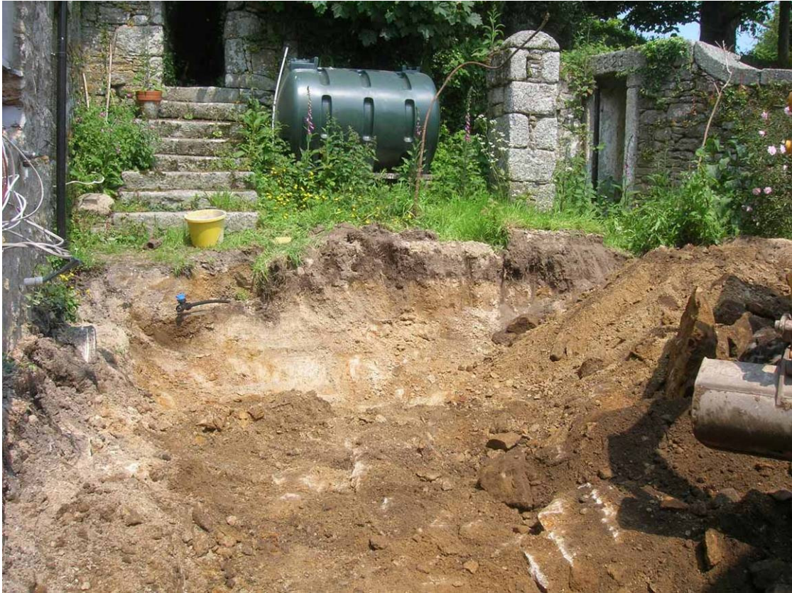
Fig 33 Soil profile within the garden area, revealing topsoil/garden soil immediately above natural decomposed granite
