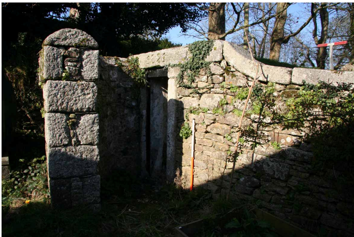
Fig 14 Granite-built earth closet, with date 1821 cut into lintel Its construction appears to be integral with the coping on the kitchen garden wall
