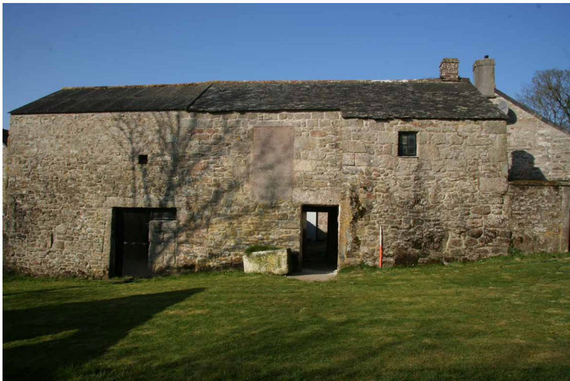
Fig 18 View of rear of cottage (right and centre) and stable (left) from the farmyard
