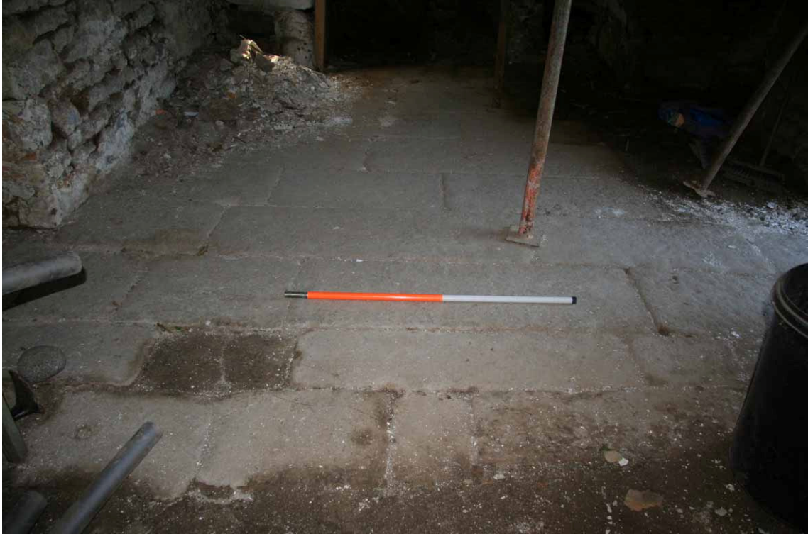
Fig 21 Granite paved floor of the cottage
