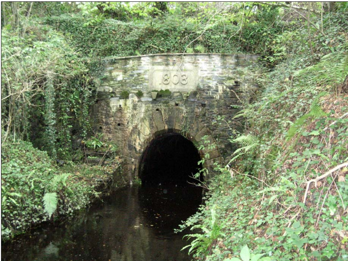
Fig 8 A view of the Tavistock Canal west tunnel portal © CC HE Projects 2002
