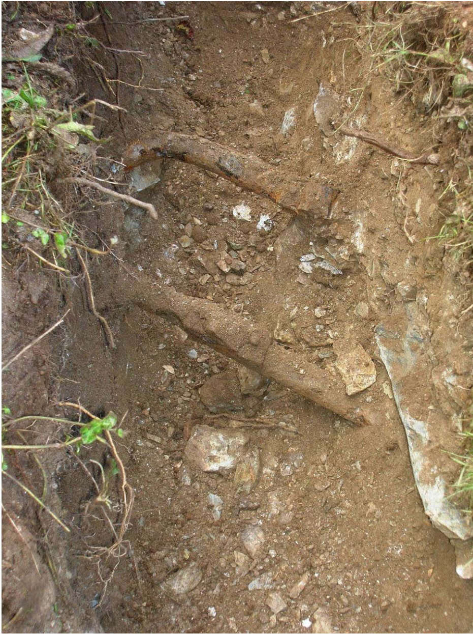
Fig 4 Armoured cable ducts at southern end of trench.
