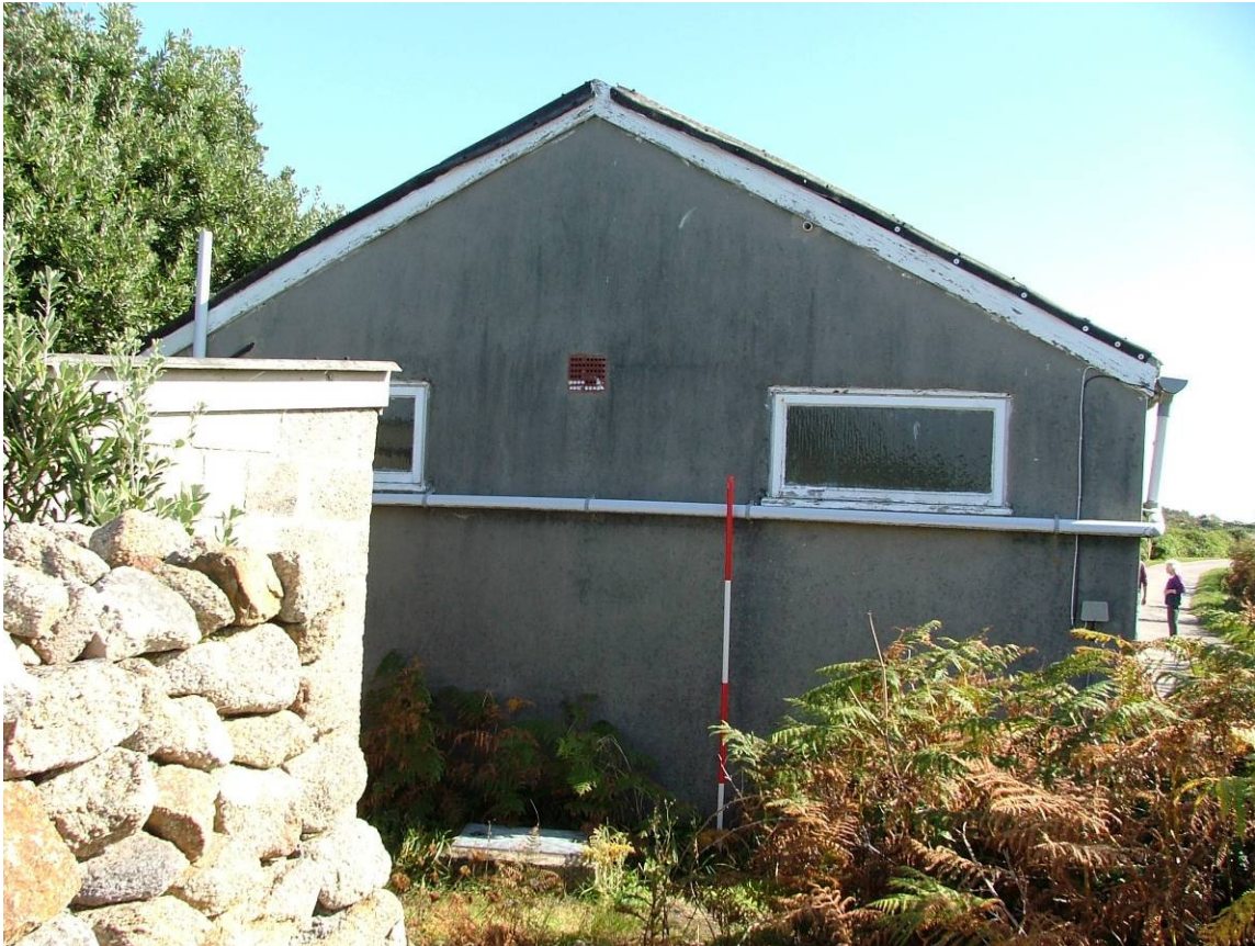
Fig 8 West elevation 1 October 2012 (photo: Katharine Sawyer)
