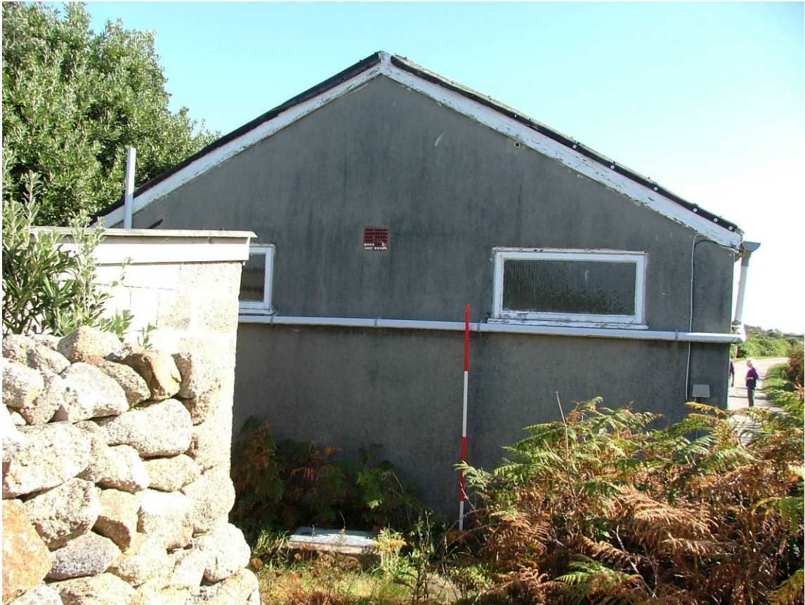
Fig 8 West elevation 1 October 2012 (photo: Katharine Sawyer)
