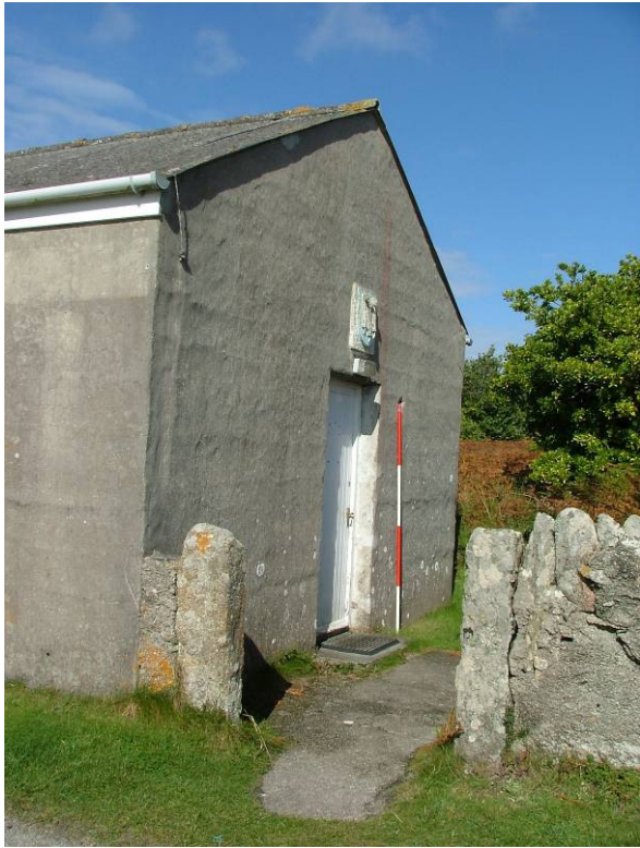
Fig 9 East elevation, 1 October 2012 (photo: Katharine Sawyer)
