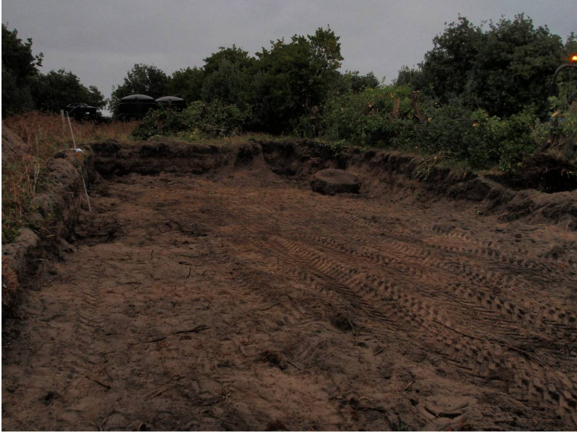
Fig 13 The site during soil stripping, 6 November 2012 (photo: Cornwall Council)
