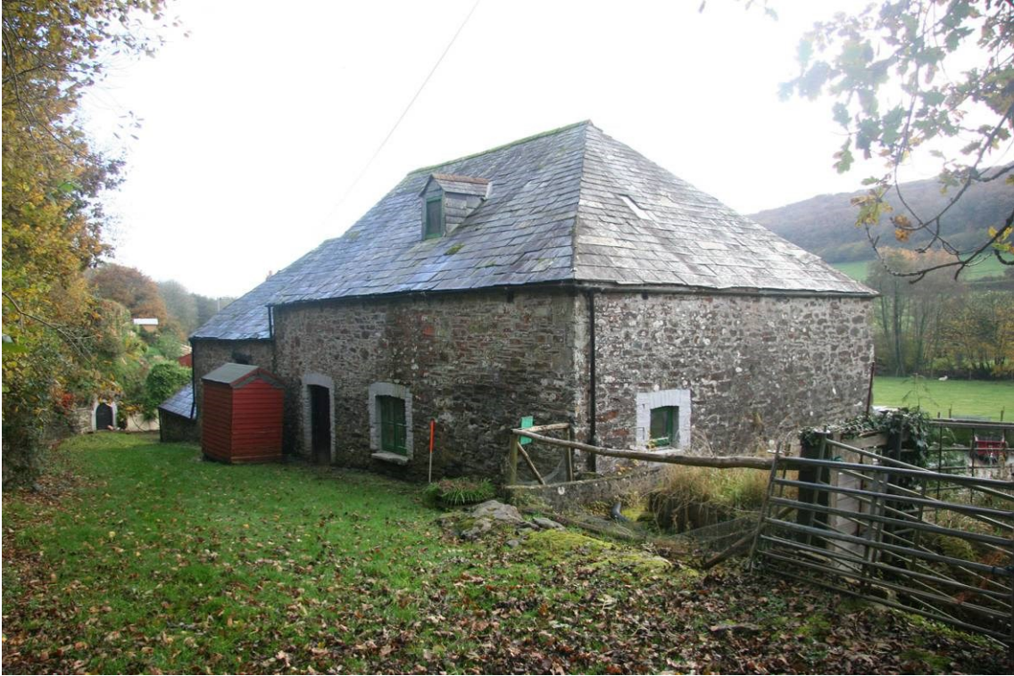
Fig 9 View from the northwest, showing the leat (to right) approaching the mill
