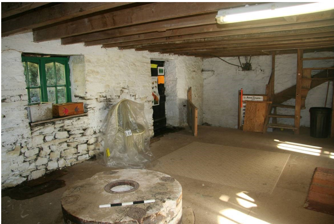
Fig 30 View of the first floor with original winder stairs to the loft at the rear A second pair of millstones was once sited in the position of the square mat
