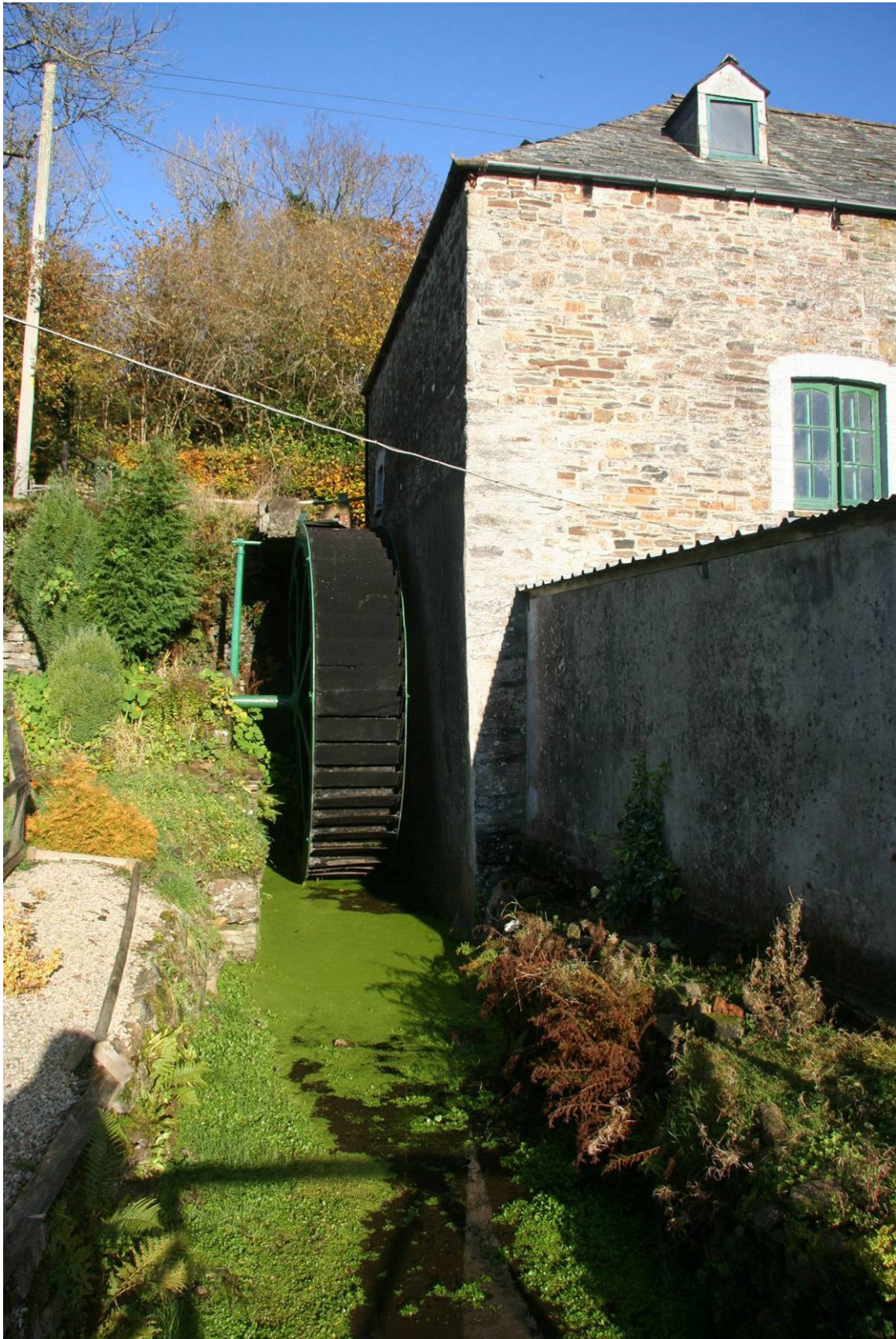
Fig 15 Waterwheel, wheel-pit and tailrace
