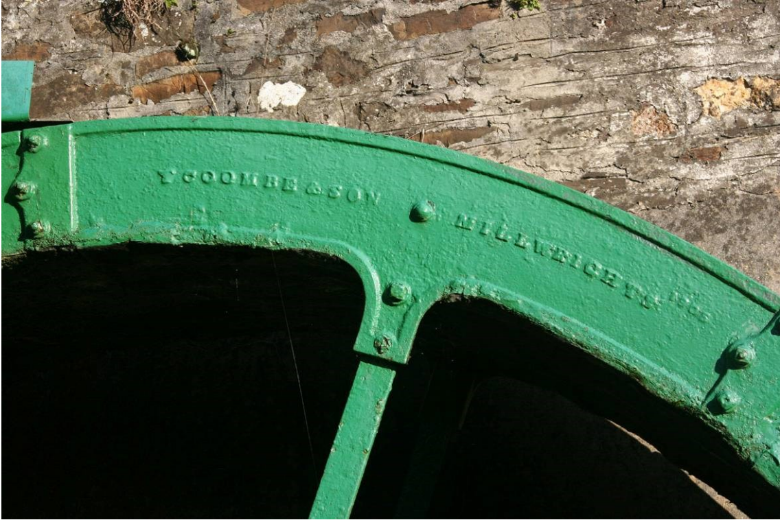
Fig 16 Waterwheel shroud, embossed 'T COOMBE & SON MILLWRIGHTS 1905'
