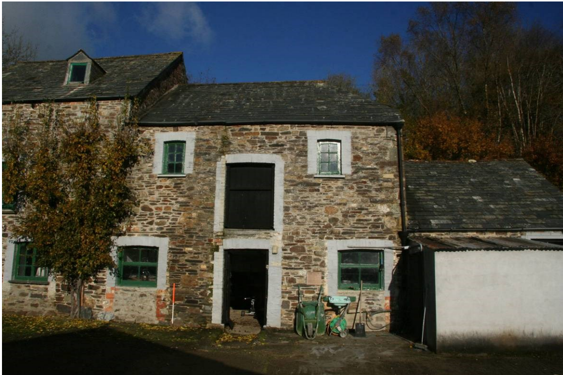
Fig 11 Front (south) elevation of the main shippon and loft/barn
