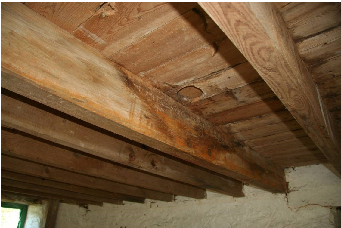
Fig 34 Hole in the loft floor where grain was once channelled into a hopper above the millstone
