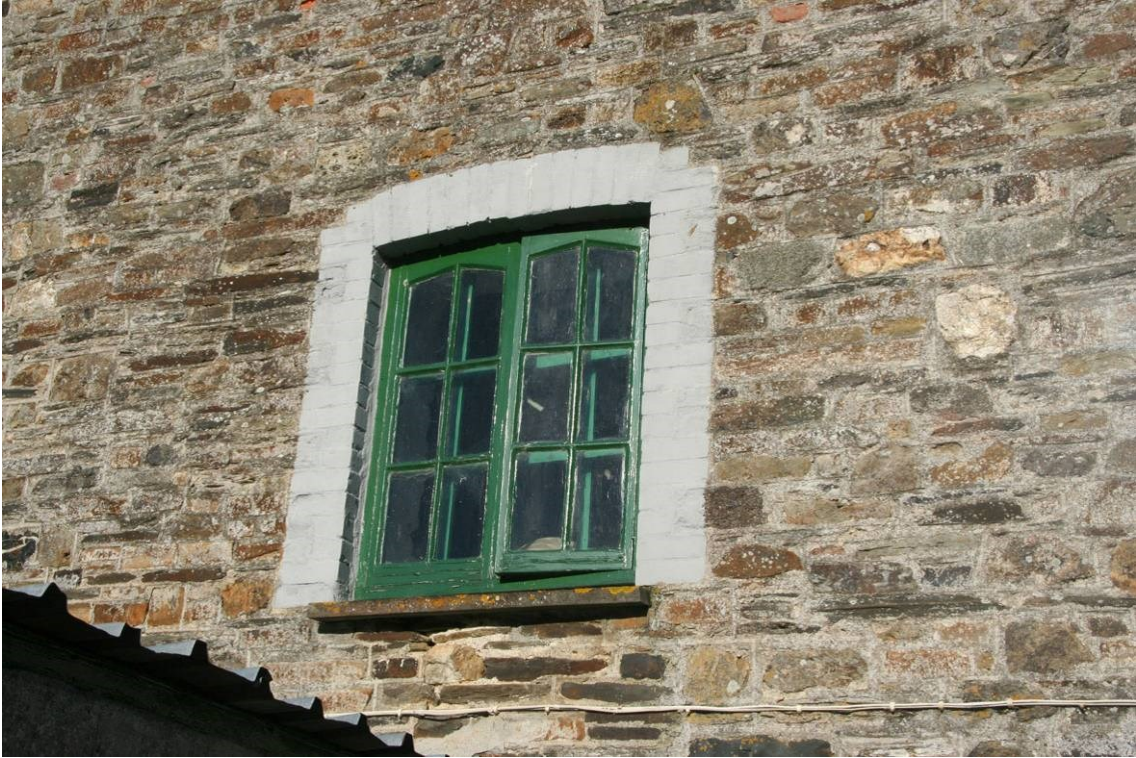
Fig 13 Upper floor window of mill, probably original to the 1905 reconstruction
