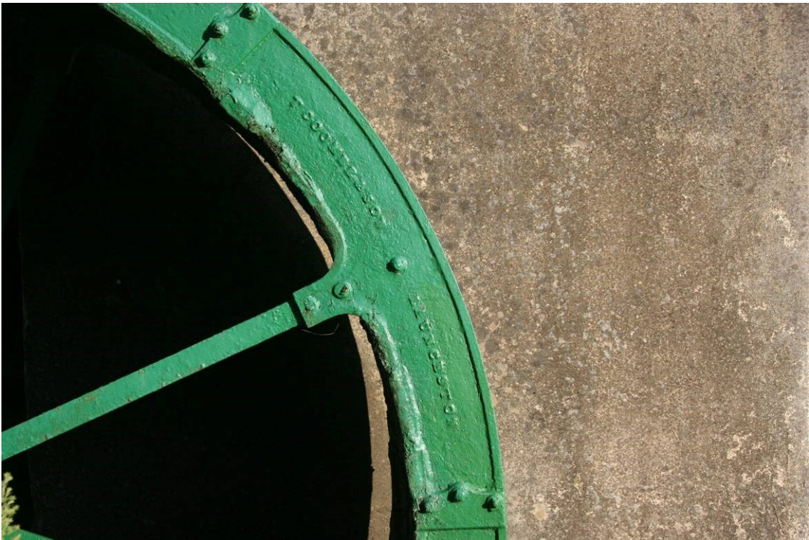
Fig 17 Waterwheel shroud, embossed 'T COOMBE & SON LAUNCESTON'
