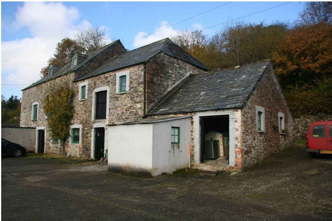
Fig 8 Shippon with loft and loosebox attached to New Mills
