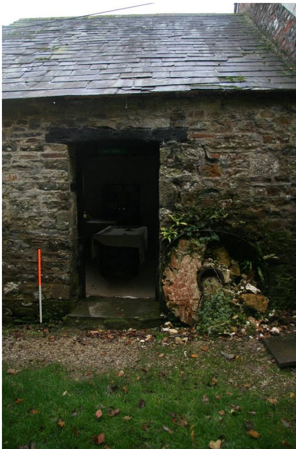
Fig 12 Rear doorway into the loft/barn above the shippon
