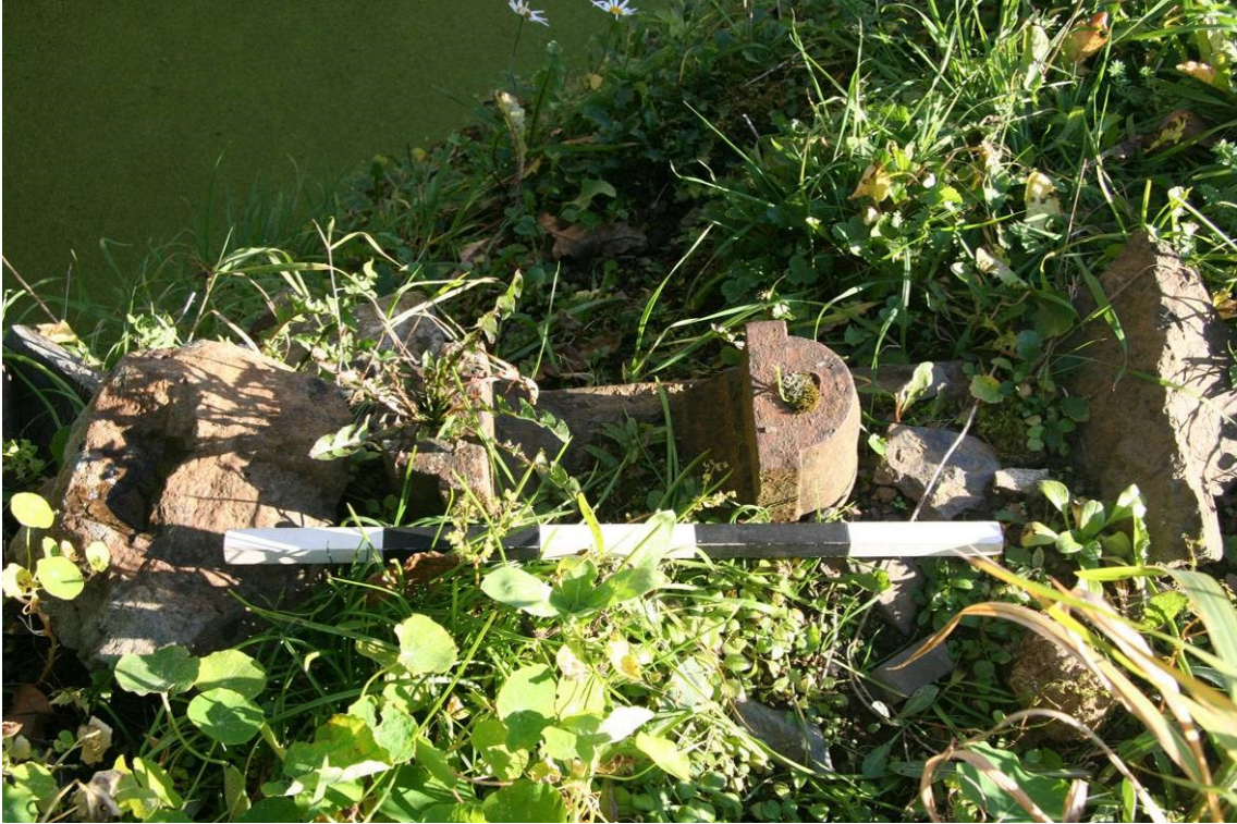
Fig 20 Displaced bottom casting of an axle bearing
