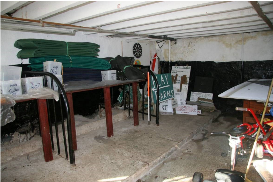
Fig 42 Ground floor of the main shippon, showing the 20 th century steel bays and feed troughs when the building was used as a milking parlour
