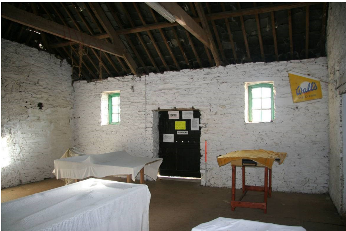
Fig 40 Another view of the loft/barn above the shippon
