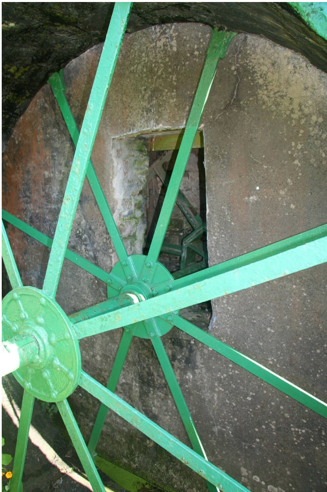
Fig 18 View of wheel hubs and spokes, with pit-wheel inside
