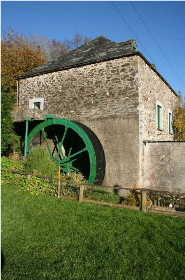
Fig 10 The west elevation of the mill with the launder and waterwheel
