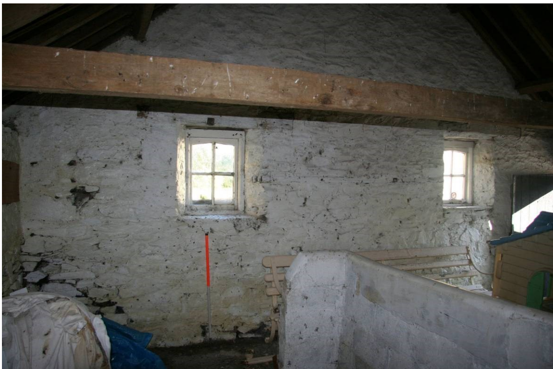
Fig 44 Subsidiary loosebox/shippon, showing reused timber lintels above the windows
