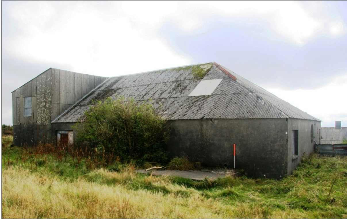
Figure 27 A view from the north of the diesel engine house (Site 7) © CC HE Projects
