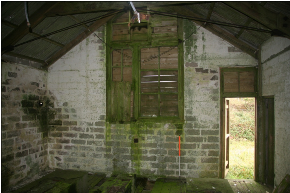
Figure 14 Internal view of the winding engine house (Site 3.1) © CC HE Projects
