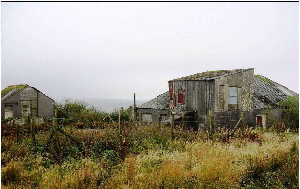
Figure 16 South Shaft complex in 2012. The ore-bin, shaft headgear and chimney have all gone (© CC, HE Projects)
