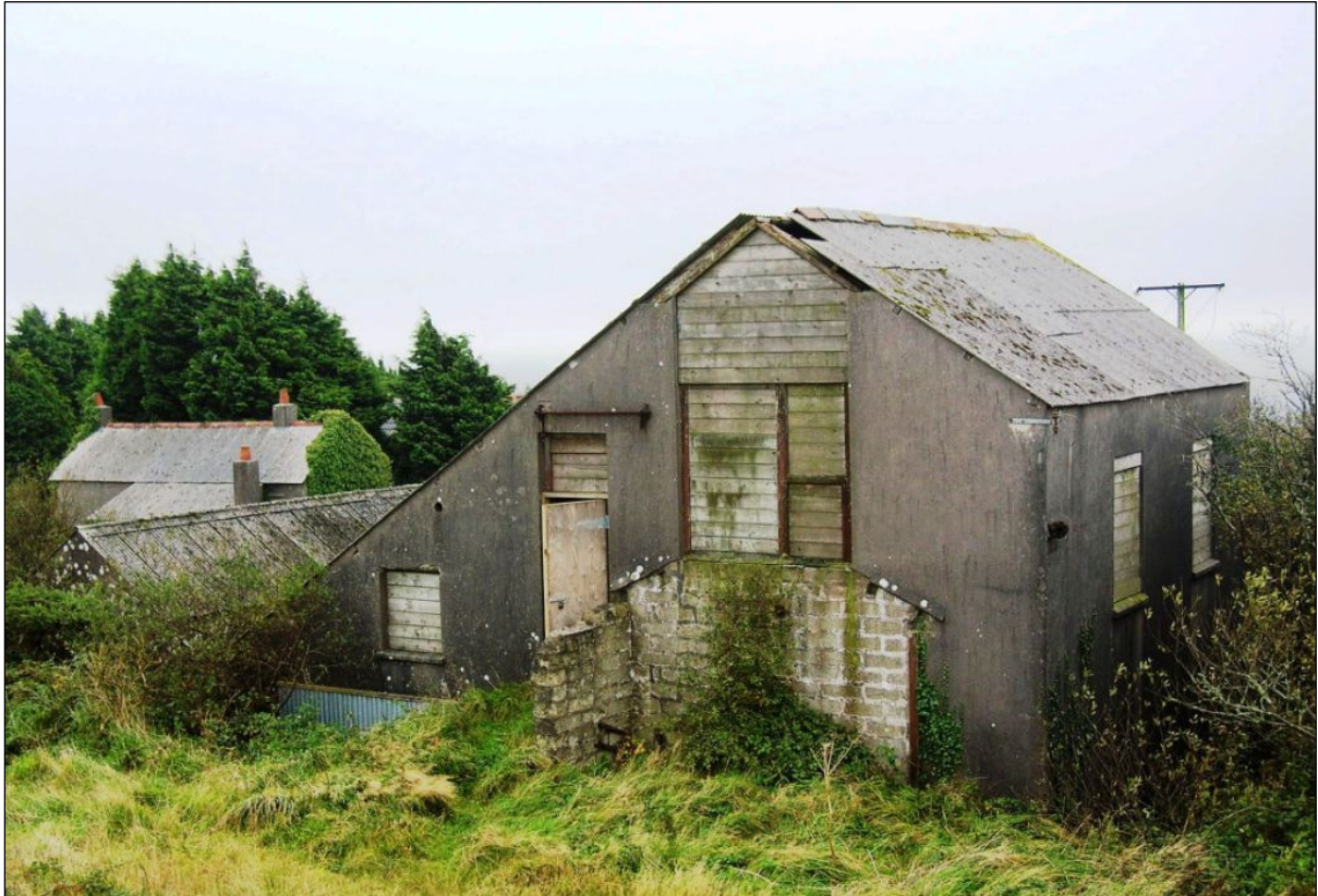
Figure 24 The winding engine house (Site 3.1), boiler house (Site 3.2), and auxiliary boiler house (Site 4) from the north (© CC HE Projects).
