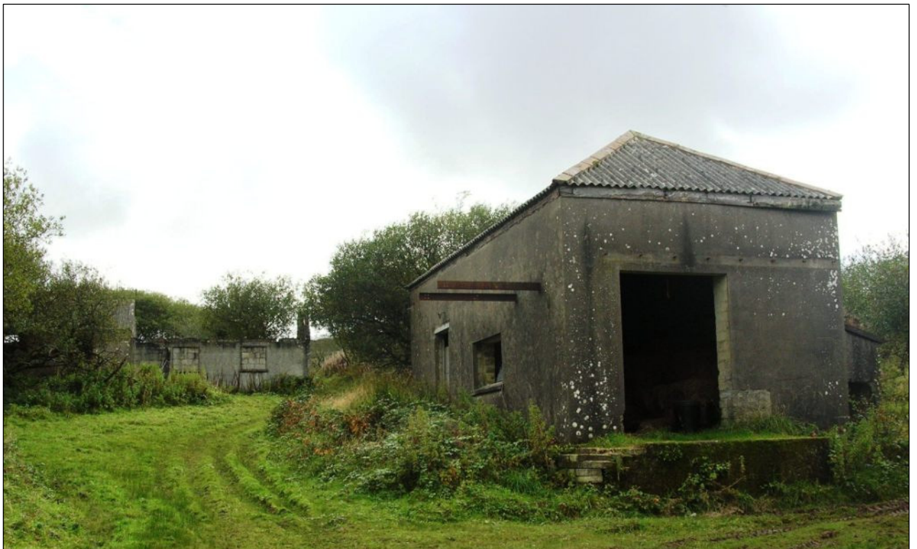
Figure 8 North Shaft complex in 2012. (Later) Diesel Mill engine house (Site 45) in foreground, Miners' Dry (Site 43) in background (© CC HE Projects)
