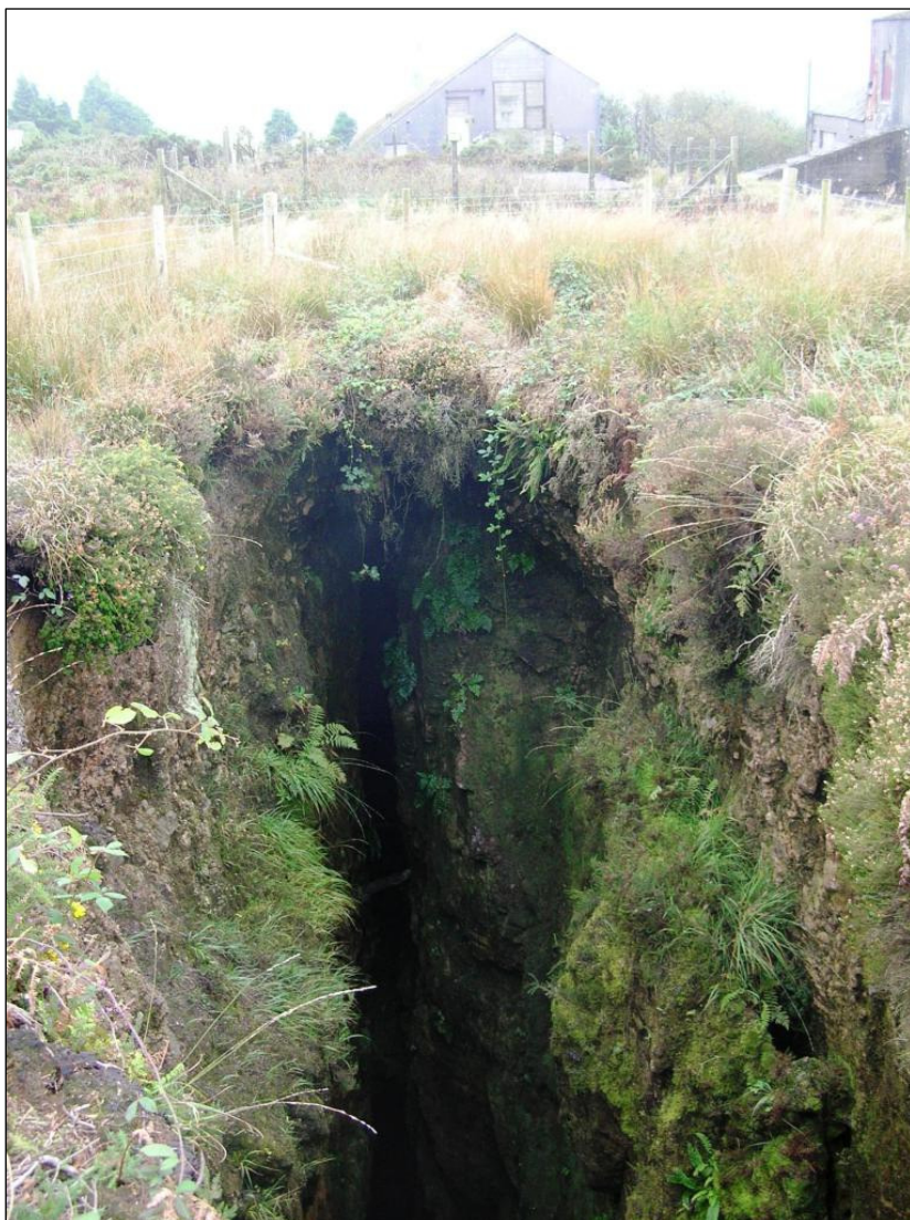
Figure 29 A view from the north of the surface collapse of the ground above the stope (Site 12) (© CC HE Projects)
