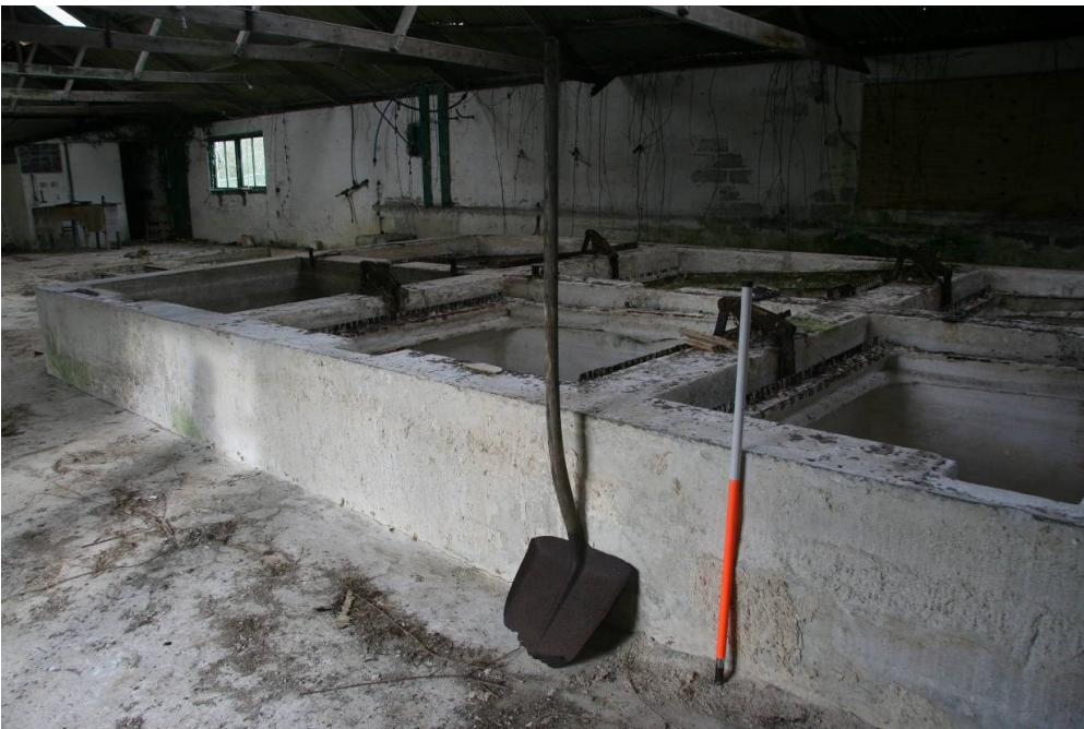
Fig 95 Liming pits inside building 18, plus cleaning shovel
