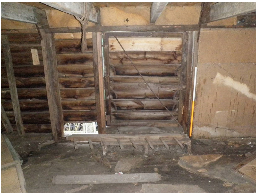
Fig 61 Building 9a, first floor interior showing adjustable louvered opening
