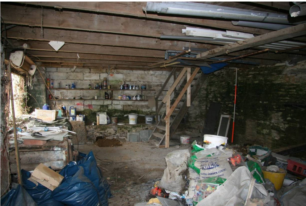
Fig 91 Ground floor interior of Building 15, looking NE
