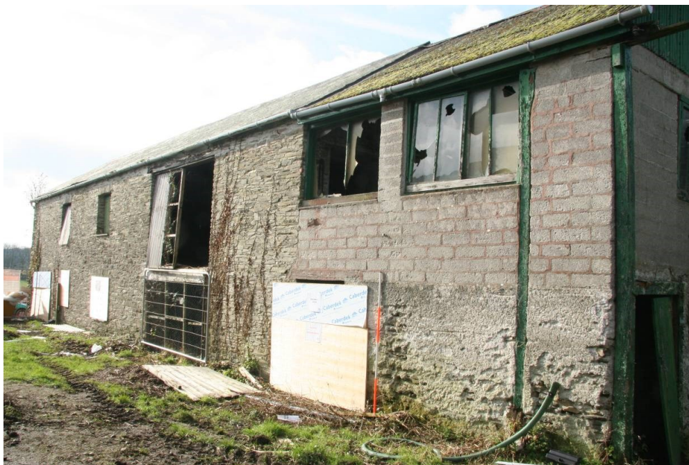
Fig 65 Building 11, east elevation
