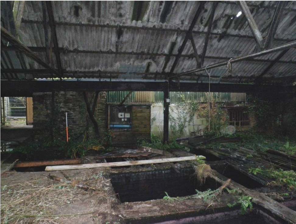
Fig 54 Building 8a, interior looking east to west elevation of Building 9a
