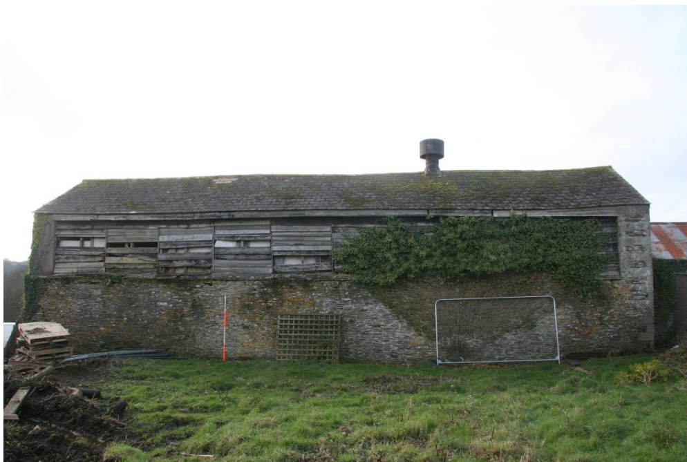
Fig 85 Building 14, east elevation
