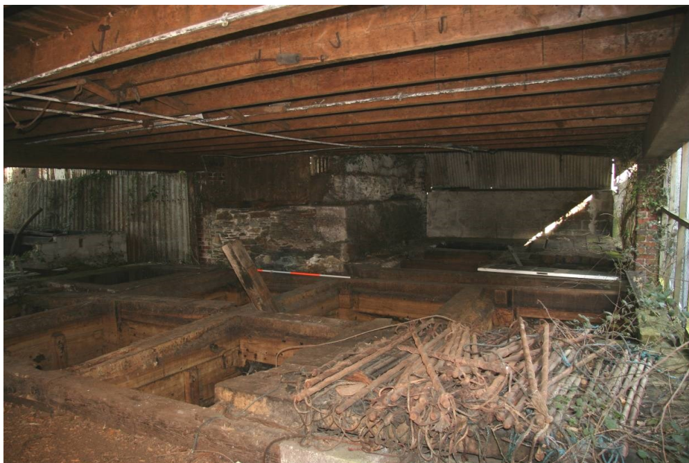
Fig 60 Buildings 9a and 9b, ground floor interior looking north
