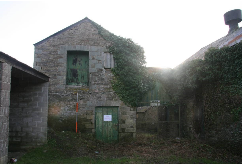
Fig 83 Building 14, north elevation
