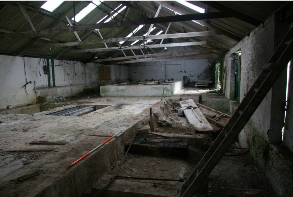
Fig 94 Interior of Building 18, looking E
