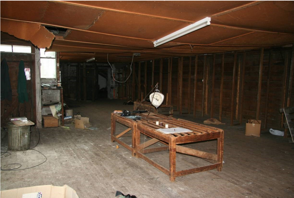
Fig 50 Buildings 7a and 7b, first floor interior looking north-east
