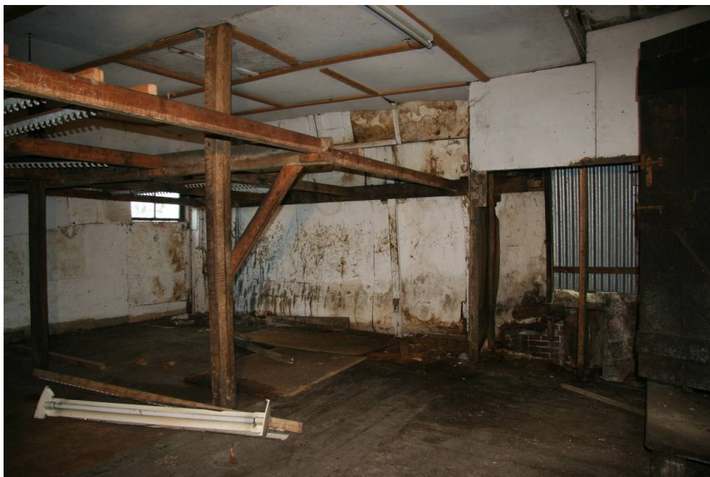
Fig 56 Building 8c, interior looking north-east
