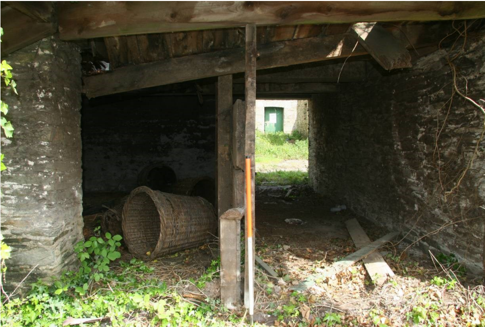
Fig 70 Building 11b, ground floor interior looking east
