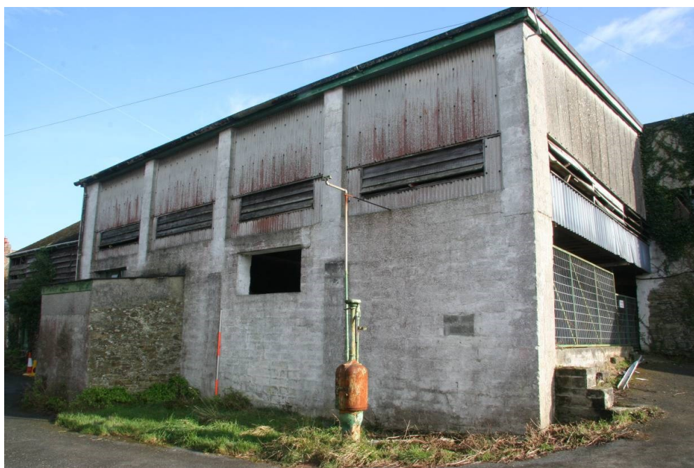
Fig 37 Building 5, west elevation
