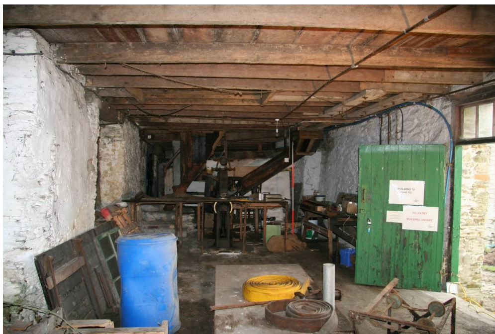
Fig 77 Building 12b, ground floor interior looking south
