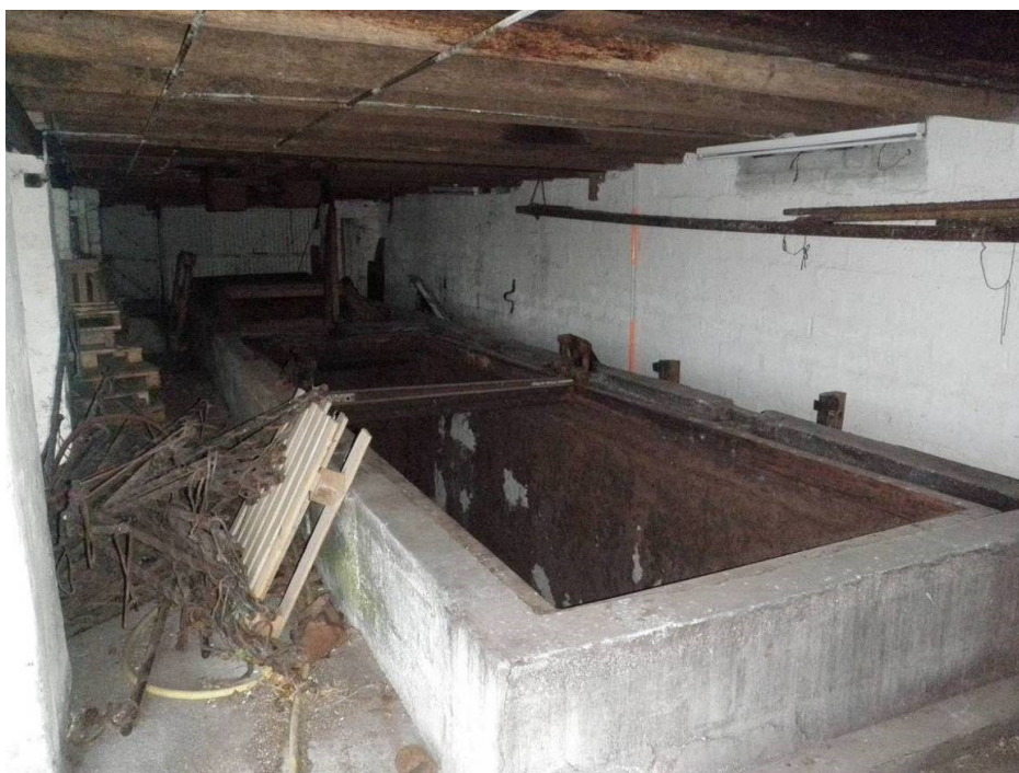
Fig 41 Building 6, ground floor interior looking north-east showing tanning pits with rockers
