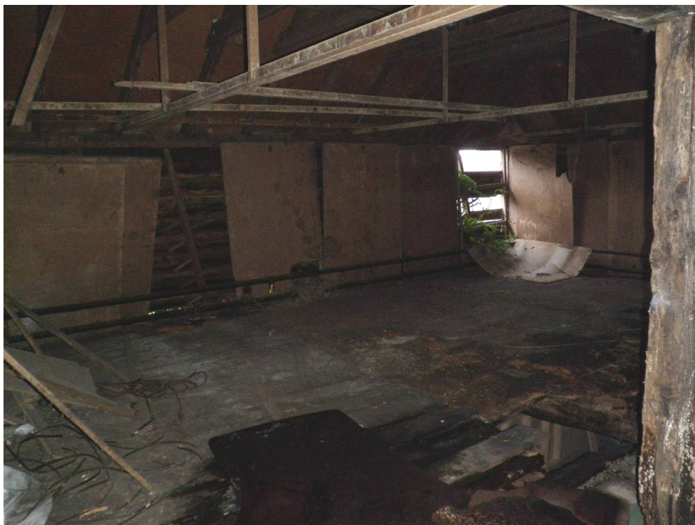
Fig 33 Building 3, first floor interior looking north-west
