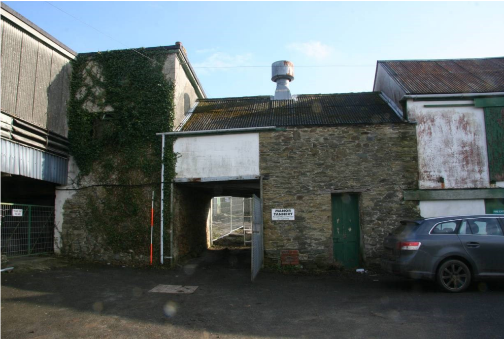
Fig 46 Buildings 6, 7d and 7c, west elevation
