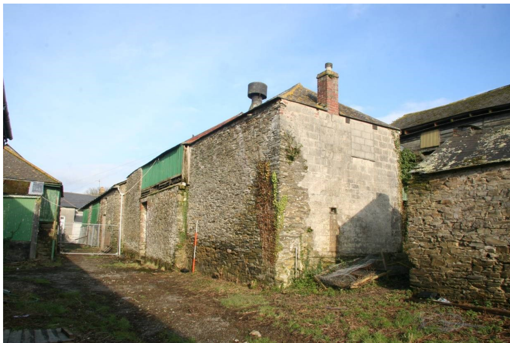
Fig 75 Building 12, west elevation
