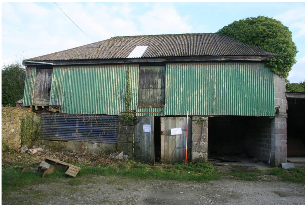
Fig 89 Building 15, looking east
