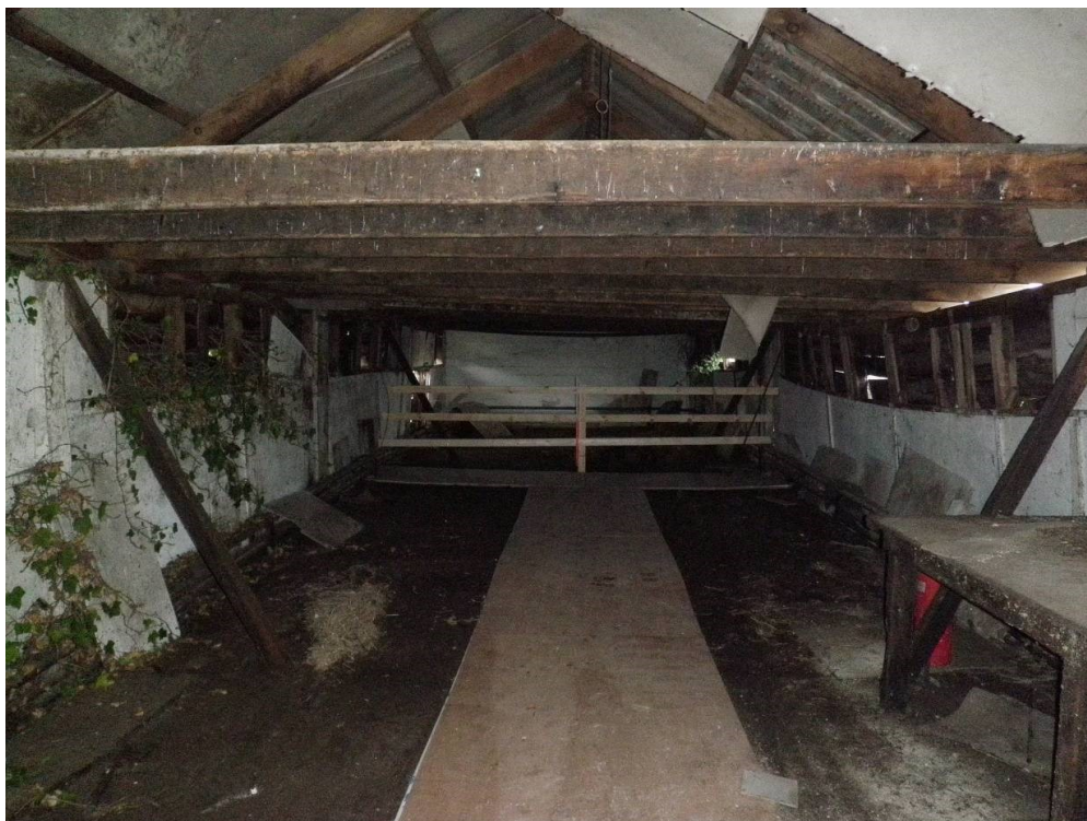
Fig 88 Building 14, first floor interior looking south
