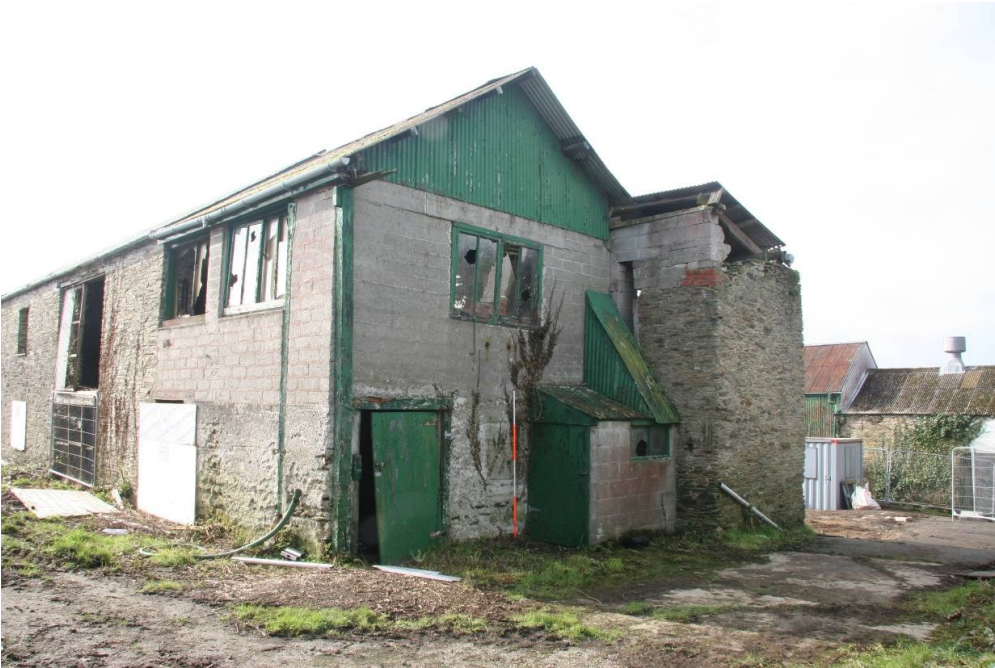
Fig 66 Building 11b, east and north elevations
