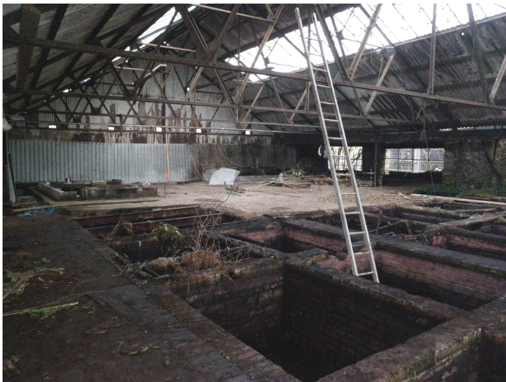
Fig 53 Building 8a, interior looking north-east
