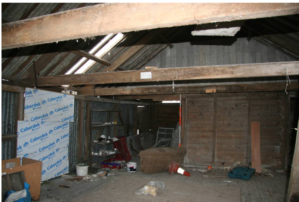
Fig 92 First floor interior of Building 15, looking N
