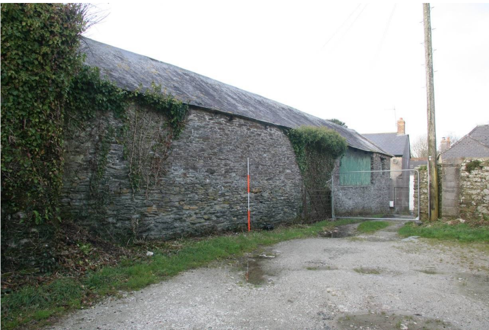
Fig 63 Building 10, east elevation
