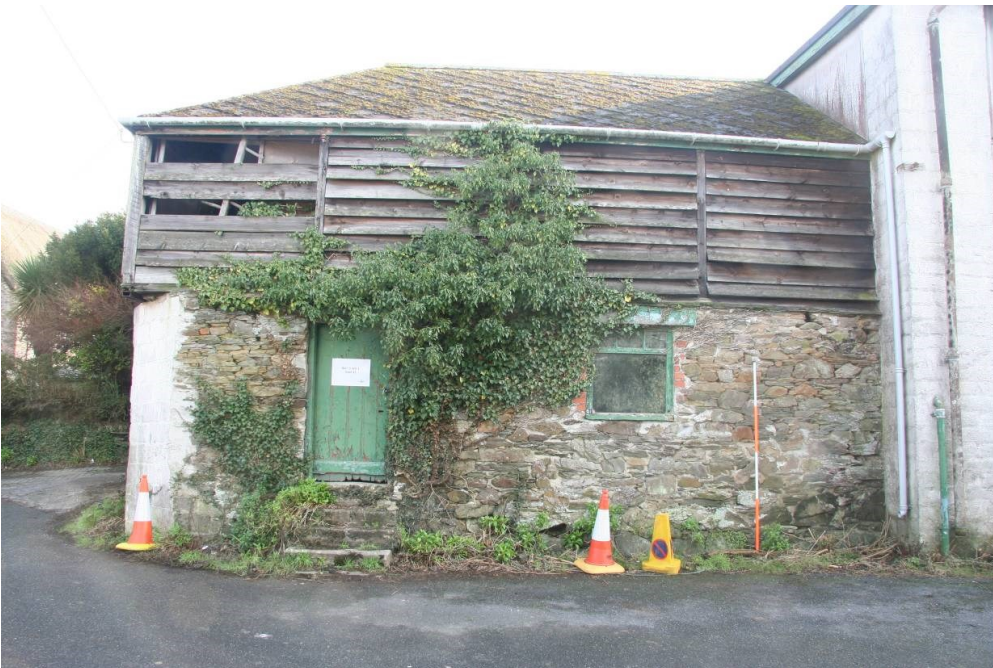
Fig 31 Building 3, west elevation (frontage)
