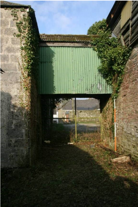
Fig 82 Aerial walkway between buildings 12 and 14 looking north
