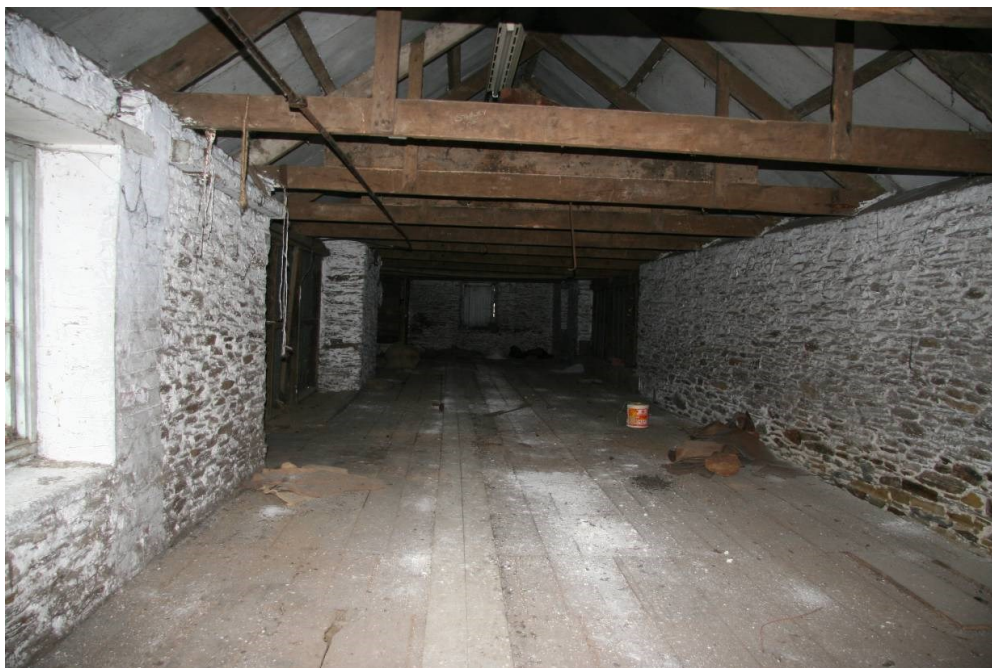
Fig 64 Building 10, first floor interior looking north
