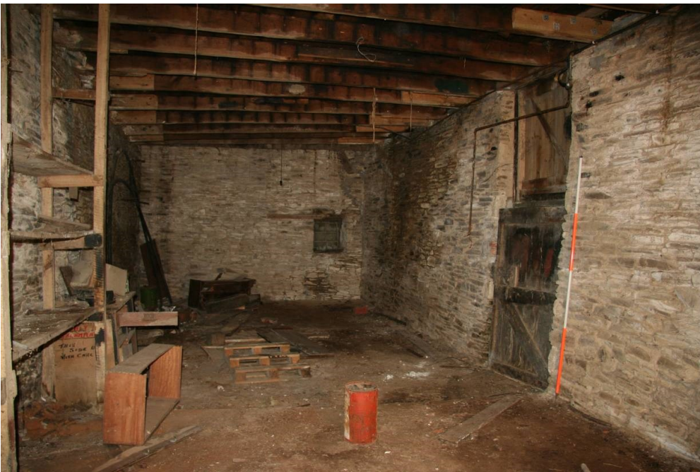
Fig 87 Building 14, ground floor interior of southern room looking south
