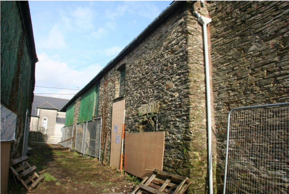
Fig 62 Building 10, west elevation
