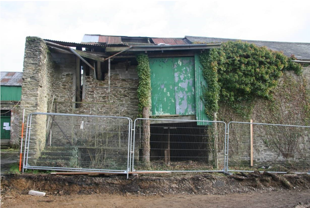
Fig 67 Building 11b, west elevation
