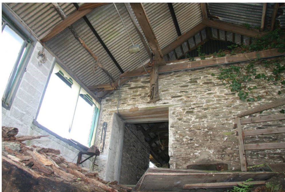
Fig 74 Building 11b, first floor interior looking south
