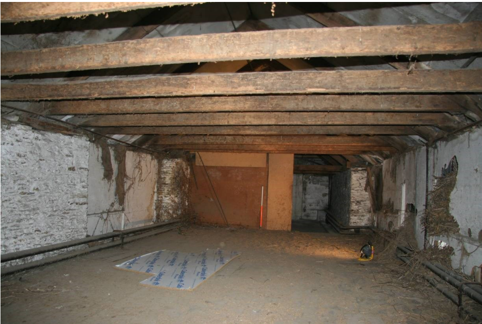
Fig 79 Building 12b, first floor interior looking south
