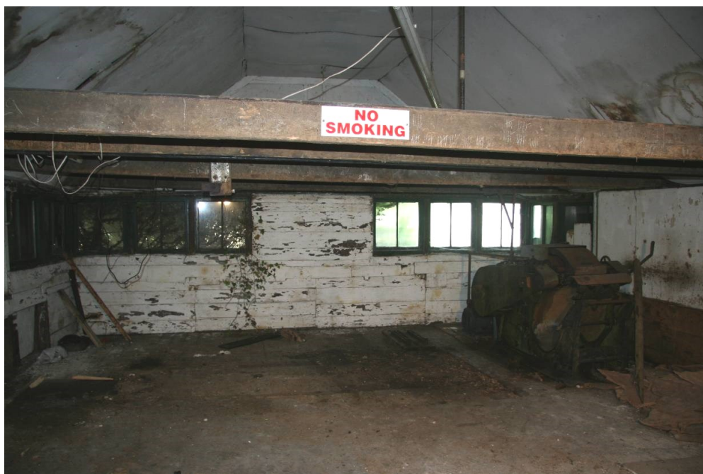
Fig 36 Building 4, first floor interior looking north
