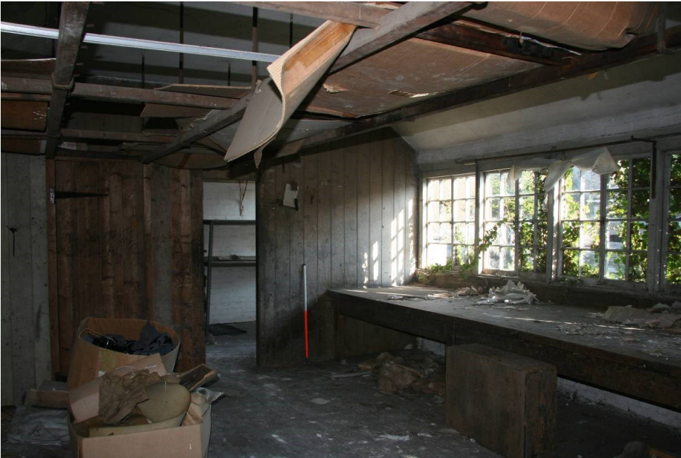
Fig 30 First floor of building 1 looking north-east
