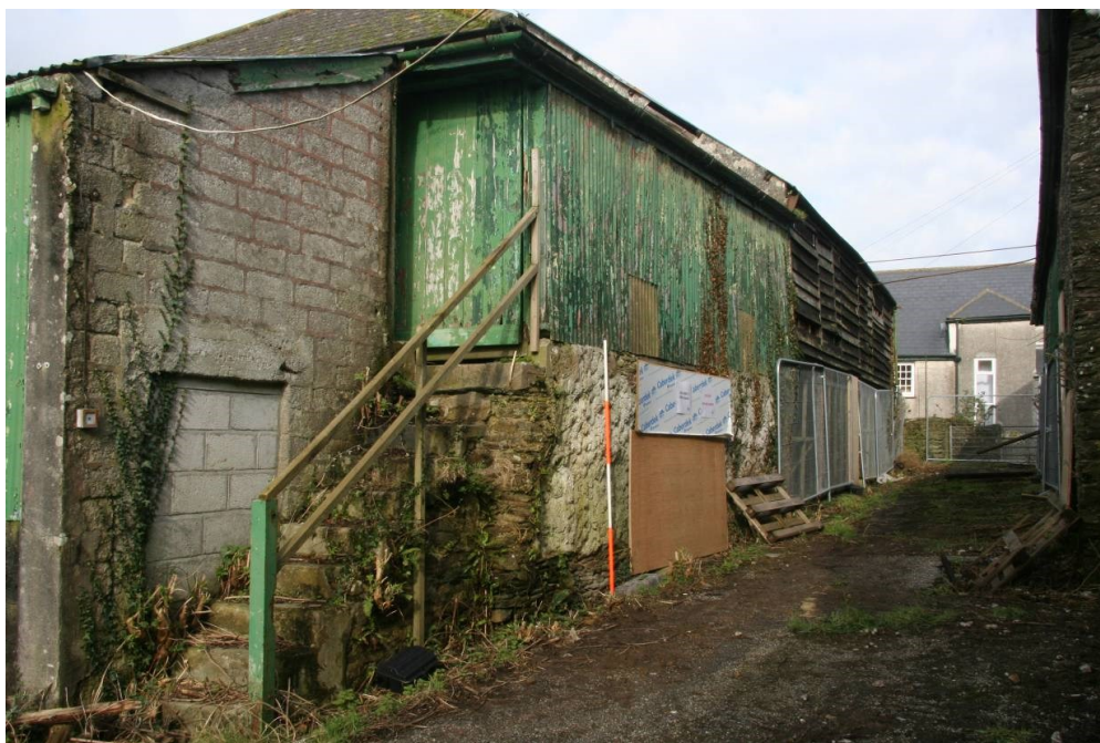
Fig 57 Building 9, east elevation of 9a and 9c
