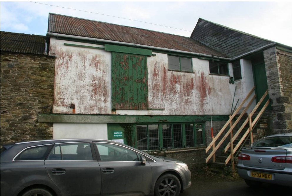
Fig 47 Building 7b, west elevation
