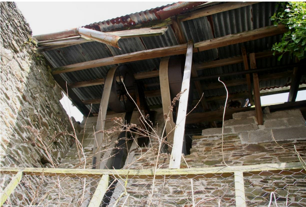
Fig 71 Building 11b, west elevation showing wheel and belt drives for mills
