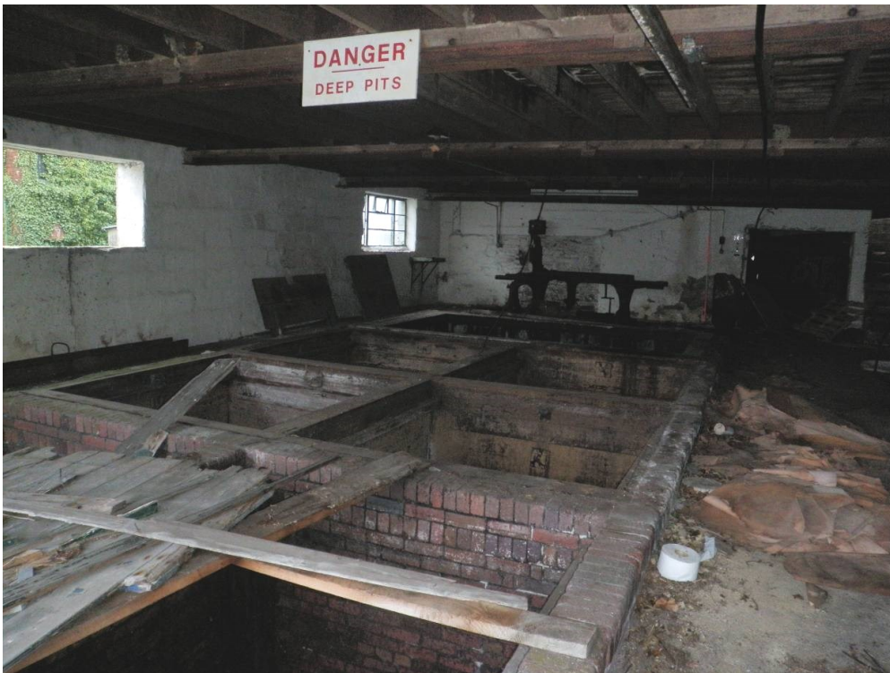
Fig 38 Building 5, ground floor interior looking north-west
