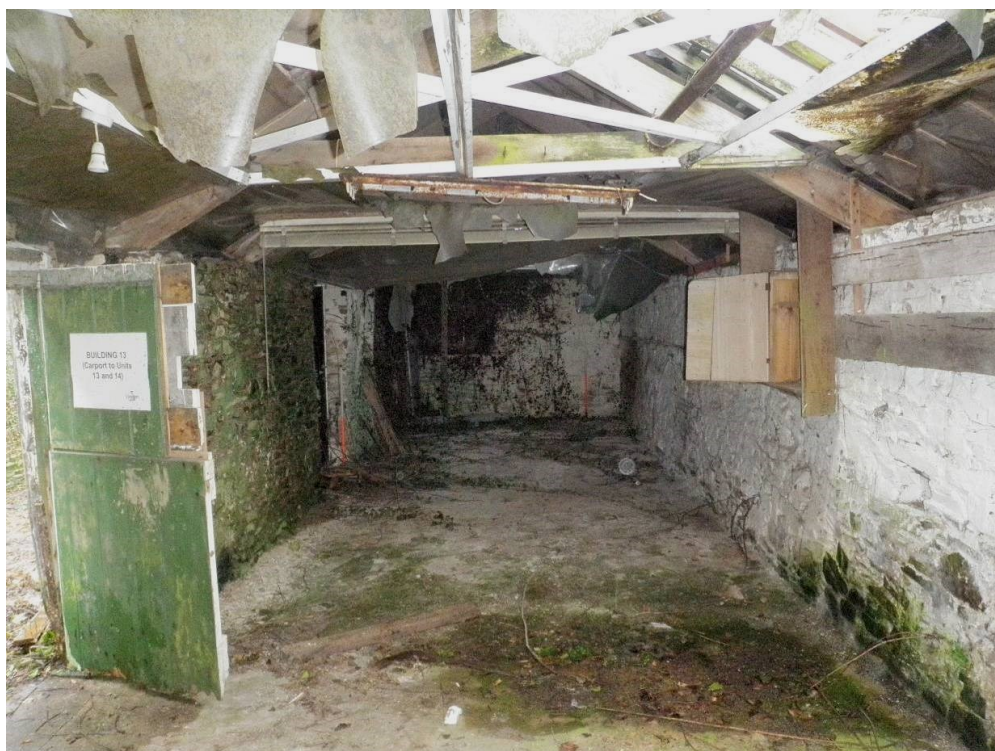
Fig 81 Building 13, interior looking south
