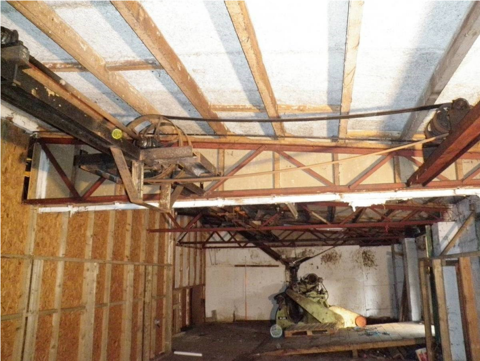
Fig 55 Building 8b, interior looking north, showing machine and drive belts
