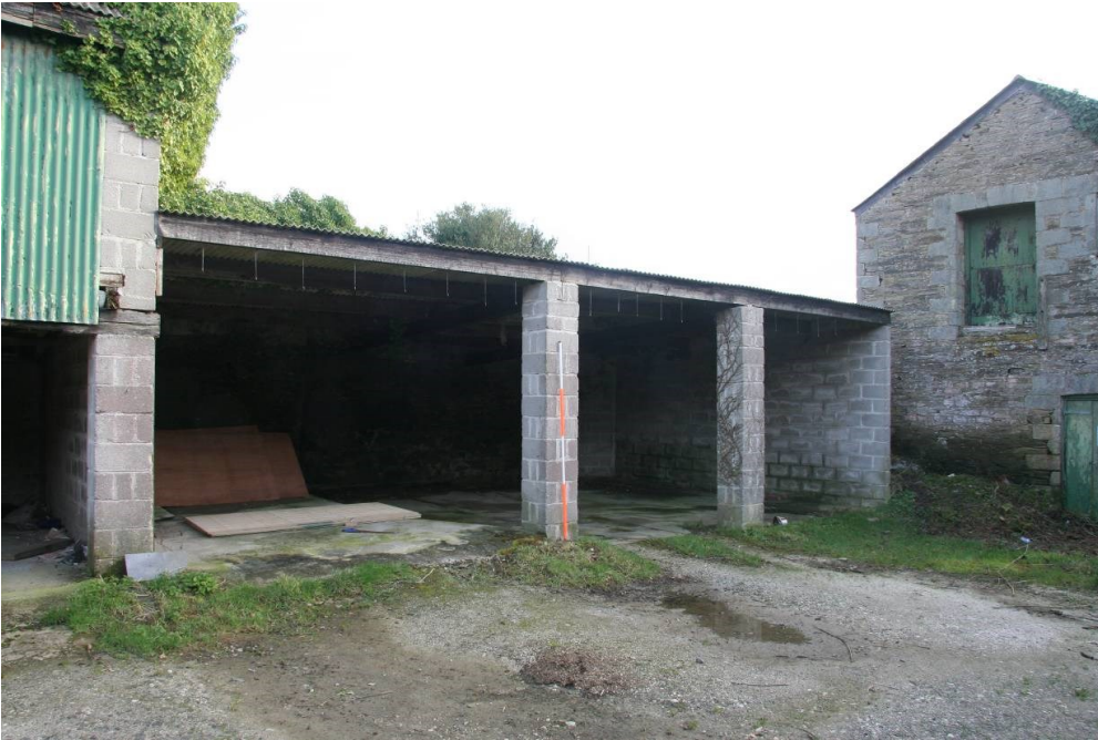
Fig 90 Late 20 th century blockwork at S end of Building 15
