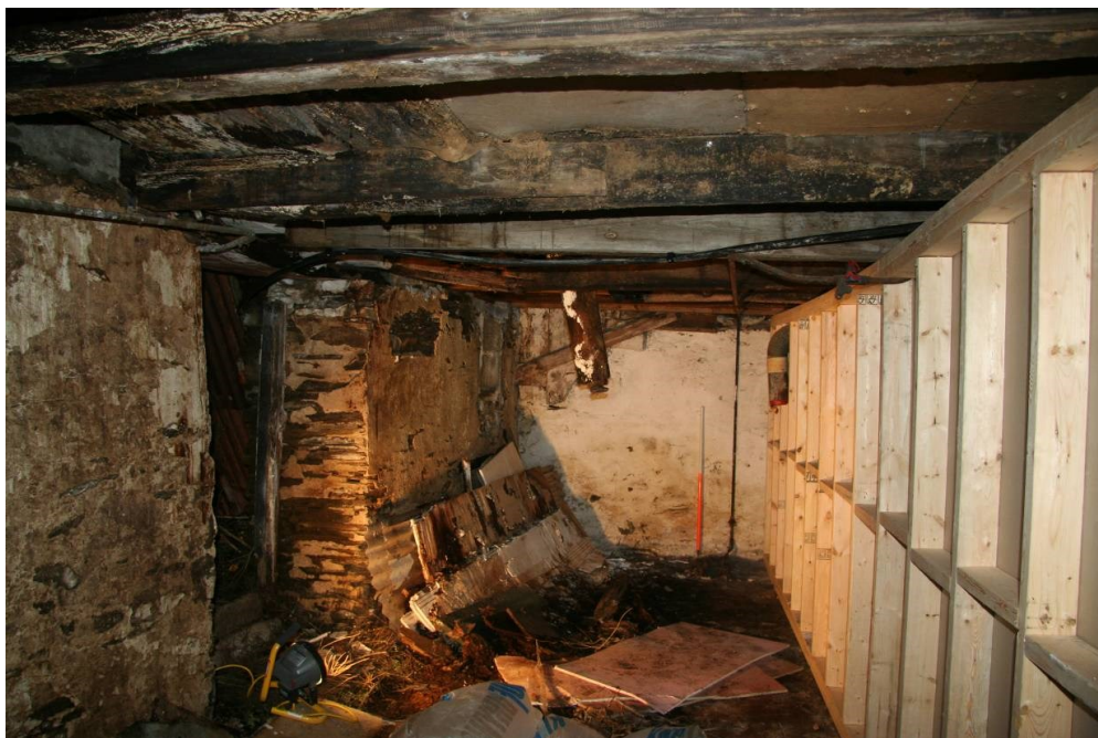
Fig 32 Building 3, ground floor interior looking north
