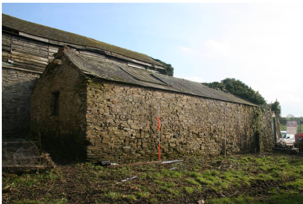
Fig 80 Building 13, west elevation
