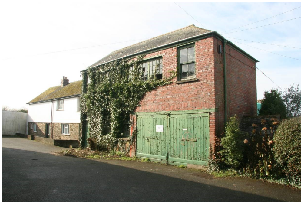
Fig 28 Buildings 1 (foreground) and 2, east elevation (frontage)
