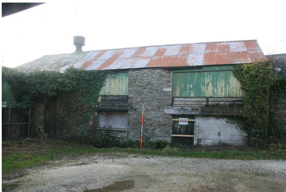
Fig 76 Building 12b, east elevation
