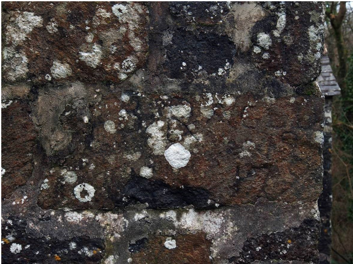
Plate 18 Dated stone reused within quoin of SW extension
