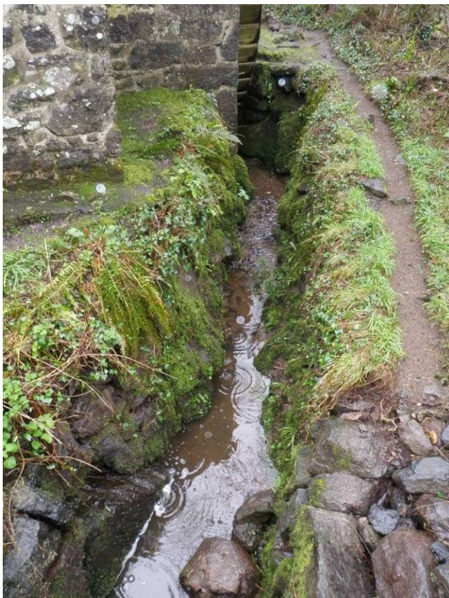
Fig 23: Poltesco Mill tailrace, part of leat 92520 looking west
