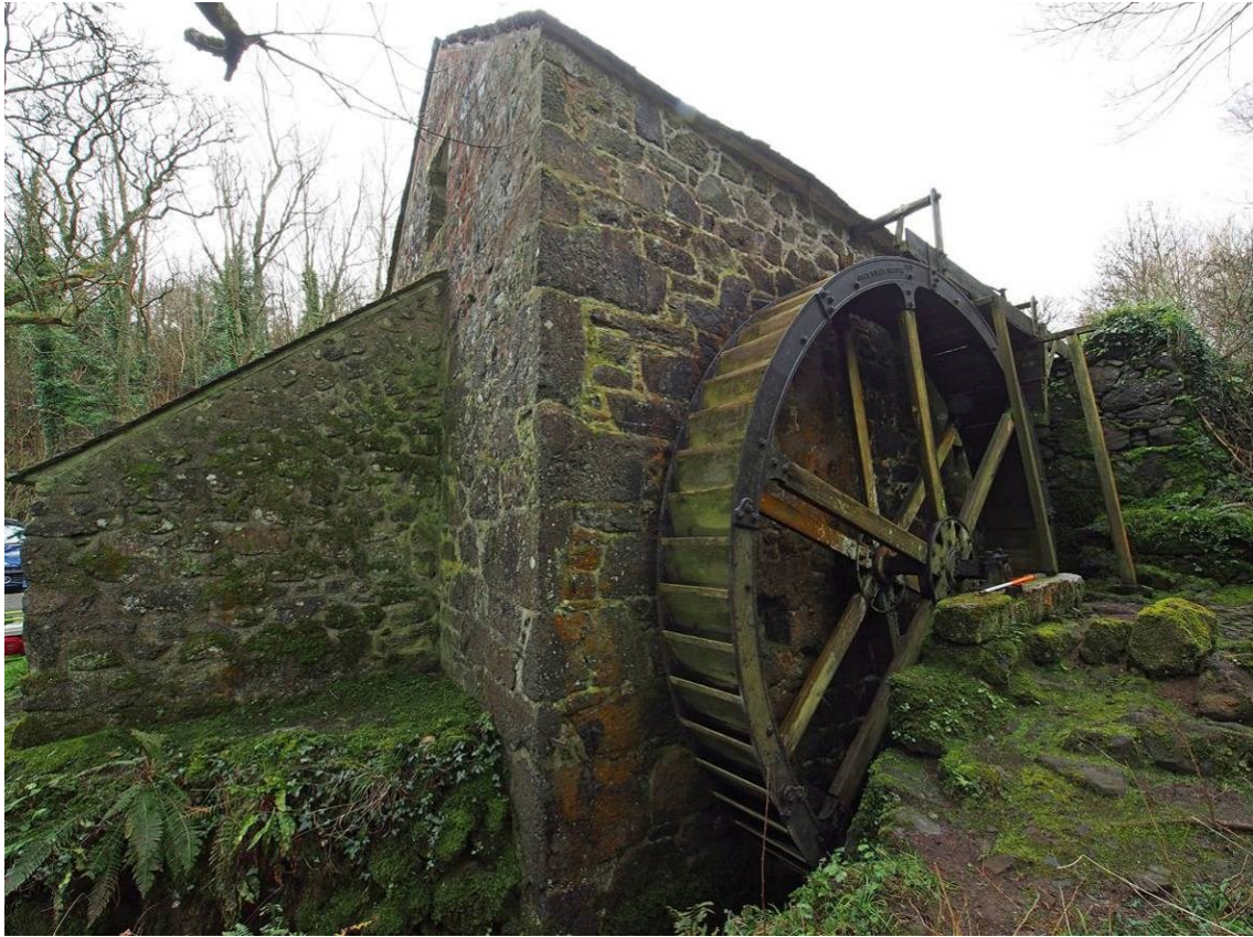
Plate 5 Poltesco Mill from the N, showing the waterwheel and tailrace
