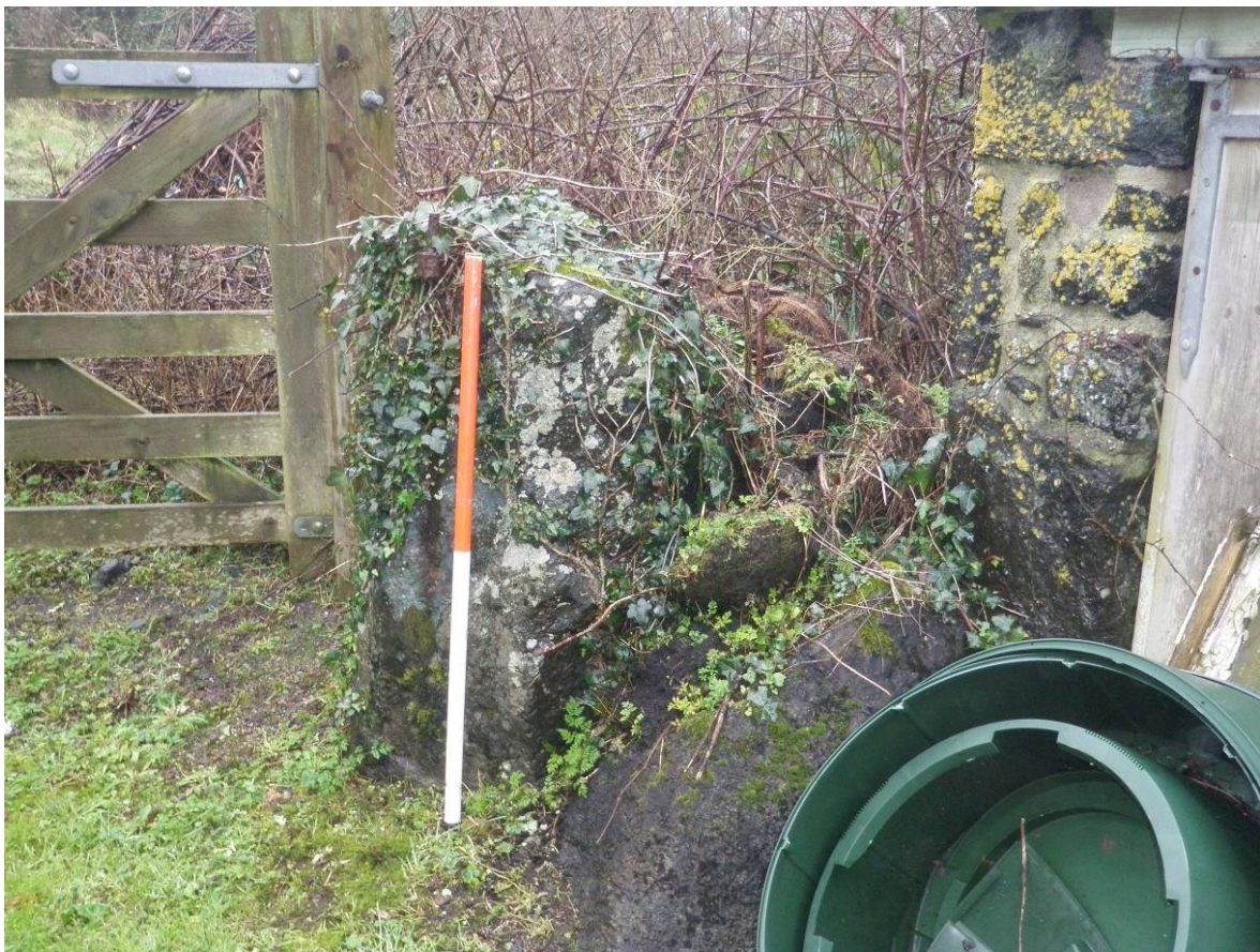
Fig 37: Serpentine gate post 92620 looking west
