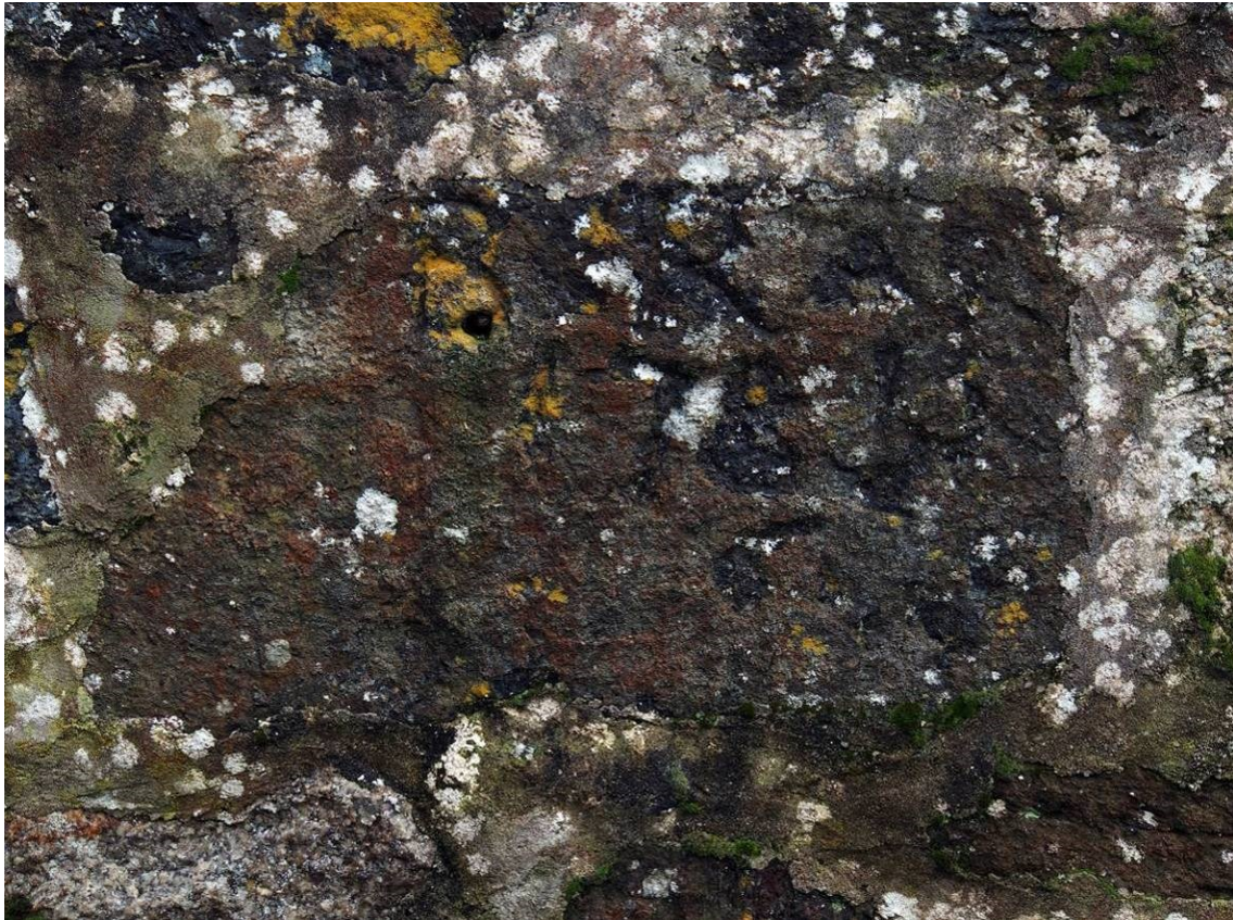
Plate 19 Dated stone reused within quoin of SW extension
