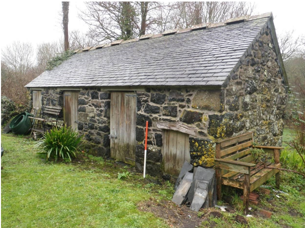
Fig 29: Piggery 92523 looking north-west
