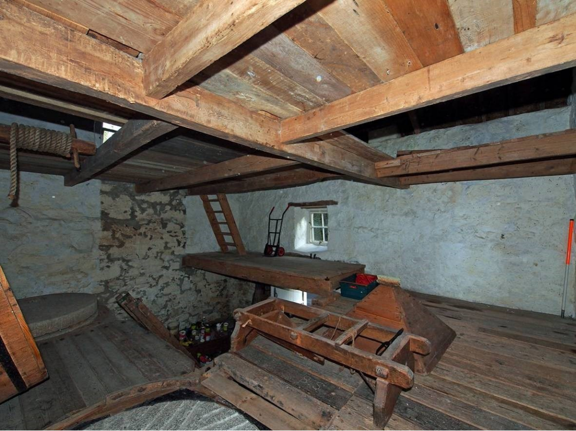
Plate 33 View of first floor looking E
