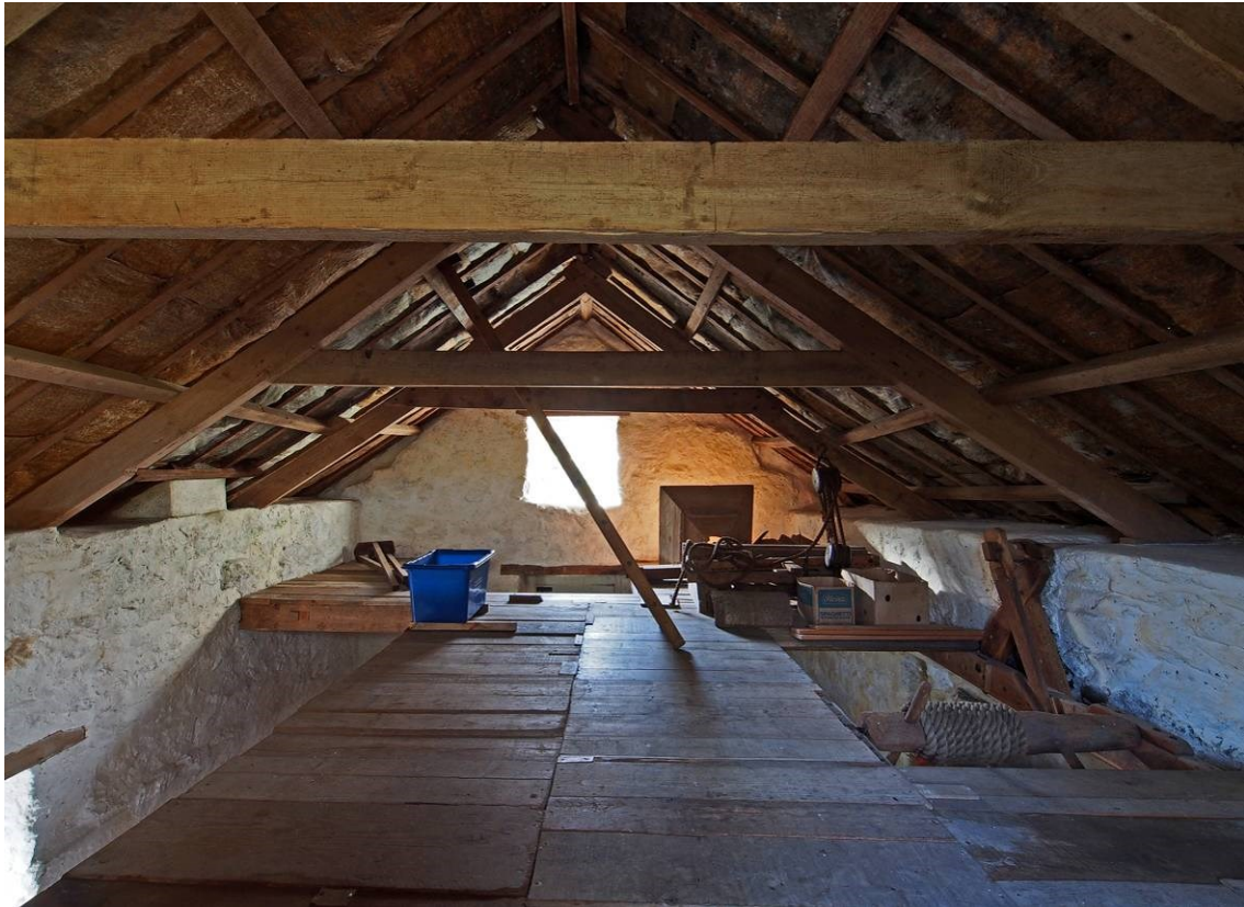
Plate 41 View of the loft floor looking SW
