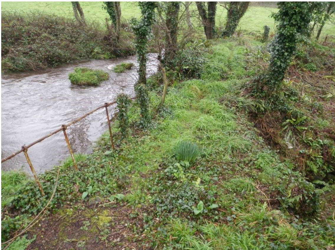
Fig 41: Raised bank 92629 retaining north side of millpond. Taken at west end looking north
