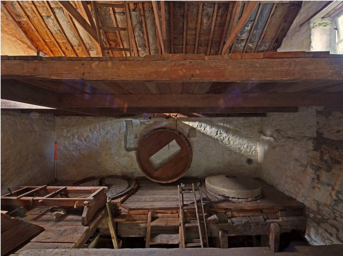
Plate 31 View of the millstones on the first floor (looking NW)
