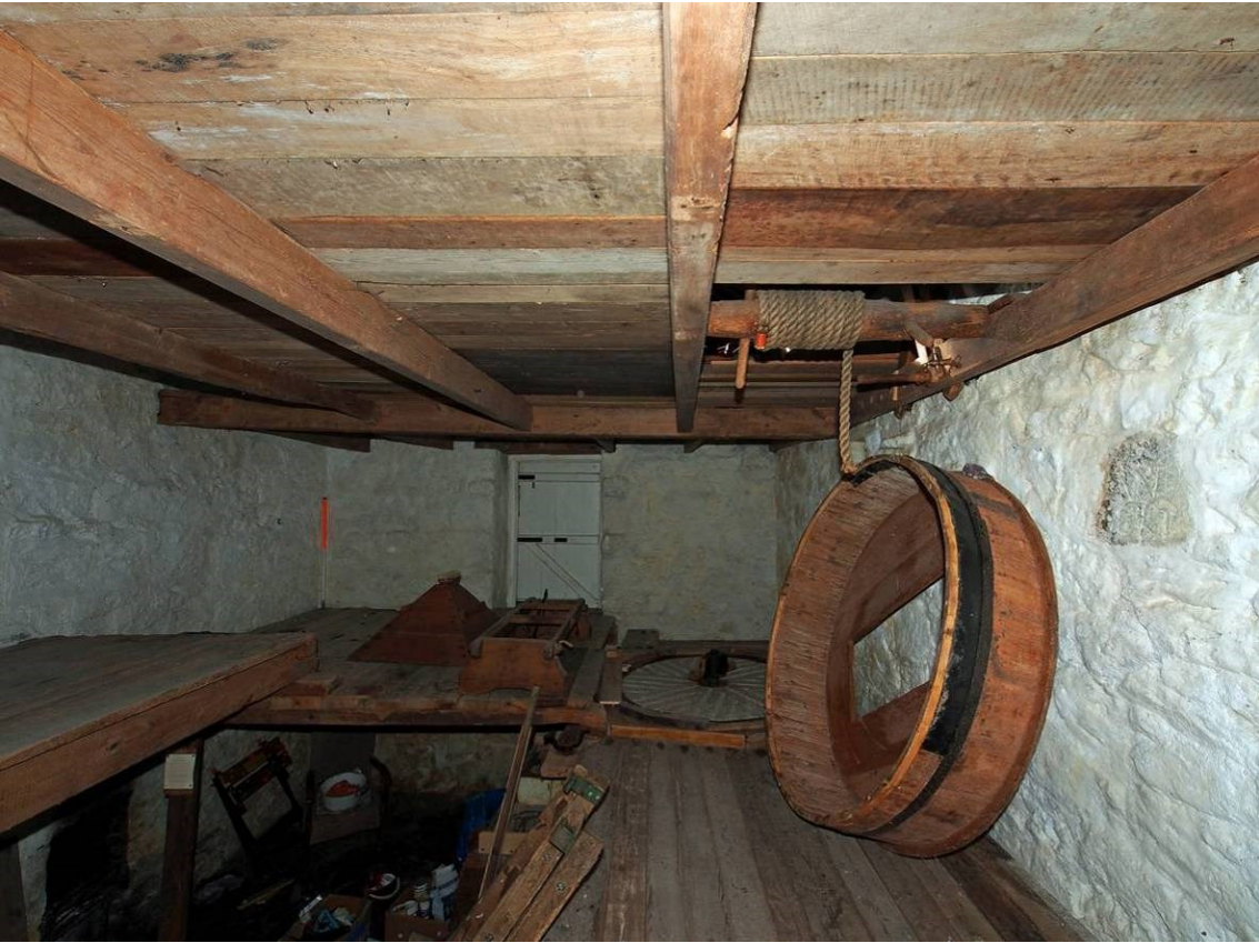
Plate 34 View of first floor looking SW
