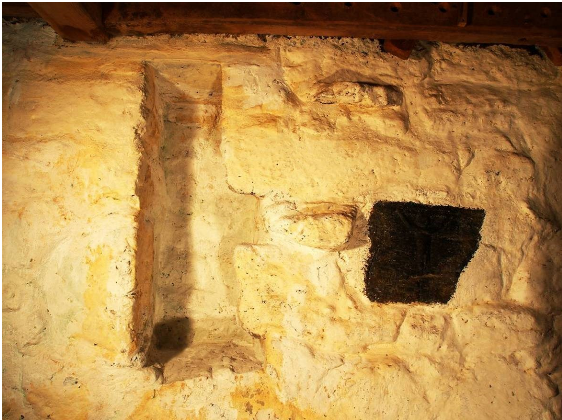
Plate 38 Recess in NW wall on first floor, which appears to have been created from where the earlier SW wall formed a quoin. Note the stones protruding from the wall to the right
