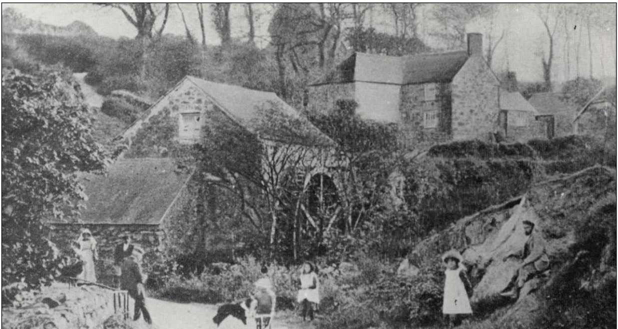
Fig 13: Postcard view of Poltesco Mill, site 92519 , and Poltesco Mill House, site 92522 , in 1906 (from Ivey nd)
