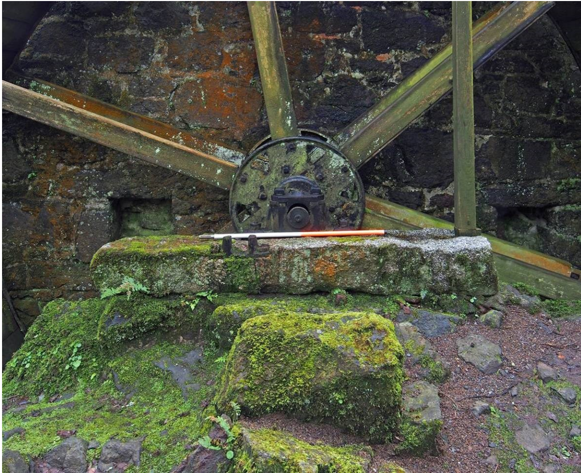
Plate 13 Reused granite block supporting the bearings of the waterwheel. Note the earlier bracket position on the outside of the stone
