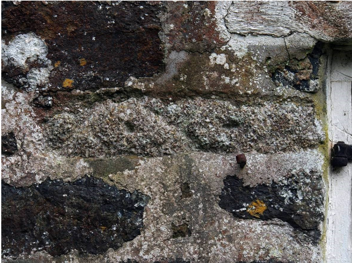
Plate 21 A granite central portion from a composite early millstone, reused in the SW extension
