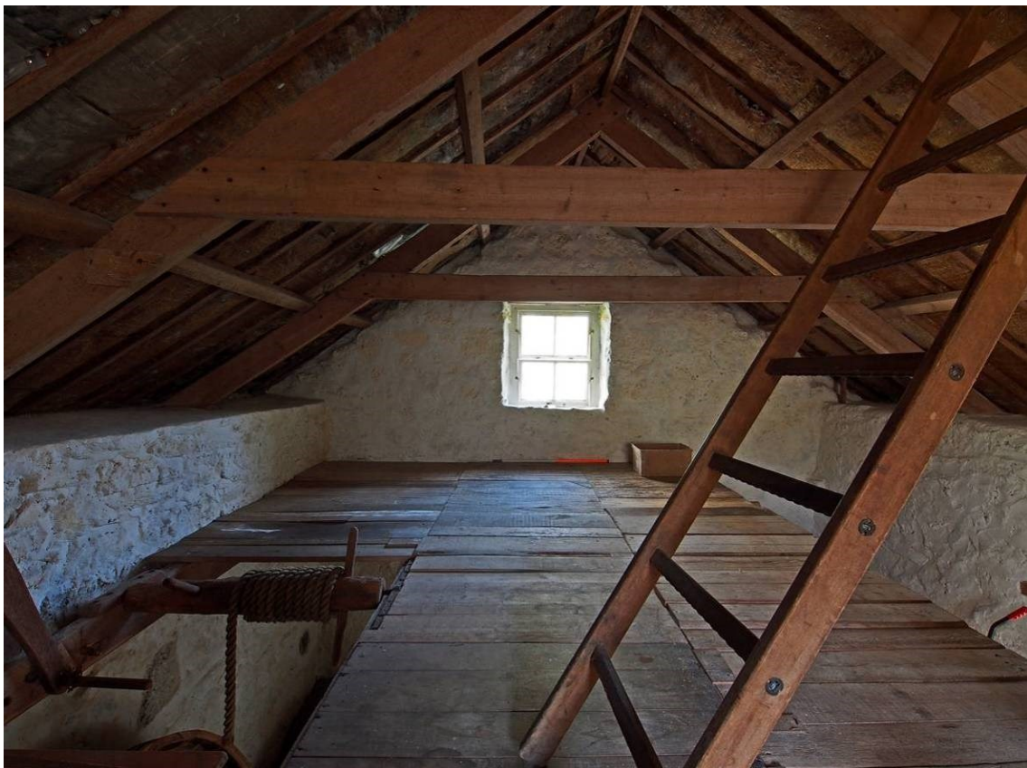
Plate 40 View of the loft floor looking NE
