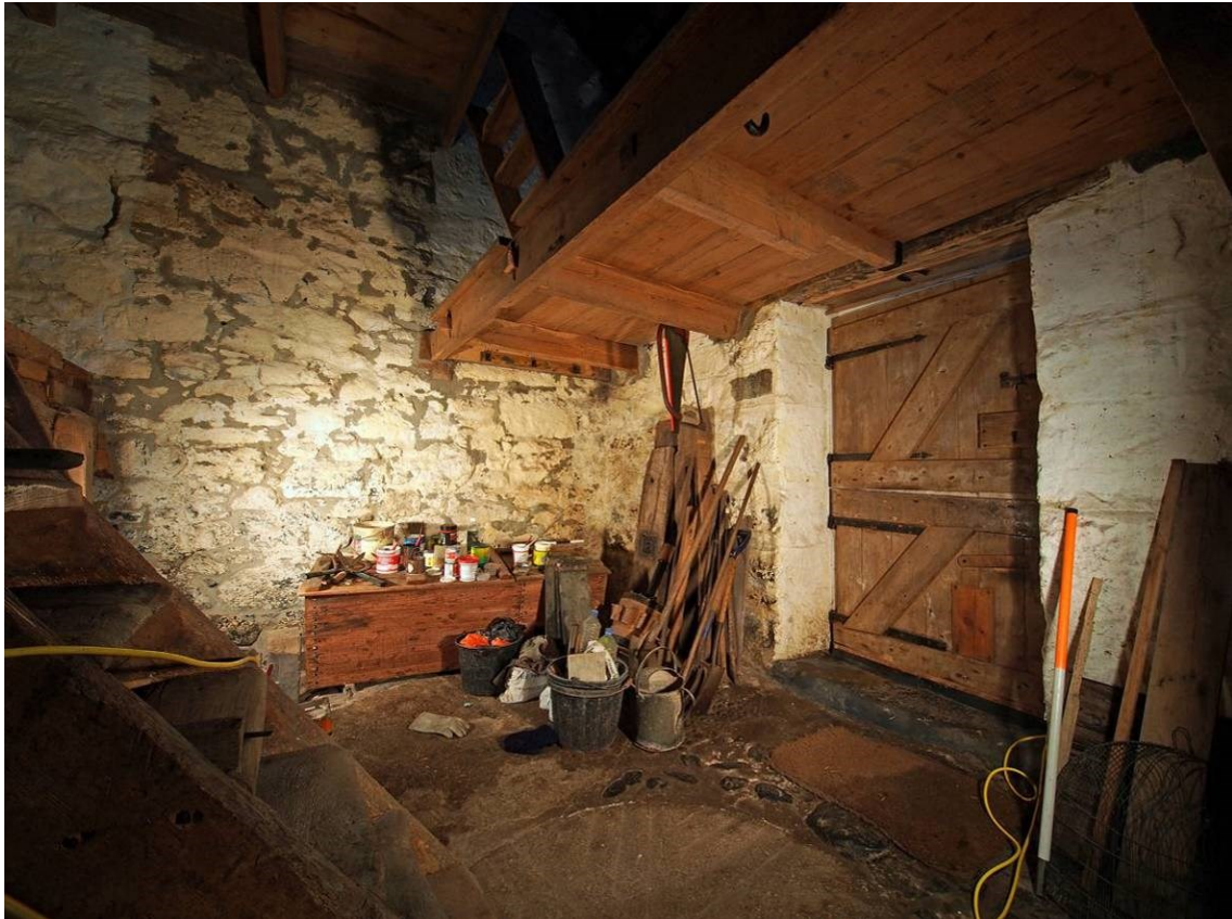
Plate 23 Ground floor of the mill, showing the main door and reused millstones in the floor. The boarded floor above was added c1910 when grading machines were accommodated
