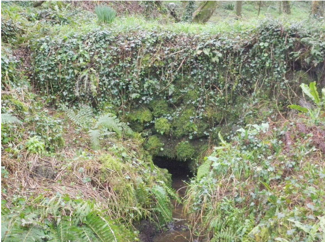
Fig 40: Culvert 92628 at west end of leat 92627
