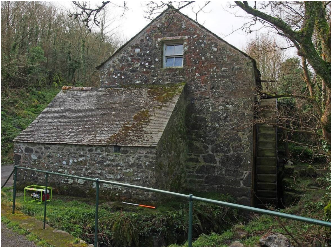
Plate 4 Poltesco Mill from the NE, showing the waterwheel and tailrace
