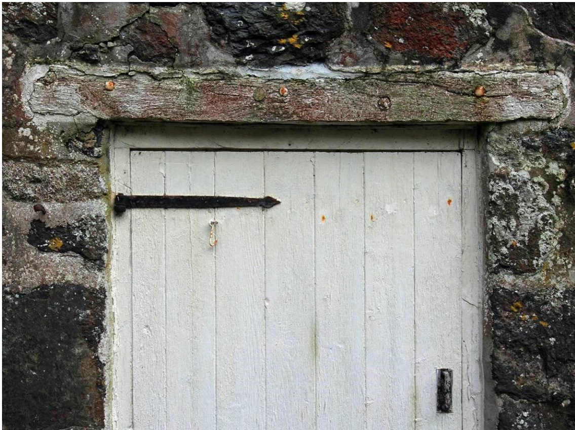
Plate 20 Part of a ships timber reused as a lintel in the SW extension
