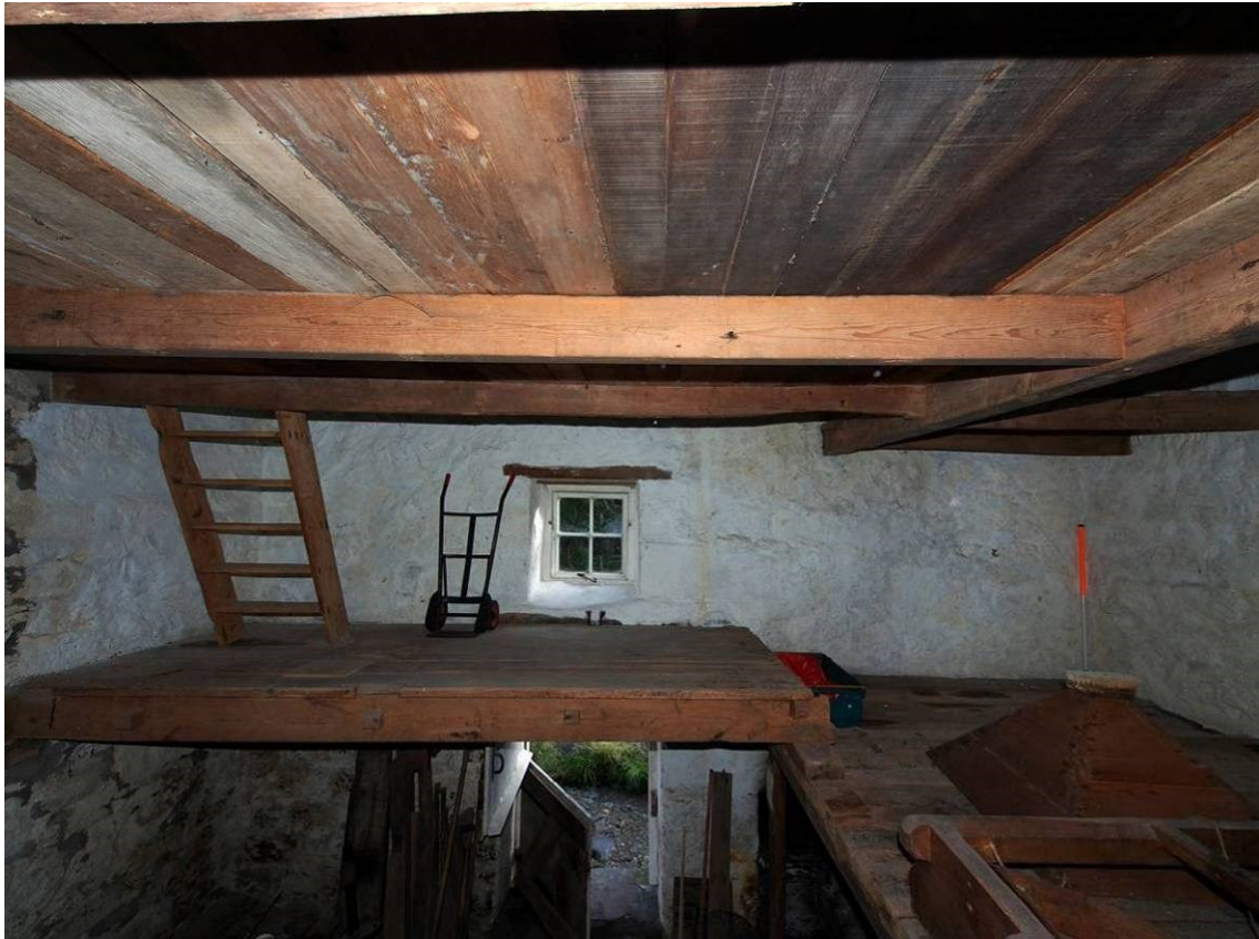
Plate 35 View of first floor looking SE
