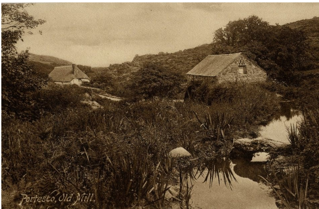
Fig 16: Postcard view of Poltesco Mill, site 92519 , looking along the leat 92520 from the millpond and house to east (now demolished), not dated (image kindly supplied by Sarah Legge via Jeff Lee)
