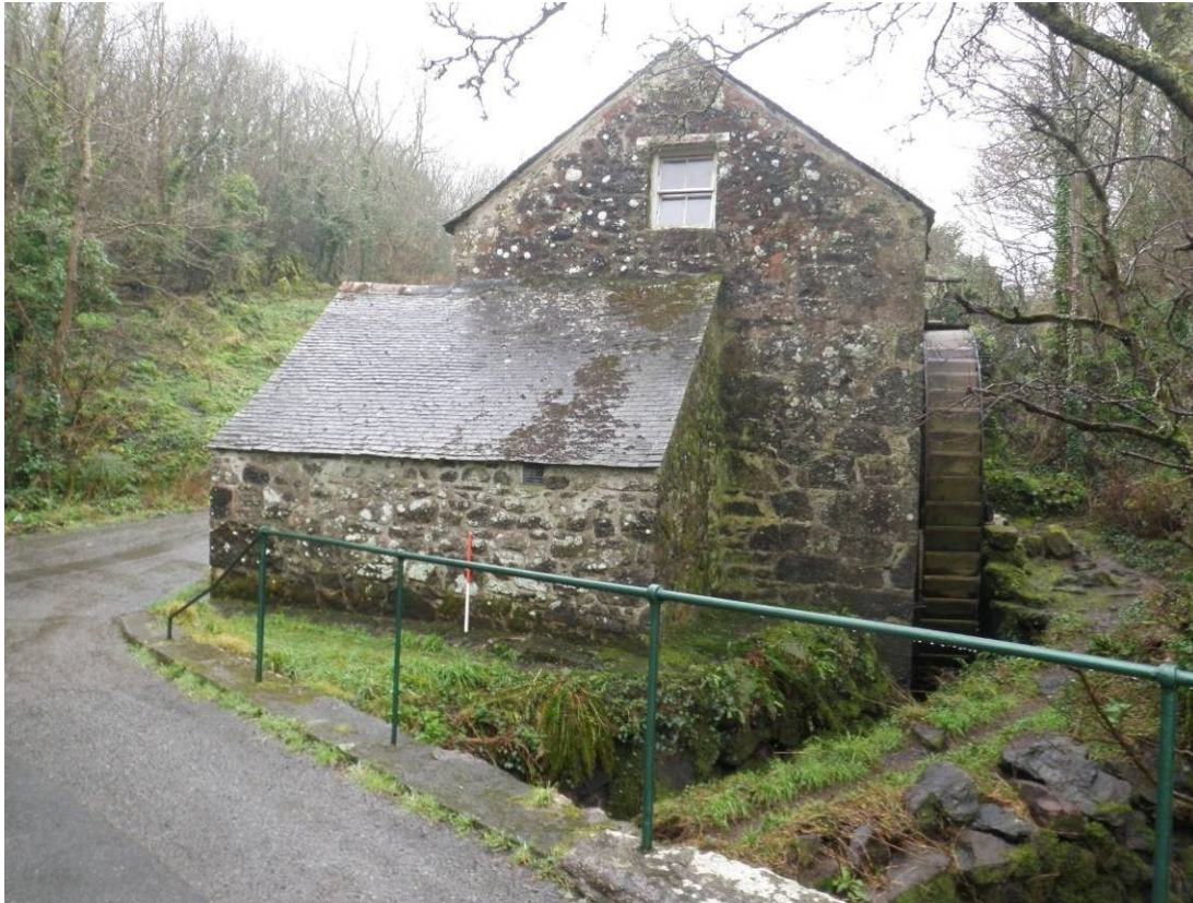
Fig 22: Poltesco Mill 92504 looking south-west
