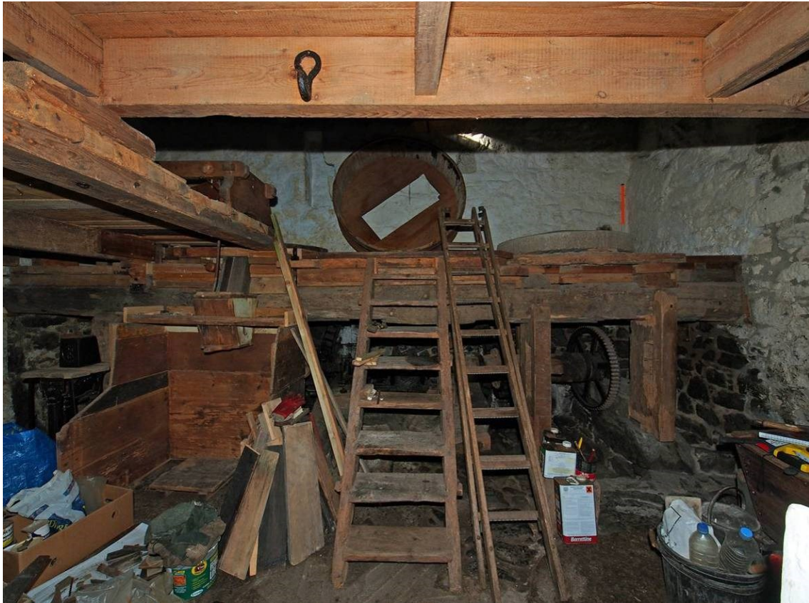
Plate 25 Ladder to first floor (millstones visible towards upper right)
