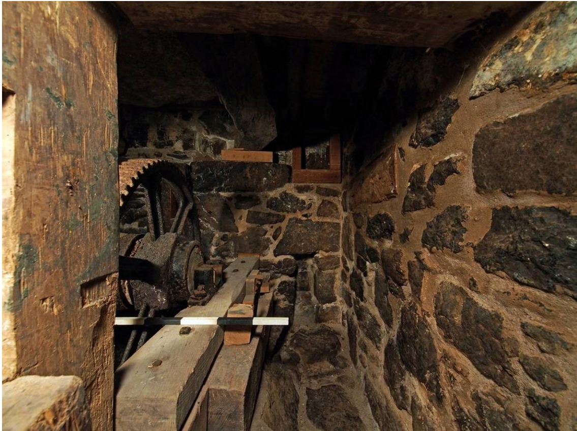
Plate 29 Vertical slot in NE corner shows hints at earlier arrangement of bridgework
