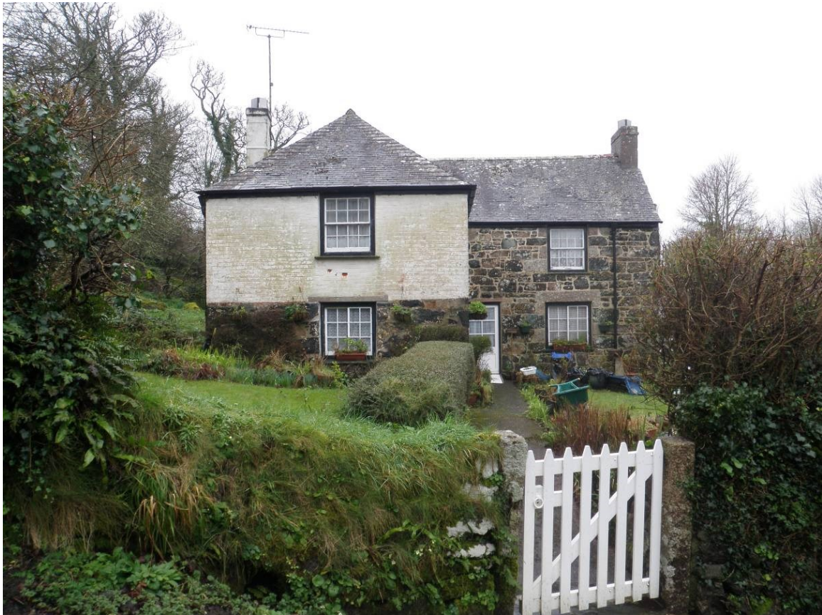
Fig 27: Mill House 92522 looking west
