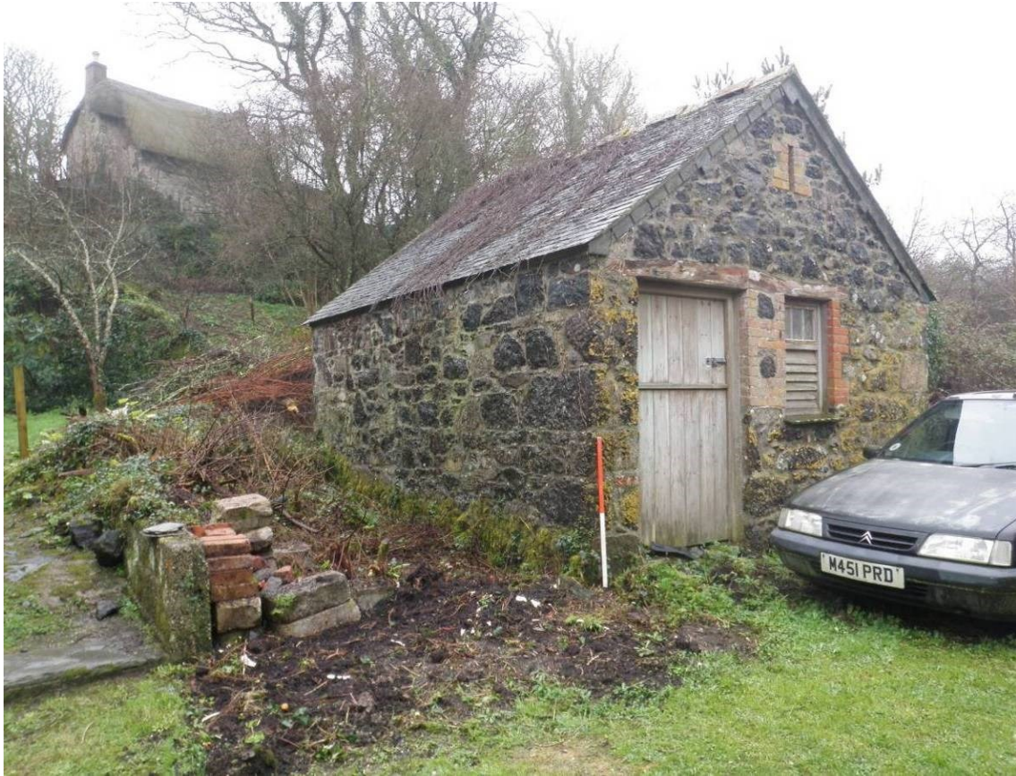
Fig 30: Stable 92524 looking south-west
