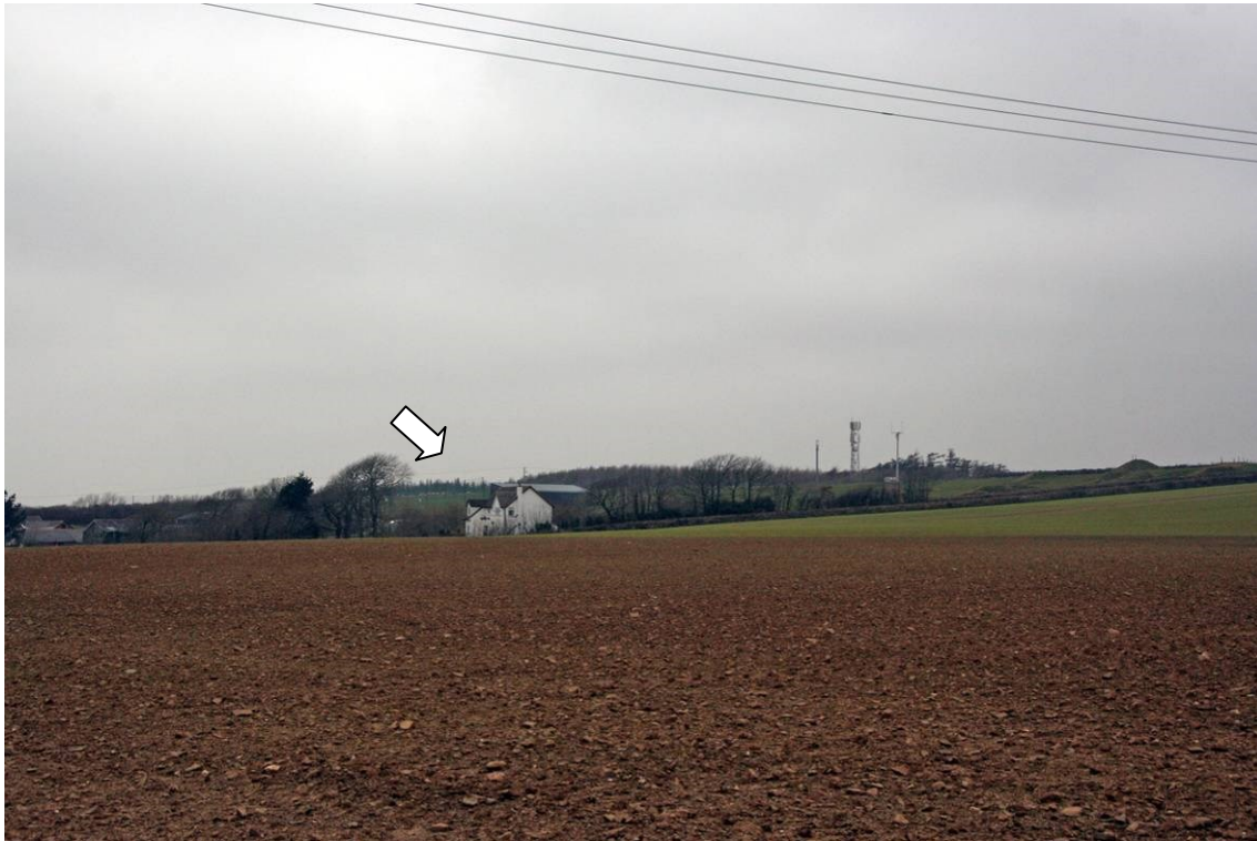
Fig 35 View north west upslope from Herdbury round towards Ivyleaf farm and the proposed turbine site (arrowed)
