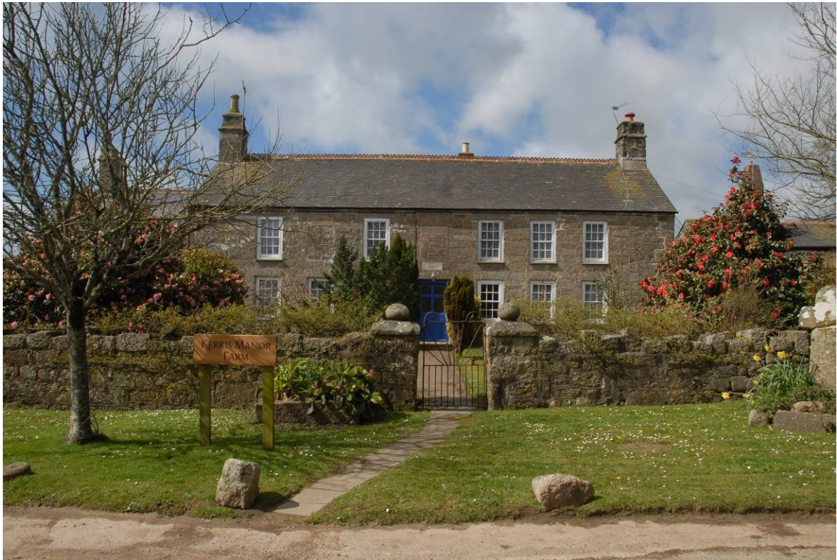
Fig 43. The eastern (principal) frontage of the Grade II* Listed Kerris Manor farmhouse.
