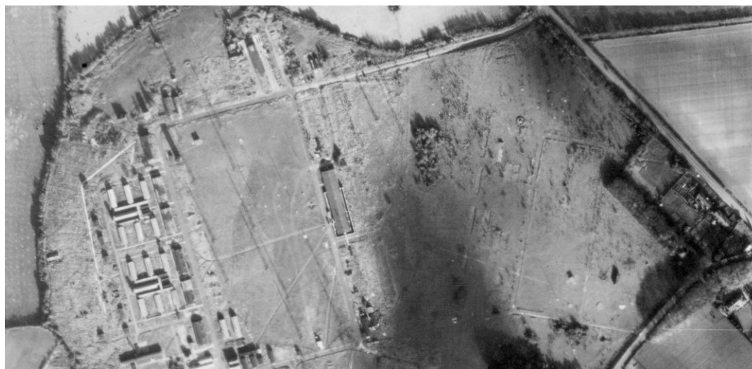
Figure 78. Second World War radar or radio station at Sir John Moore Barracks. The locations numerous masts are visible as long linear shadows on this image taken in low light in November 1946, MKM3113. Photograph: RAF/CPE/UK/1842 Frame 3115 18 th November 1946. English Heritage RAF Photography.
