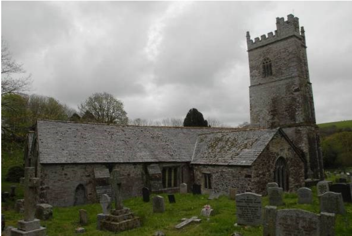
Fig 27. Looking across Lanteglos-by-Camelford church in the general direction of the proposed wind turbine, whose upper mast and blade would be visible in this view in the winter when the leaves are off the trees.
