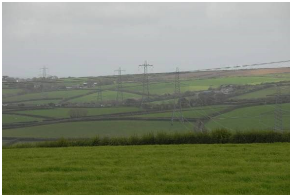
Fig 16. The prominent run of high voltage pylons crossing the landscape to the north and west of the site at Bodulgate.
