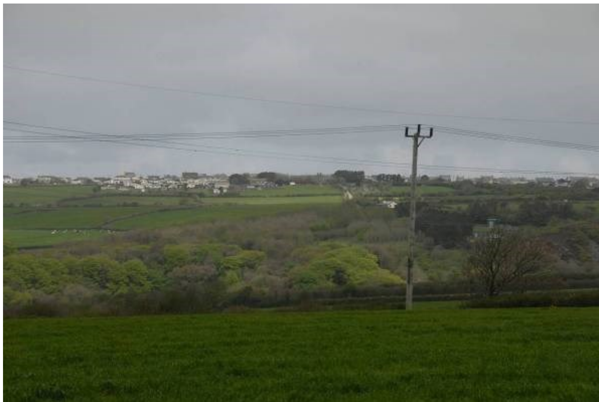
Fig 24. Pengelly (Delabole) to the north west of the site forms the skyline, the Methodist chapel being far left in this view.
