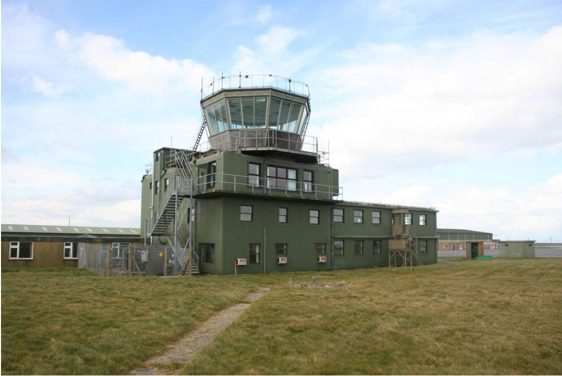
Fig 5 The former RAF ATC tower viewed from the east
