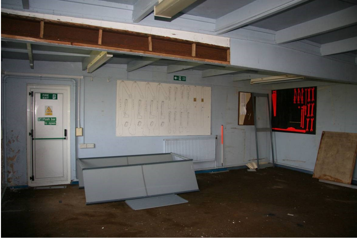
Fig 31 Unidentified room within the SE Wing, with boards for equipment surviving
