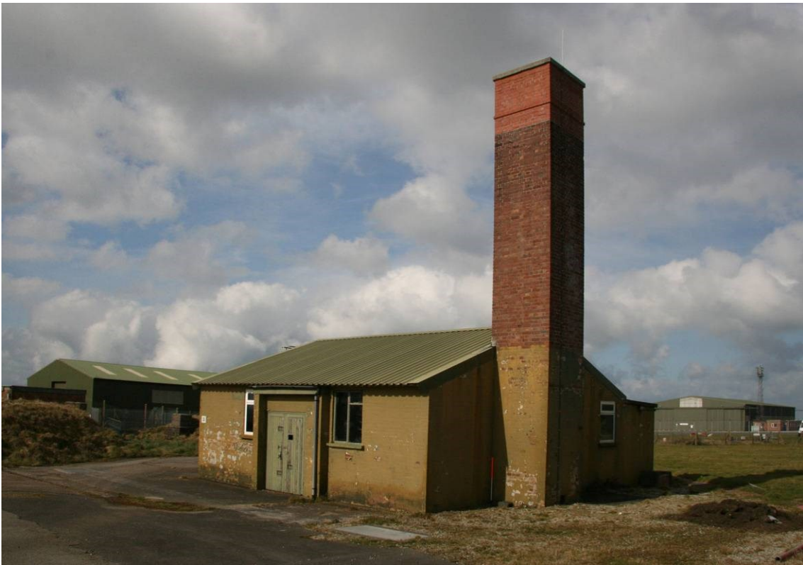
Fig 10 Boiler house and chimney, viewed from the east
