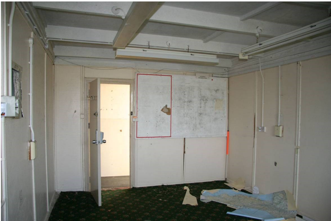
Fig 32 Unidentified room within the SE Wing
