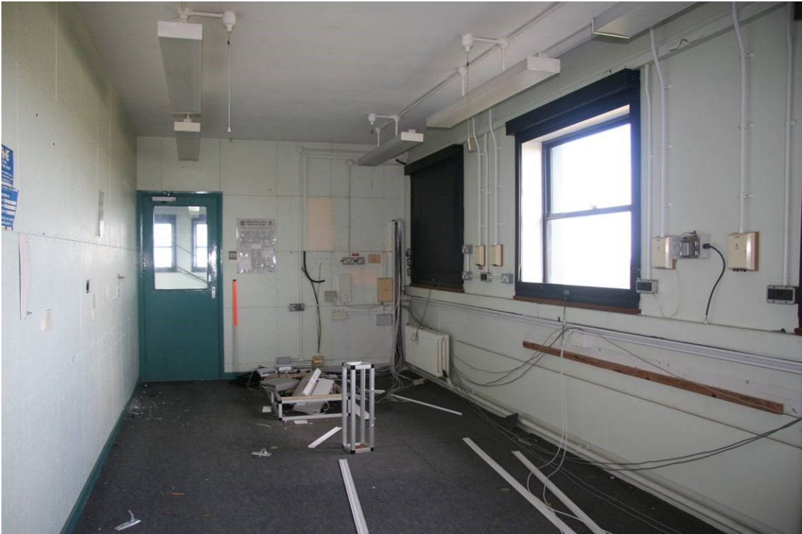
Fig 46 Met Office Teleprinter room within NW Wing, looking northwest
