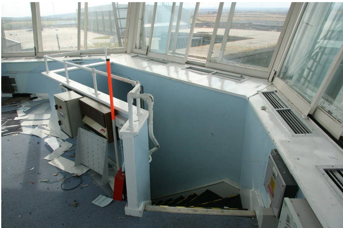
Fig 59 Access stairway into the Visual Control Room
