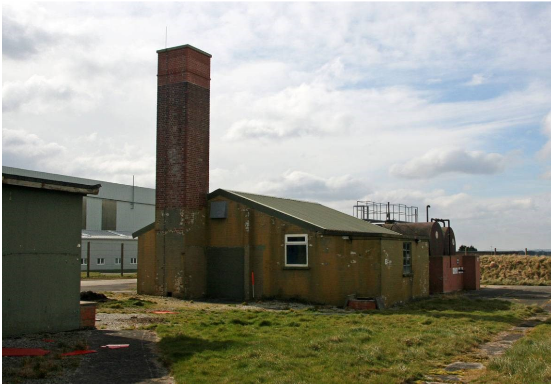
Fig 11 Boiler house, viewed from the northeast
