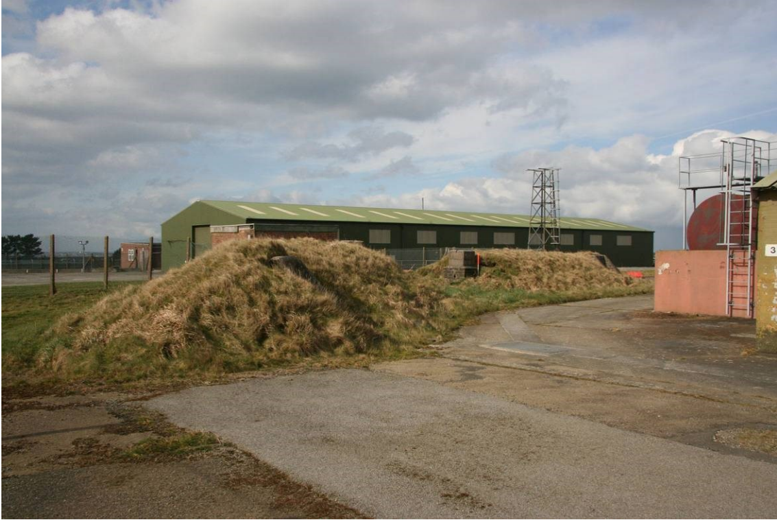
Fig 13 Two air raid shelters, situated south and west of the boiler house
