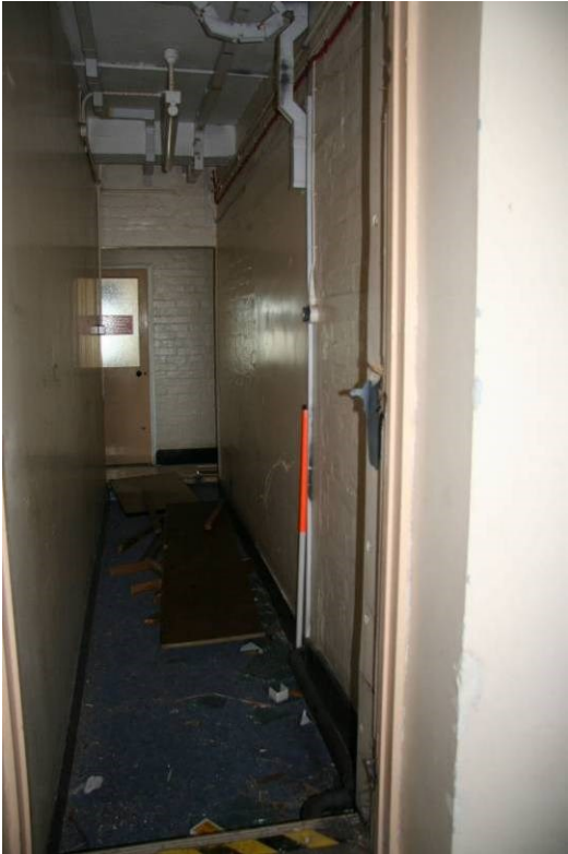
Fig 45 Corridor connecting original ATC tower to NW Wing
