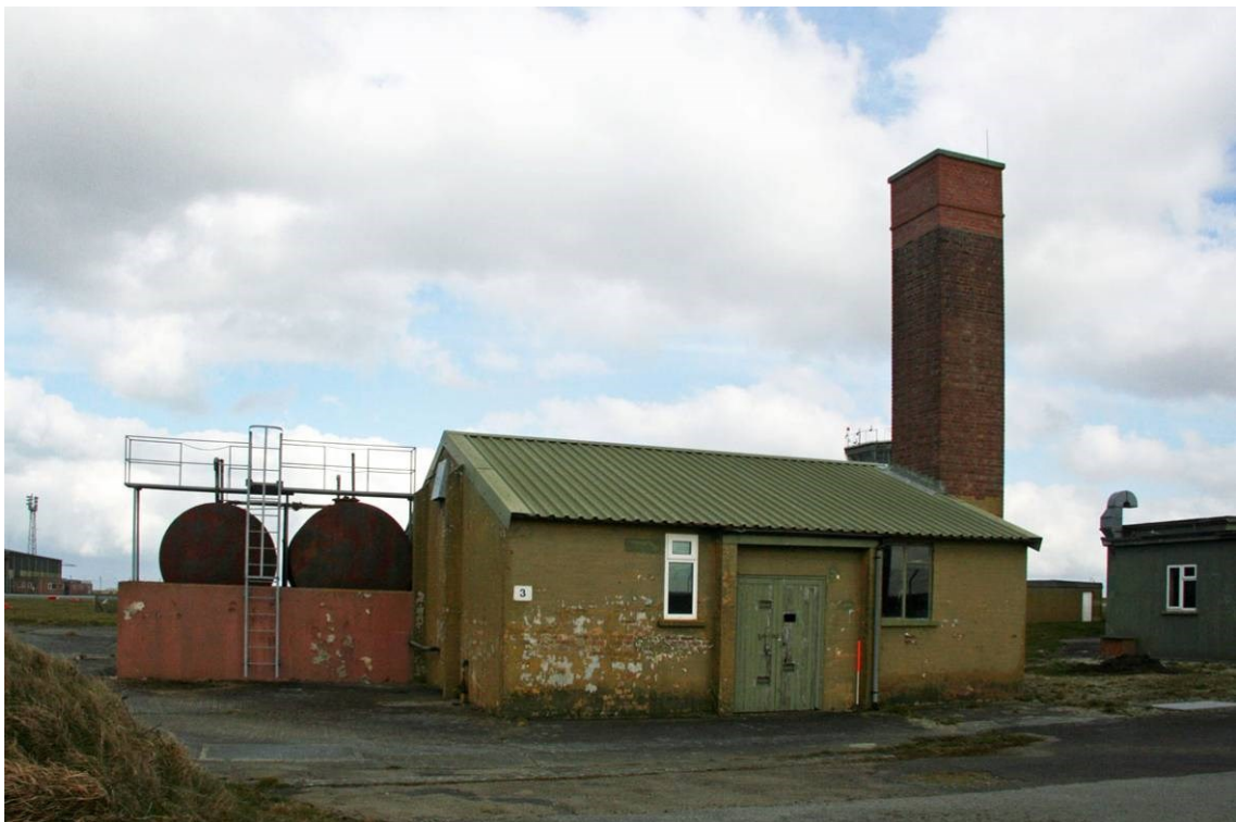
Fig 12 Boiler house, viewed from the south
