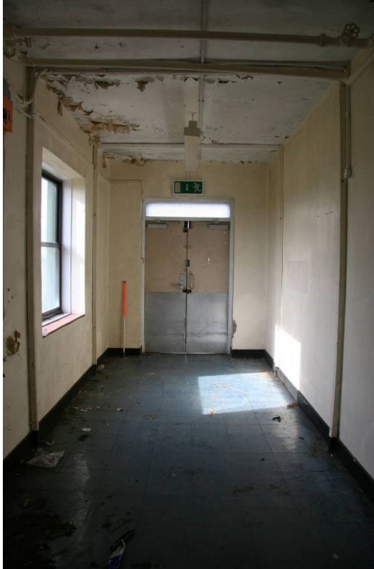
Fig 21 Entrance hall and external doors of ATC tower
