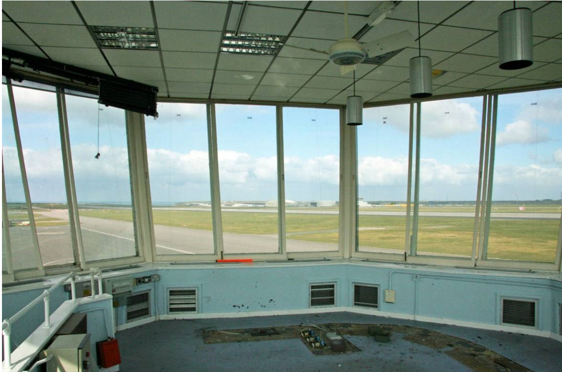
Fig 58 Interior of the Visual Control Room
