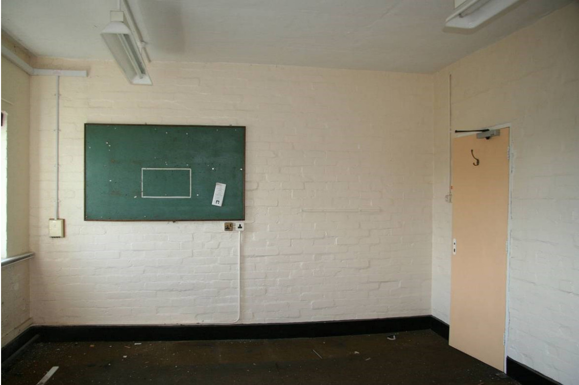
Fig 38 Met Office Admin room, looking southwest
