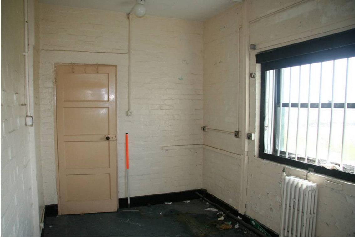
Fig 49 First floor Store Room, looking southeast Note the original panelled door
