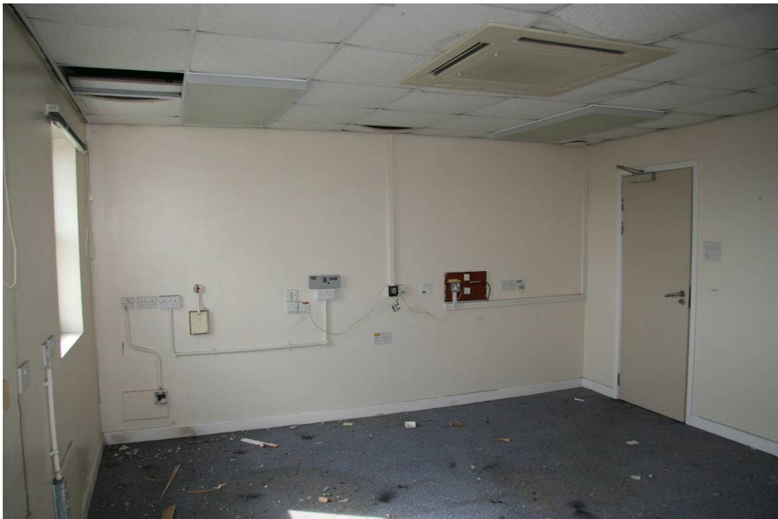
Fig 52 Principal Flight Operations Manager's room, looking west
