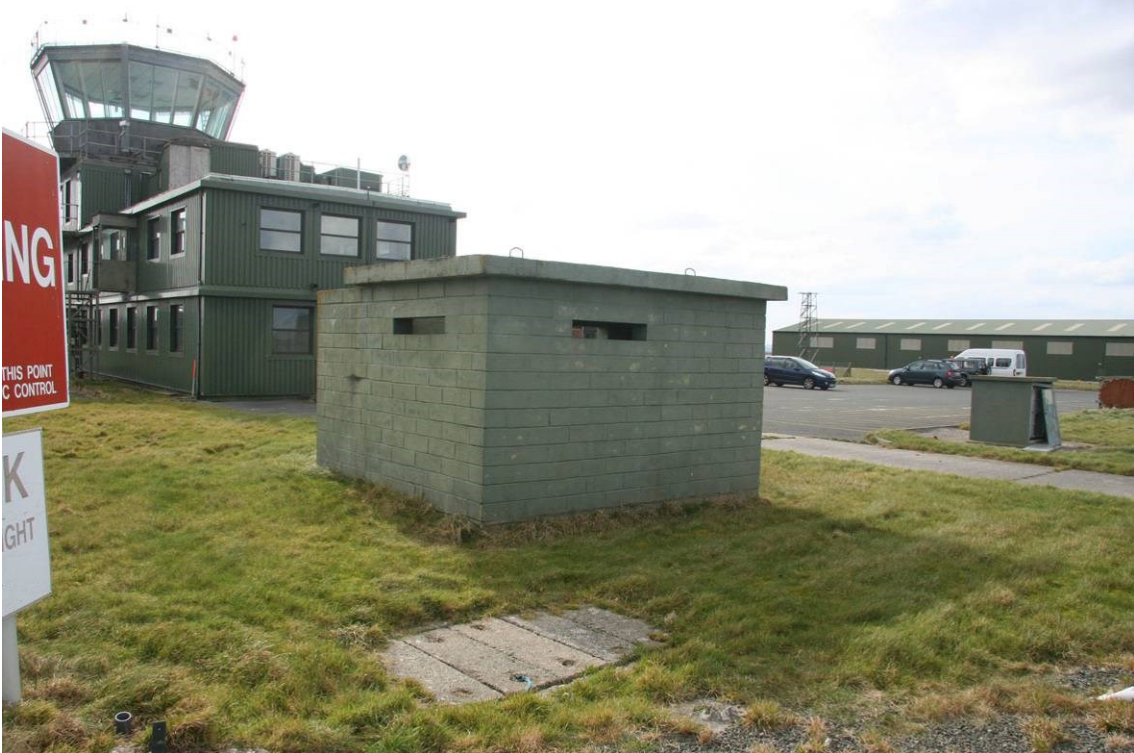
Fig 18 Pill box (and flare store, to the right), viewed from the north
