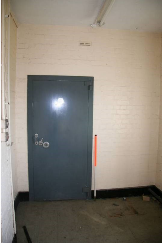
Fig 50 Store room and safe/strong-room on first floor, looking southeast
