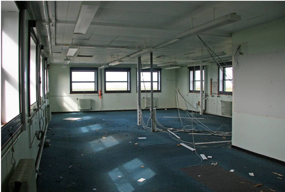
Fig 47 Met Office Forecasters' Room, looking northwest
