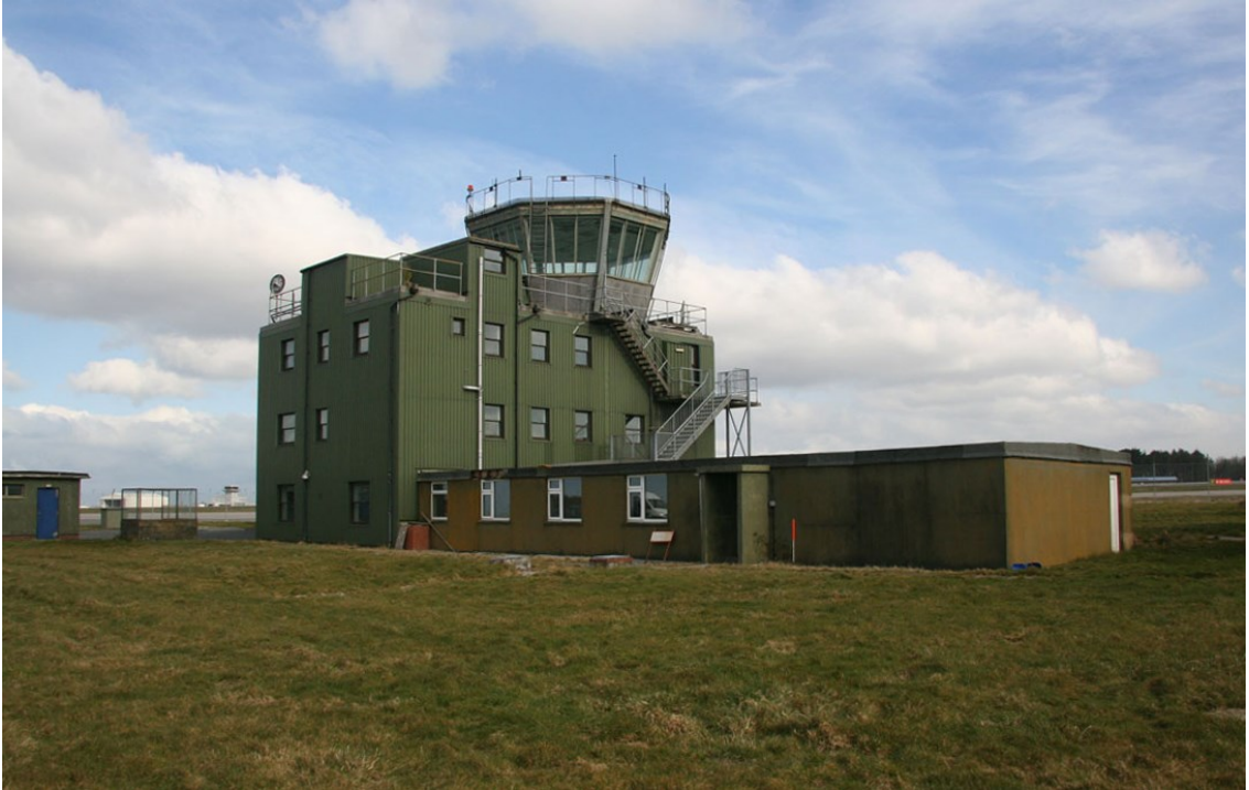
Fig 6 The former RAF ATC tower viewed from the south
