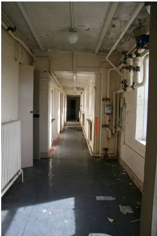
Fig 22 Entrance hall, looking into SE Wing (Seco range)
