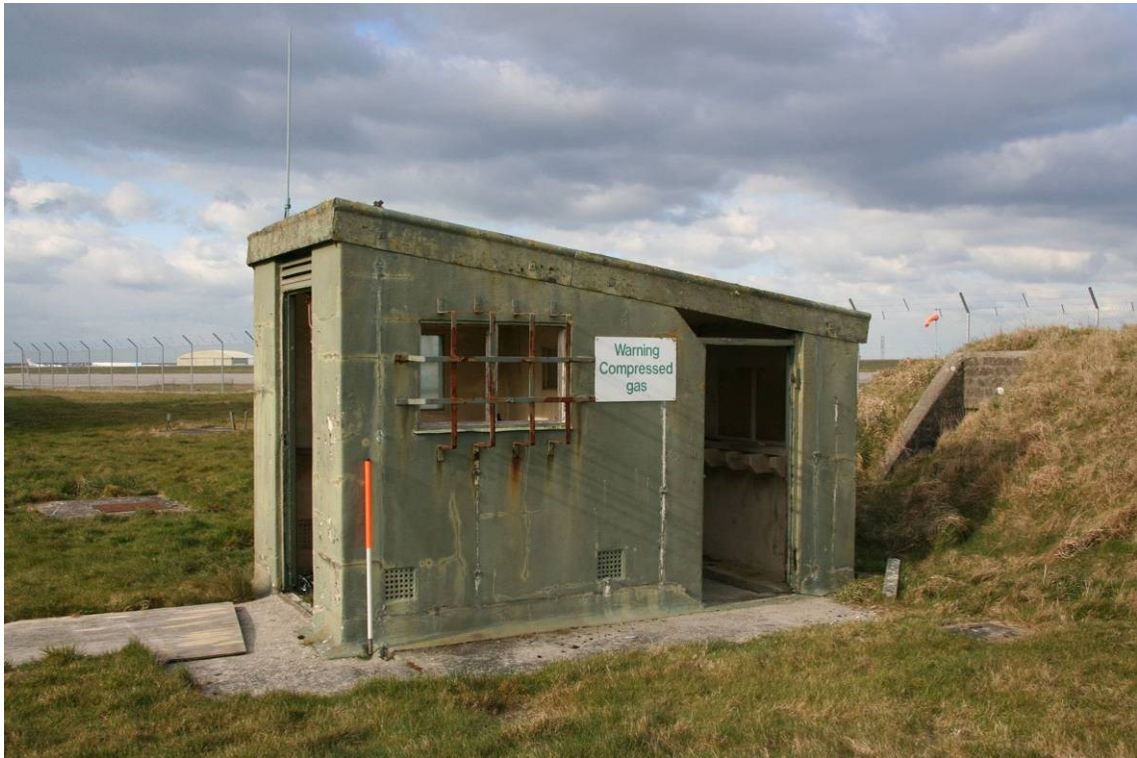
Fig 15 Gas store, viewed from the southeast
