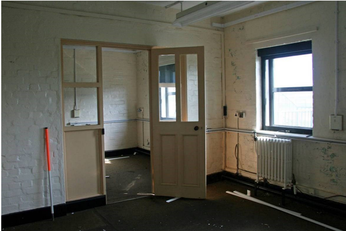
Fig 39 Met Office Admin room, looking east
