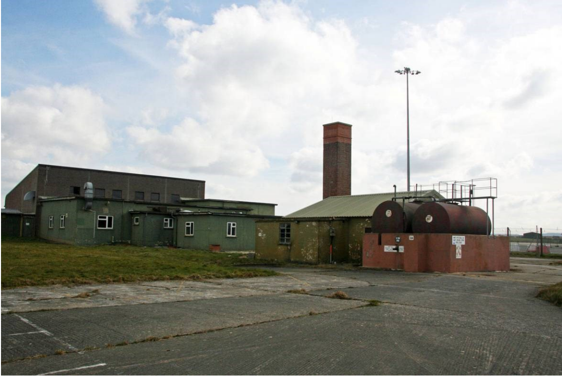
Fig 9 Rear of the fire station (left) and boiler house (right)
