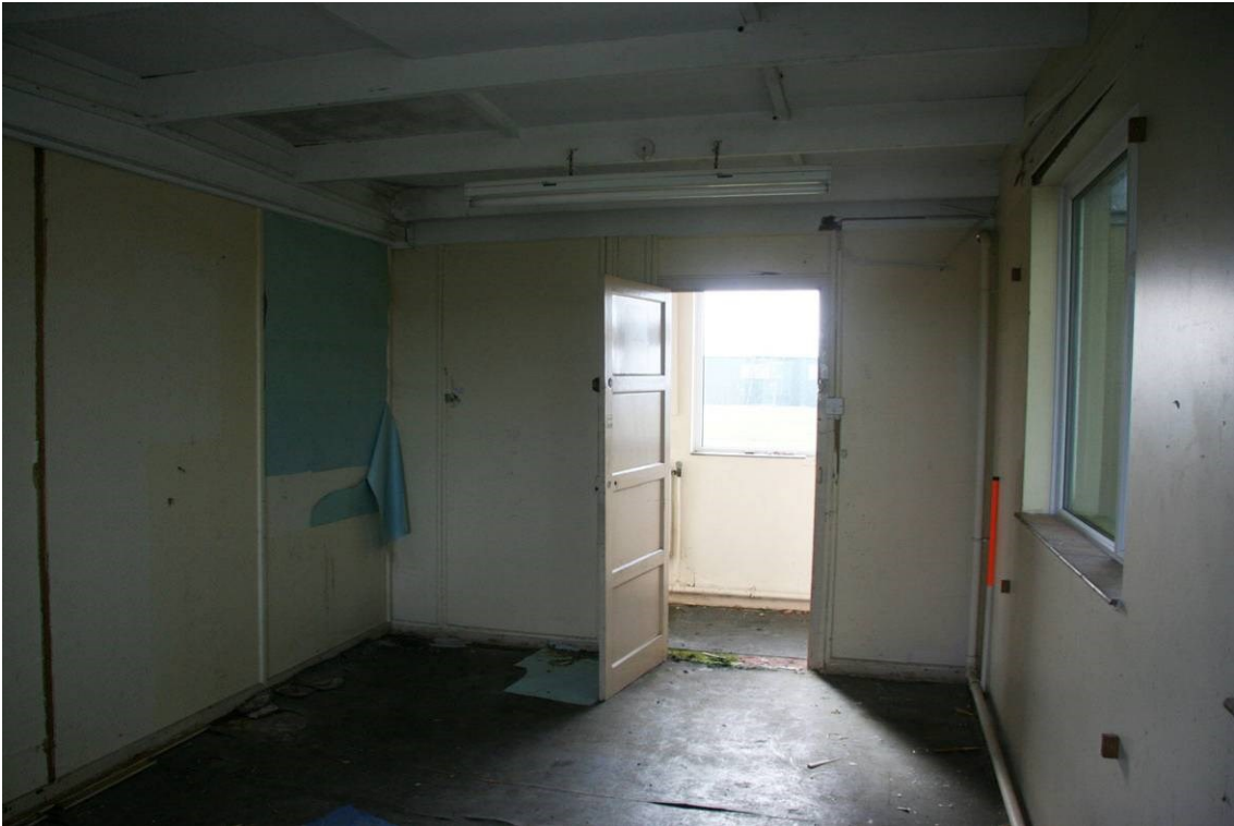
Fig 34 Unidentified room within the SE Wing Note the original panelled door
