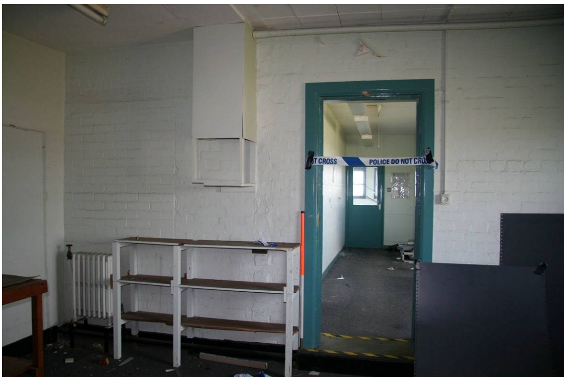
Fig 44 Met Office Records room, looking west and into NW Wing
