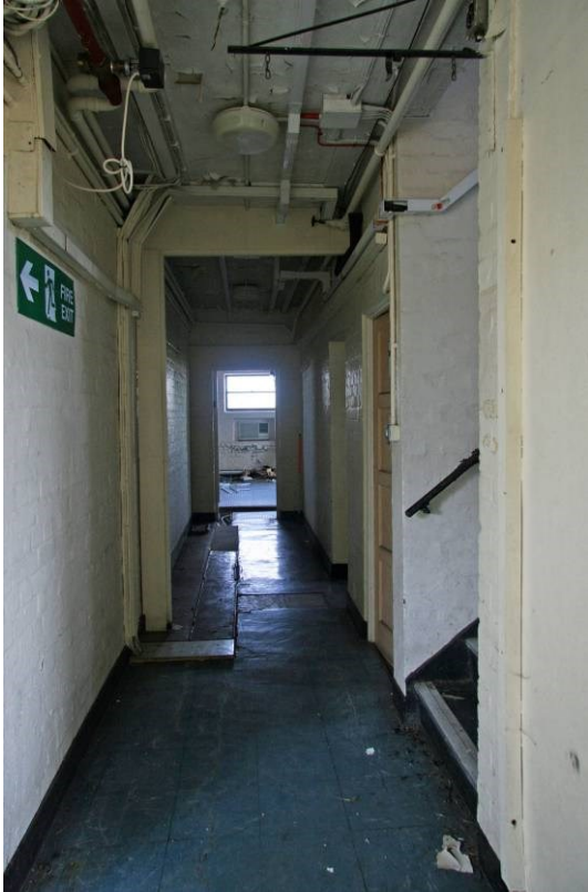
Fig 23 Ground floor corridor, with stairs to upper floors to right
