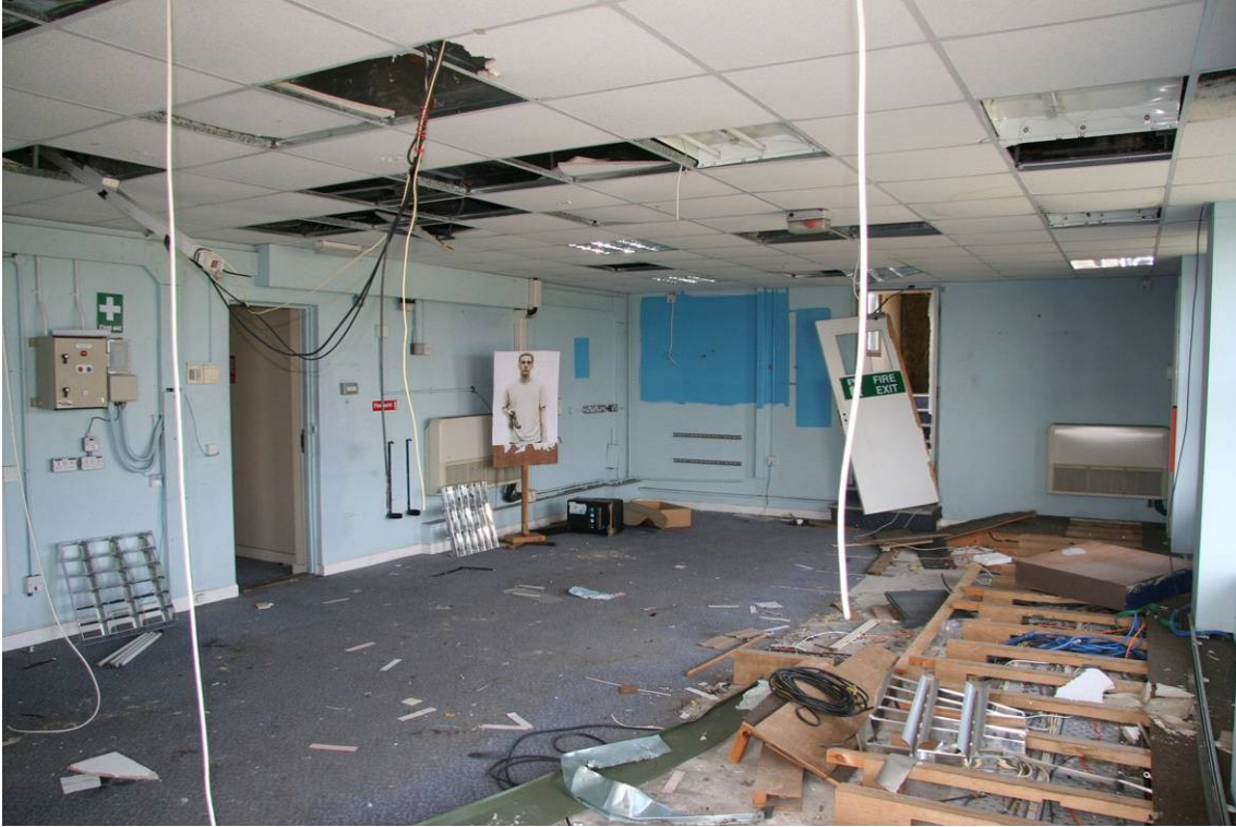
Fig 53 Radar Control Room, looking west
