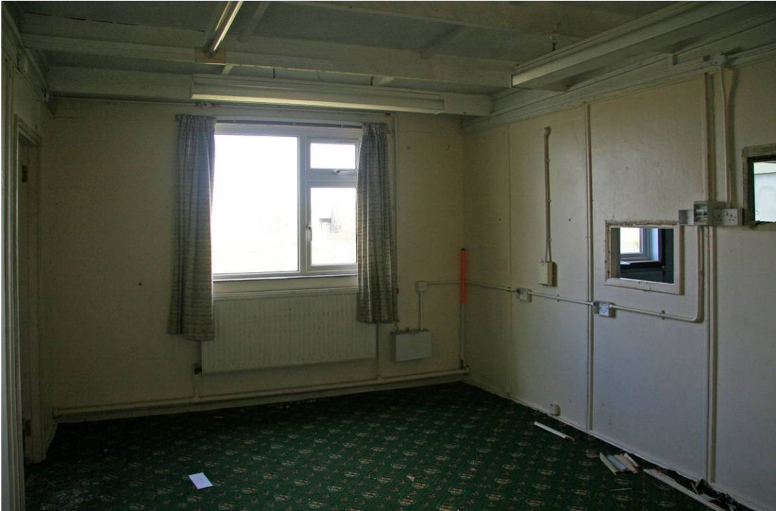
Fig 33 Unidentified room within the SE Wing
