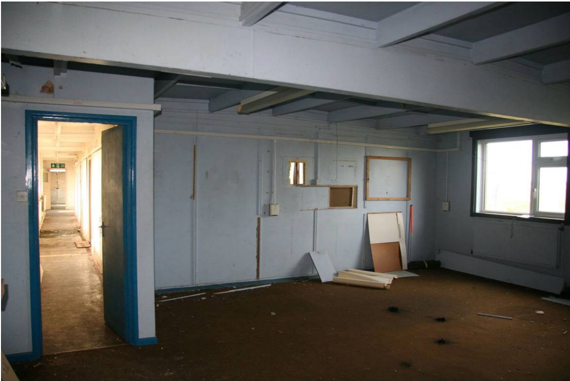
Fig 30 Corridor and unidentified room within the SE Wing (Seco buildings)
