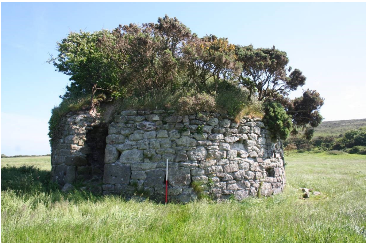
Fig 12 North elevation of kiln
