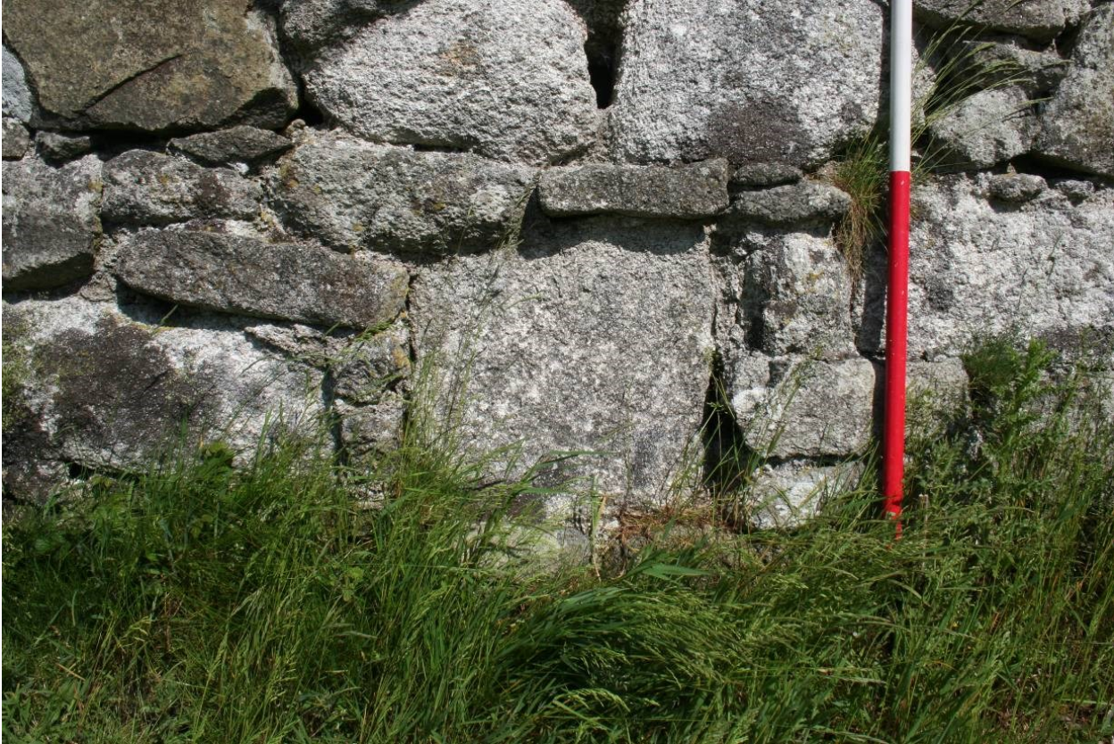
Fig 17 Possible blocked opening in west elevation of kiln
