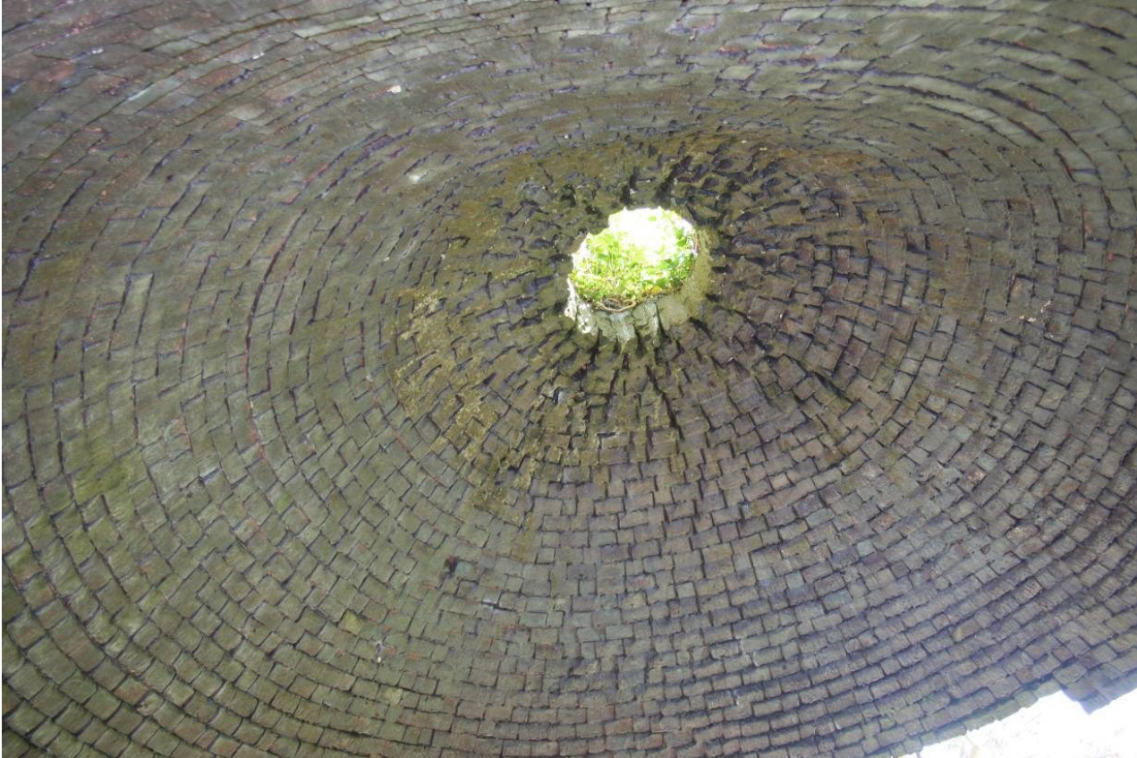
Fig 29 Interior of brick roof structure
