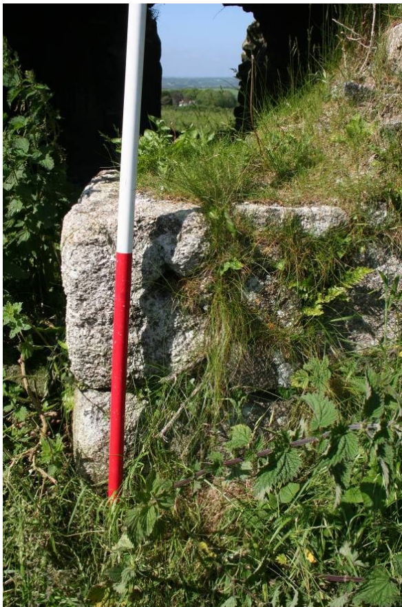
Fig 20 Remains of south jamb of former south-west loading door showing drill hole for fitting
