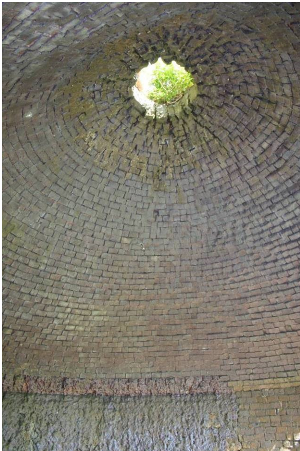
Fig 28 Interior of brick roof structure looking south
