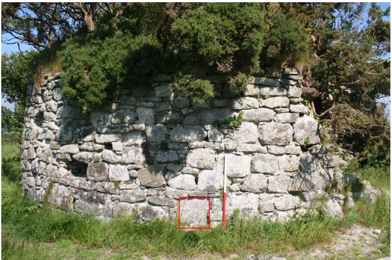
Fig 16 West elevation of kiln with red box showing possible blocked opening
