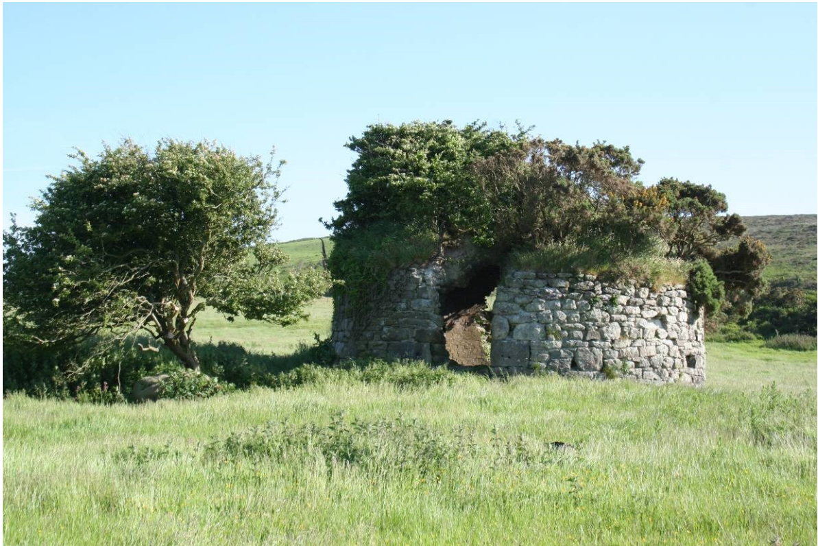
Fig 11 North-east elevation of kiln, its chimney once located in the area of the tree to the left
