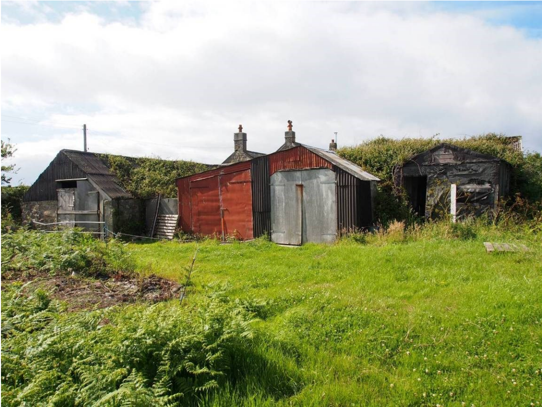
Fig 35 Southern side of the flower packing shed, showing adjoining structures
