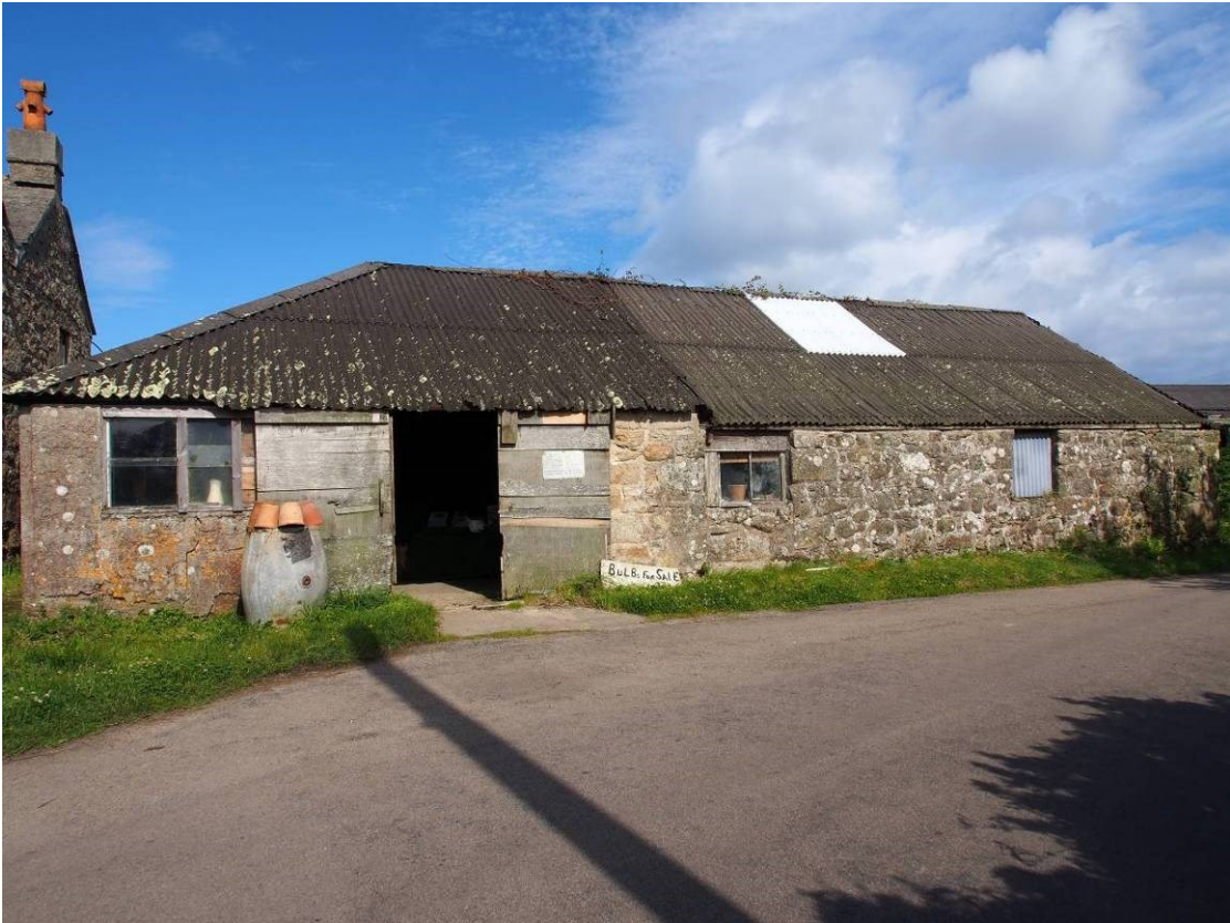
Fig 31 West (front) view of flower packing shed
