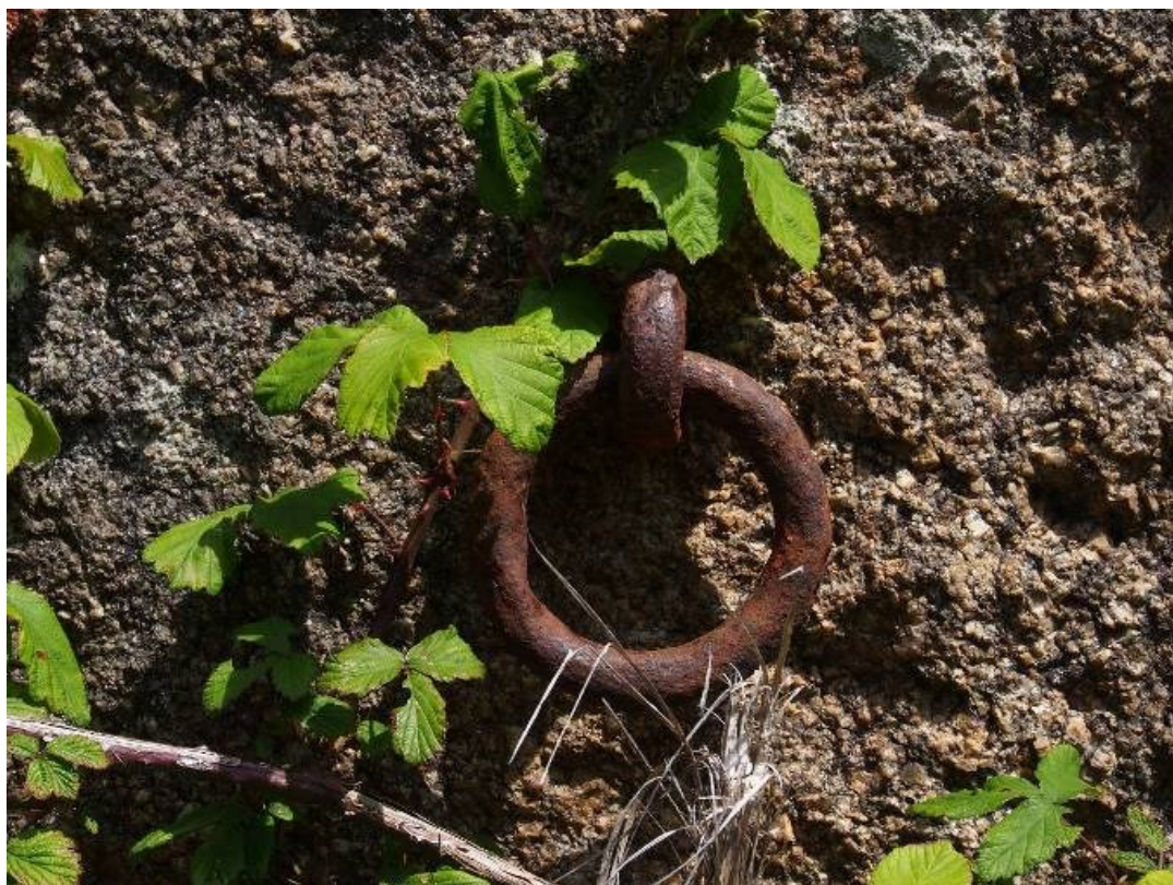
Fig 10 Iron tethering ring set into granite block on the front of the farmhouse
