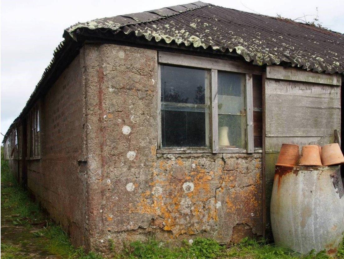
Fig 32 Shuttered concrete corner of flower packing shed, with round moulded detail
