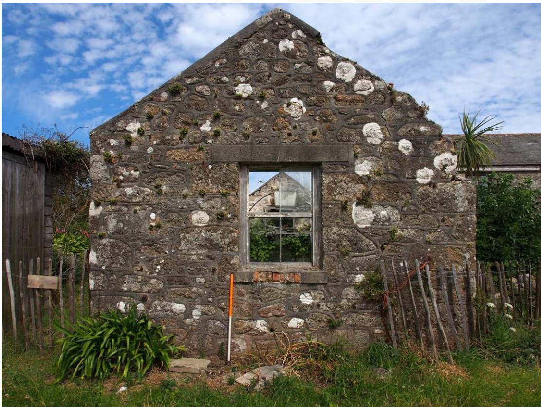
Fig 46 West gable of 'Fish house' or stable/outhouse
