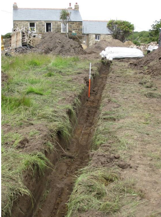
Fig 54 The southern soakway trench
