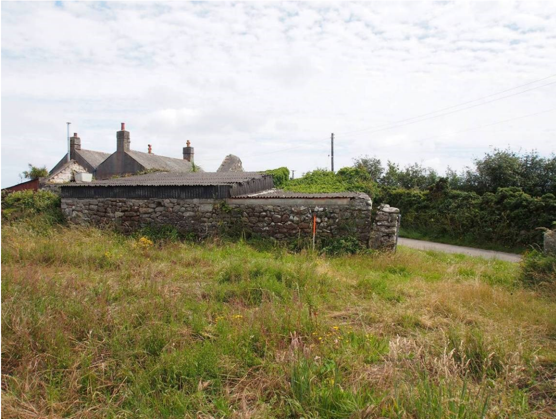
Fig 51 Rear of tractor shed and adjoining field and lane
