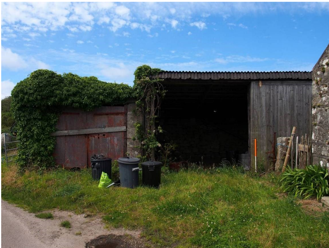
Fig 50 Front of tractor shed
