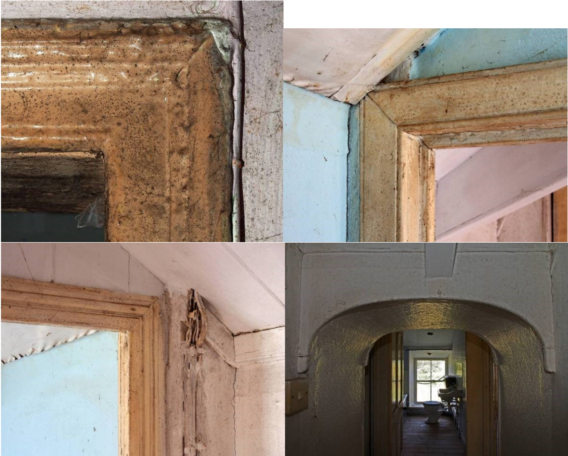
Fig 27 Examples of mouldings on architraves and stair corridor arch
