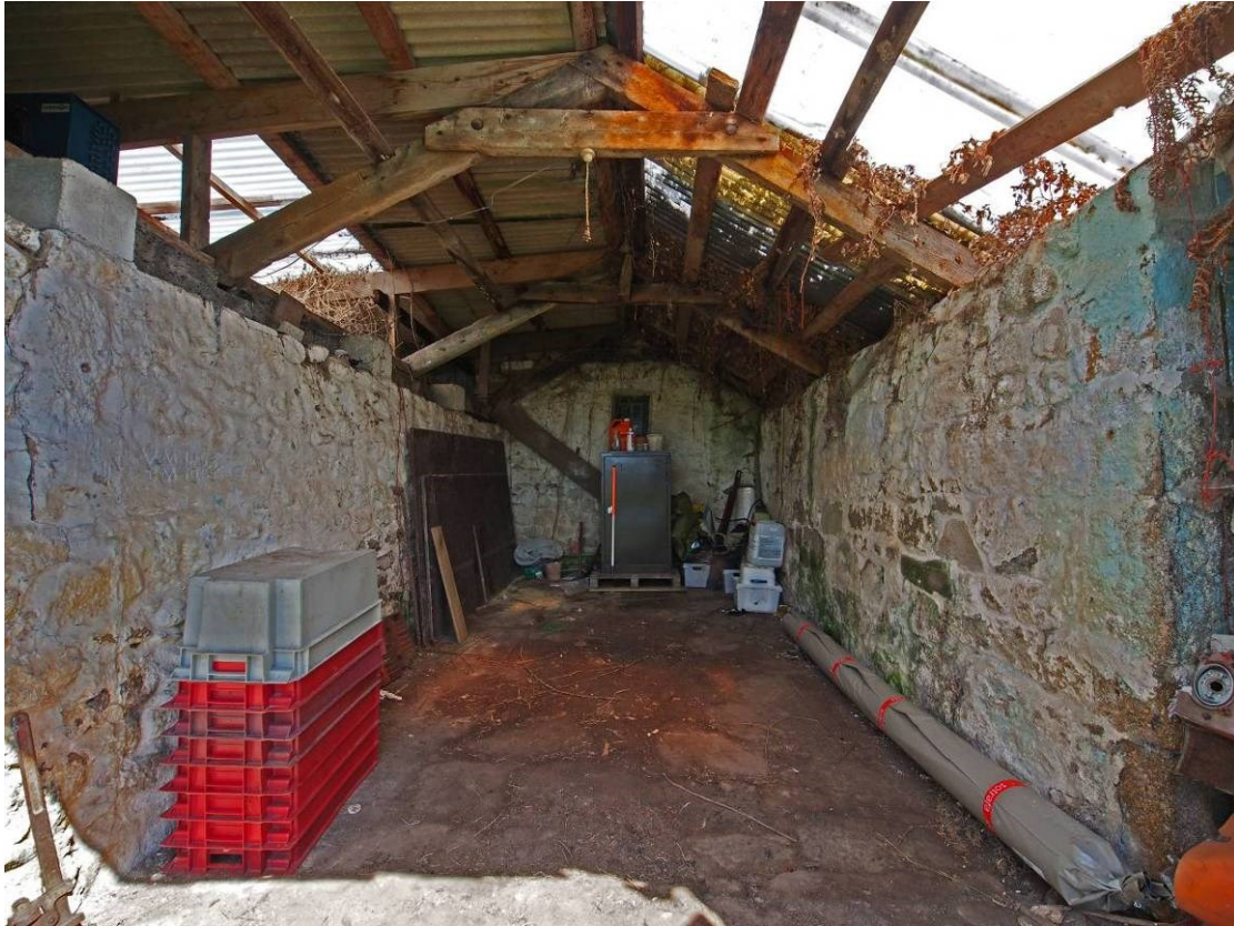
Fig 41 Former cart house showing stone flagged floor
