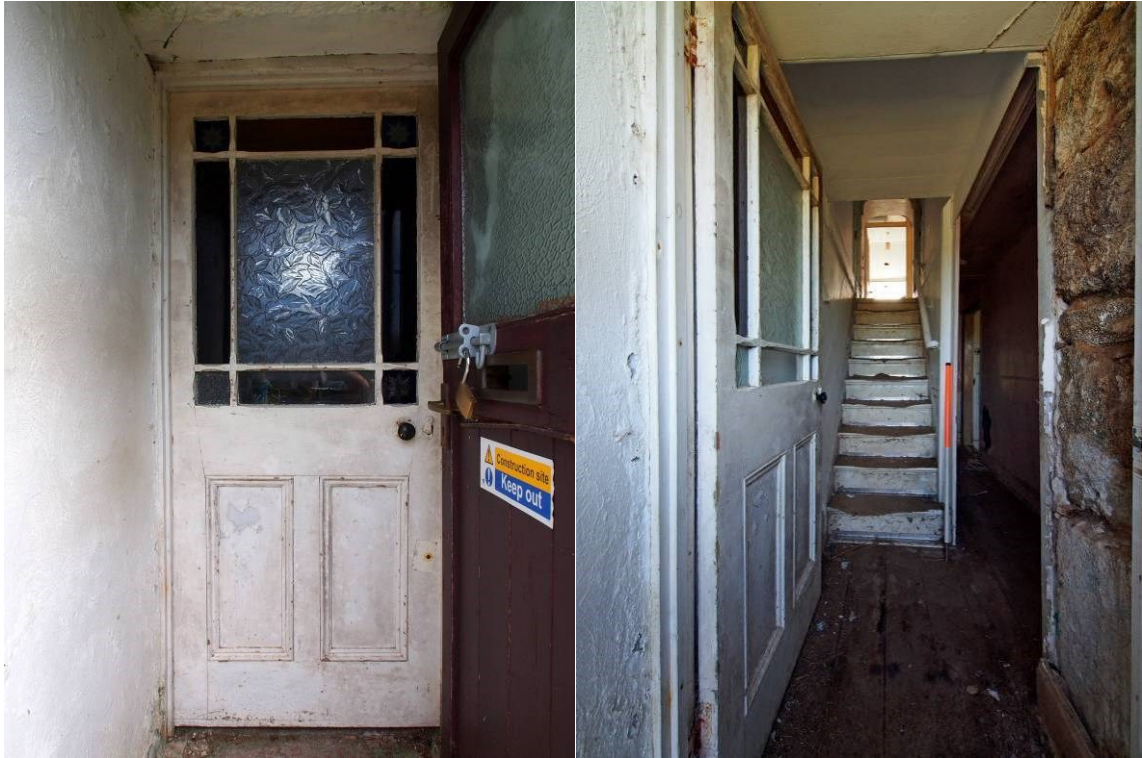
Fig 29 Glazed front door and original stairway in hall behind
