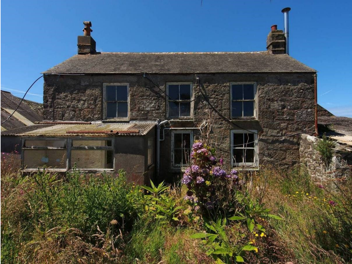
Fig 8 Rear of Borough farmhouse, with twentieth century blockwork conservatory to left
