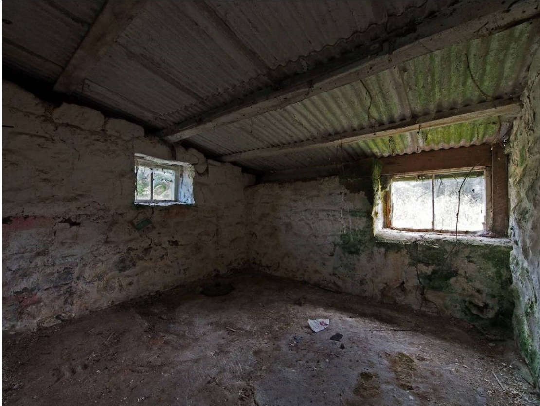
Fig 25 Former piggery or wash house
