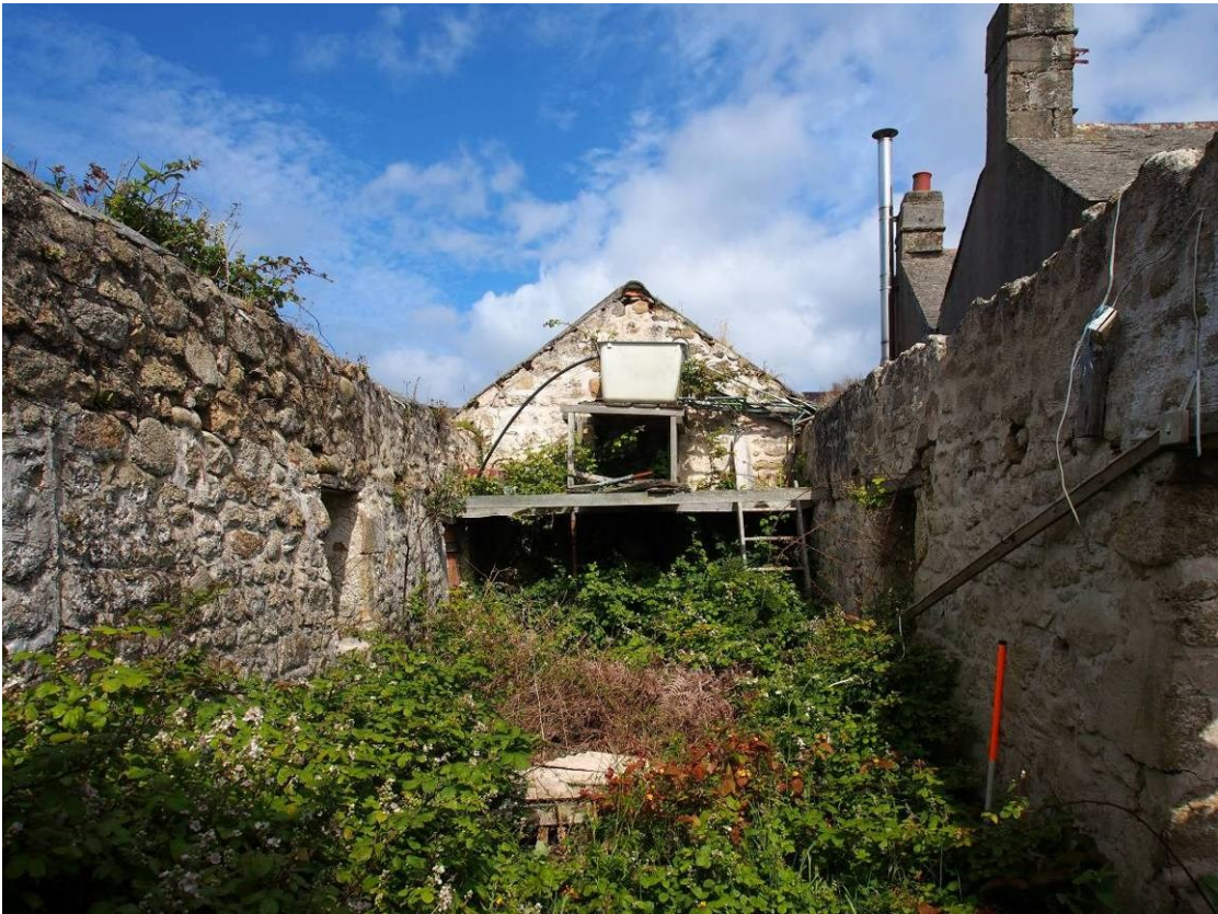
Fig 48 Interior of 'Fish house' showing water tank inside E gable
