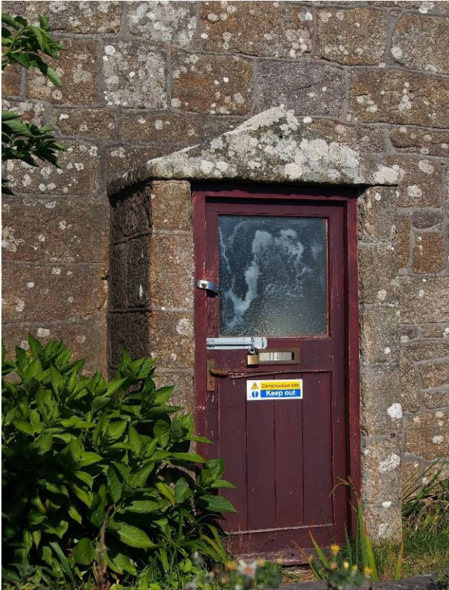
Fig 11 The probably unique granite ashlar and stone roofed front porch
