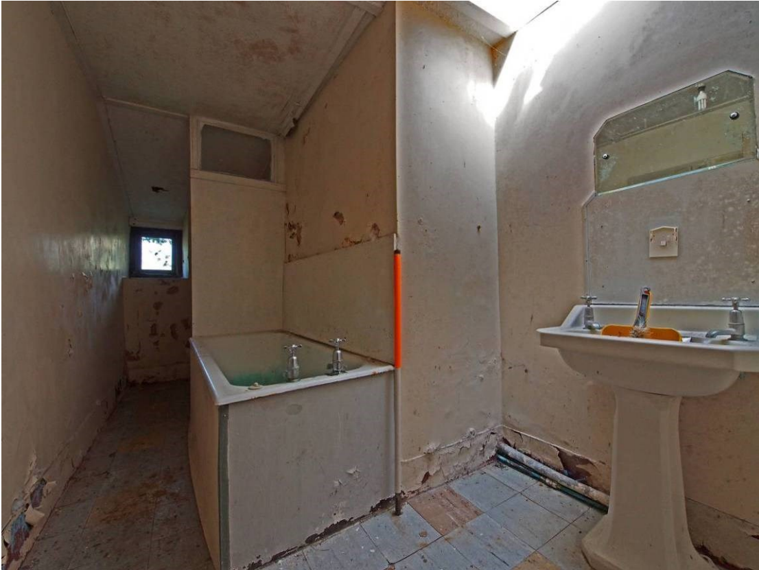
Fig 23 Bathroom in ground floor annexe
