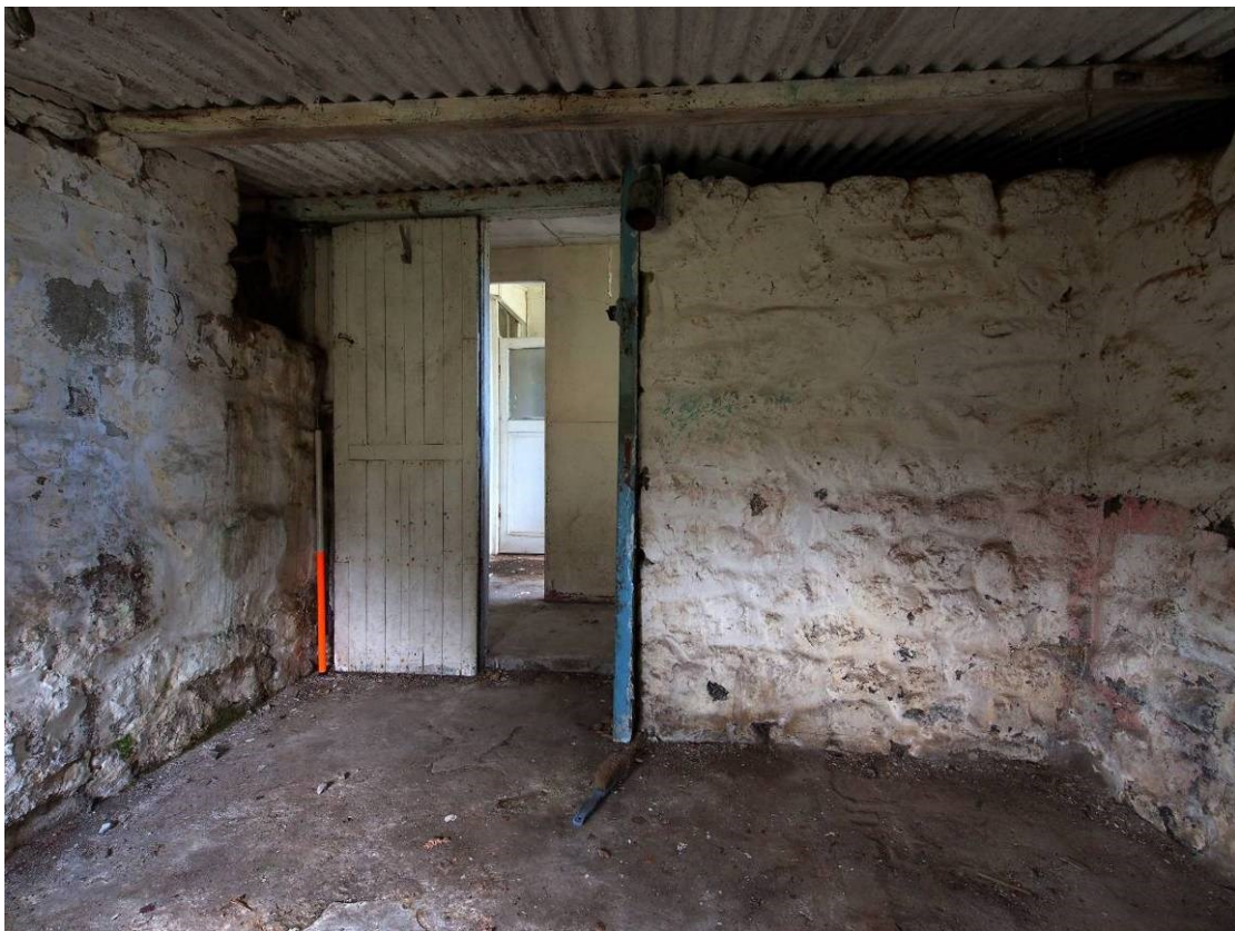
Fig 26 Doorway into former piggery or wash house
