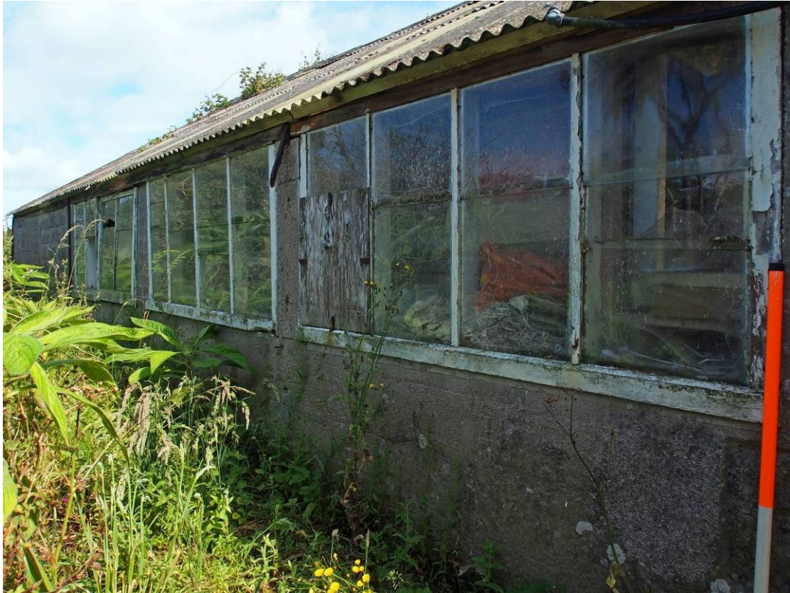
Fig 33 Window glazing in north wall of flower packing shed
