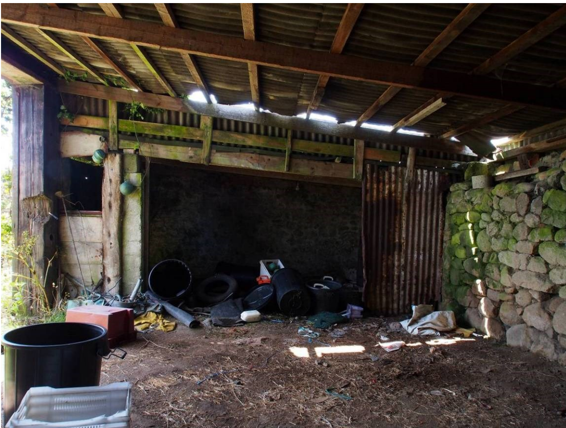
Fig 52 Interior of tractor shed
