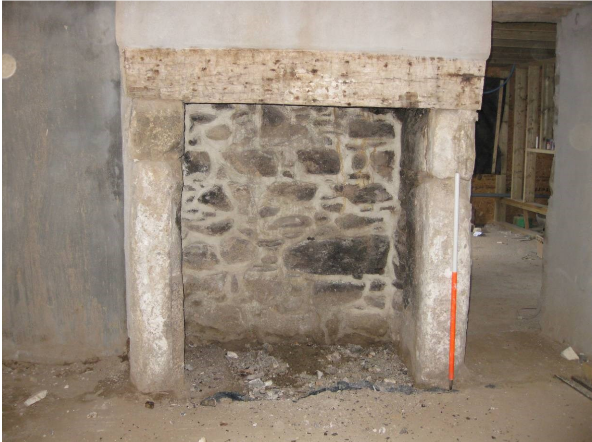
Fig 53 Fireplace revealed in the farmhouse during the watching brief
