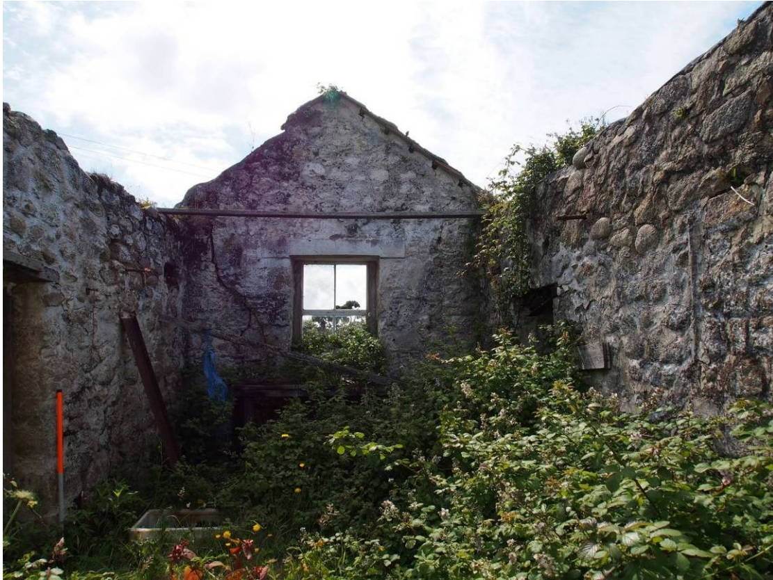
Fig 49 Interior of 'Fish house', looking W
