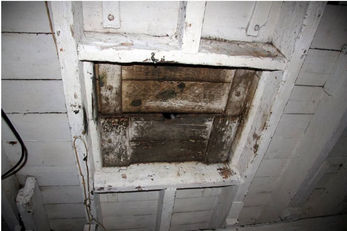
Fig 16 Trapdoor associated with a sack hoist, viewed from beneath
