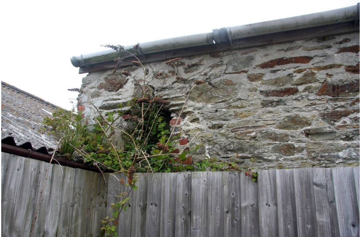
Fig 13 An inserted (and subsequently infilled) slot for a belt drive to machinery inside the building
