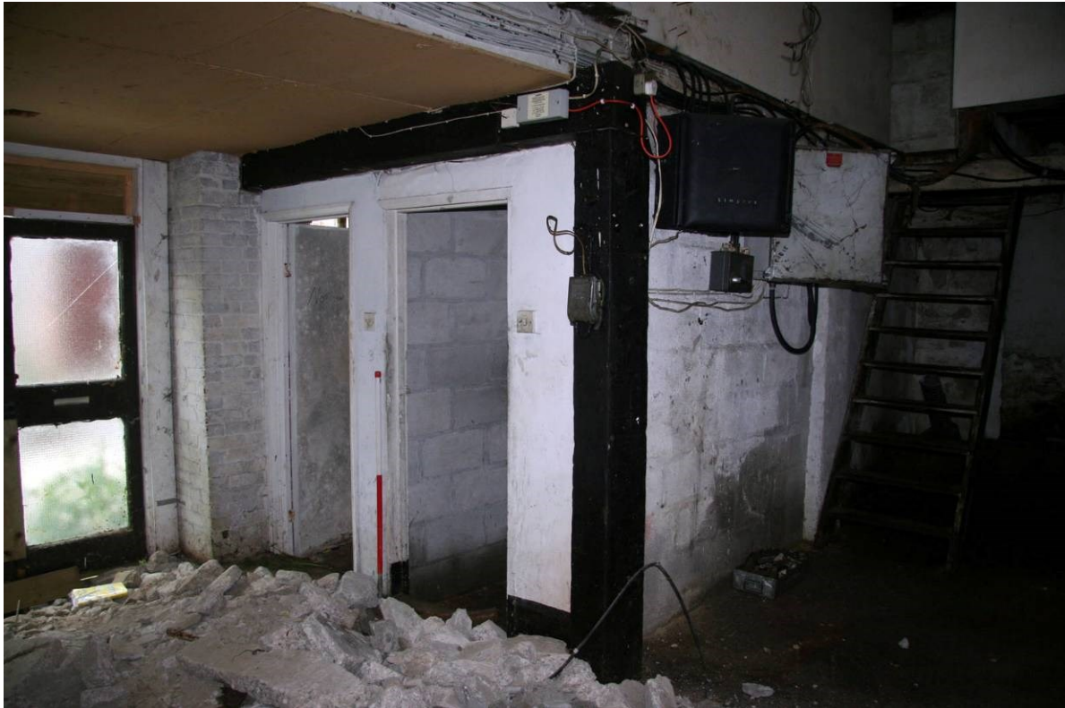
Fig 30 The upper floor of Building 2 was originally supported on central piers running the length of the building; a brick pier survives at the front of the building (towards left) and the horizontal black painted timber running into the pier is a truncated fragment of a principal floor beam
