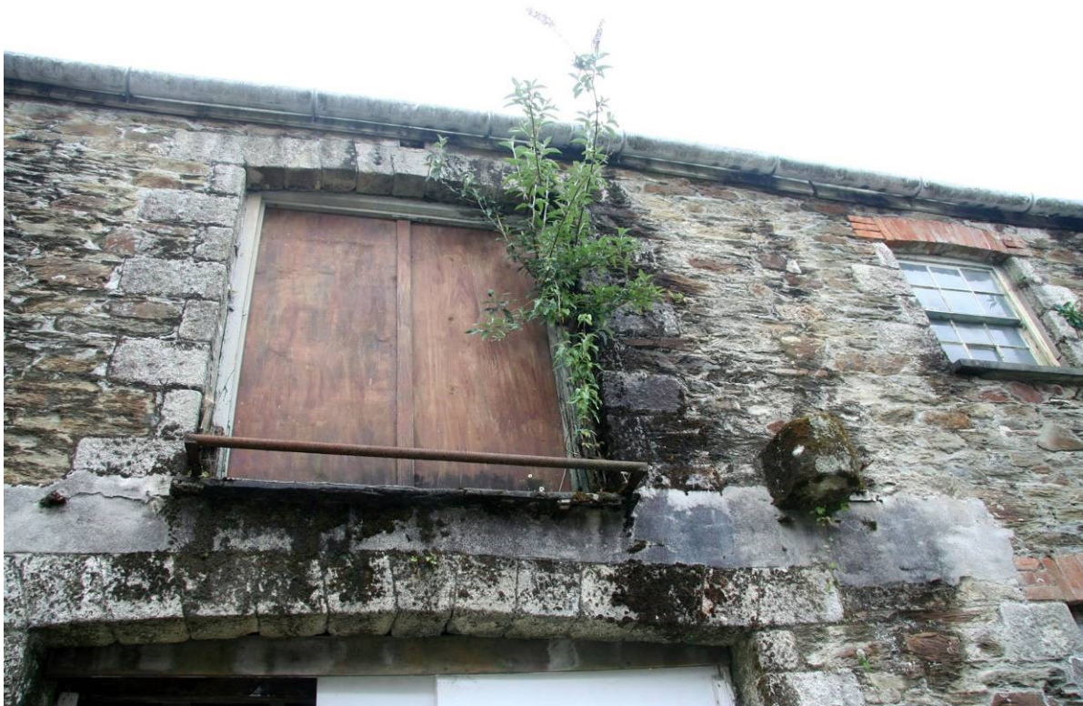
Fig 12 The front loading doors on Building 1 Note the projecting corbel to the right, probably to support a loading crane, and a slot for an overhead loading beam above the keystone of the upper arch
