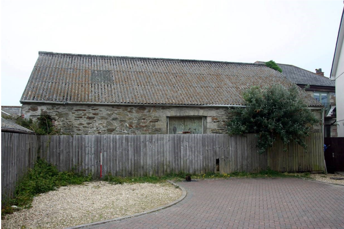
Fig 11 The rear of Building 1 showing central loading doors into the upper floor An inserted window lies behind the bush to the right, and at extreme left is a slot (now infilled) for a belt drive
