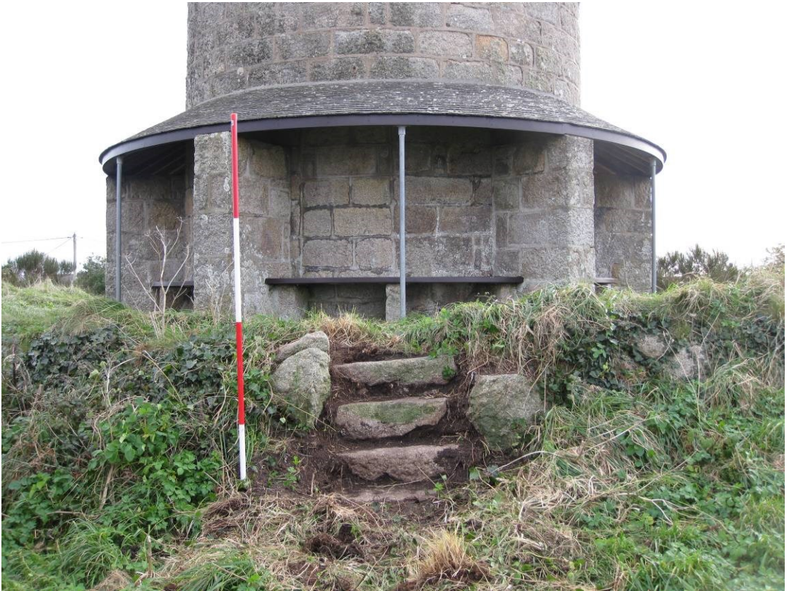
Fig 10 Steps to the north west and blocked doorway
