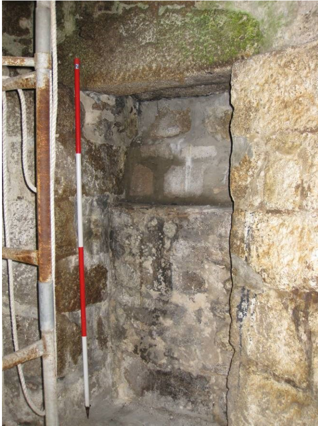
Fig 11 Interior view of blocked north west doorway
