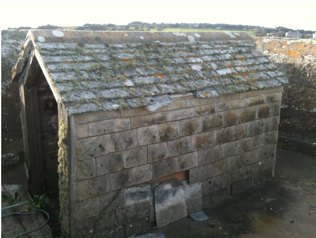
Fig 12 Shed on roof plinth, now removed
