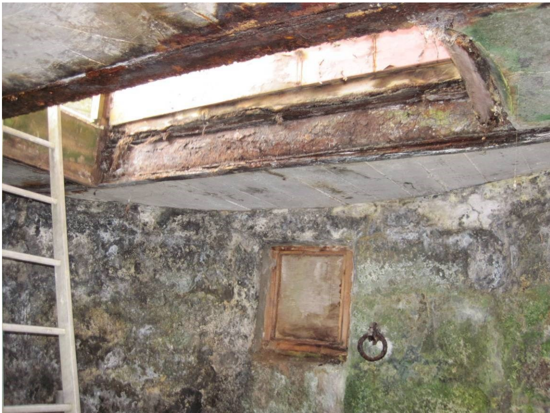
Fig 16 Iron ring and second floor south west window opening
