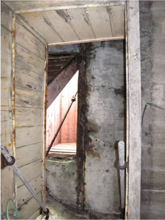
Fig 14 Vertical view of stairwells and concrete roof
