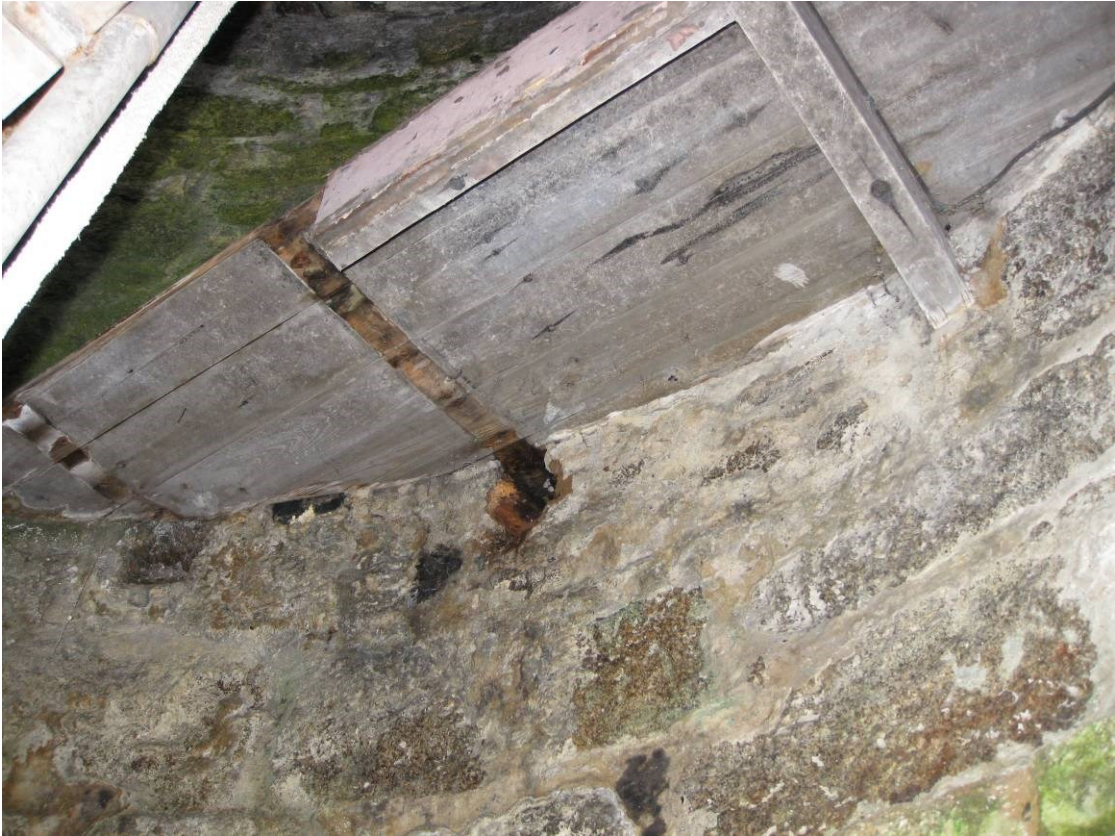
Fig 13 Wooden floor to first storey, now replaced
