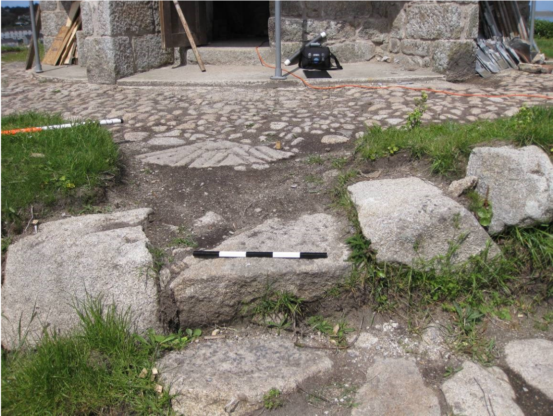
Fig 9 Millstone in surround and steps to the south east
