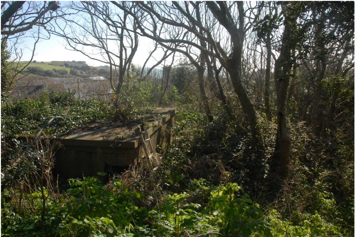
Fig 31 The concrete water tank on top of the castle mound
