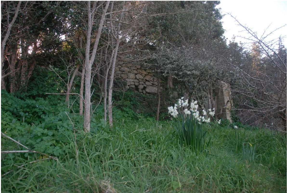
Fig 19 The surviving walling on the northern side of the castle mound
