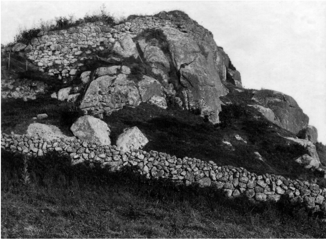
Fig 9 A late 19 th century Gibson view of the Ennor Castle site from the west clearly showing the remains of the castle walling, and the absence of trees on the site (Image supplied by kind permission of the Isles of Scilly Museum)
