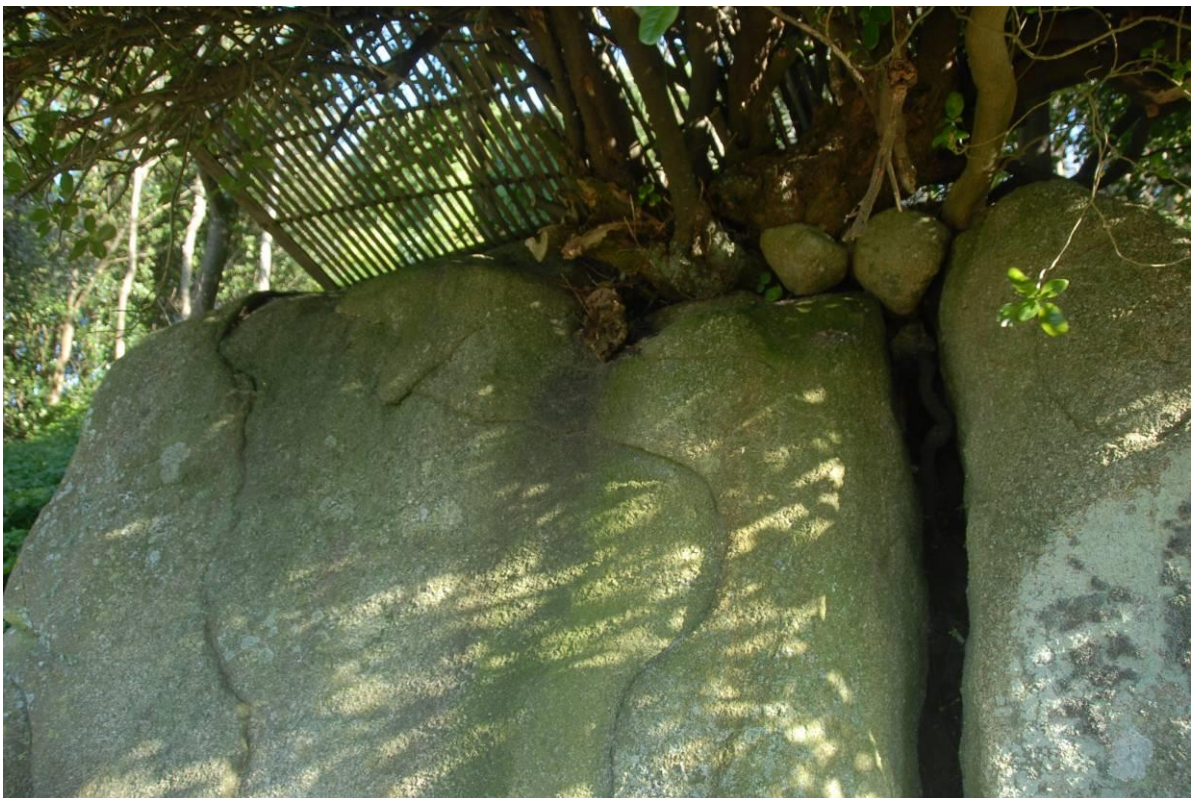
Fig 32 The roots of a Tamarisk which have taken hold in a boulder on site
