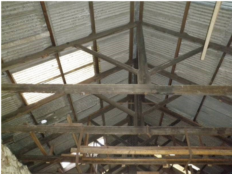
Fig 42 Building 7a phase 2 king post trusses
