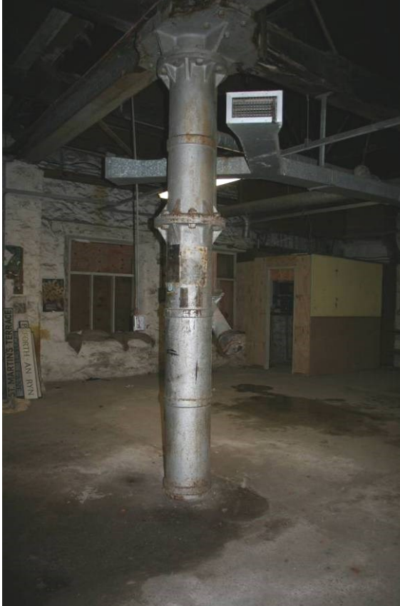
Fig 44 Building 7b and 7c interior showing cast-iron pillar bearing the name F Bartle and Sons (Carn Brea) supporting the roof valley
