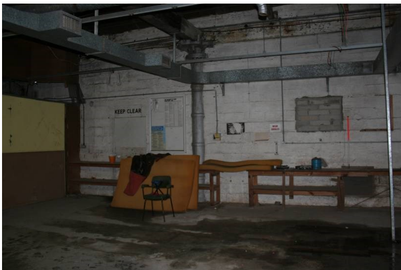
Fig 43 Building 7b interior showing cast-iron pillar supporting the roof valley between 7a and 7b along with inserted concrete block-built wall
