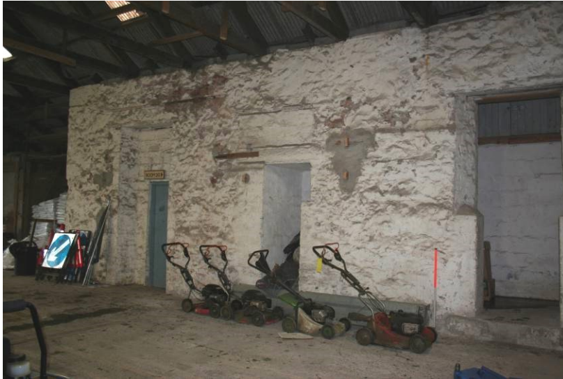
Fig 41 Building 7a interior showing altered phase 2 window openings in east wall
