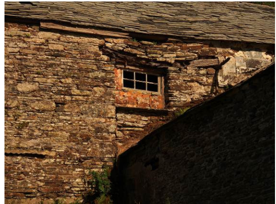
Fig 27 Former threshing-floor doorway, blocked by addition of horse-engine house roof
