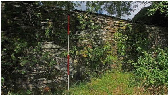
Fig 13 Barn 2 from south
