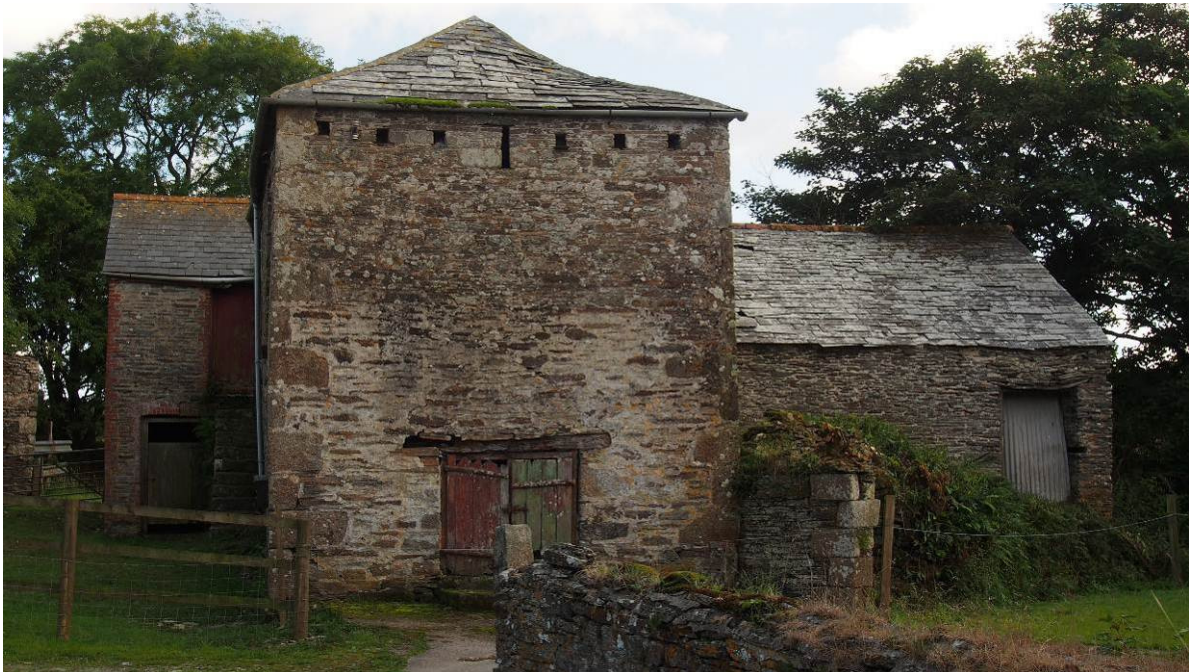
Fig 22 Barn 1 NNW end with goose-house doorway, and horse-engine house on right
