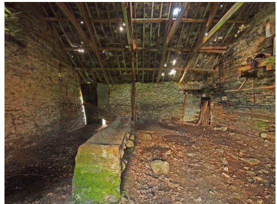
Fig 42 Horse-engine house from SSE
