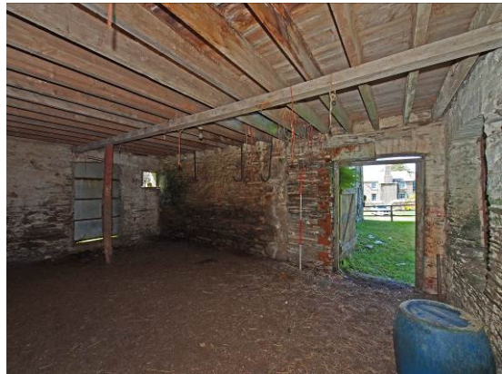
Fig 34 Later cow-house interior from SE
