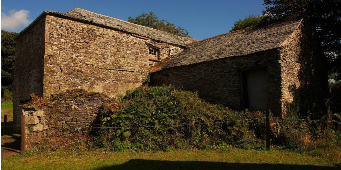
Fig 24 Barn 1 and adjoining horse-engine house from NW
