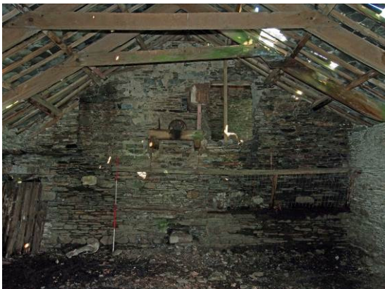
Fig 40 Barn 2 rear wall adapted when horse-engine house added
