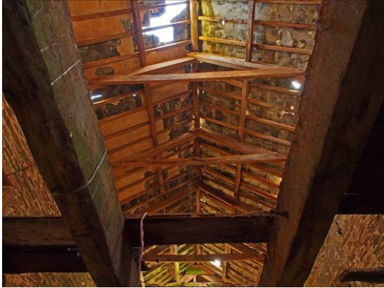
Fig 38 Barn 1 roof from cow-house
