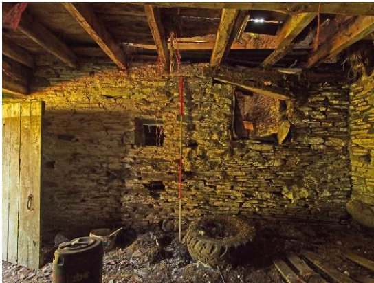
Fig 30 Cow-house interior from NNW
