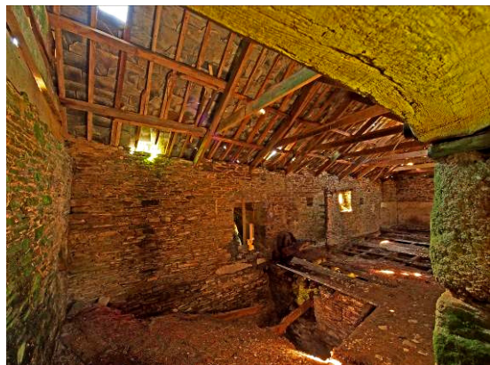
Fig 36 Barn 1 loft from SE
