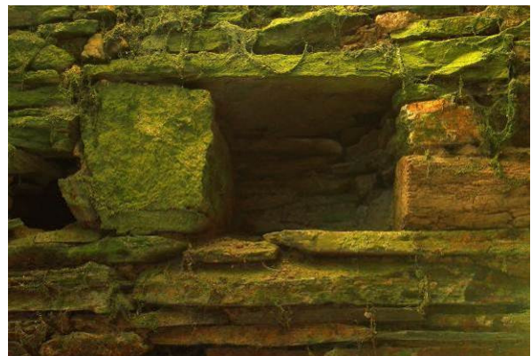
Fig 20 Barn 2: beam socket in front wall
