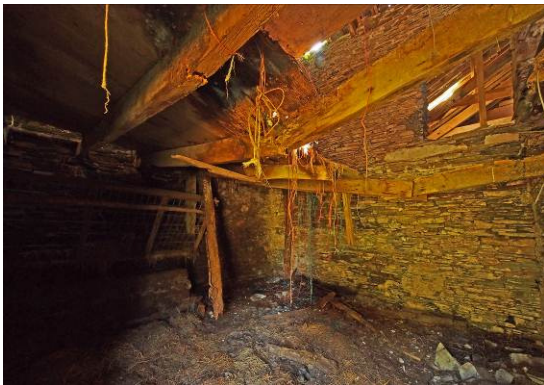
Fig 31 Loose-box interior from SSE
