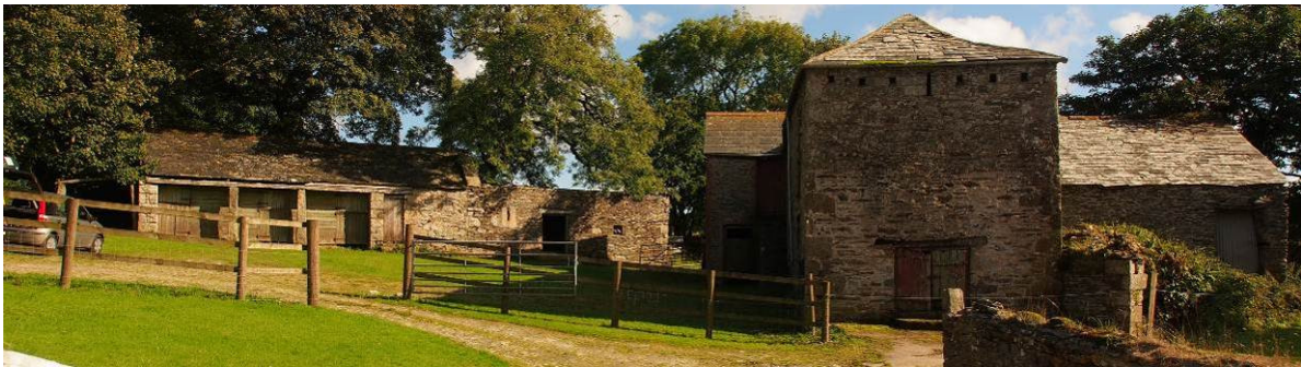
Fig 10 Subject buildings from NW: Barn 1 (right) and Barn 2 (left)
