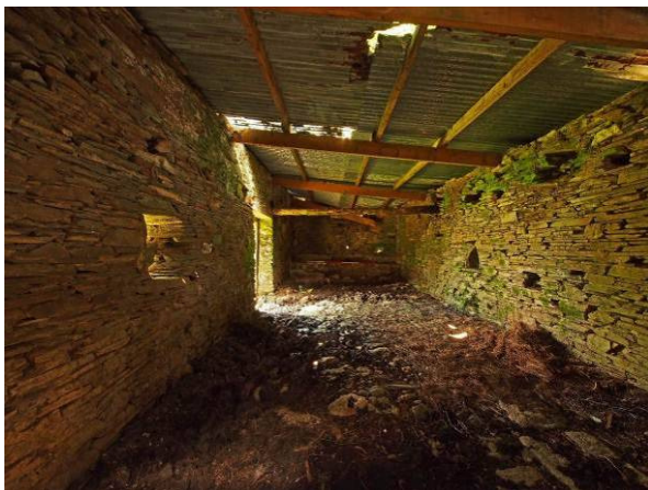
Fig 15 Barn 2 interior from SW
