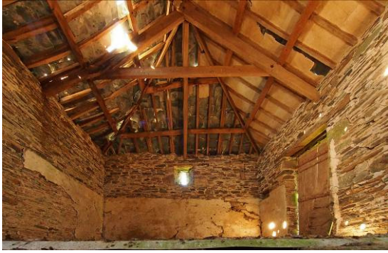
Fig 37 Barn 1 loft from SSE
