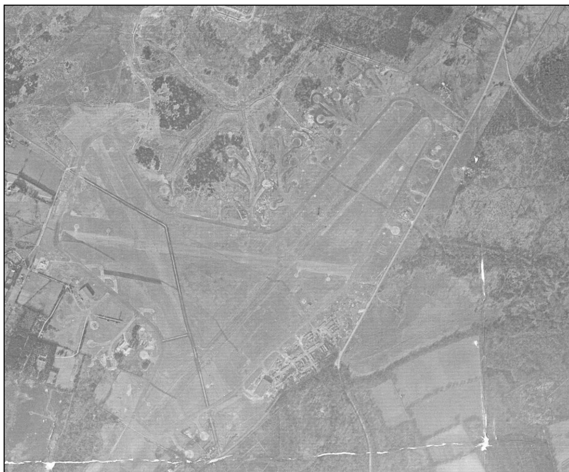
Figure 68. Holmsley South Second World War military airfield. The runways appear to have been partially camouflaged on this photograph taken in 1944. (MKM4460) Photograph: US/7PH/GP/LOC231 Frame 5001 15 th Mar 1944. English Heritage USAAF Photography
