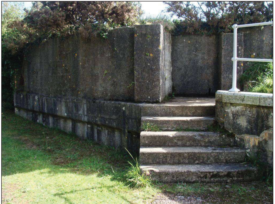
Figure 5: View of blocked rear access to infilled gun emplacement (facing SE)
