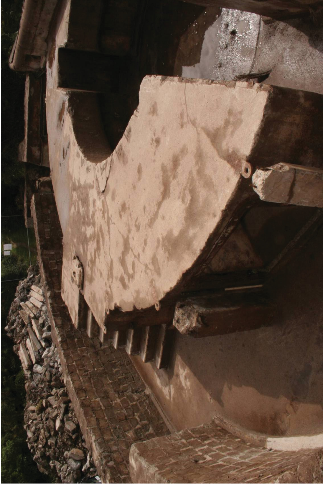
Fig 26 Store 3 (f), steps (l), and gun pit (r), facing north east (1m scale)
