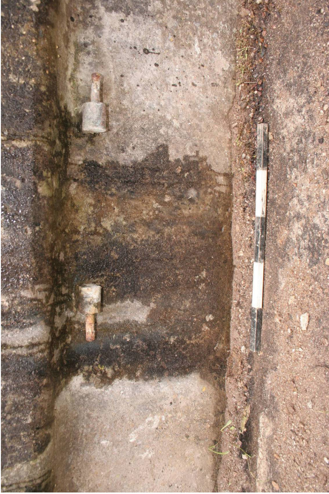
Fig 31 Fixings for fold-down benches on northern exterior wall, facing south (0.5m scale)
