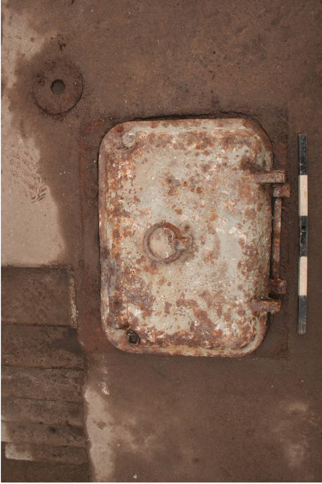
Fig 20 Shell hoist with cover, vertical (0.5m scale)
