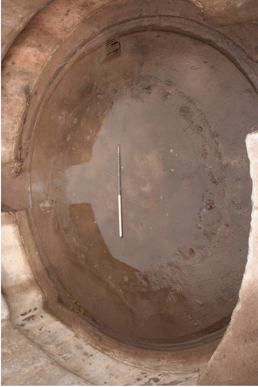
Fig 29 Gun pit, facing west showing remains of gun pedestal mounting bolts (1m scale)
