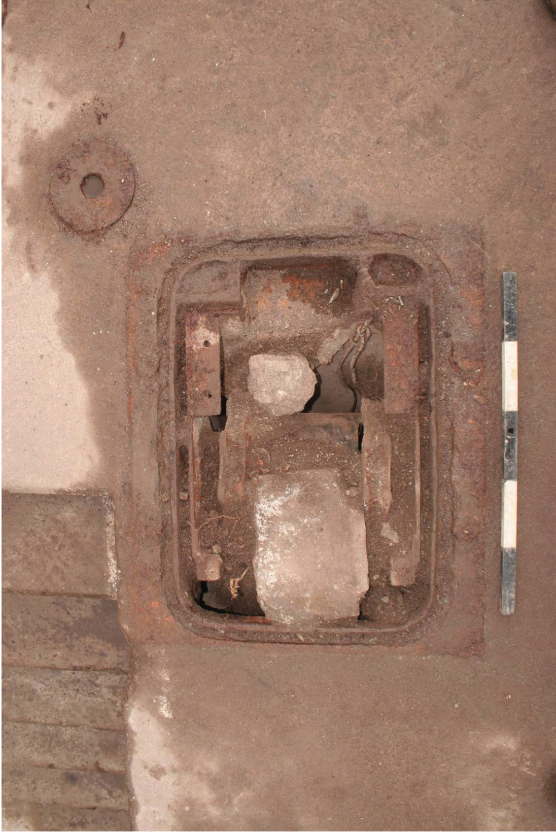
Fig 21 Shell hoist without cover, vertical (0.5m scale)
