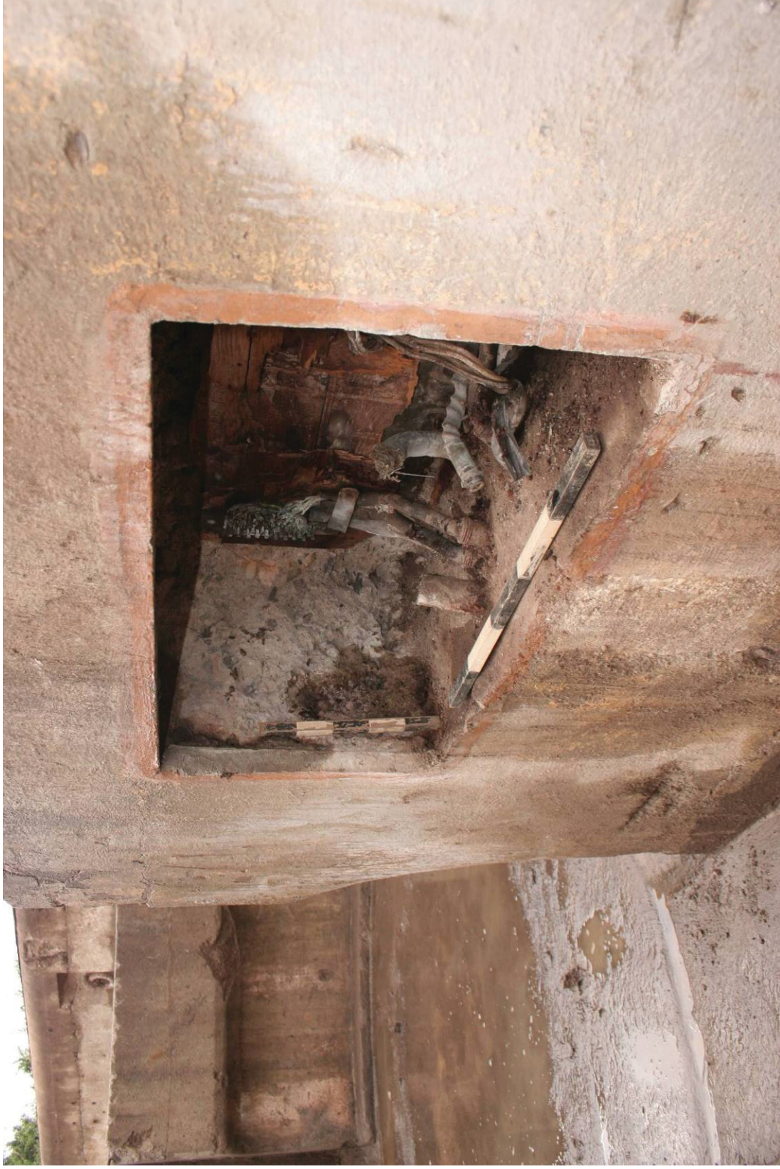
Fig 7 Junction box, facing south east (0.25m and 0.5m scales)
