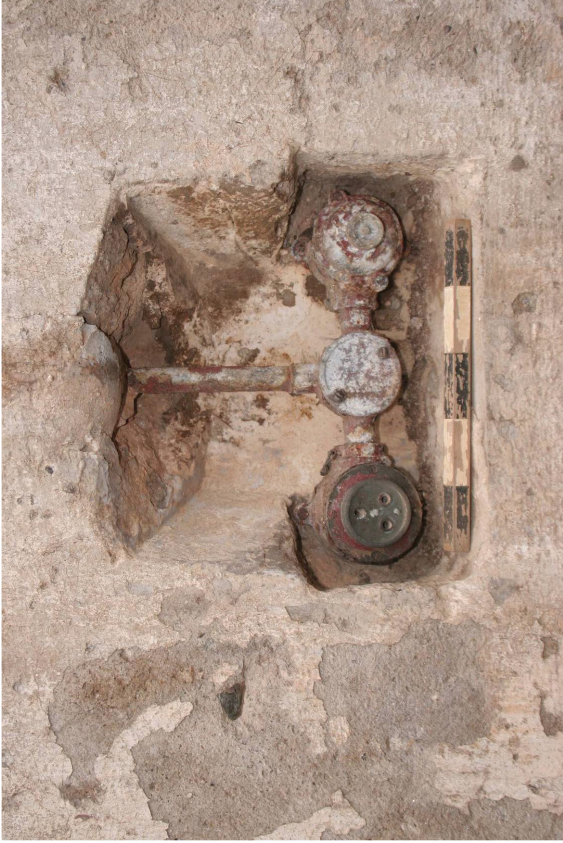
Fig 3 Switches on the southern side of the gun pit, facing south (0.25m scale)
