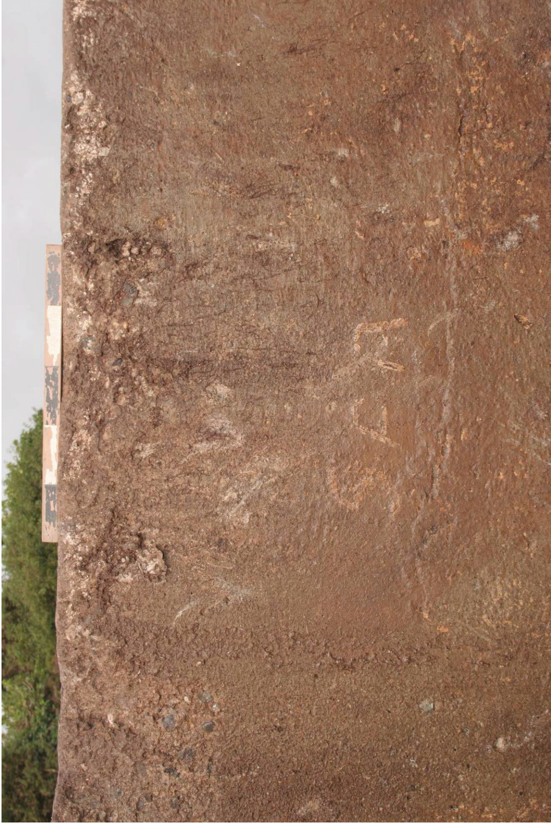
Fig 12 Graffiti "SPA" or "SFA" on wall, facing west (0.25m scale)
