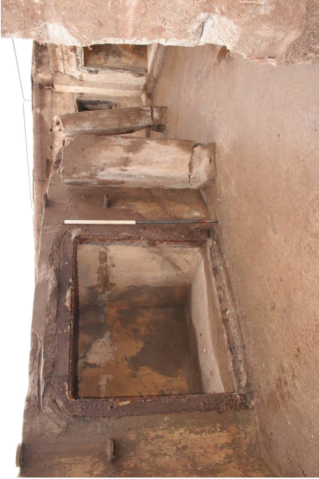
Fig 11 Store 3, facing south. This view also shows the remains of two of the reinforced legs which held up the anti-strafting roof (1m scale)
