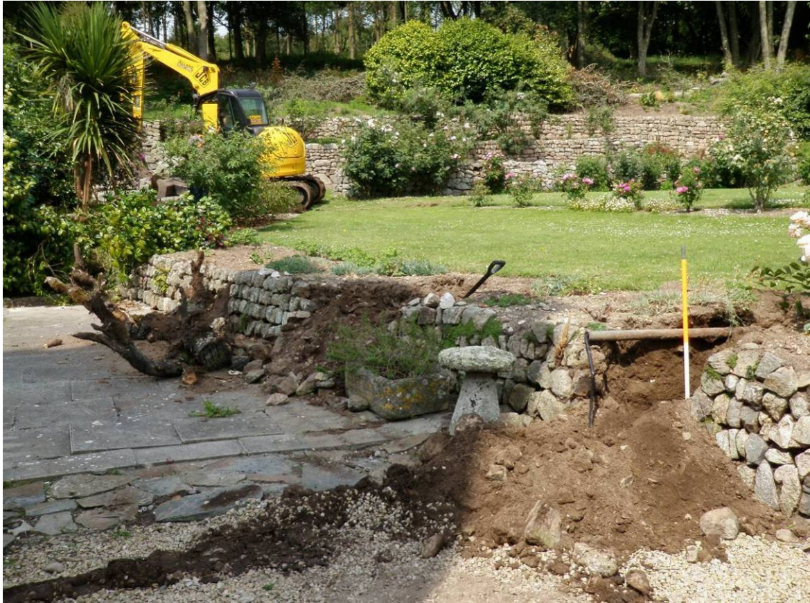
Fig 23 View of lower terrace, after removal of cherry tree stumps
