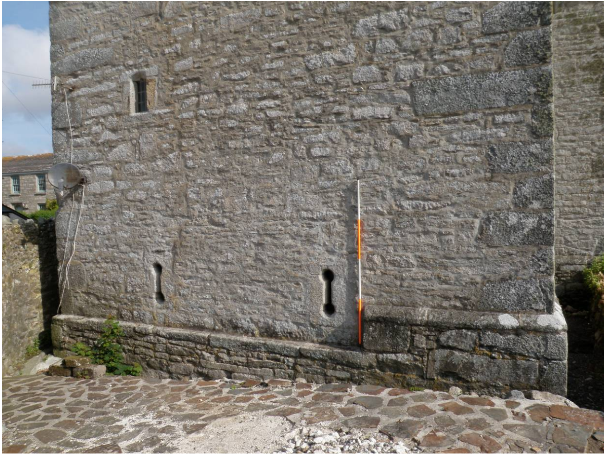
Fig 16 Southern wall of the tower, showing gun loops and related plinths
