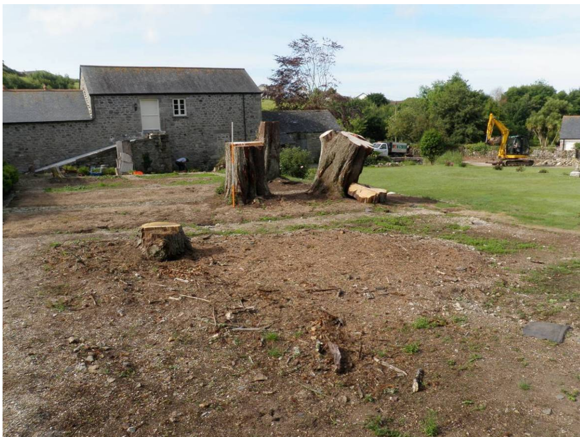
Fig 21 Upper terrace, prior to removal of stumps
