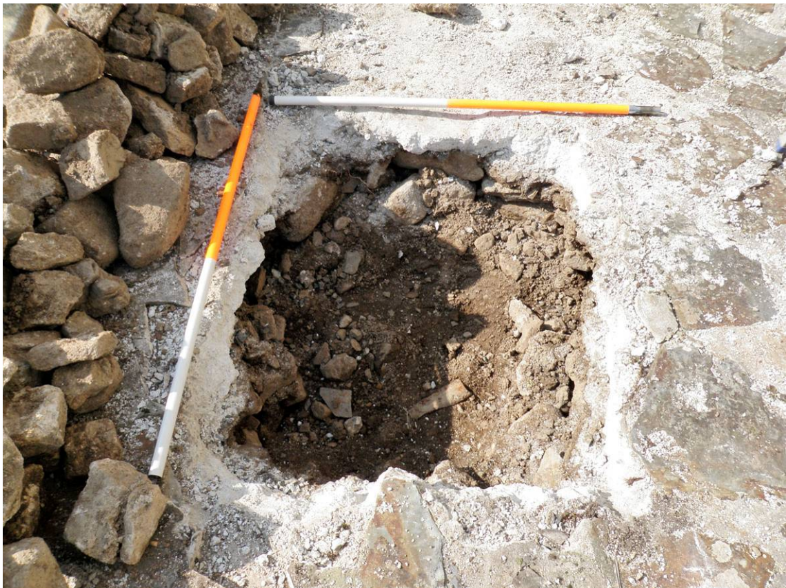
Fig 13 Drain test pit 8
