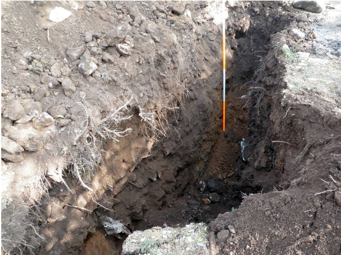
Fig 14 Drain test pit 9
