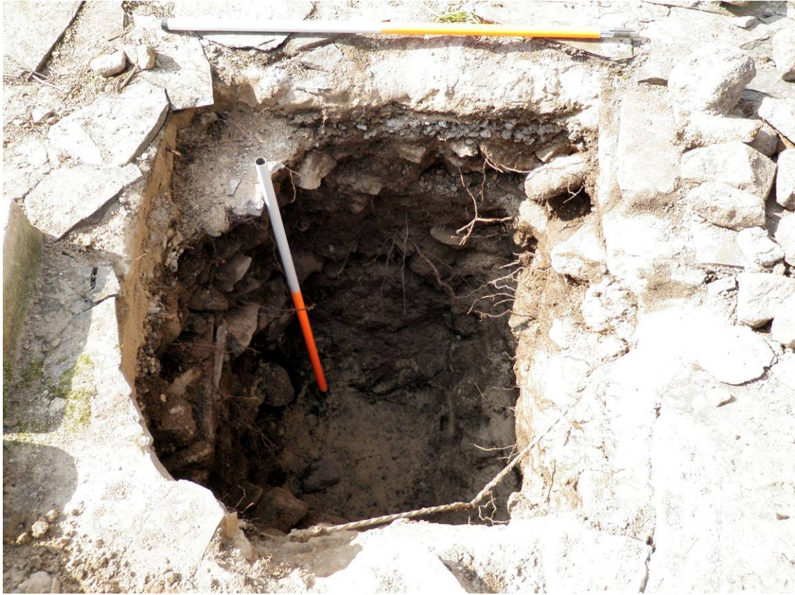
Fig 12 Drain test pit 2
