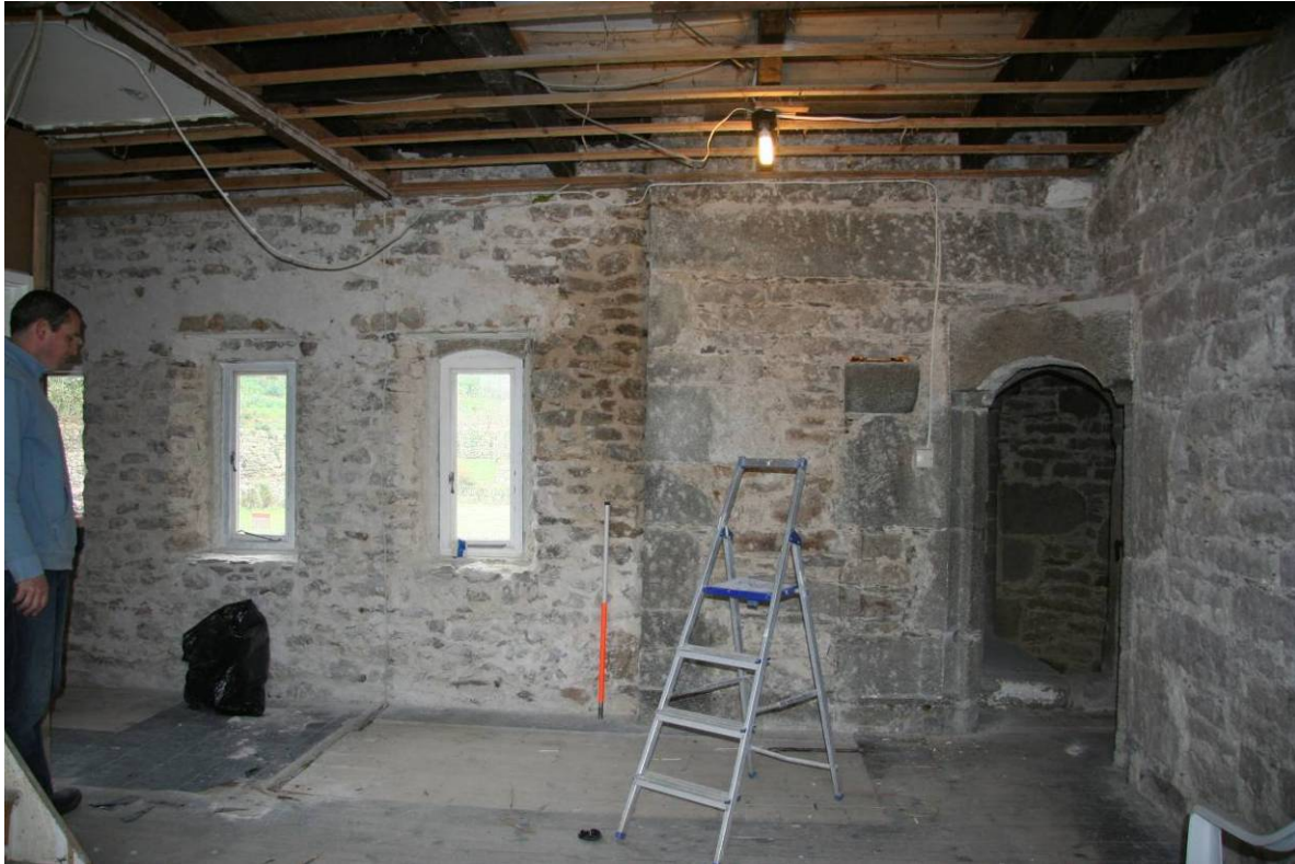
Fig 28 Interior of the first floor room adjoining the tower
