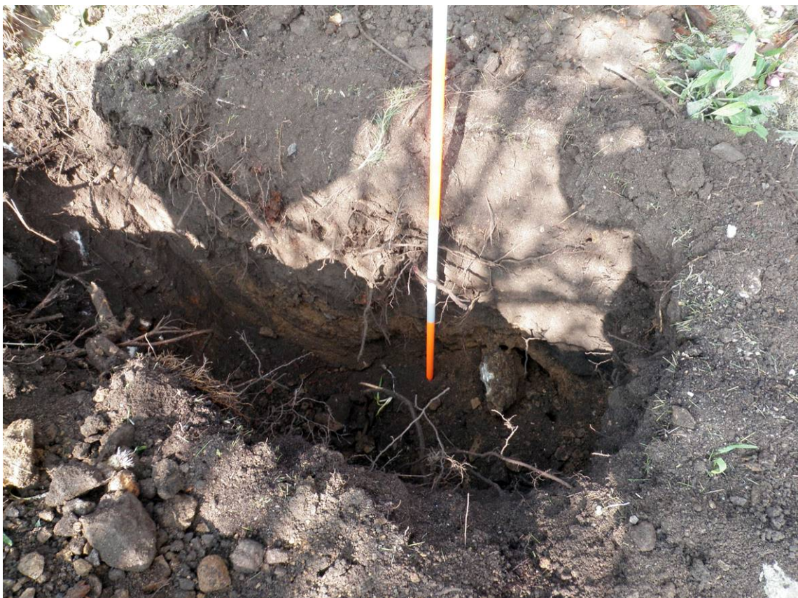
Fig 15 Drain test pit 10
