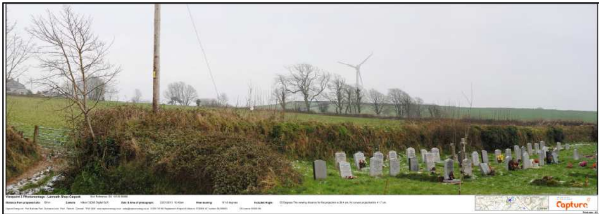
Fig 80 A reduced scale copy of a photomontage provided by Capture-Energy looking from the shop car park at Lanreath across the corner of the churchyard towards the proposed turbine site at Tresawson, about 600m distant, centre shot. This is included for information only, but indicates that the upper parts of the turbine mast and its blades will be substantially visible from some areas within Lanreath, including views of, and across, the Grade I Listed church
