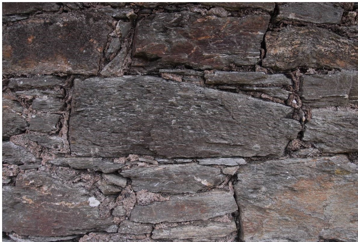
Fig 46. Roughly coursed masonry on the chimney showing indications (centre stone) of final shaping in situ.
