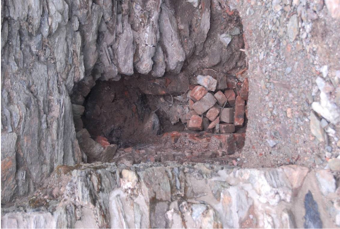
Fig 54. The condition of the flue from the chimney into the former boiler house prior to works.
