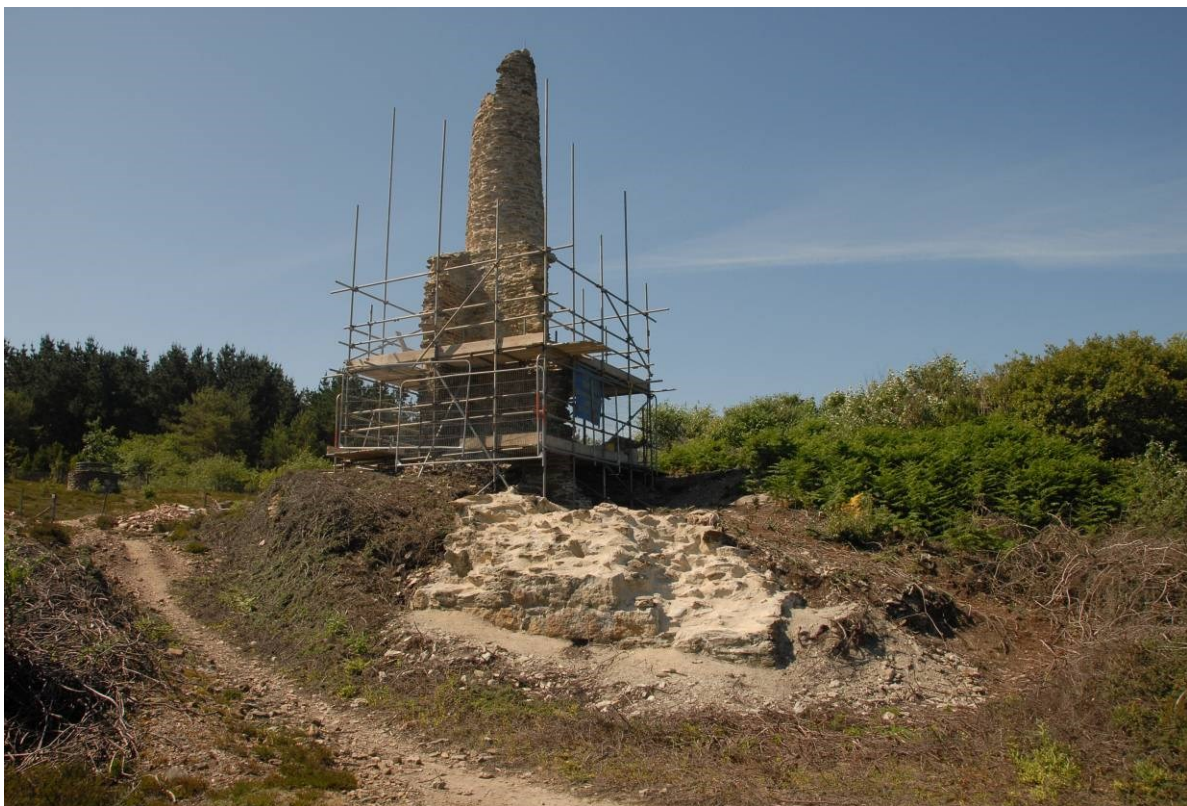
Fig 58. Scaffold erecting on Taylor's whim. The remains of the loadings had been stabilised by pointing. In retrospect, the visual impact of the pointing is unwelcome, but stabilisation would probably not have been possible in any other way.
