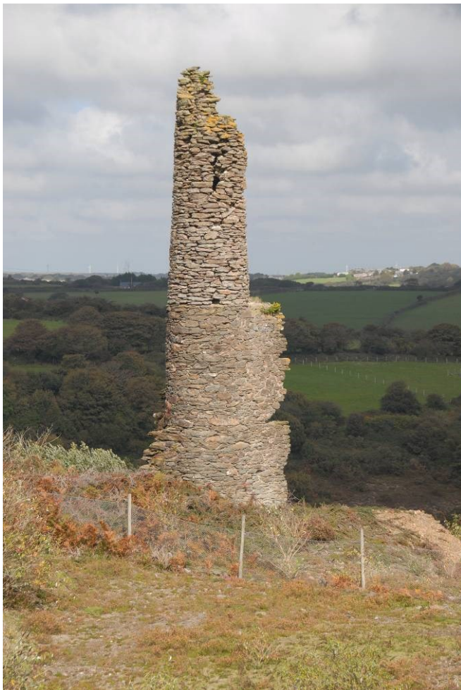
Fig 50. Taylor's whim from the south east prior to works, showing the poor state of the upper part of the chimney and the small amount of the remainder of the building which survived.
