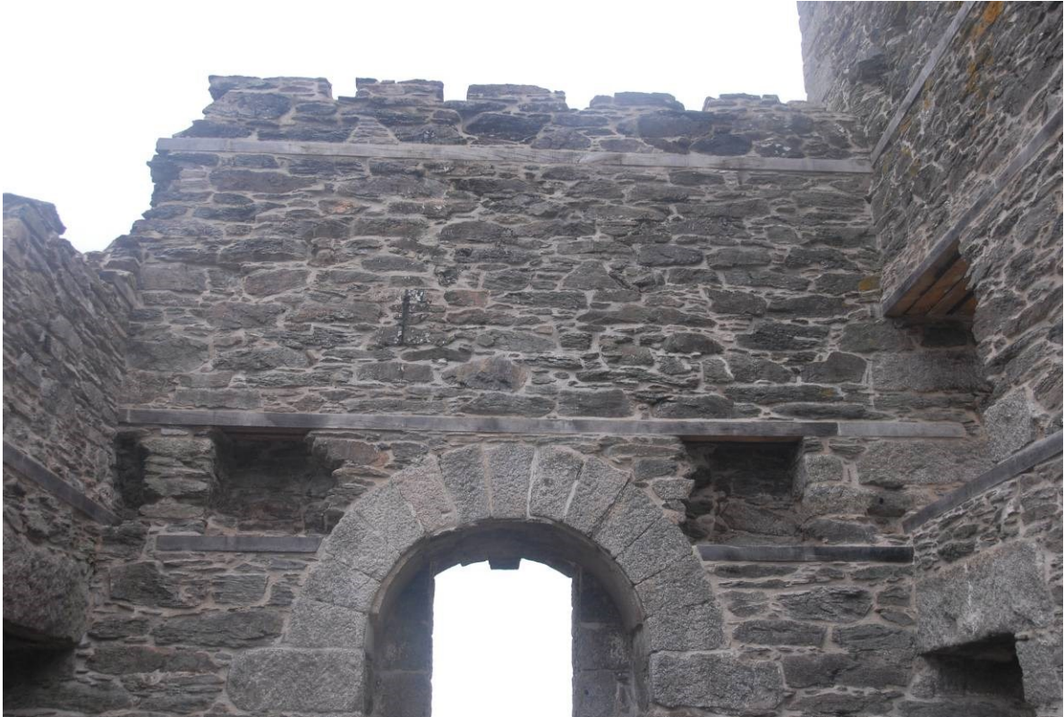
Fig 29. The internal elevation of the bob (northern) wall of Taylor's engine house, showing replacement incorporated oak timbers and the newly-revealed cut outs on the wall head.
