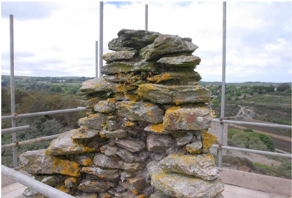
Fig 60. The topmost section of Taylor's whim chimney, showing the almost complete loss of pointing, and the extremely ragged profile.
