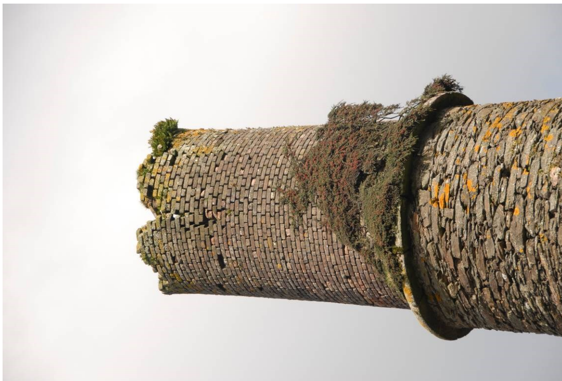
Fig 37. Taylor's chimney brickwork from the west, showing its poor condition.
