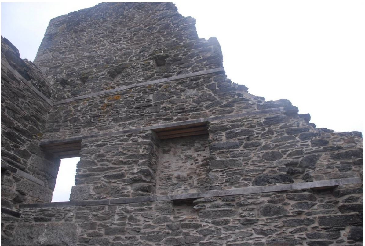
Fig 28. The internal eastern elevation of Taylor's engine house, showing the new timbers installed within the face of the wall, and the appearance of the new pointing.
