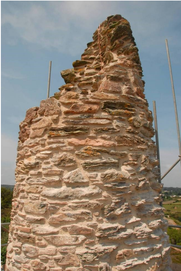
Fig 67. The reconstructed upper section of Taylor's whim chimney with its unobtrusive lightning conductor.
