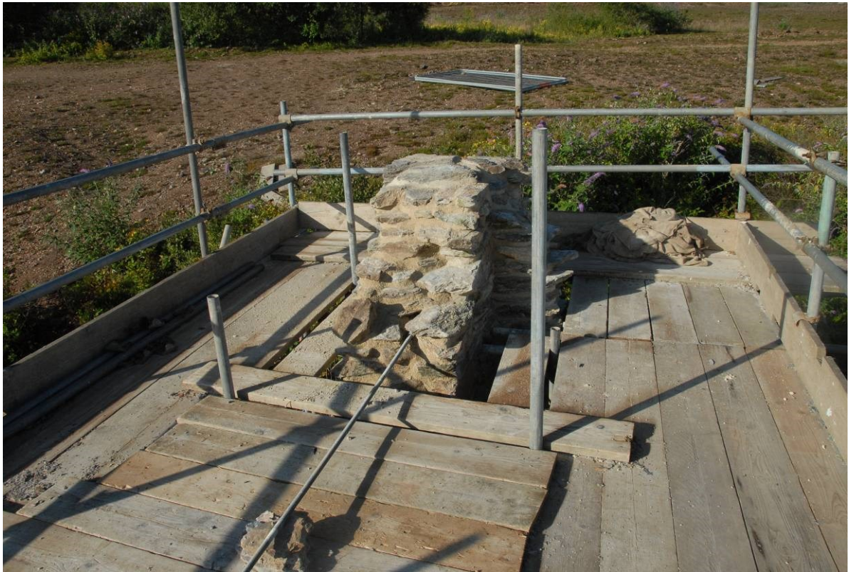
Fig 77. The rebuilding of the formerly unstable south eastern wall incorporated a tie bar through the wall cores.
