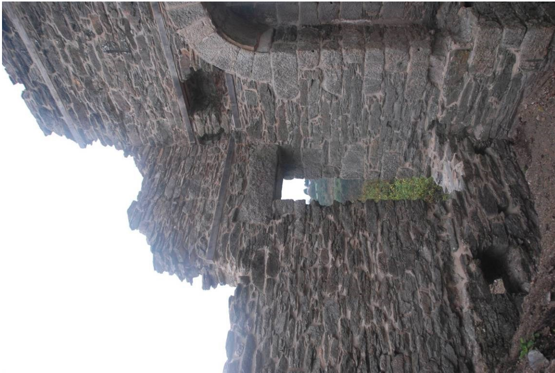
Fig 31. The western internal elevation of Taylor's engine house, showing the reconstructed masonry above the replaced lintel.
