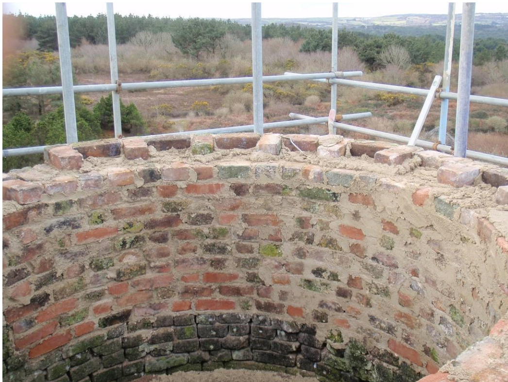
Fig 40. Reconstruction of the upper chimney brickwork courses under way, a mixture of old and new bricks being used for its interior.
