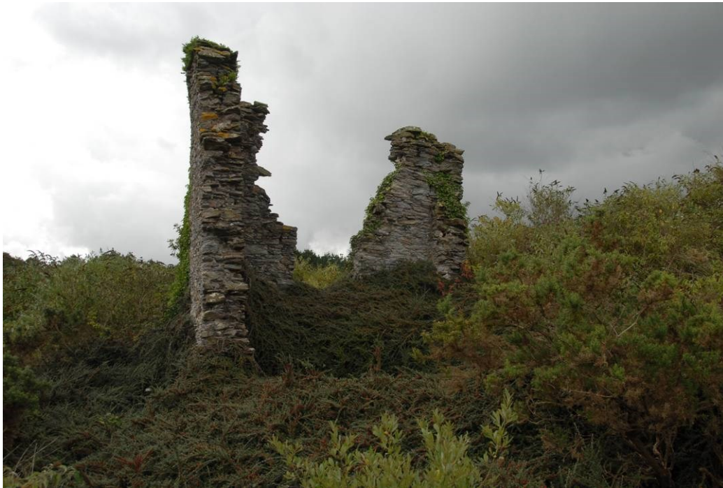
Fig 73. Davey's whim from the north prior to works. Cotoneaster completely covered the cylinder plat. The splayed nature of the upper sections of the walls is clearly visible.
