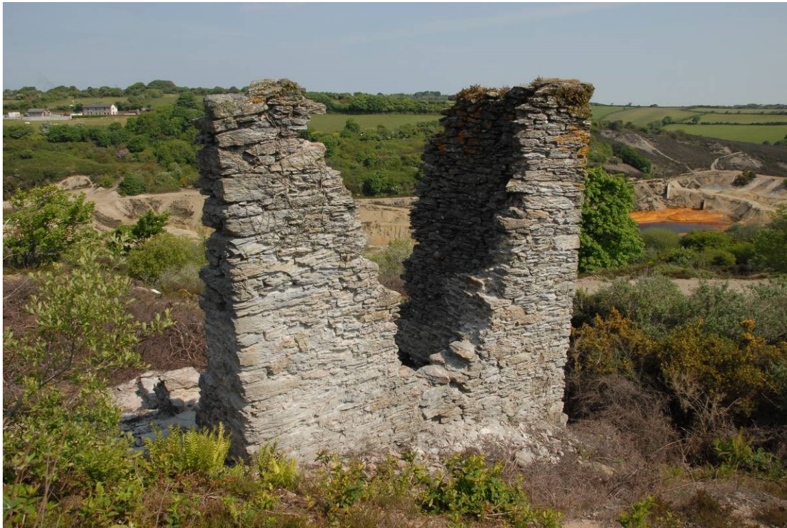
Fig 71. The south eastern elevation of Davey's whim following the removal of ivy and other vegetation.
