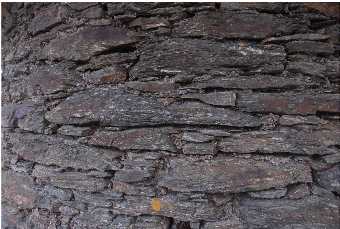
Fig 44. Much of the pointing on the lee (northern and eastern) sides of the chimney had been eroded away. Note also the elongated shaped stones used in the structure.
