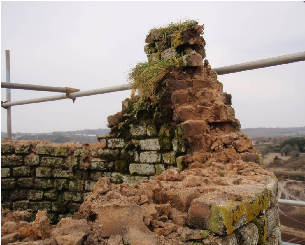
Fig 39. The condition of the upper courses of the chimney brickwork, much of which could be picked off by hand.
