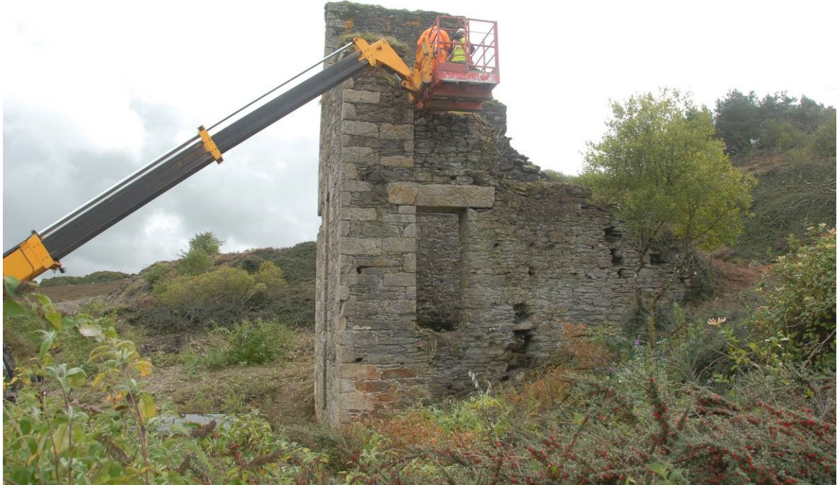
Fig 17. Utilising a cherry picker allowed the tree ivy to be removed from Taylor's engine house, a bat survey to be undertaken and a detailed structural assessment made of the building.
