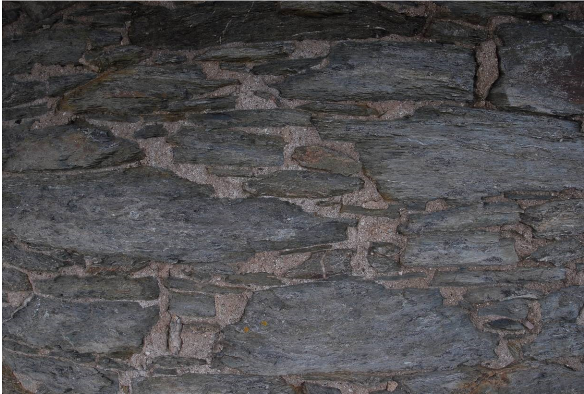
Fig 45. Remnant pointing on the lower part of the chimney. Detached sections of this were removed and patch pointed, but tight joints were left as found.
