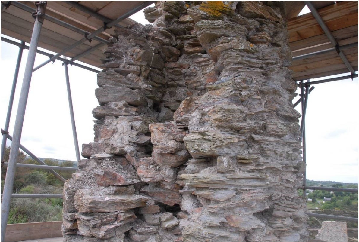
Fig 59. The extremely poor state of the upper part of Taylor's whim chimney prior to works.
