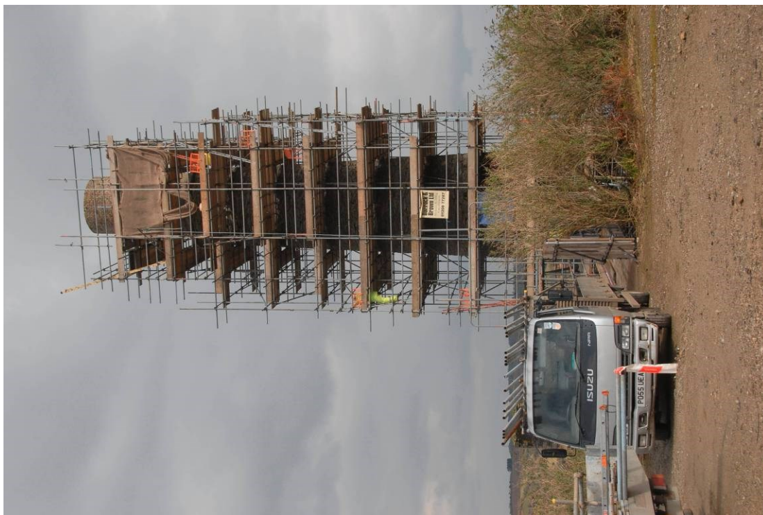
Fig 38. Scaffolding fully erected on Taylor's chimney and work on its brickwork under way.
