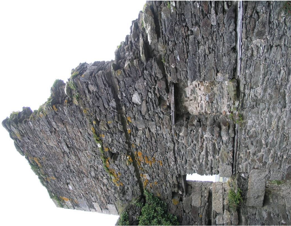
Fig 13. The internal elevation of the eastern wall, showing the two window openings (the rearmost blocked on the outside face) and the two longitudinal timbers whose decay had significantly contributed to the deterioration of the structure.
