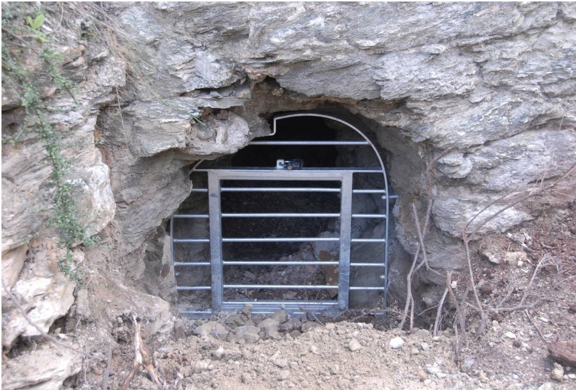
Fig 49. The bat grille fitted to the flue opening at the base of the chimney.
