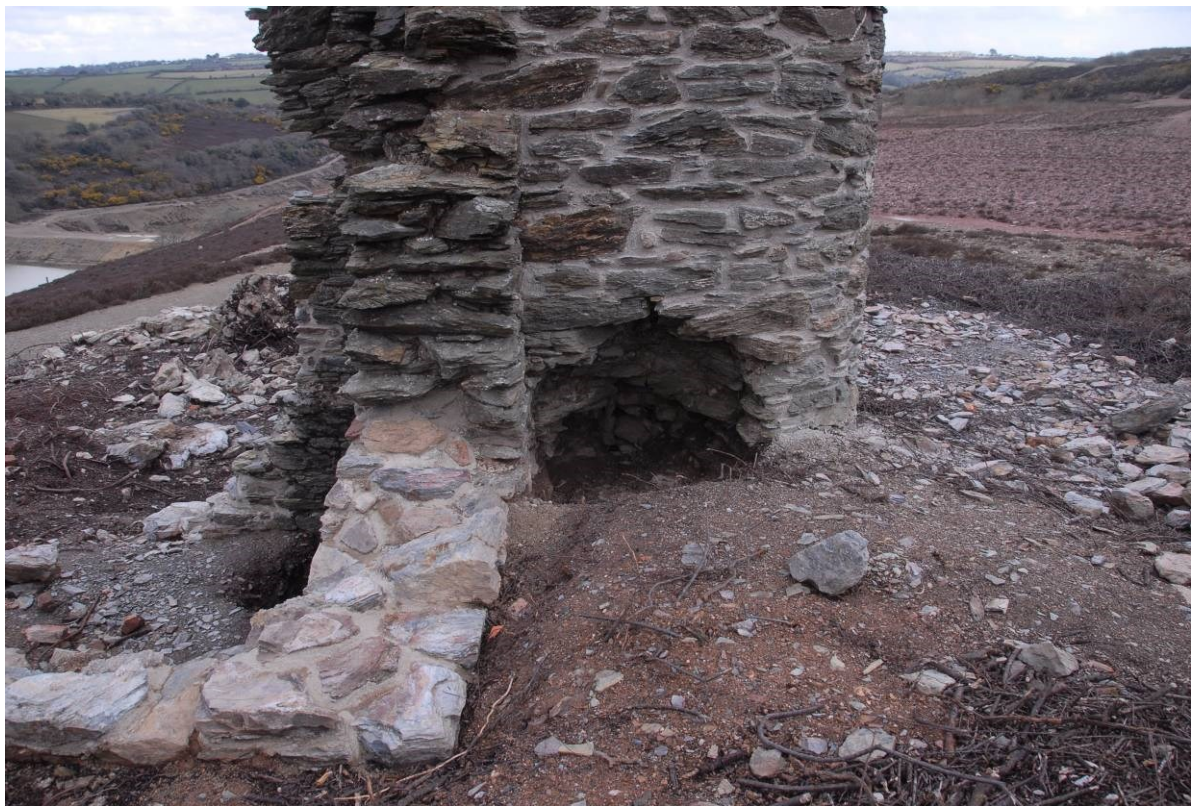
Fig 56. Repointing under way on the lower part of the chimney and the remains of the boiler house walls (left). Note also the collapsed ash clearance hole at the base of the chimney.
