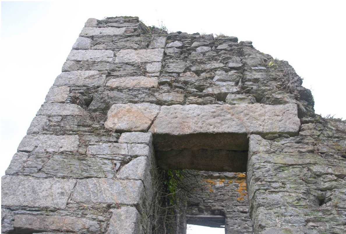
Fig 20. The cracked lintel over the boiler house door on the western elevation of Taylor's engine house.
