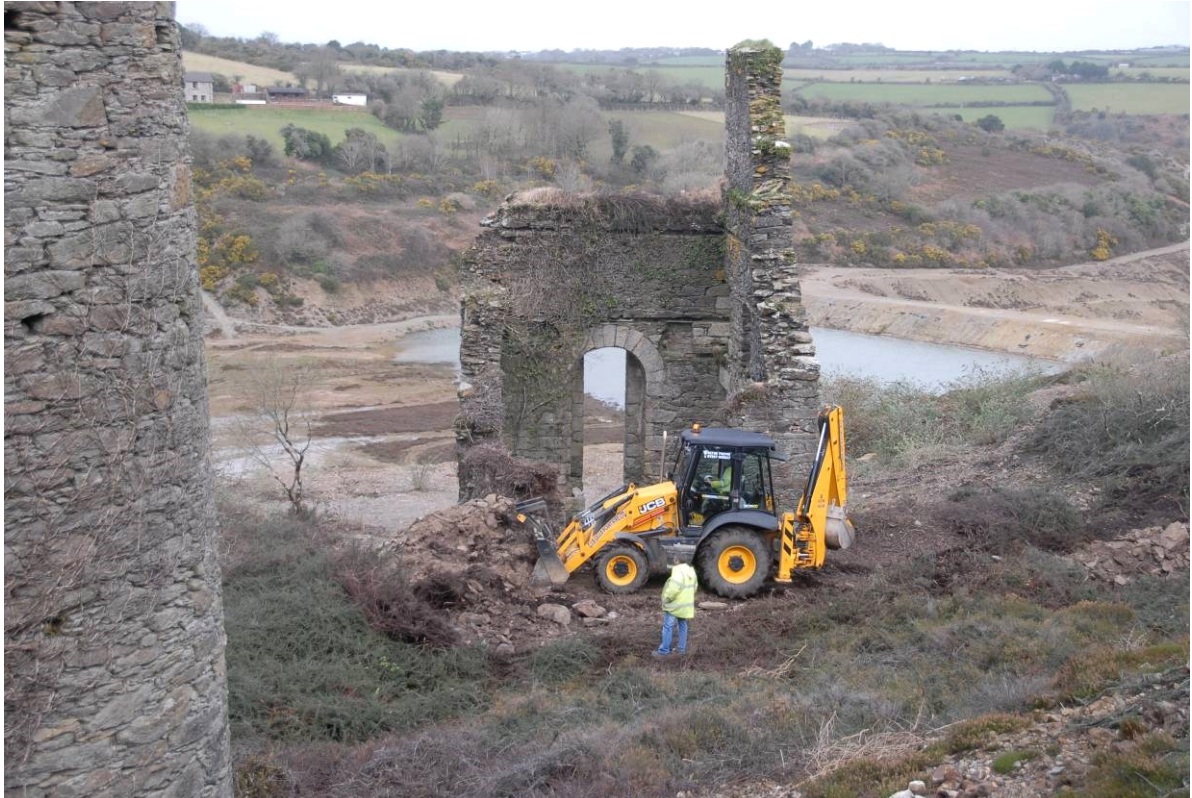
Fig 18. A wheeled excavator was used to remove Cotoneaster and rubble from around Taylor's engine house.
