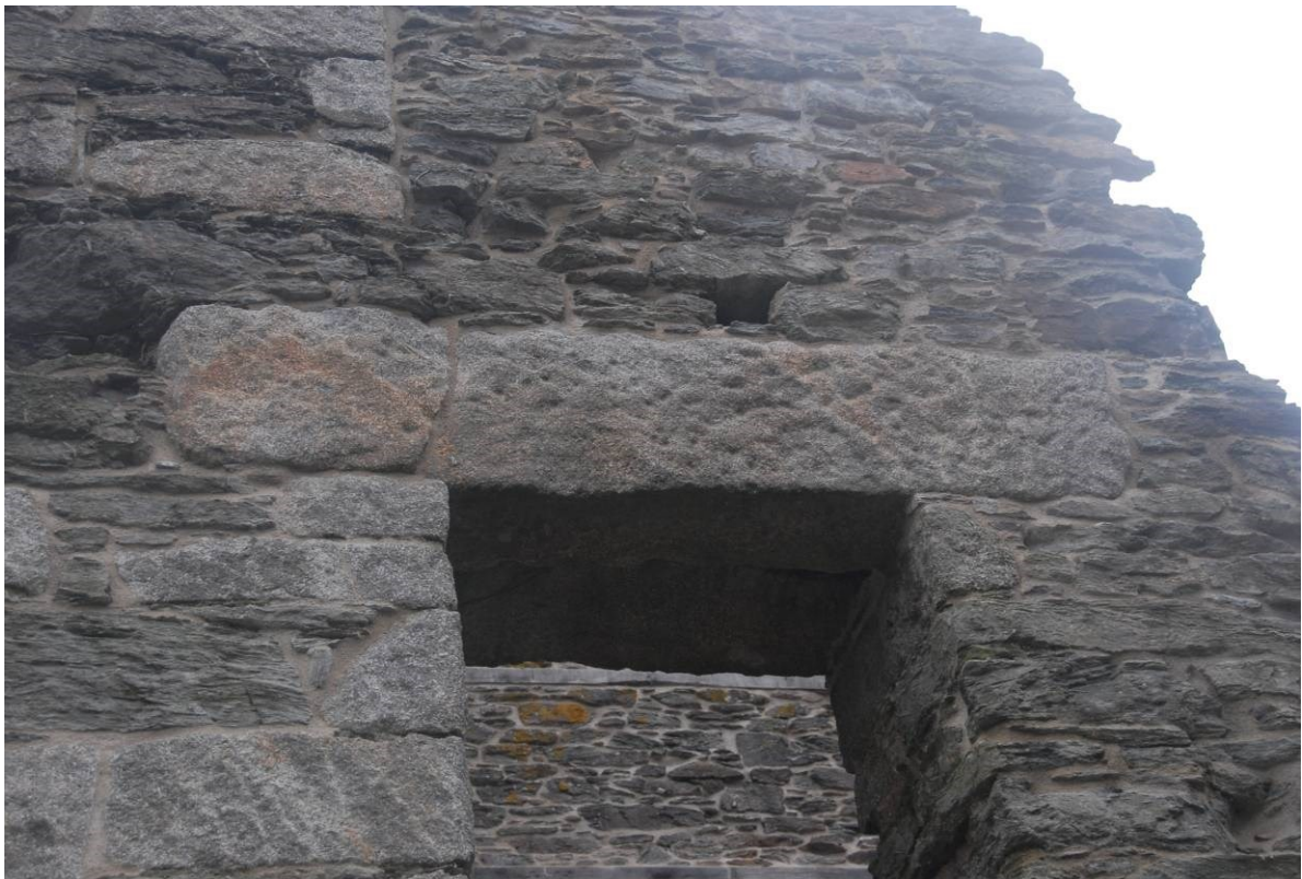
Fig 24. The lintel over the boiler house door following drilling and pinning to restore its structural integrity.
