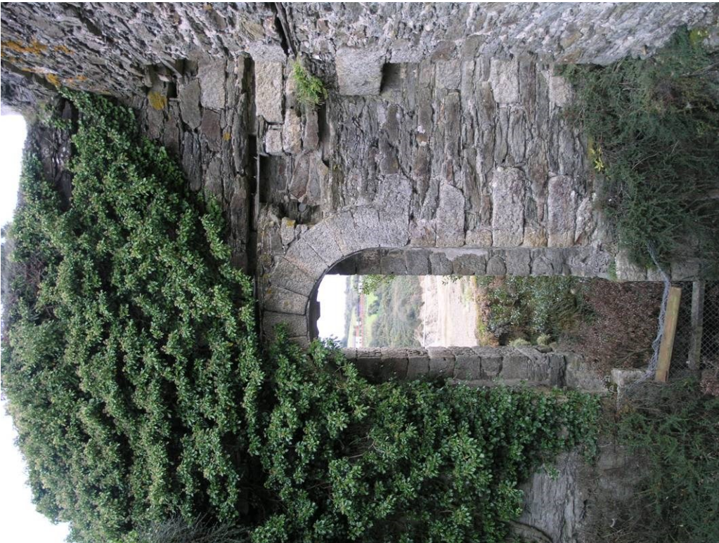
Fig 11. The interior of the bob wall, showing the characteristic part-closed plug door opening; above is the lateral slot which would have held a timber, and, below this to the right of the doorway, one of the pockets for the first floor support timbers.
