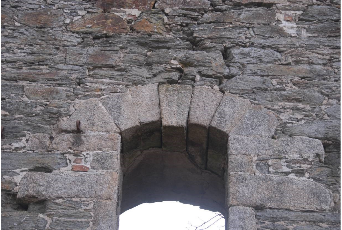
Fig 21. The dropped voussoirs over the plug door opening in the northern elevation of Taylor's engine house. Note also the remnant plasterwork in the crown of this opening.
