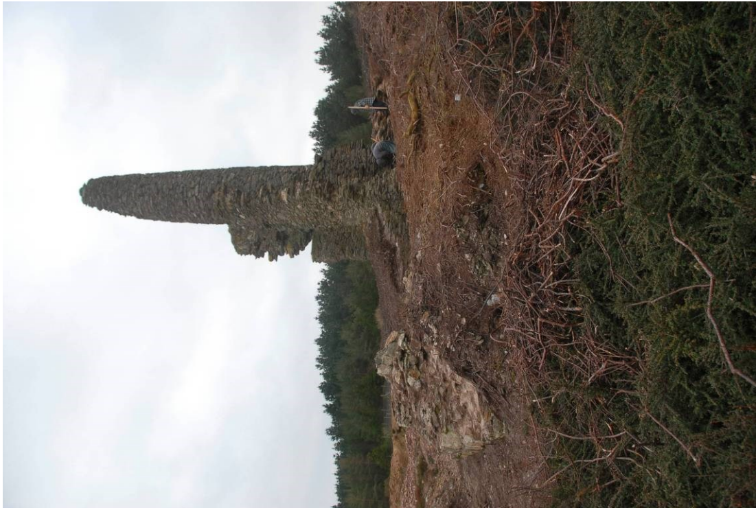
Fig 53. Taylor's whim during preliminary vegetation clearance, showing the remains of the loadings (foreground left).
