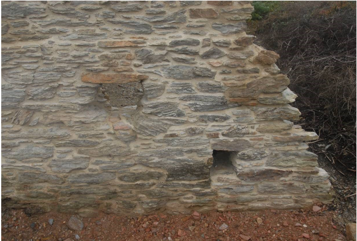
Fig 79. The north eastern wall of Davey's whim, showing the steam pipe entry and cylinder drain openings.
