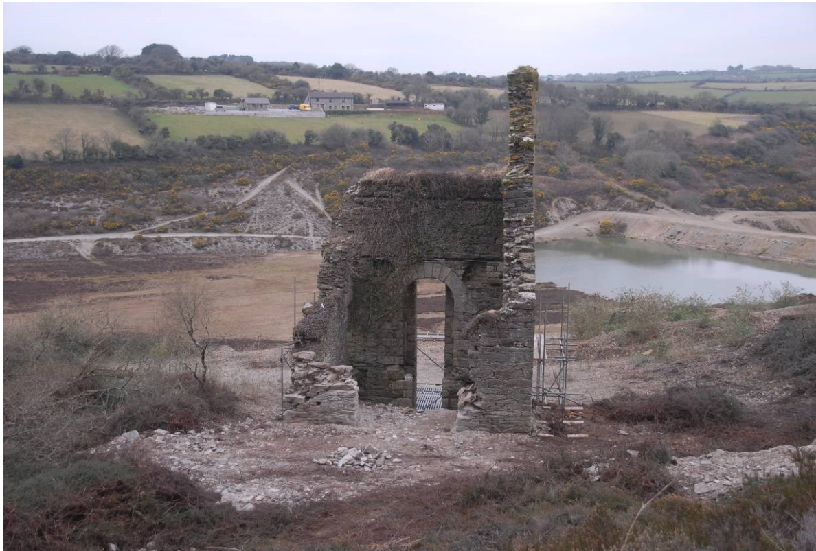
Fig 19. Taylor's engine house from the south following the clearance of rubble and scrub, showing the newly-revealed cylinder doorway.
