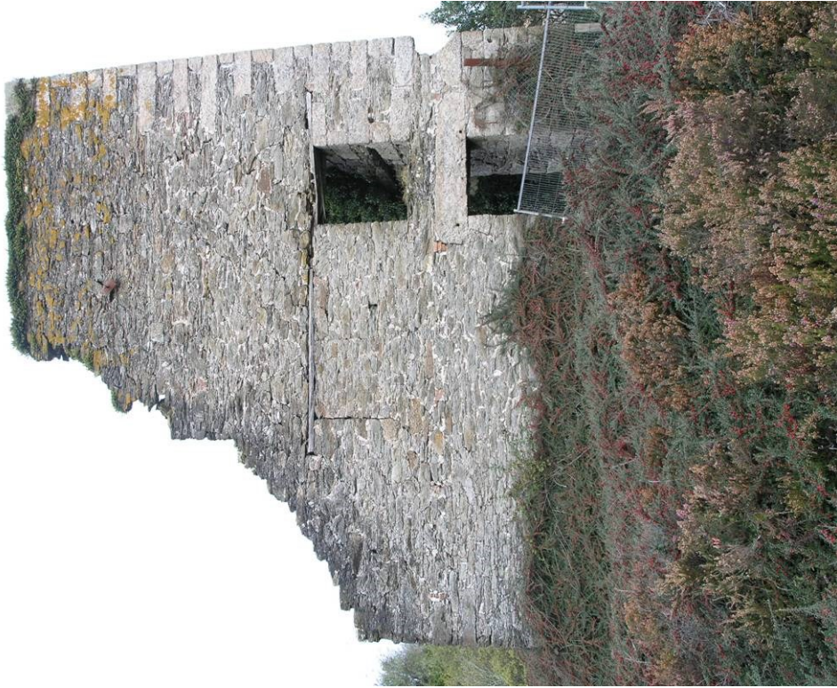
Fig 12. The eastern wall of Taylor's pumping engine house, showing the doorway and window above and blocked window to its rear, the longitudinal timber and (half-way up the rear edge of the surviving masonry) the remains of the girder opening.
