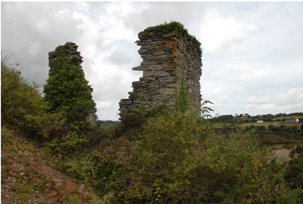
Fig 70. The south eastern elevation of Davey's whim prior to works, showing the precarious and overgrown state of the building.
