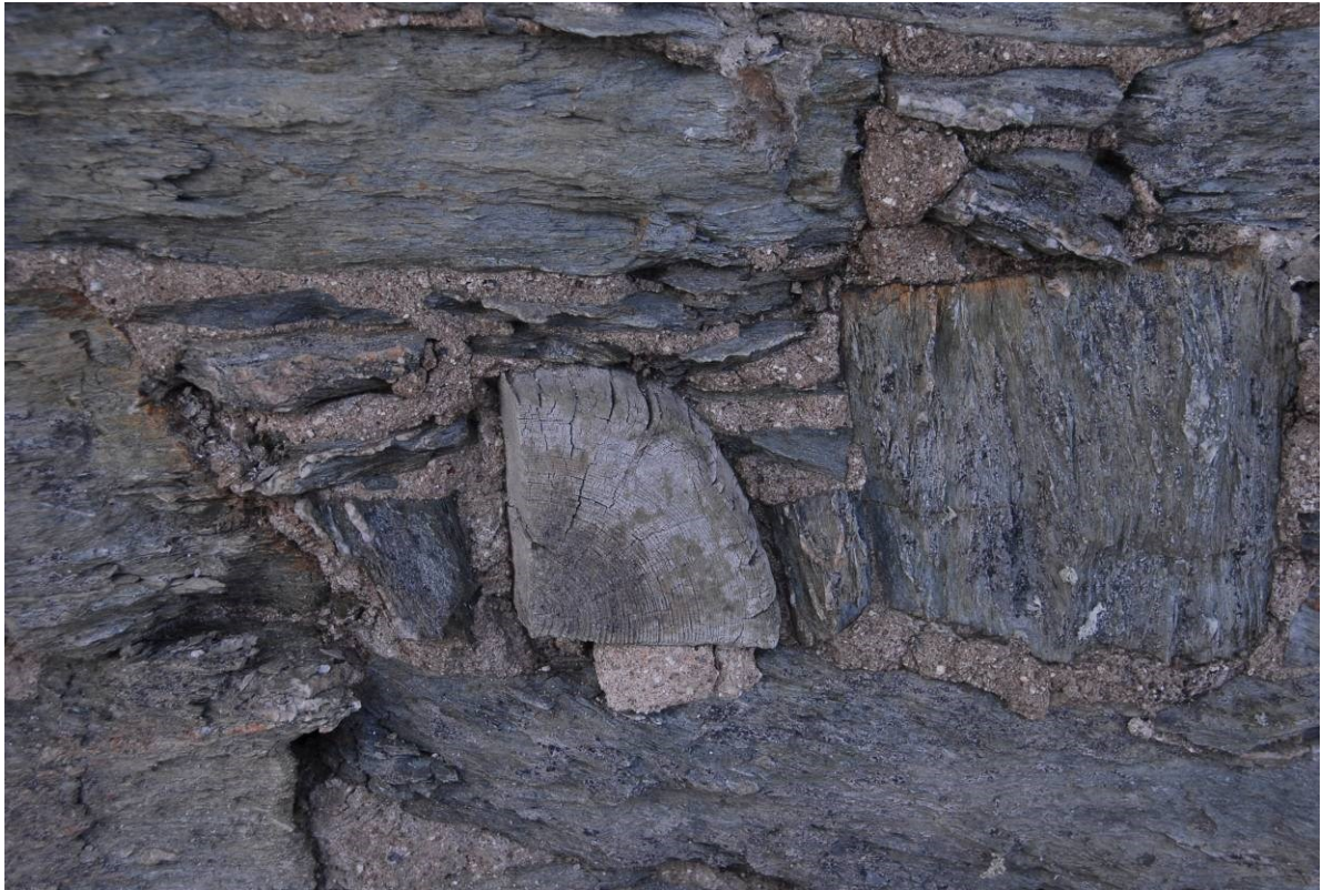
Fig 43. A remnant cut off putlog in the face of the chimney. Note also the differential erosion which has occurred in the stonework of this structure.
