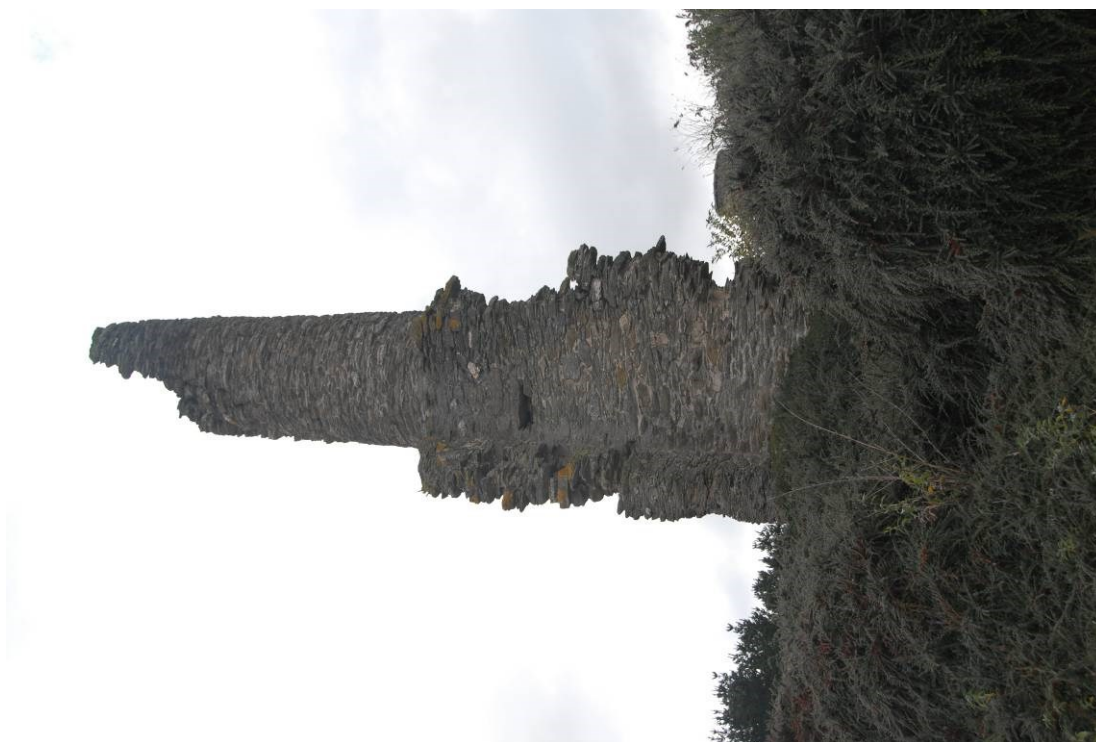
Fig 52. Another view of Taylor's whim, showing the poor state of the broken masonry at the edges of the walls.
