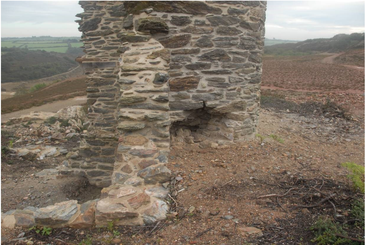
Fig 65. The completed work to the lower section of the chimney and boiler house walls at Taylor's whim following the installation of the lightning conductor.
