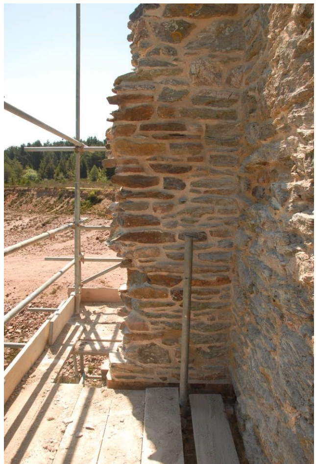
Fig 63. The rebuilt eastern edge of the lower part of the southern wall of Taylor's whim, showing the oak lintel stubs incorporated to indicate the location of the former doorway.
