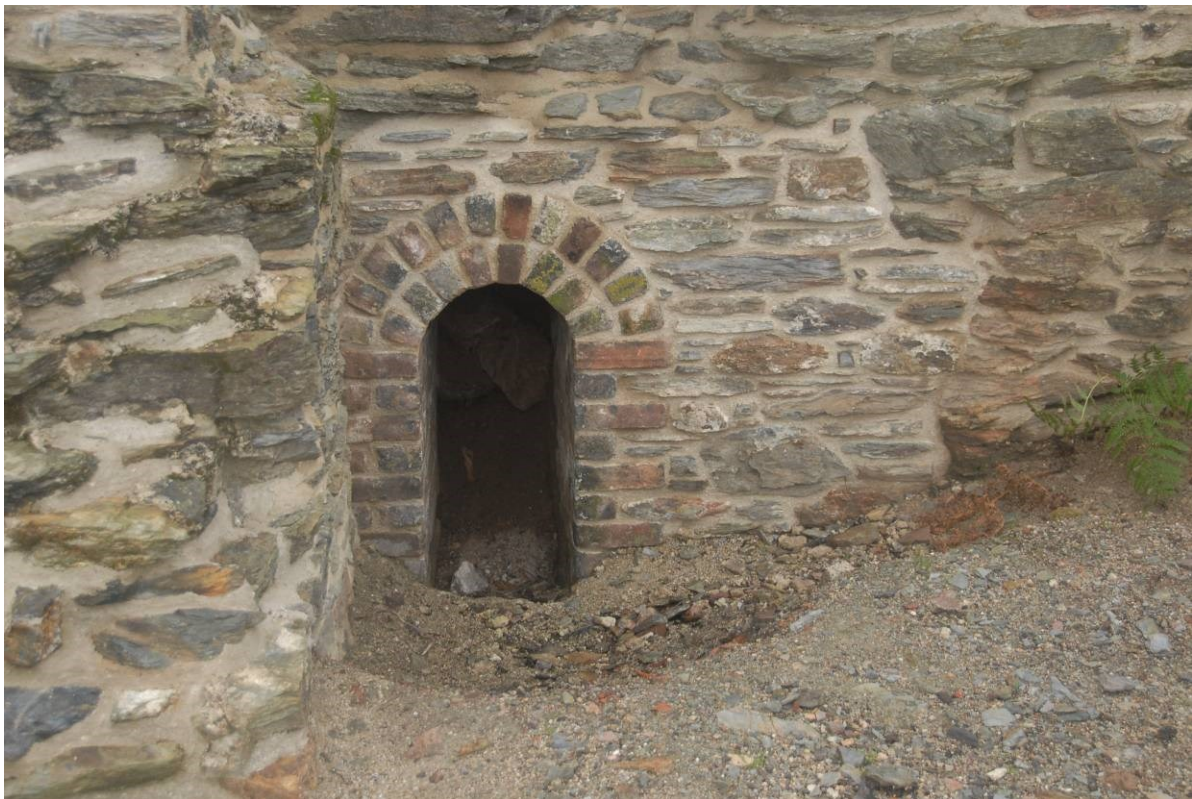
Fig 66. The repaired flue connection between the chimney and boiler house at Taylor's whim (compare with Fig 54).
