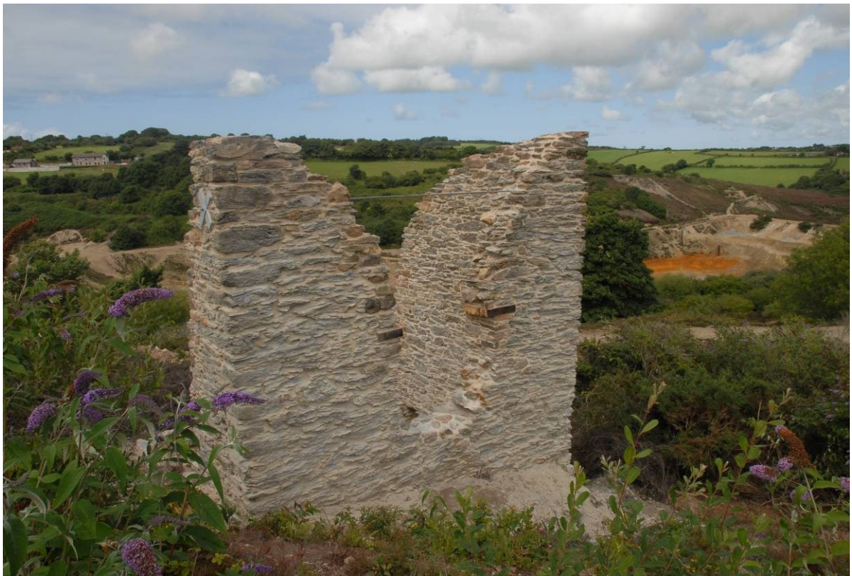
Fig 78. The completed works to Davey's whim as seen from the south. Note the tie rod and pattress and the lintel stubs inserted into their original locations. Compare with Fig 71.
