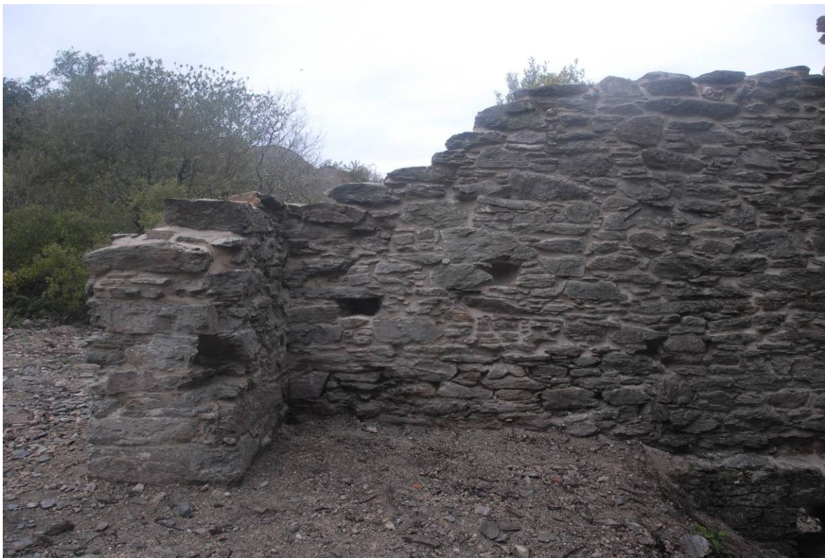
Fig 30. The consolidated southern section of the western wall elevation, together with the stabilised western section of the southern wall.
