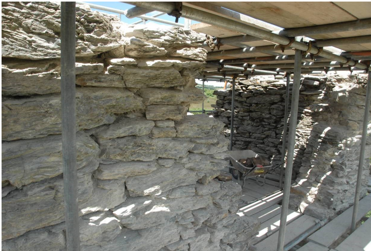
Fig 76. A closer view of the condition of Davey's whim masonry, showing the very substantial loss of pointing which had occurred.
