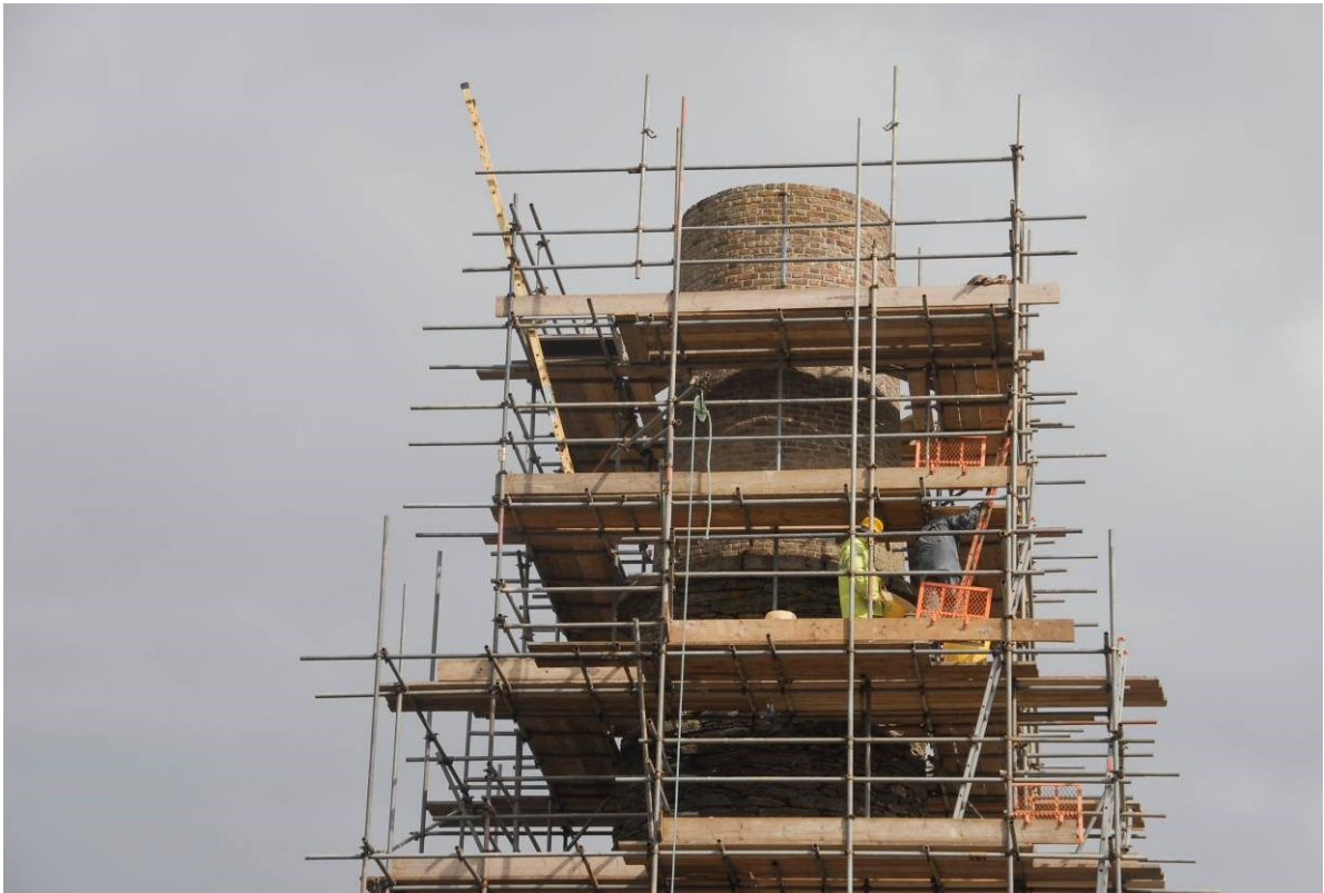
Fig 41. A general view of the conservation work to the chimney under way. The brick cap had been fully repaired by this point in the work programme.
