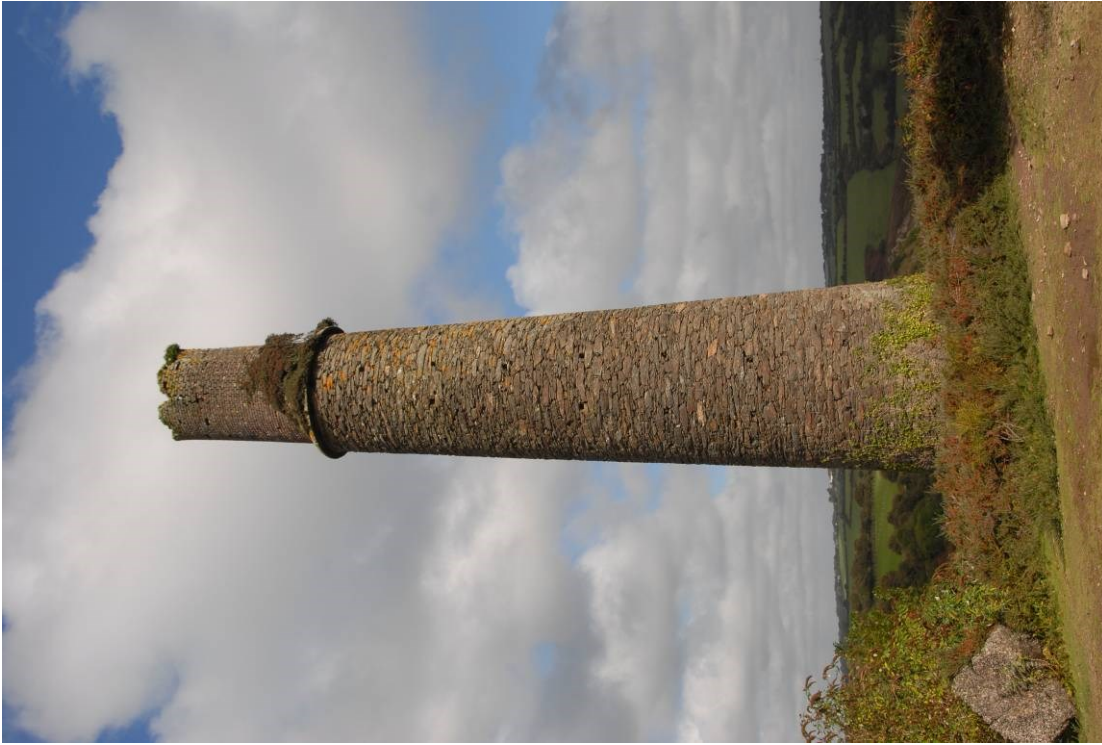
Fig 36. Taylor's chimney from the west prior to works, showing the poor state of the brickwork and the cotoneaster which had begun to grow above the drip ring.
