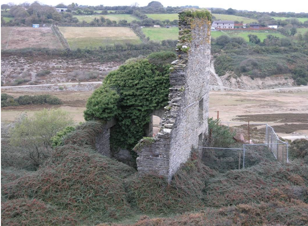
Fig 9. Taylor's engine house from the south during 2009. The amount of masonry lost from the rear half of the engine house is apparent, as is the quantity of ivy cloaking the north western corner of the building and the cotoneaster around it.
