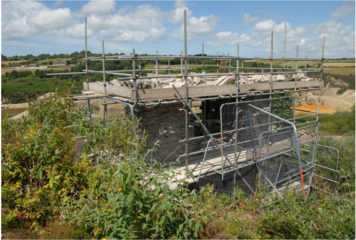
Fig 75. Conservation works under way. The unstable stonework forming the wall peaks had been recorded and dismantled by this stage.
