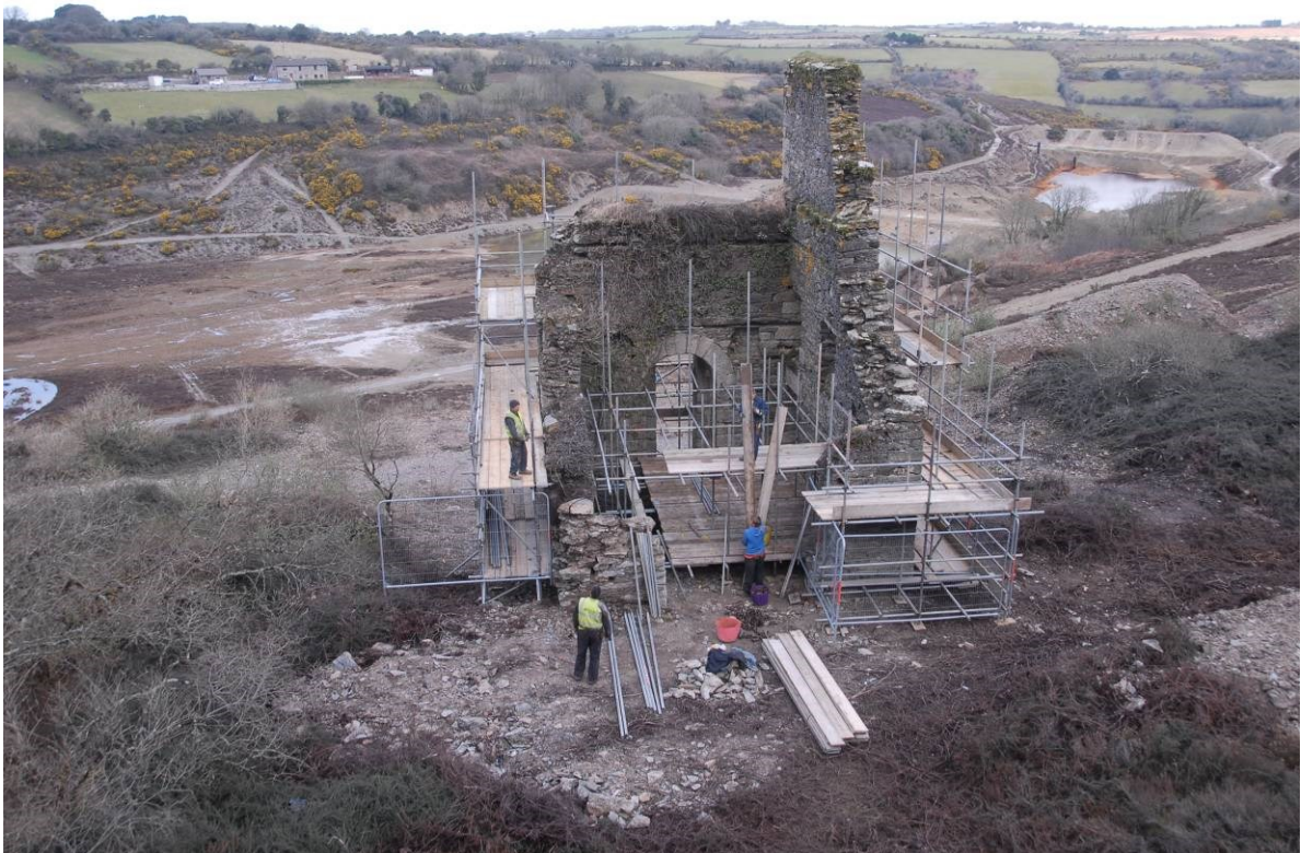
Fig 22. Erecting scaffolding on Taylor's engine house prior to works.
