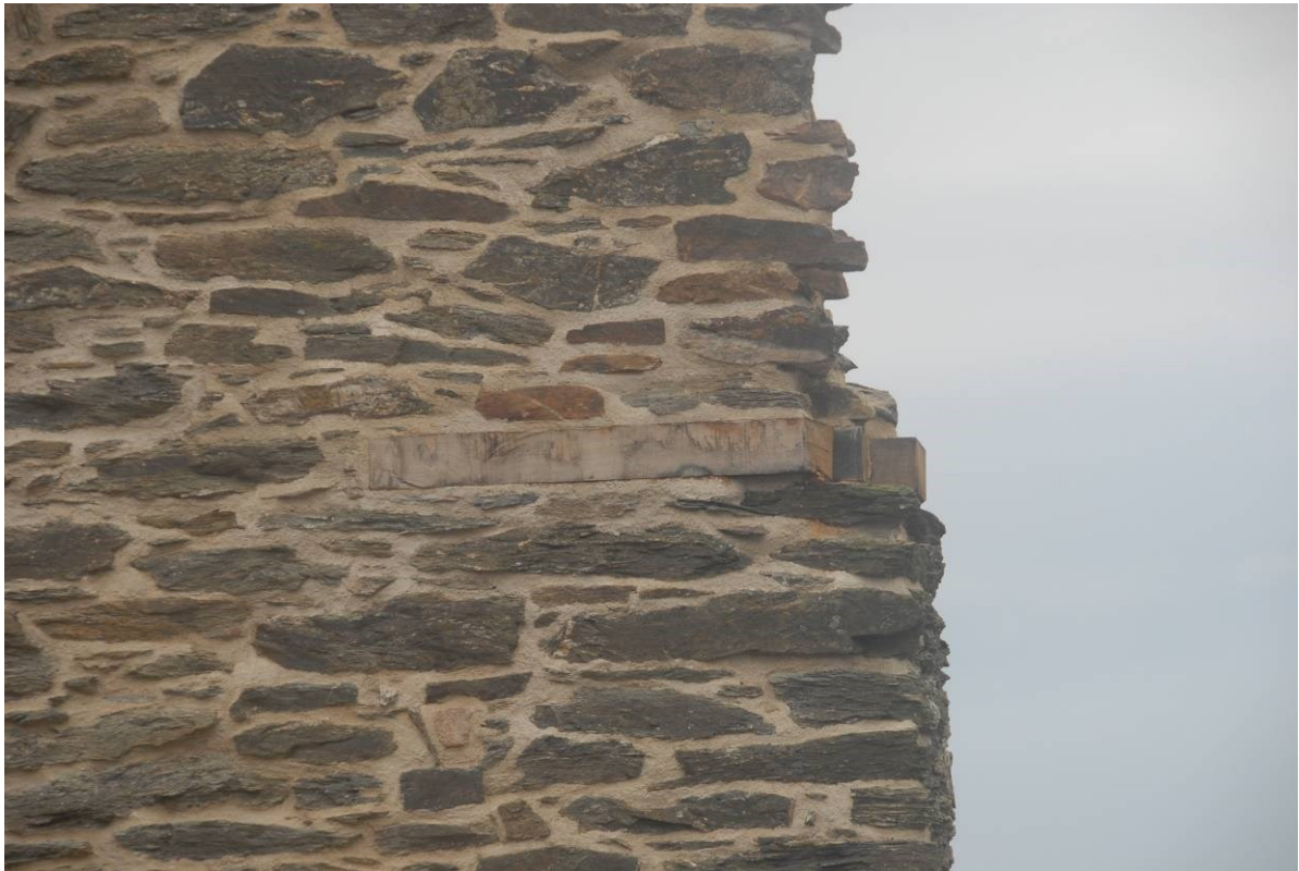
Fig 63. The rebuilt eastern edge of the lower part of the southern wall of Taylor's whim, showing the oak lintel stubs incorporated to indicate the location of the former doorway.
