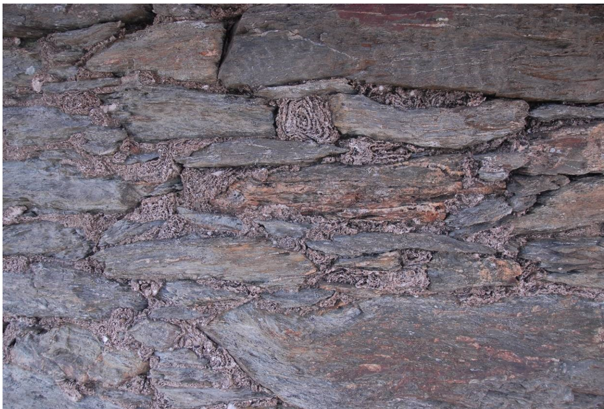
Fig 42. Original pointing on the western elevation of the chimney had a characteristic weathering appearance. Much of this pointing was sound and could be left in place.
