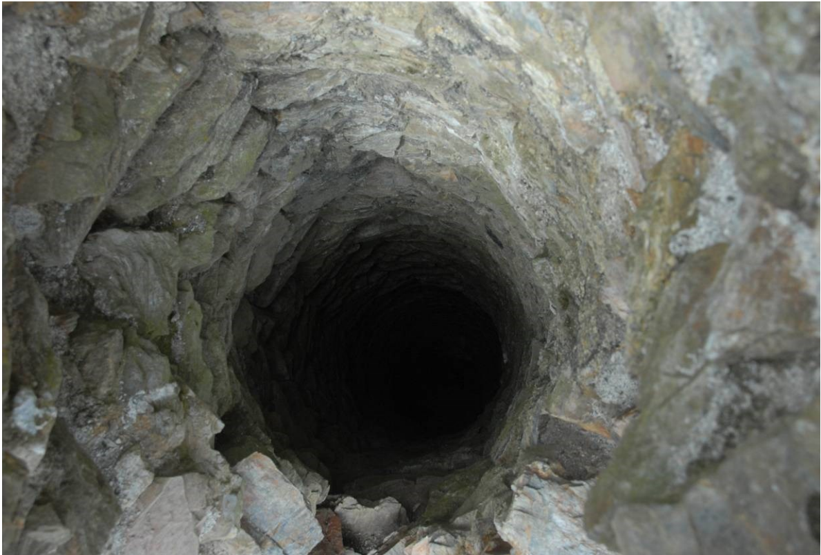
Fig 61. The interior of Taylor's whim chimney, showing the almost complete loss of its pointing.
