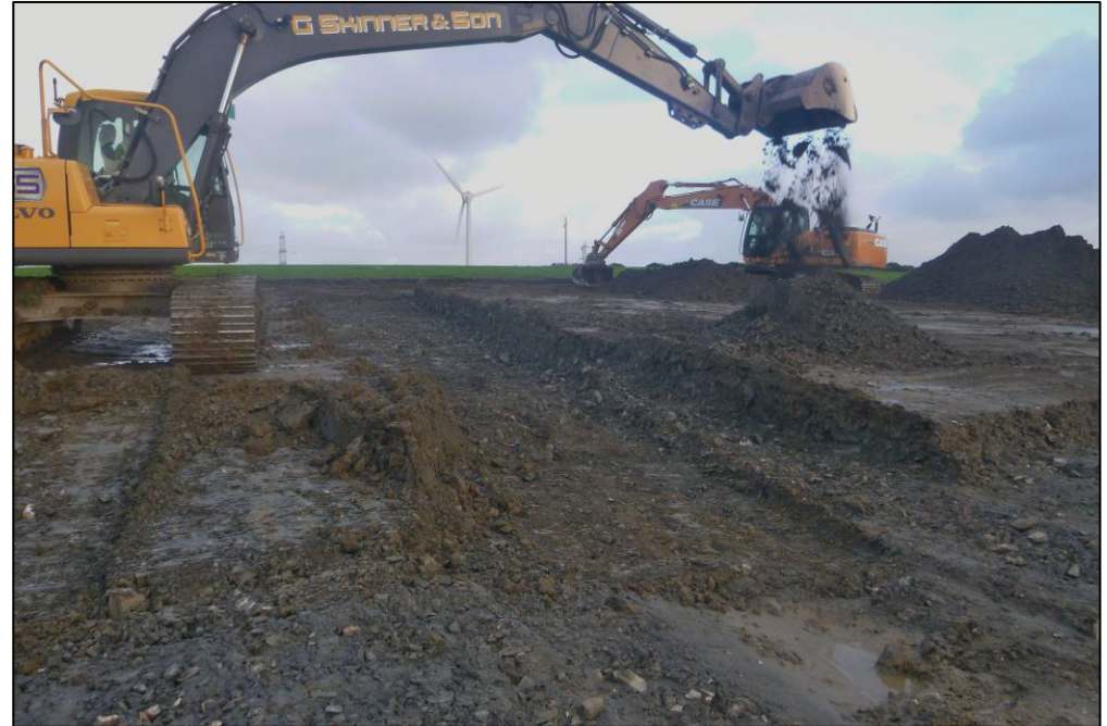
Figure 7: Removal of secondary material (102) (looking north).
