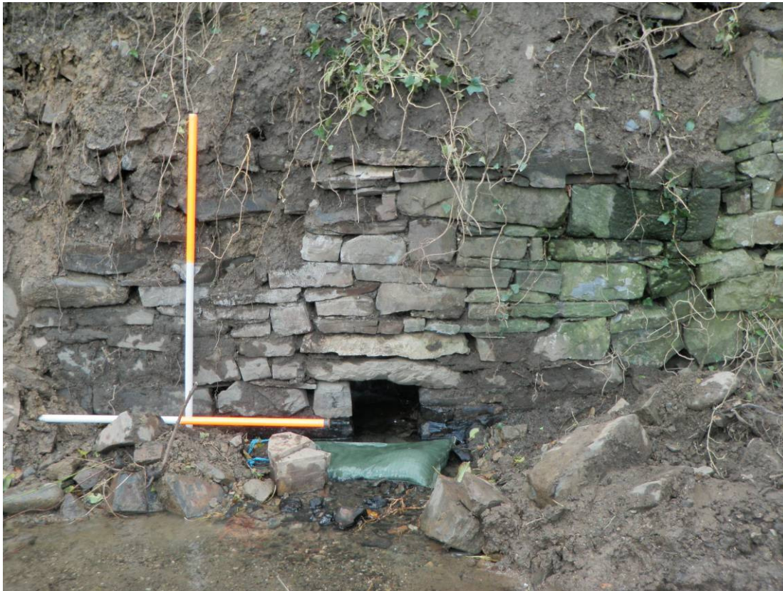
Fig 13 Stone facing around the exit of the culvert
