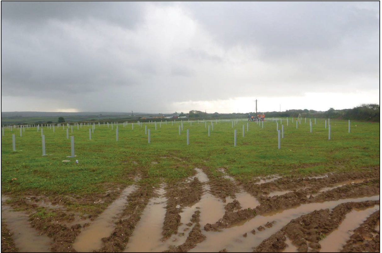
Figure 6: Field G looking east with array support piling in progress.
