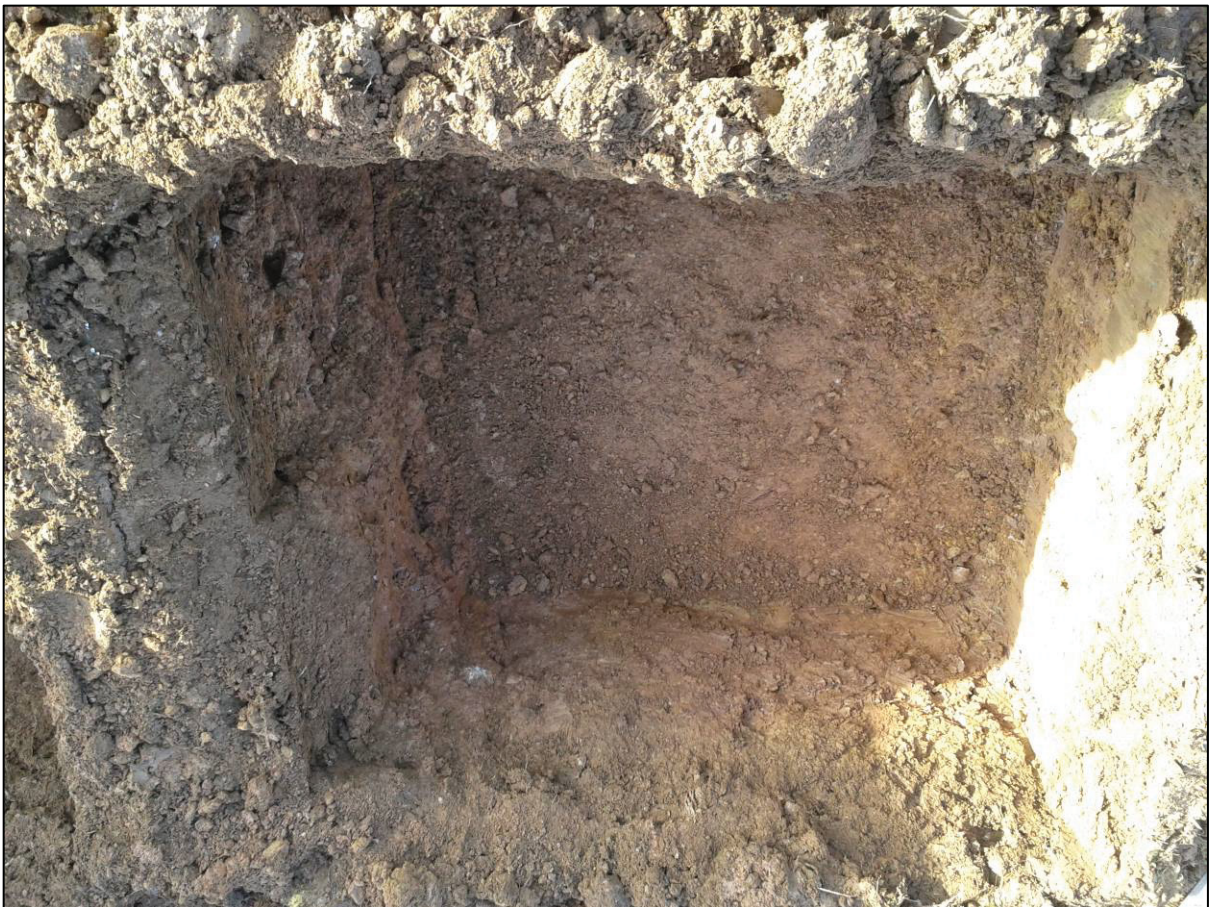
Figure 7: Field C inverter foundation pit
