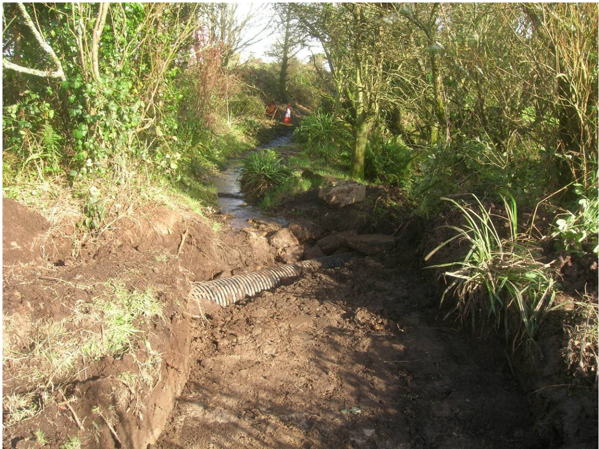
Fig 16 Insertion of the drainpipe to drain the ground upslope from the footpath and wells
