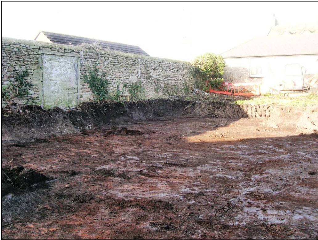
Figure 12. Overview of NW part of site after stripping.
