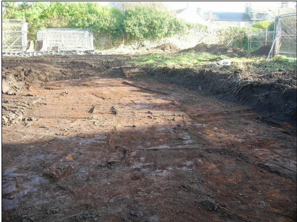
Figure 11. Overview of SE part of site after stripping
