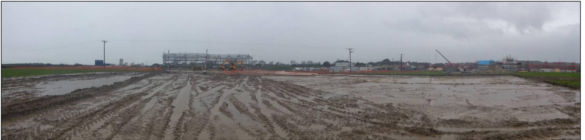
Figure 16: Overall view of excavation site post excavation (looking north).
