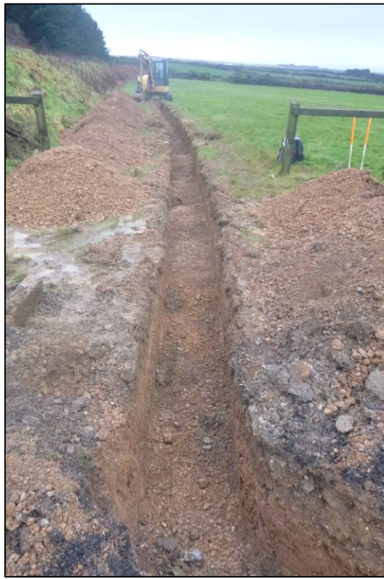
Figure 10: View of the cable trench (looking south)
