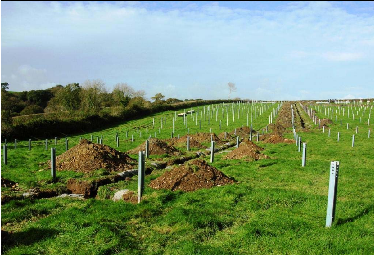
Figure 10 Image (from the south looking north) of field C after the main cable duct trenches were excavated and vertical posts forced into the ground © HE Projects, CC 5/11/2013.
