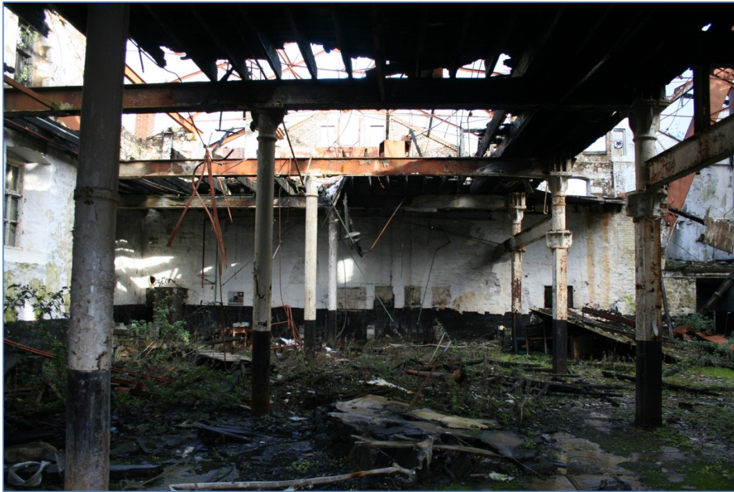
Fig 61 The interior of the old brewhouse (4), looking southeast. The cast iron pillars on the left are from Redruth Foundry.
