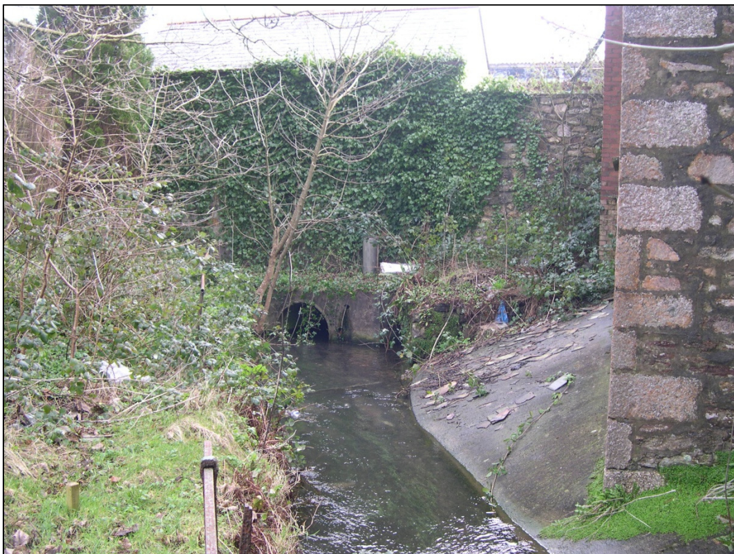
Fig 38 Brewery Leat running west past the corner of the historic brewhouse; the banks are now severely overgrown and the path and railings alongside the leat are hidden.
