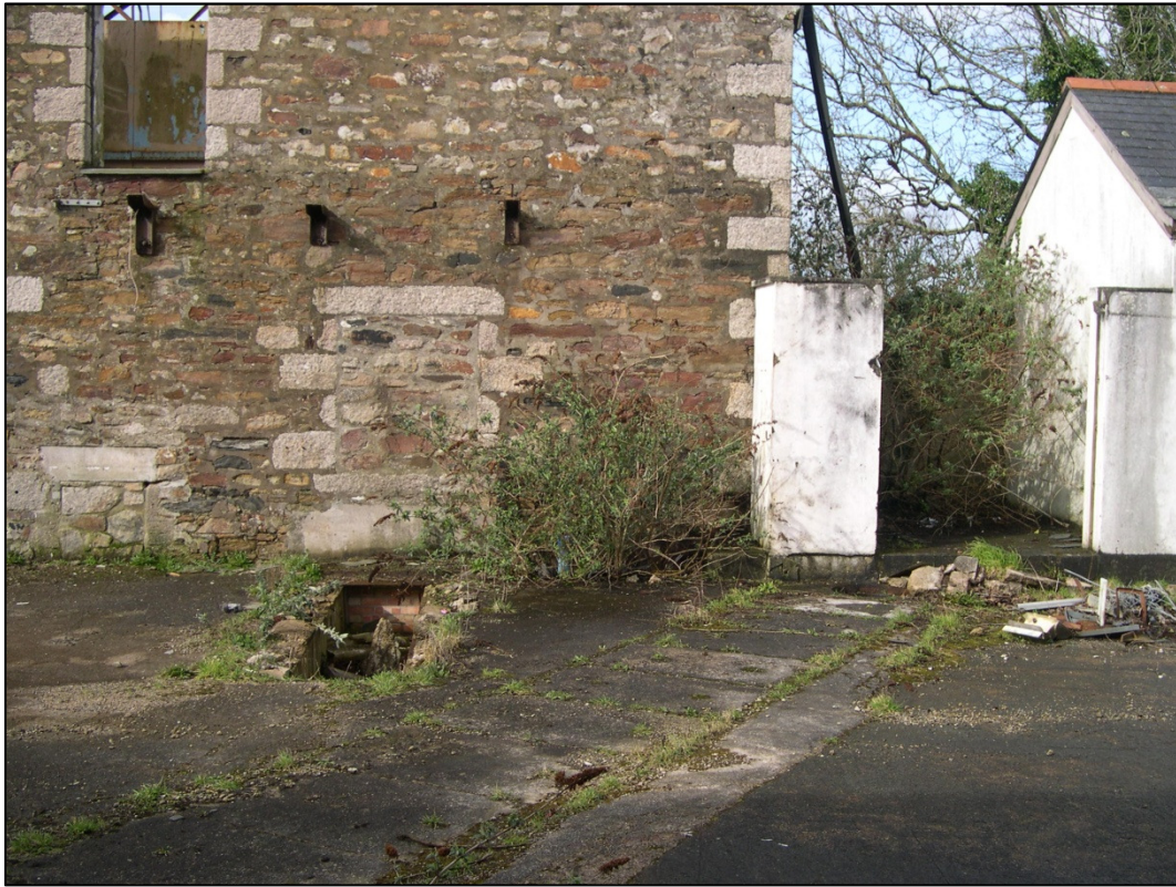
Fig 37 The historic route of Brewery Leat where it runs towards the corner of the historic brewhouse, currently paved over where it was used for electric conduit.
