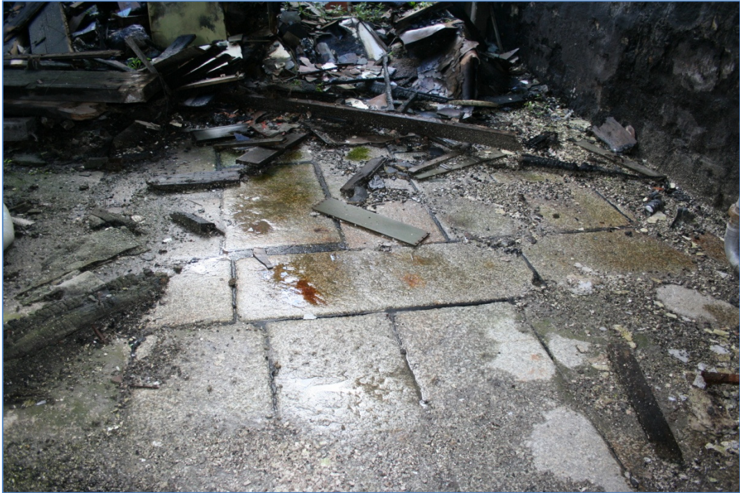
Fig 63 Granite paving covering the floor of the old brewhouse (Areas F, G and J).
