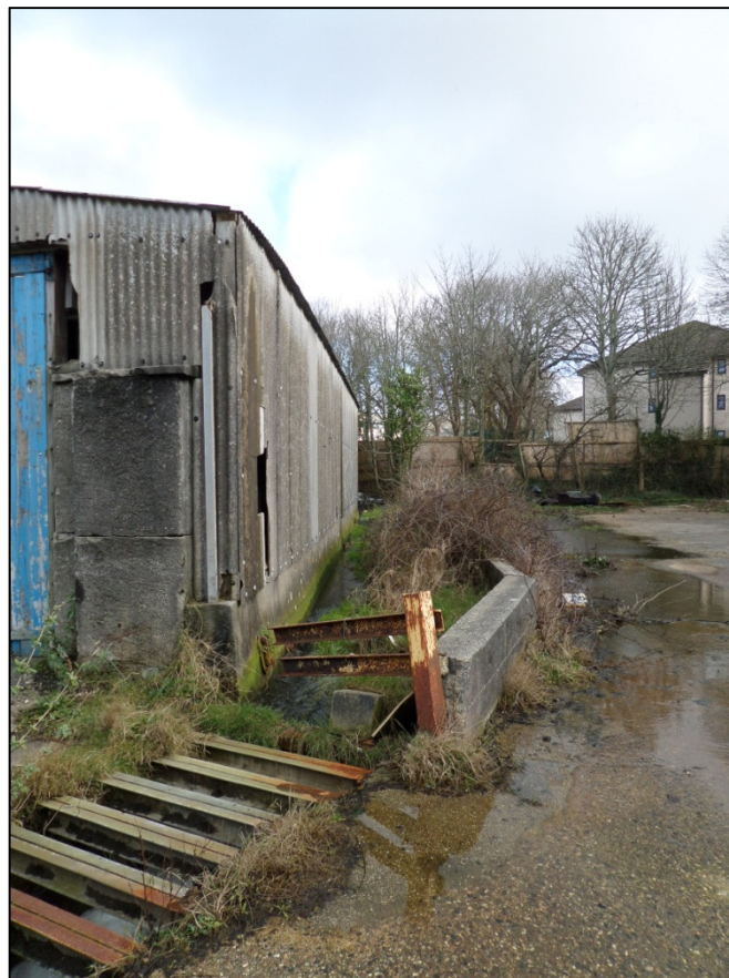
Fig 36 Brewery Leat feeding into the brewery site from the east. The leat drops away sharply beneath the iron grid and now runs northwest through a modern culvert.
