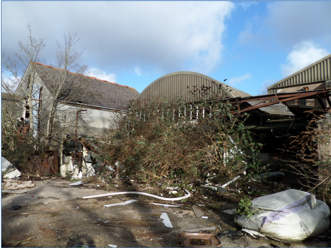
Fig 71 Looking east towards the 1950s building (19) with building (9) to the left. Both would originally have had curved roofing; the curved framework for the roof of building (9) survives in situ beneath its later pitched roofline.
