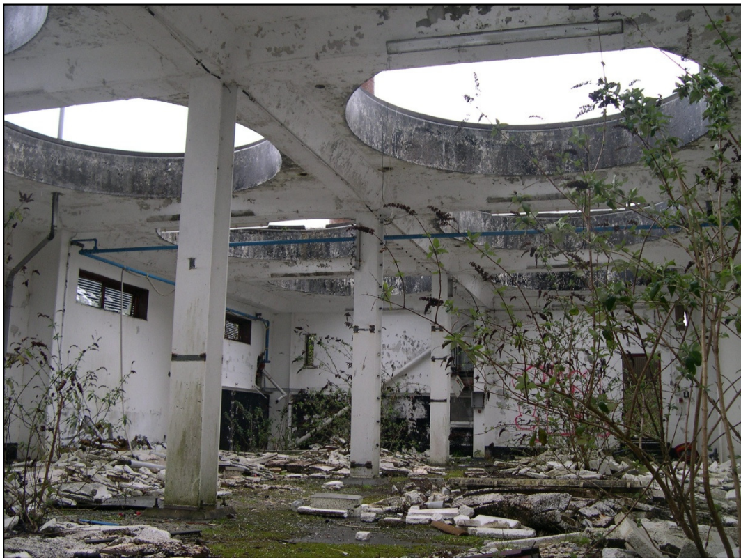
Fig 56 The surviving interior of a late 20 th century conditioning room (25). The circular vents left by the removal of the brewery vats lend a distinctive modern architectural character to this building, meriting its reuse within any planned redevelopment.
