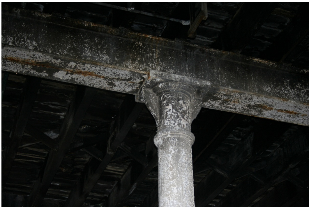
Fig 62 Closer detail of one of the cast iron pillars in the old brewhouse. The wooden floor of the upper storey retains much of its latticed support detailing.
