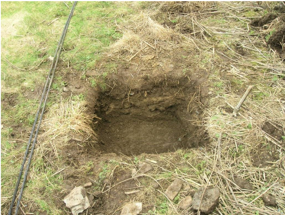
Figure 6. Trial Pit 1 after excavation looking south east showing section
