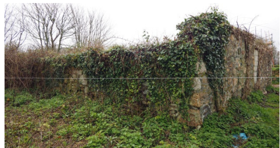
Fig 47 Remains of House 1 from NW
