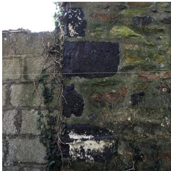
Fig 25 Barn D phase 3 NE corner (scoria blocks)
