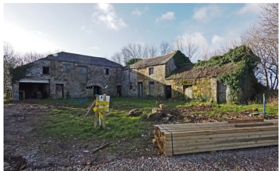
Fig 57 Context: Barns A and B, SW of farmhouse
