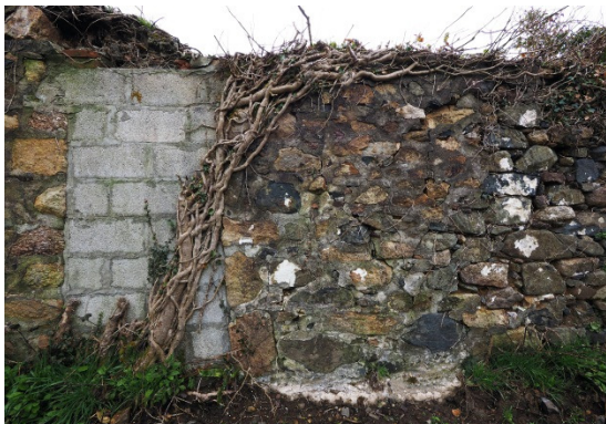
Fig 43 Remains of House 1 (blocked openings)
