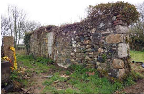
Fig 41 Remains of House 1 from SW
