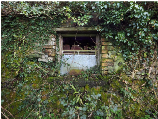
Fig 28 Barn D phase 2 rear window left
