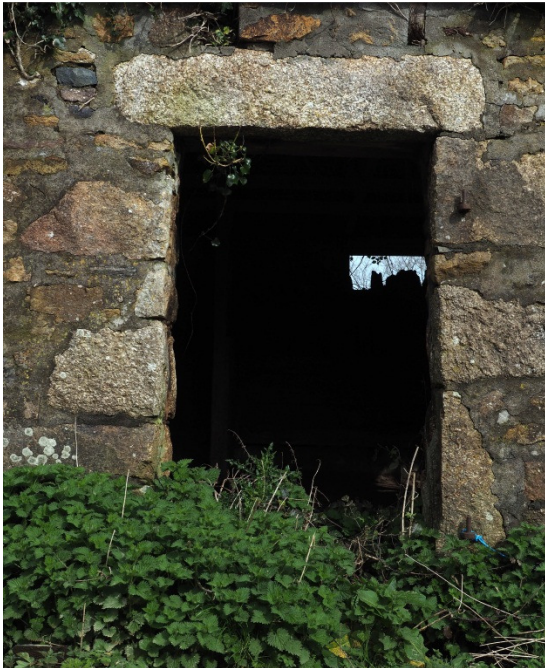
Fig 20 Barn D phase 2 central doorway
