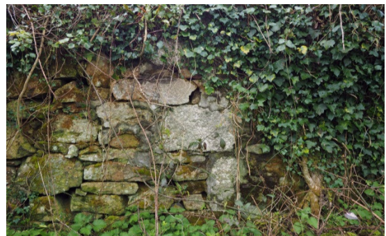
Fig 49 NW corner of House 1 extension from N
