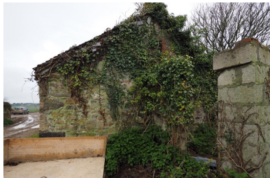
Fig 23 Barn D, E end (note gable vent)
