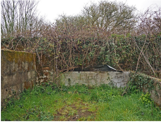
Fig 50 Part of shelter shed (and remains of house extension to left)
