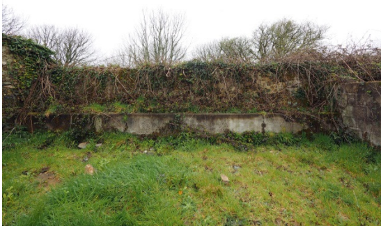
Fig 52 Rear wall of shelter shed
