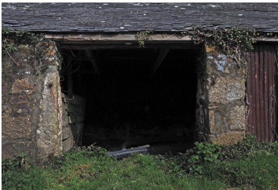
Fig 21 Barn D phase 2 front far right
