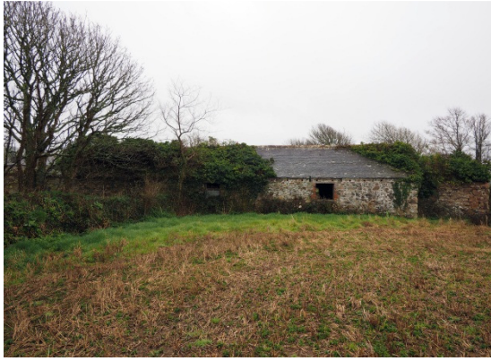
Fig 26 Barn D rear (north) elevation
