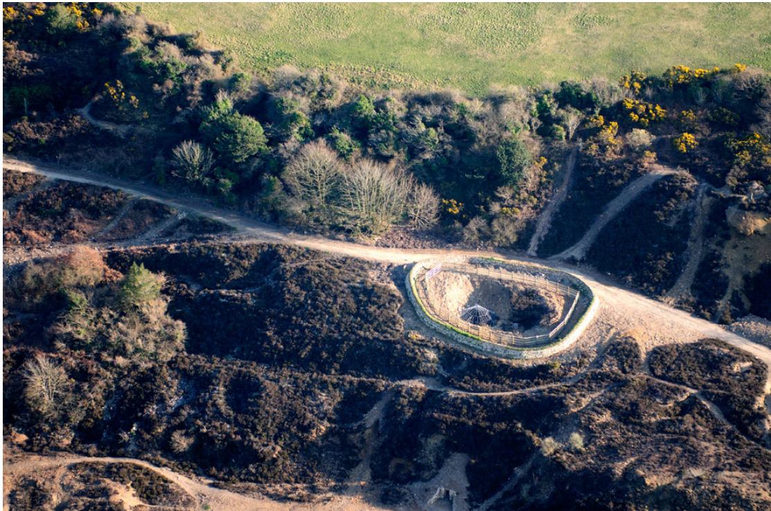
Figure 16. Works at West's Shaft, Wheal Fortune on the Mineral Tramways trail, showing coned shafts enclosed by a hedge and fence, and West's Adit portal, bottom centre. (F90-228)
