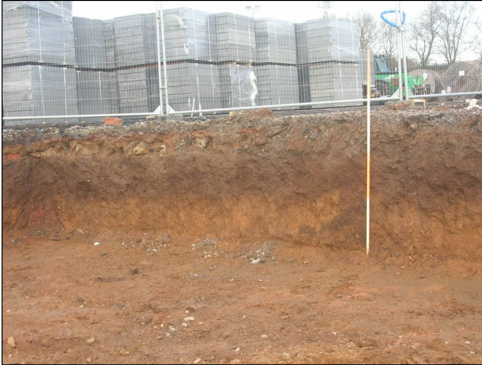
Figure 16. Attenuation tank. Sample of NE section showing nature of the ground.
