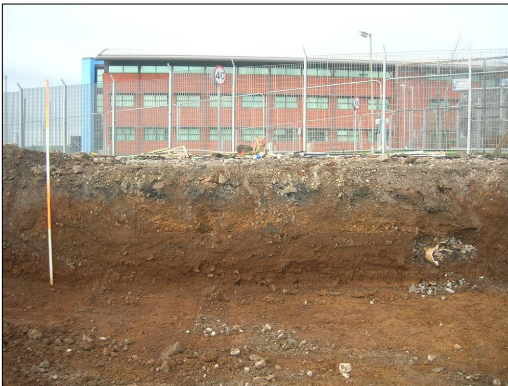
Figure 17. Attenuation tank. Sample of NW section showing nature of the ground.
