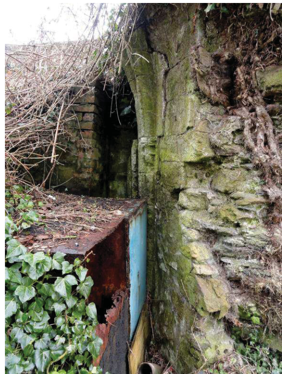
The wall with the oil tank to the left
