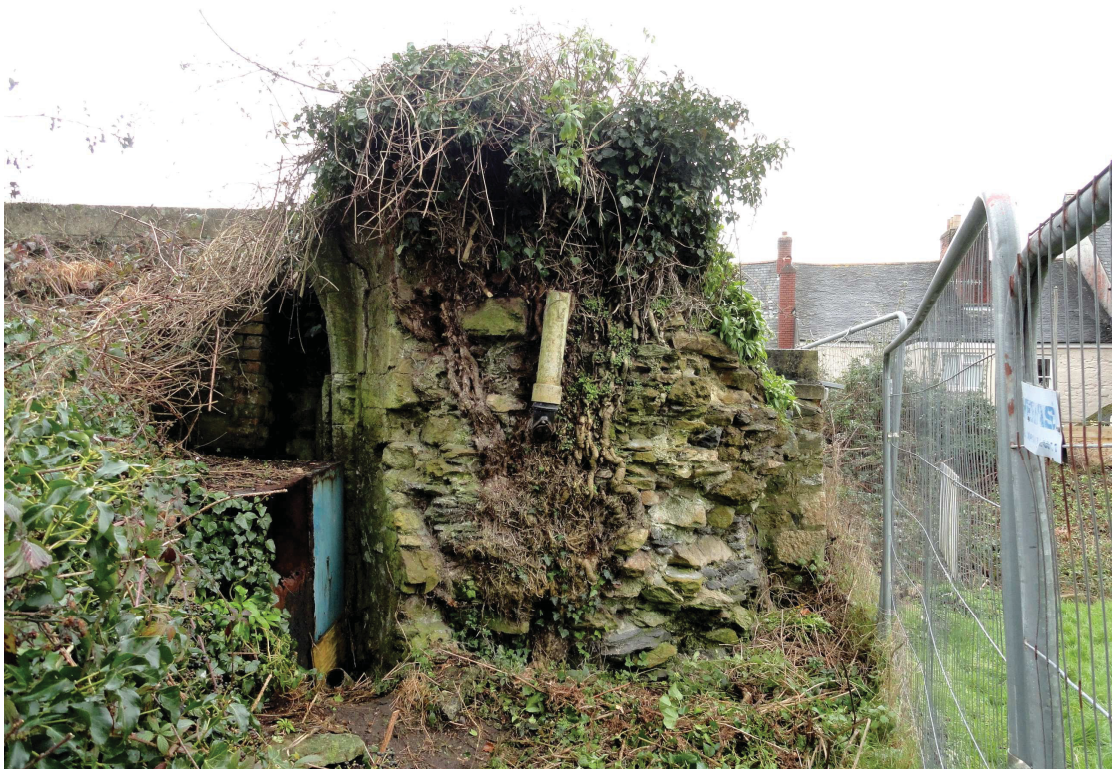
Fig 8 Photos showing the condition of the wall before conservation work. Above in 1987, courtesy of Barry Searle; below, in 2011 from behind the Heras security fence. The old oil tanks are visible on the left, and the security fence separating the wall from the playing field is on the right. In the centre, the stove pipe can be seen emerging from the wall, which has a thick thatch of ivy
