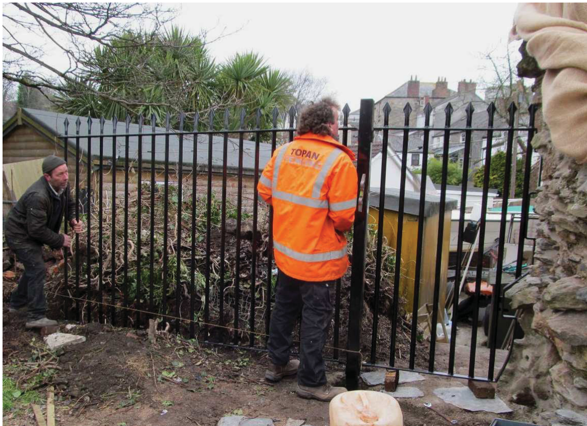
Fig 16 Ian Wilton and Fred Hooper installing the new fence in March 2013
