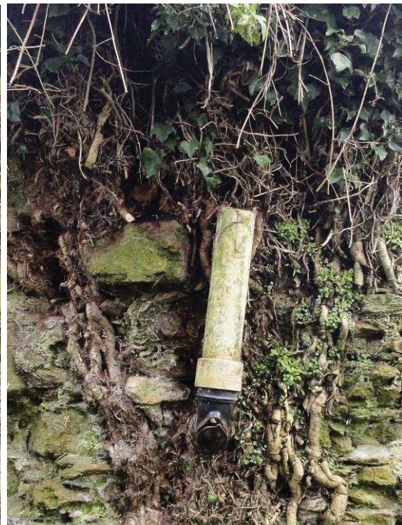
The carved window arch, showing cracking due to ivy penetration and (right) the stove pipe emerging from a putlog hole. Both also show the extent of ivy roots on the wall
