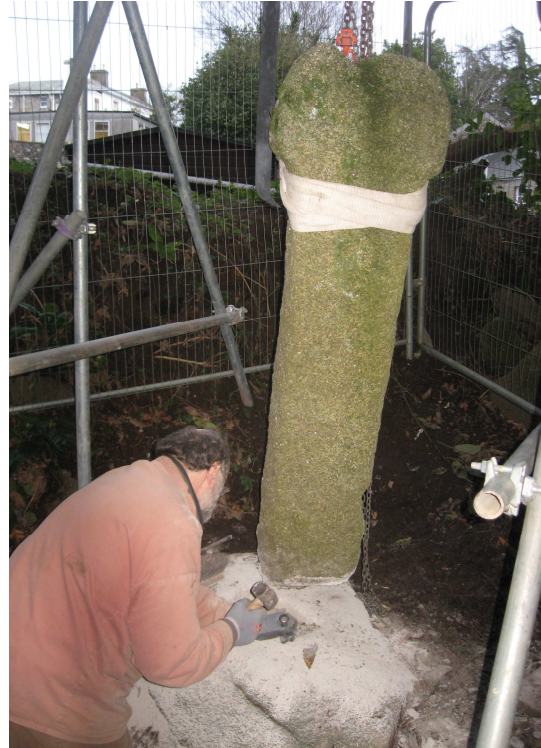
Fig 8 Lawrence Kelland chipping away the cement mortar from the base of the cross in order to remove it from its base at Pendean
