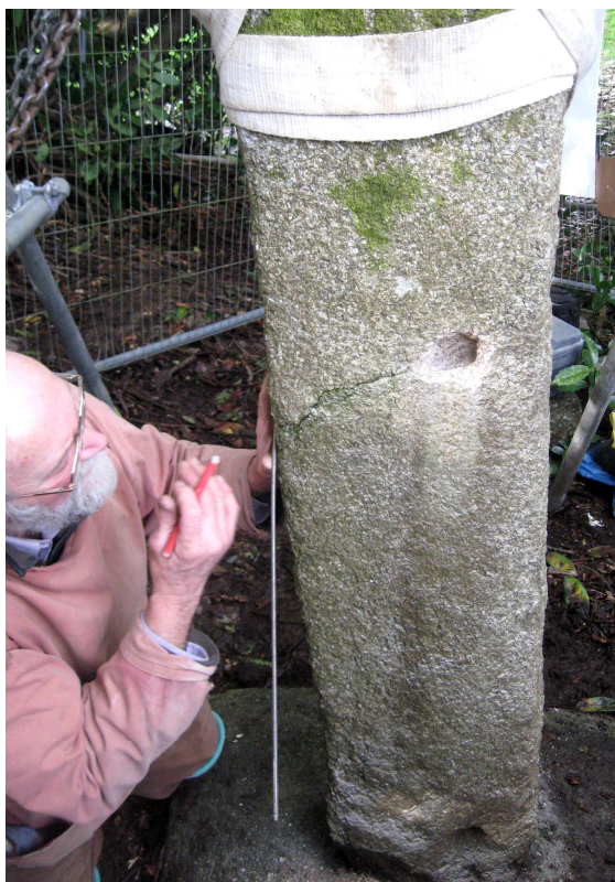
Fig 6 Lawrence Kelland removing the iron fixing from the cross-shaft
