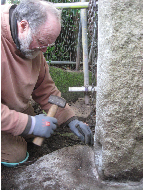
Fig 8 Lawrence Kelland chipping away the cement mortar from the base of the cross in order to remove it from its base at Pendean
