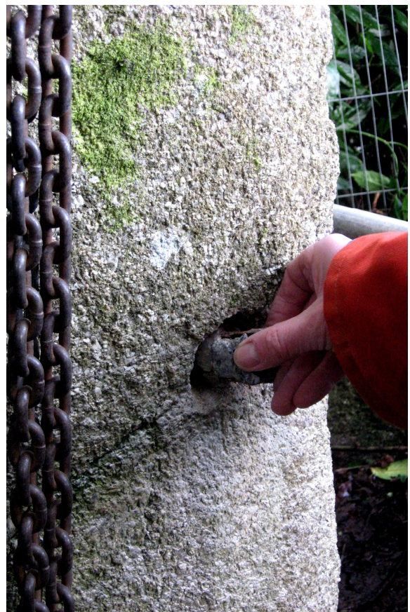
Fig 6 Lawrence Kelland removing the iron fixing from the cross-shaft
