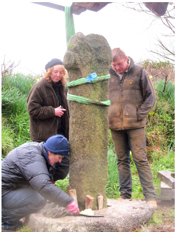
Below left: Sue Kelland fixes the stone in its base with stones and resin, watched by Angela Redman and Toby Roger
