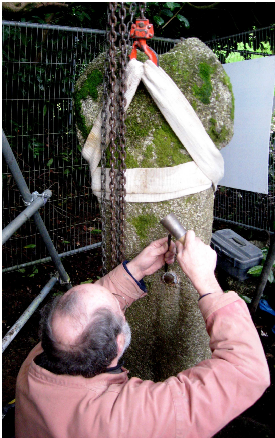
Fig 6 Lawrence Kelland removing the iron fixing from the cross-shaft
