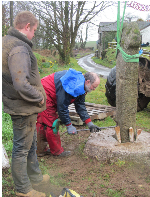
Above right: Tractor driver Toby Roger and Lawrence Kelland securing the cross in its base
