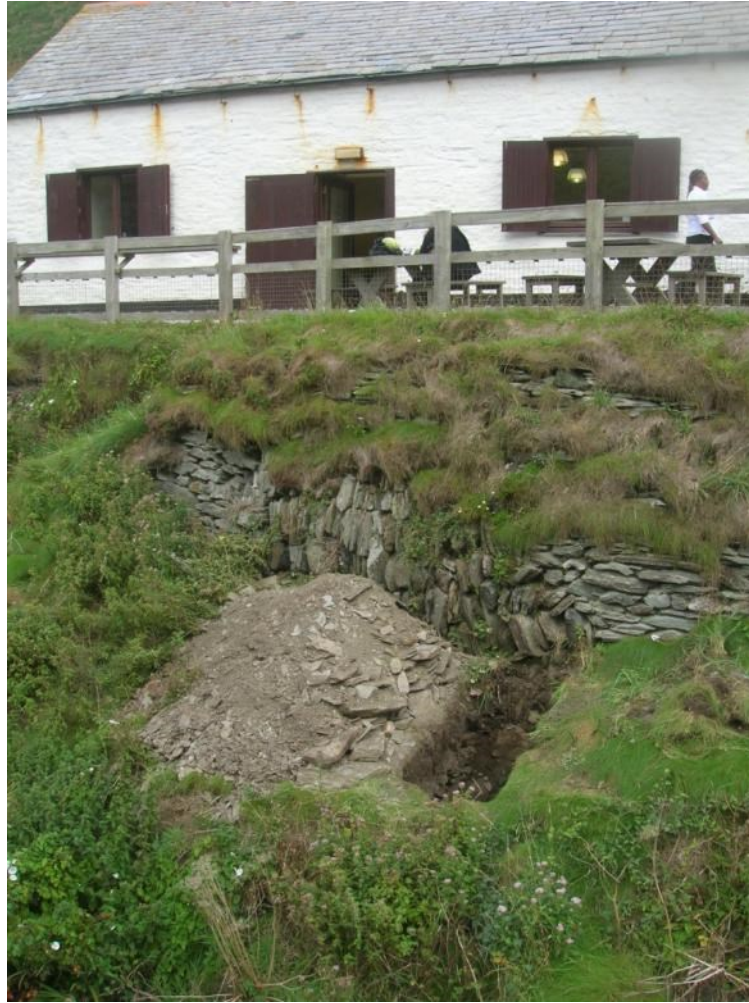
Figure 8. Trial Pit 1. Excavated trench showing location, looking northeast..
