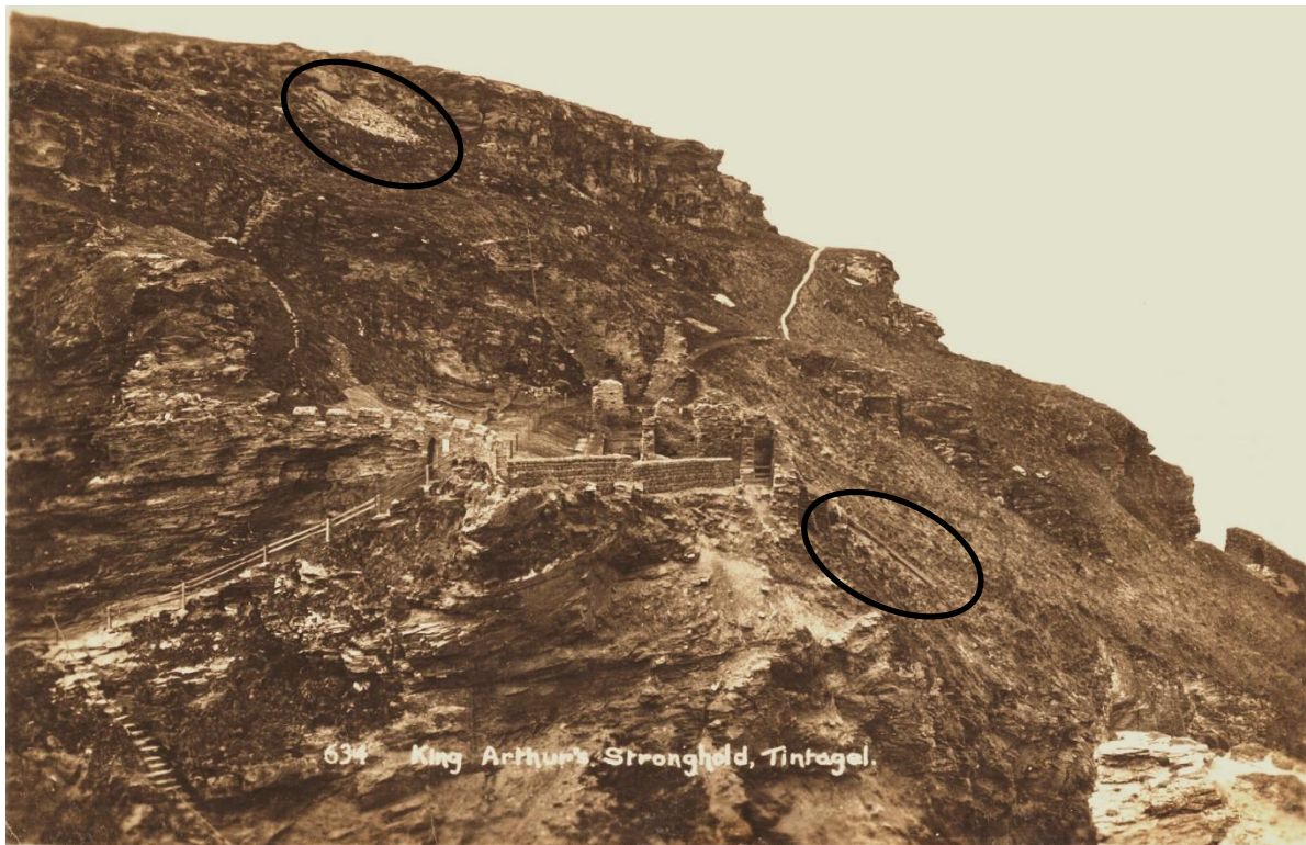
Fig 20. A postcard which is likely to date to the early 1930s showing the short-lived cliff-edge barrier constructed between Kinsman's wall and the eastern curtain wall, as well as excavation spoil from the chapel (circled, left of centre, top) and a wooden rubble chute (circled, on the slope to the right of the Great Hall).
