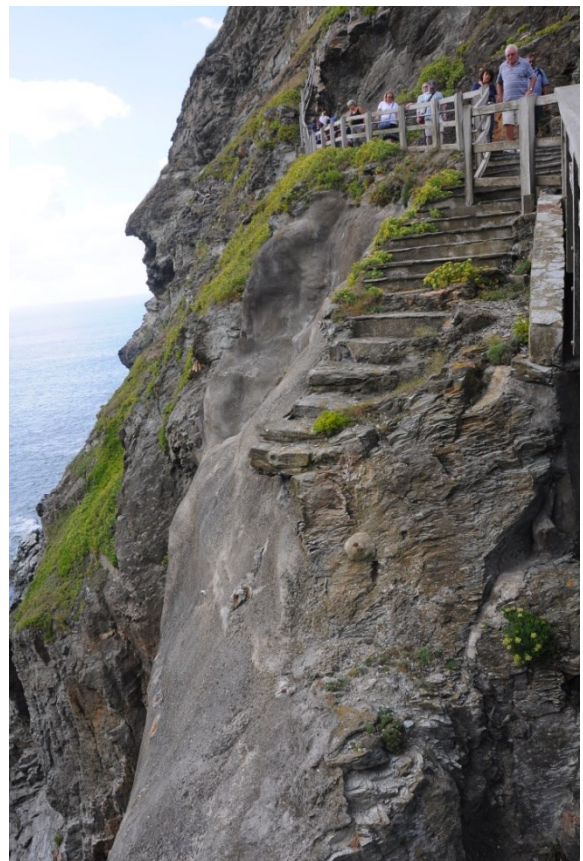
Fig 28. And the existing steps are also rather prone to being lost to erosional processes – whether maritime, or through the collapse of the rock on which they were built.
