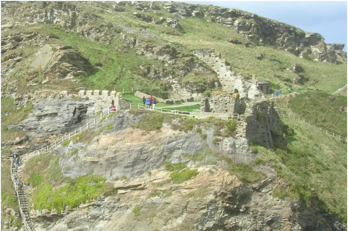
Fig 22. A broadly equivalent modern view to that shown in Fig 21. The cliff slope below the Great Hall has been meshed and rock bolted. A further metre of Kinsman's wall has collapsed since the earlier postcards were produced.
