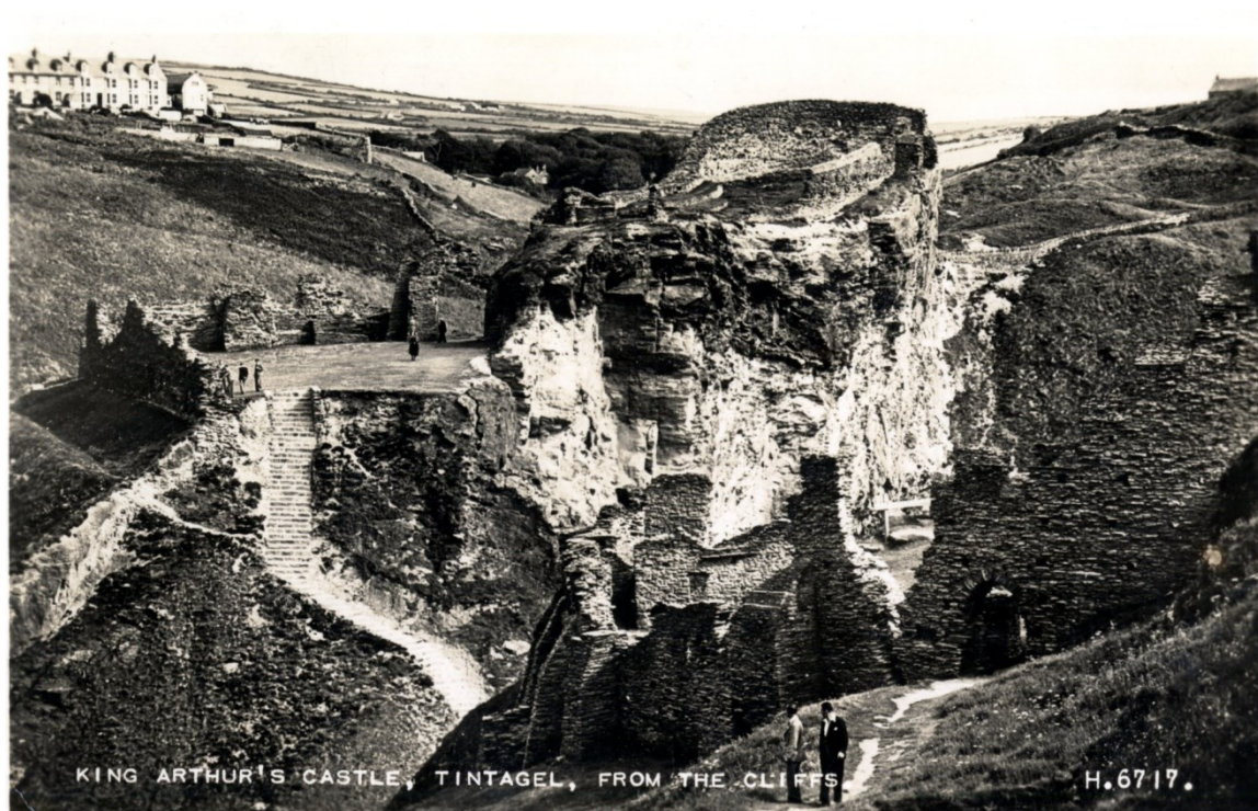
Fig 15. An early 20 th C postcard, showing the flight of steps constructed to give access from the Lower Ward down to the path across the neck and on to the Island. Note that the wall across the northern end of the Lower Ward had by this time gone.
