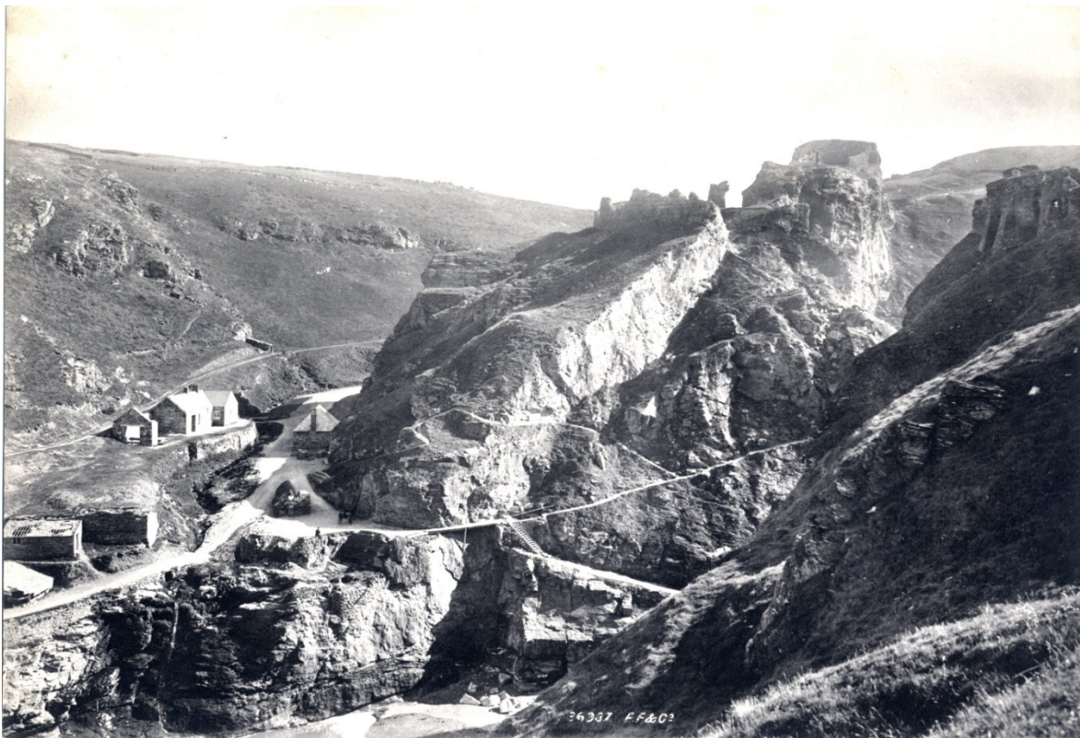
Fig 13. Another Frith postcard showing access arrangements from the valley base. The higher paths routes led to the neck and the cliff path up to the Island.
