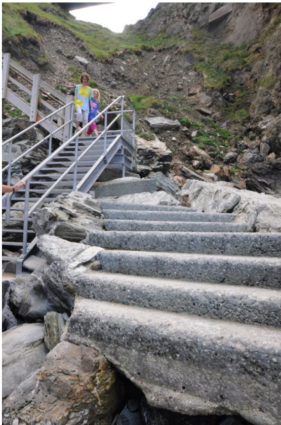
Fig 28. And the existing steps are also rather prone to being lost to erosional processes – whether maritime, or through the collapse of the rock on which they were built.
