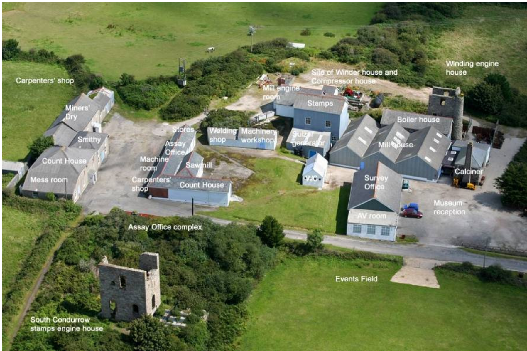
Figure 2 A HES aerial photograph (2009) of King Edward Mine with building functions labelled (before the horizontal steam engine winder and compressor house was rebuilt).
