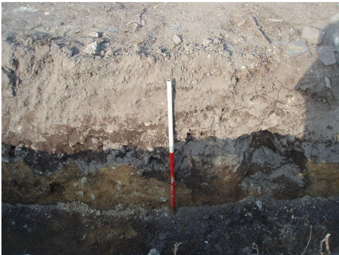
Figure 8: A sample, south-west facing, section of the foundation trench showing the greater depth of the topsoil at the south-western end of the new house.
