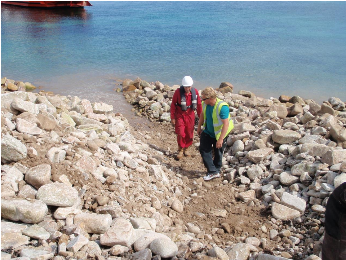
Fig 5 The cable trench at Pendrathen, St Mary's, Monday 21 July.
