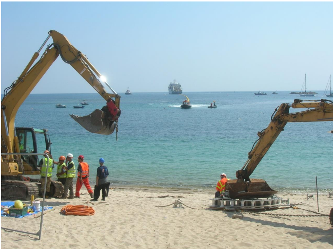
Fig 8 The cable being brought ashore at Porthcressa, St Mary's, Wednesday 23 July.
