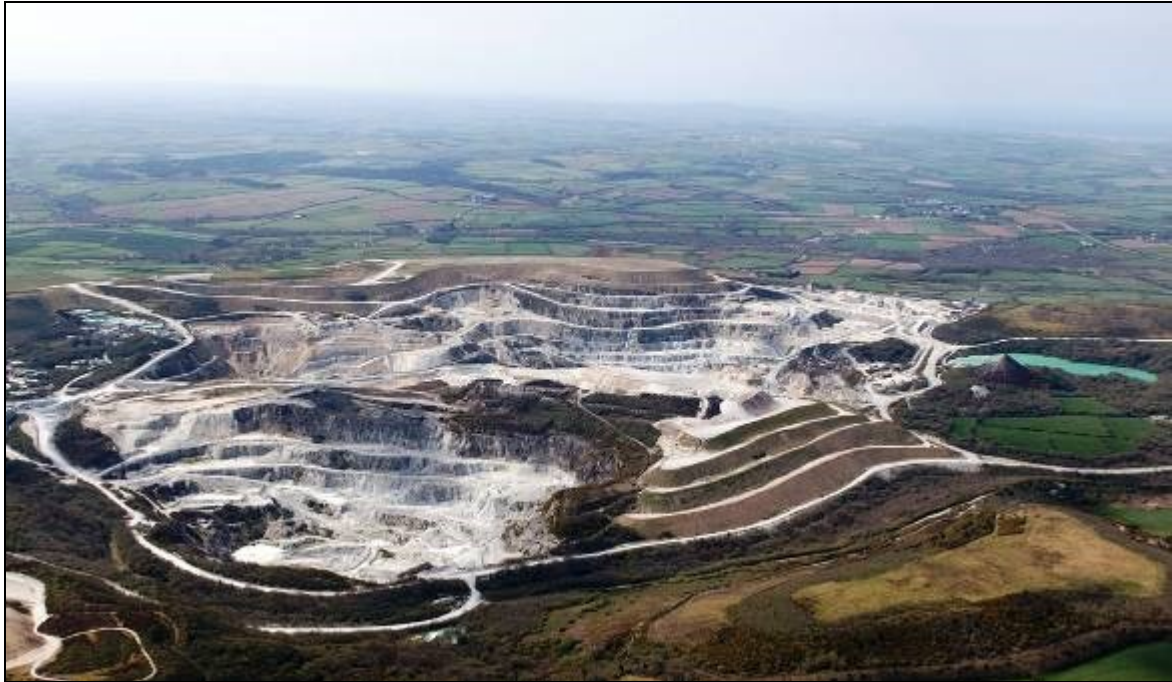
Figure 25 The Melbur, Wheal Remfry and Virginia clay operations from the air in 2008. The differences between modern working and that of even the relatively recent past are highlighted by the contrast in scale and form between the modern Virginia and Melbur clay works (centre and left) and the vegetation-cloaked sky-tip and flooded pit of New Halwyn clay works at right (cf Fig 24). (Photograph: Historic Environment, Cornwall Council: F82-013; 16 April 2008.)
