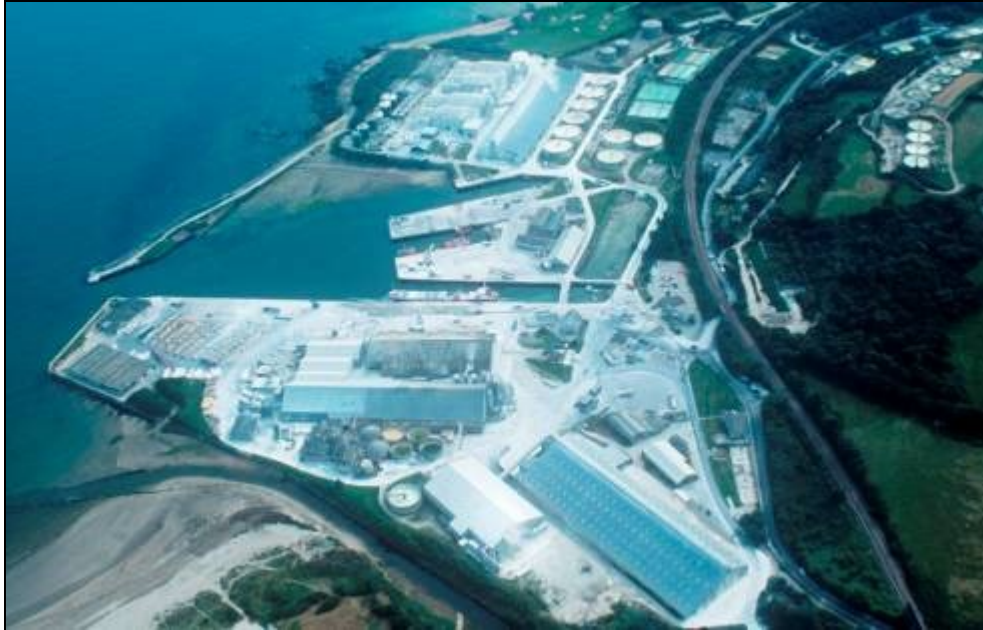
Figure 5 Par Docks, opened as a mineral port in 1840, equipped for mechanised drying after World War II and with major investment in the 1960-80s to expand shipping and processing facilities (Bowditch 2013). Much of the clay was brought by pipeline. (Photograph: Historic Environment, Cornwall Council; ACS 5983, 7 August 2003.)
