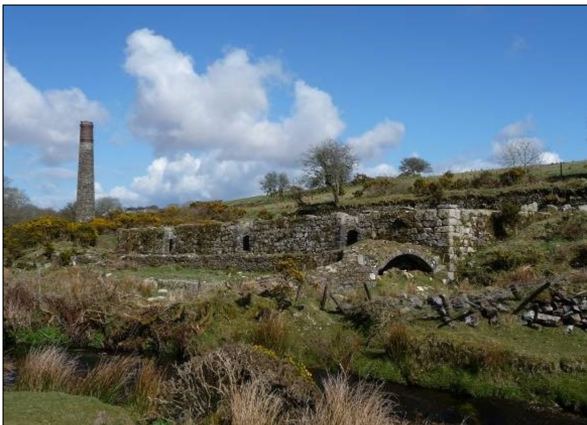
Fig 101 The surviving clay kiln and stack at Heneward, Bodmin Moor, part of a small working begun in the 1870s but substantially redeveloped during subsequent phases in 1913 and then during the 1920s and 1930s. The remains were assessed for Listing in 2011 but 'failed to meet the required criteria' (Pastscape record: Heneward china-clay works). (Photograph: Graeme Kirkham.)
