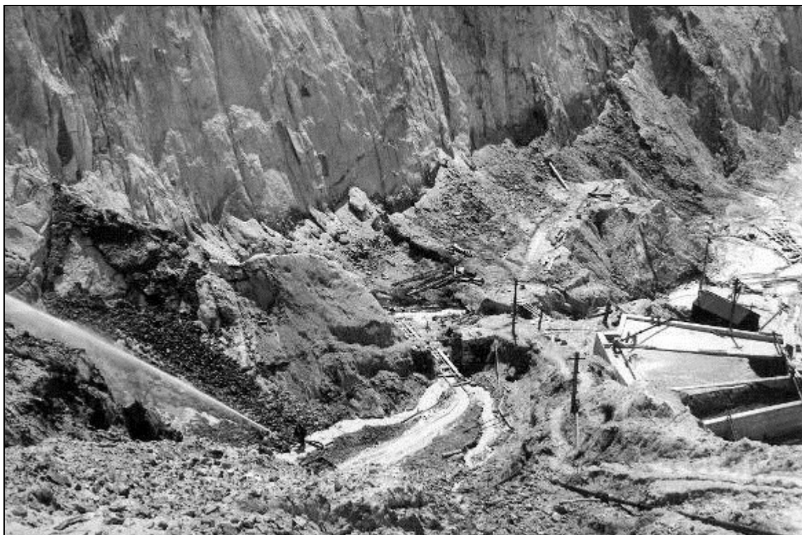
Figure 34 High-pressure water power in use to remove clay at Great Beam clay works (undated). (Photograph: China Clay History Society archive, 45658.)
