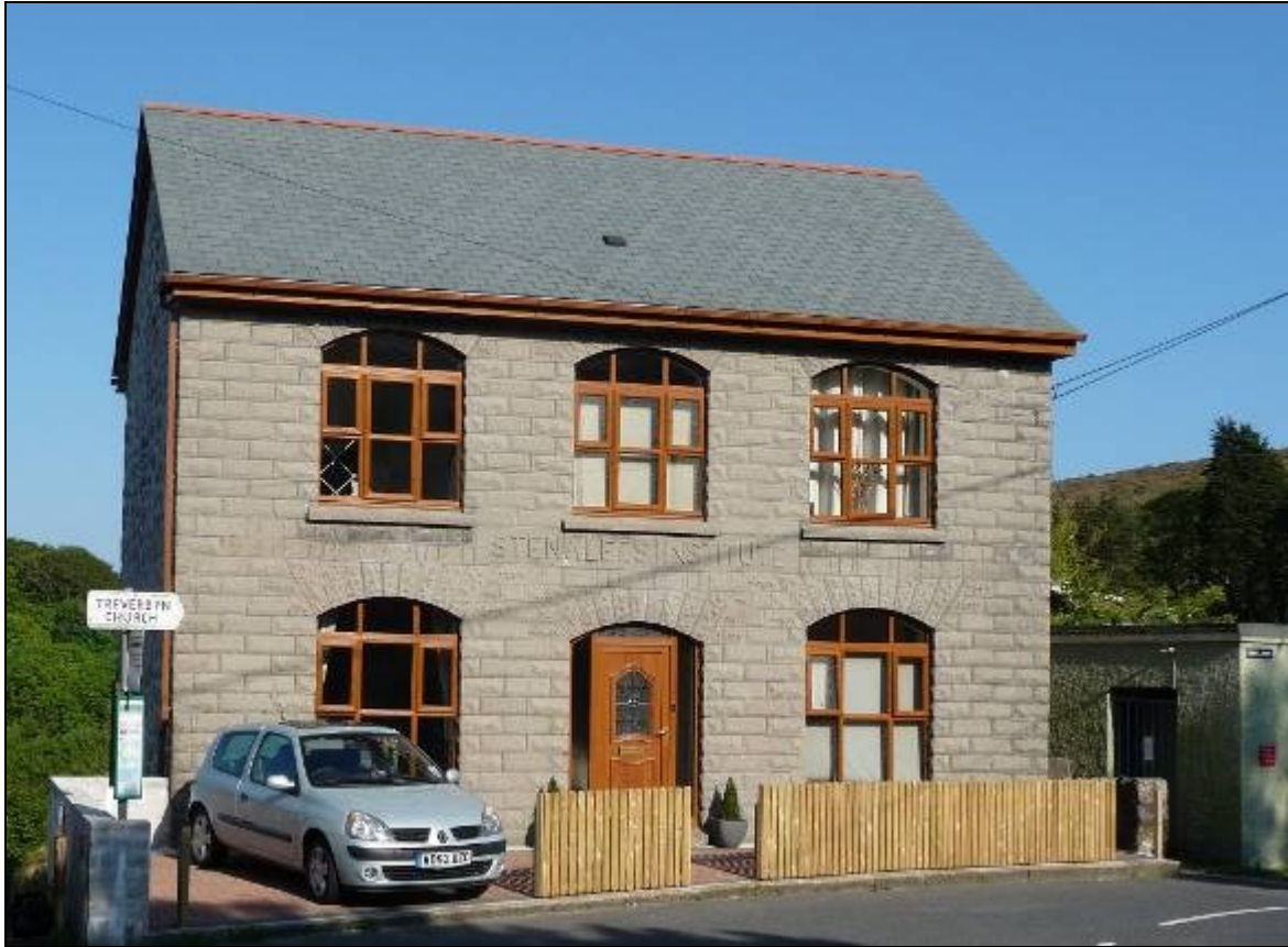
Fig 109 The former Stenalees Institute was highlighted in the Cornwall Industrial Settlement Initiative (CISI) report on Stenalees: ' . . . one of the most interesting buildings in the whole area. It is a neat, well-designed little building standing in a prominent position at the central junction in the village, made of concrete blocks, but richly decorated with cast patterns of rustication, fleur-de-lys, and lettering – an example of what could be achieved with what is usually considered a poor-quality facing material' (Cahill Partnership and Historic Environment Service 2005, 21-2). The building has subsequently been altered for domestic use. (Photograph: Graeme Kirkham.)
