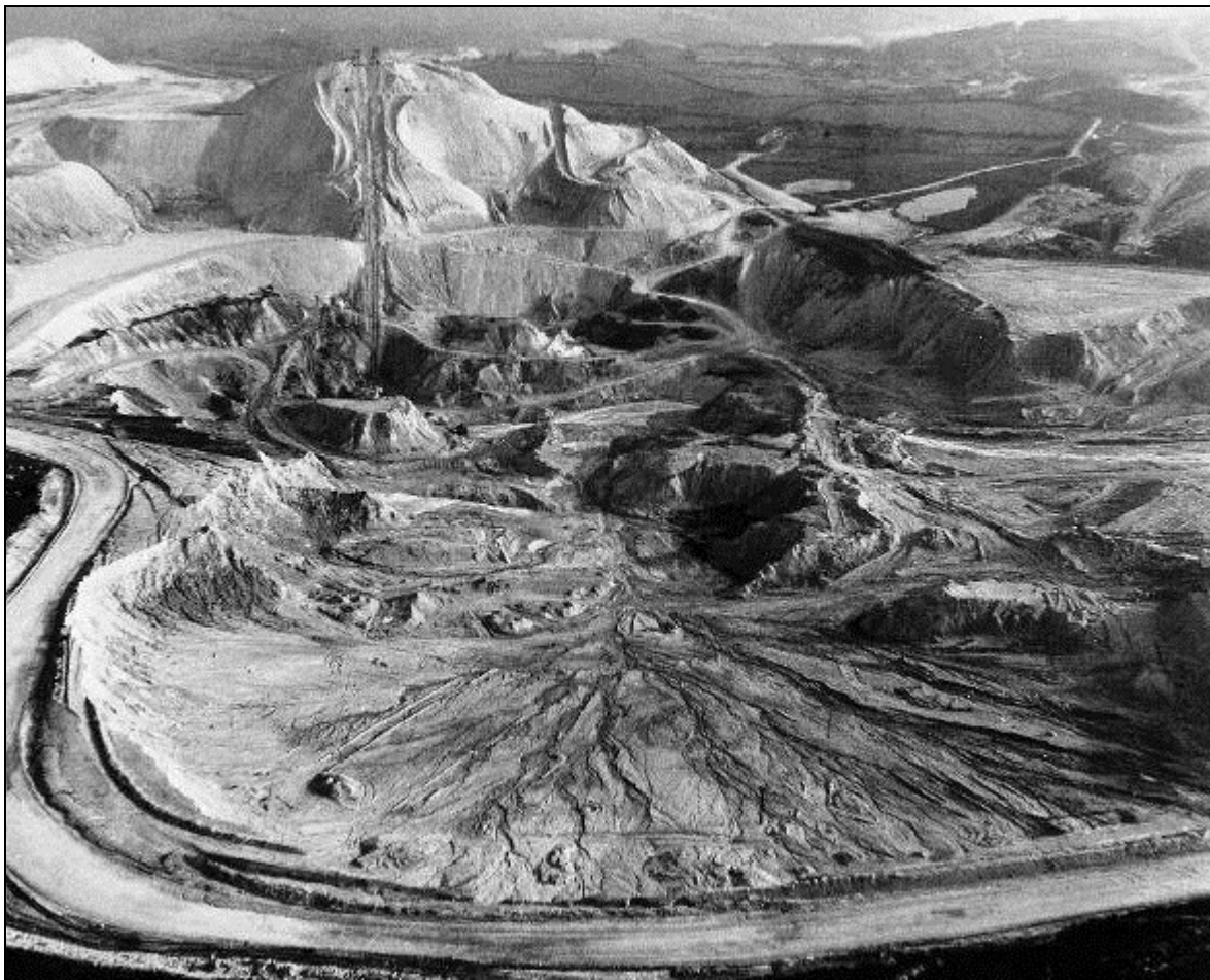
Figure 30 Whitehill Yeo pit, on south-west Dartmoor, from the north, with a double incline mounting a waste tip; July 1971. (China Clay History Society archive, 17218.)
