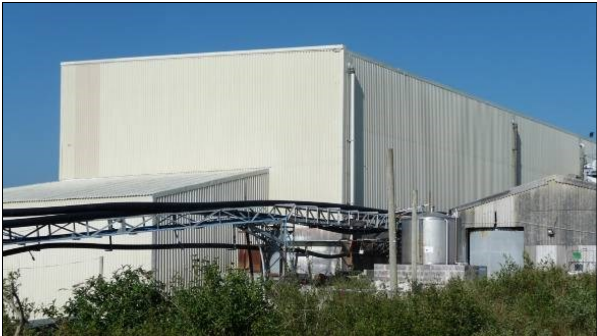
Figure 69 Industrial buildings and installations at the Greensplat pit complex. (Photograph: Graeme Kirkham)
