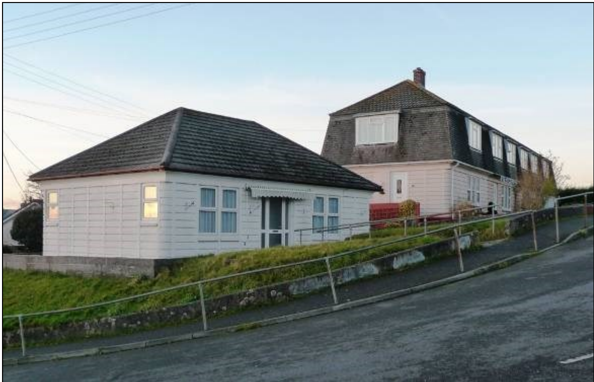
Figure 23 Post-World War II 'Cornish units' at Chegwyns, Foxhole, including an unusual single-storey type. The 'units' were prefabricated using china-clay waste. (Photograph: Graeme Kirkham.)
