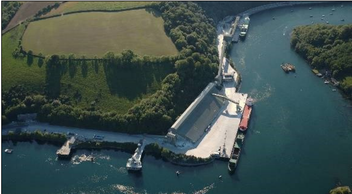
Figure 31 China-clay wharves and jetties at Fowey. A large proportion of clay production is now shipped by this route. (Photograph: Historic Environment, Cornwall Council: F67-059; 8 June 2005.)
