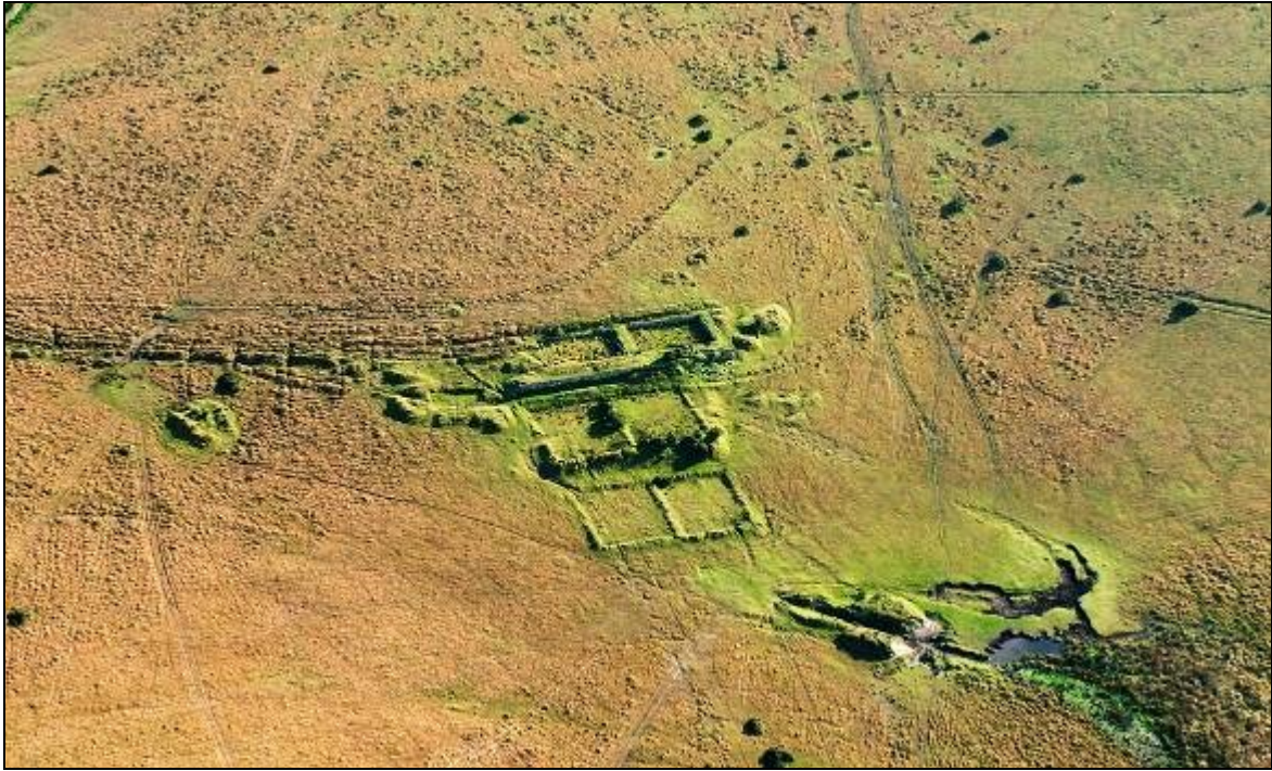
Figure 98 A complex of settling tanks and leats or liquid clay channels on Greenbarrow Downs, near Temple, on Bodmin Moor. These were shown as 'disused' on the 1st edition Ordnance Survey 25in map of c 1880 and represent an early phase of china-clay working in the Temple area (Smith 2008b, 115). (Photograph: Historic Environment, Cornwall Council, F100-164; 16 October 2010.)
