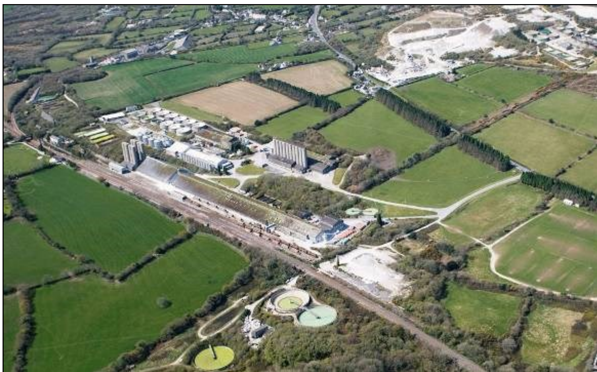
Figure 33 Blackpool dryers, refinery and pit at Burngullow, the site of a proposed 'eco-community'. The first phase of the processing complex, located alongside the Great Western main line, adjacent to the junction with the important mineral branch line to St Dennis, dates to the late nineteenth century. The site was the focus for major investment in new clay processing technology in the 1960s and 1970s, at which time the distinctive belts of evergreens screening the site from view from the St Austell – Newquay road were also planted (Bowditch 2013). The Blackpool complex lies over the sites of the former manorial centre of the manor of Burngullow and the medieval farm settlement of Methroes in an area of Anciently Enclosed Land. The potential for buried archaeology around the site is likely to be high. Beyond the St Austell – Newquay road to the north is an area of Recently Enclosed Land taken in from rough ground in the post-medieval period. (Photograph: Historic Environment, Cornwall Council: F82-075; 16 April 2008.)
