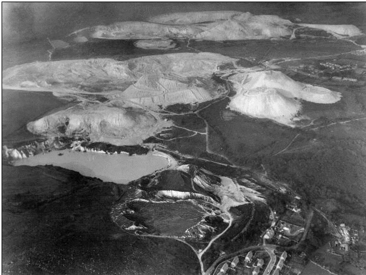
Figure 68 A dynamic industrial landscape expanding across rough ground on south-west Dartmoor in 1971, looking east from Wotter (foreground) towards Lee Moor, Whitehill Yeo and Cholwichtown. Tipping from the modern Lee Moor clay working has subsequently expanded to cover the area between Wotter and Lee Moor and the road linking them visible in the middle ground no longer exists. (Photograph: English China Clays, by courtesy of Dartmoor National Park.)
