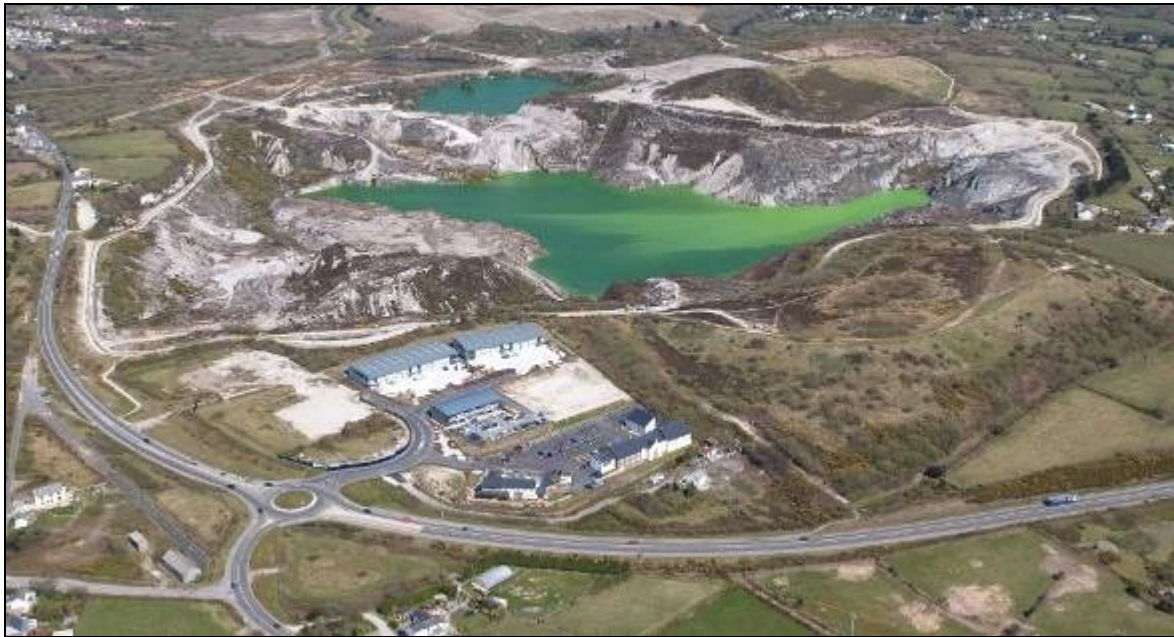
Figure 106 Great Carclaze (Baal) pit. The site was renowned in the eighteenth and nineteenth centuries as an unusual open-cast tin working on a vast scale and subsequently became a major china-clay operation. It is currently one of the six proposed 'eco-community' sites in the St Austell china-clay area, with proposals for significant housing and industrial development in and around the pit. Some development (foreground) has already taken place on the former Carclaze Downs, alongside the enhanced through route of the St Austell North-East Distributor Road. (Photograph: Historic Environment, Cornwall Council, F82-079; 16 April 2008.)
