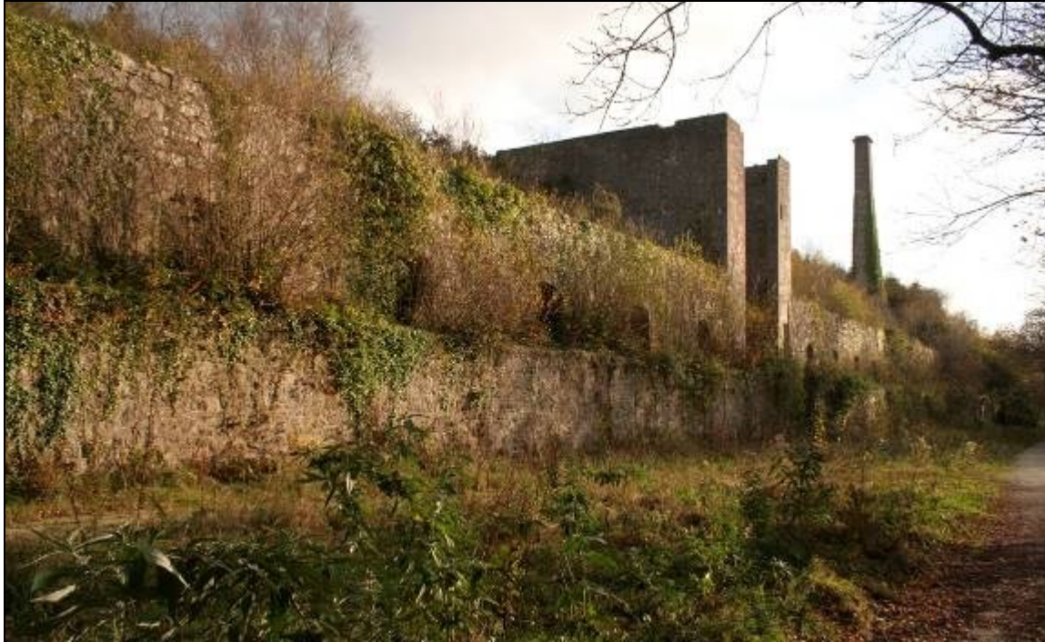
Figure 78 Carlyon Farm clay dry, in the Trenance valley, near St Austell, was constructed in 1921, soon after construction of a branch line up the valley from the Great Western main line. It was the largest dry ever built and combined two kilns in a single building. The structure is a Grade II Listed Building. It was recorded in advance of proposed conversion, with recommendations for further mitigation (Taylor 2008). (Photograph: Cornwall Archaeological Unit, Cornwall Council.)
